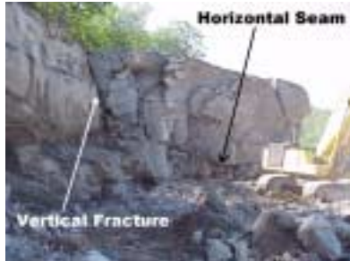
Figure 24: Horizontal seam and vertical fracture
