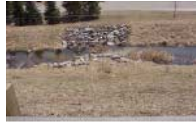
Figure 44: Test boring wash water emerging at base of embankment
