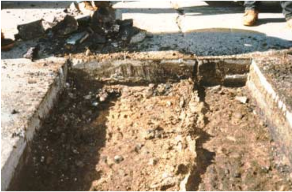
b. Site 1 – surface of base course during pit excavation.
