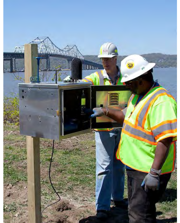
Installation of an environmental monitoring station at Losee Park in Tarrytown, N.Y.
