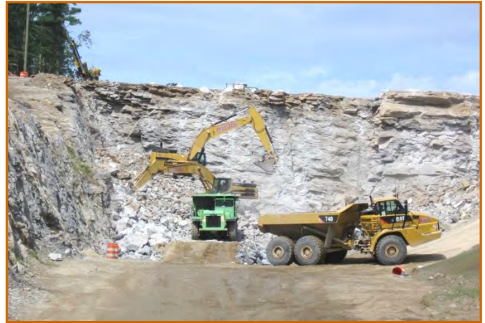
BLASTING & LEDGE/ROCK REMOVAL OPERATIONS
