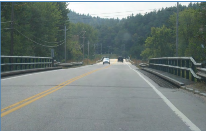
The Bearcamp Bridges on NH Route 16
