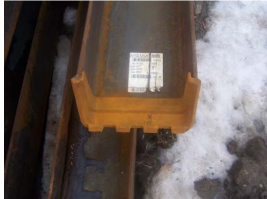
Pile Point K before driving
