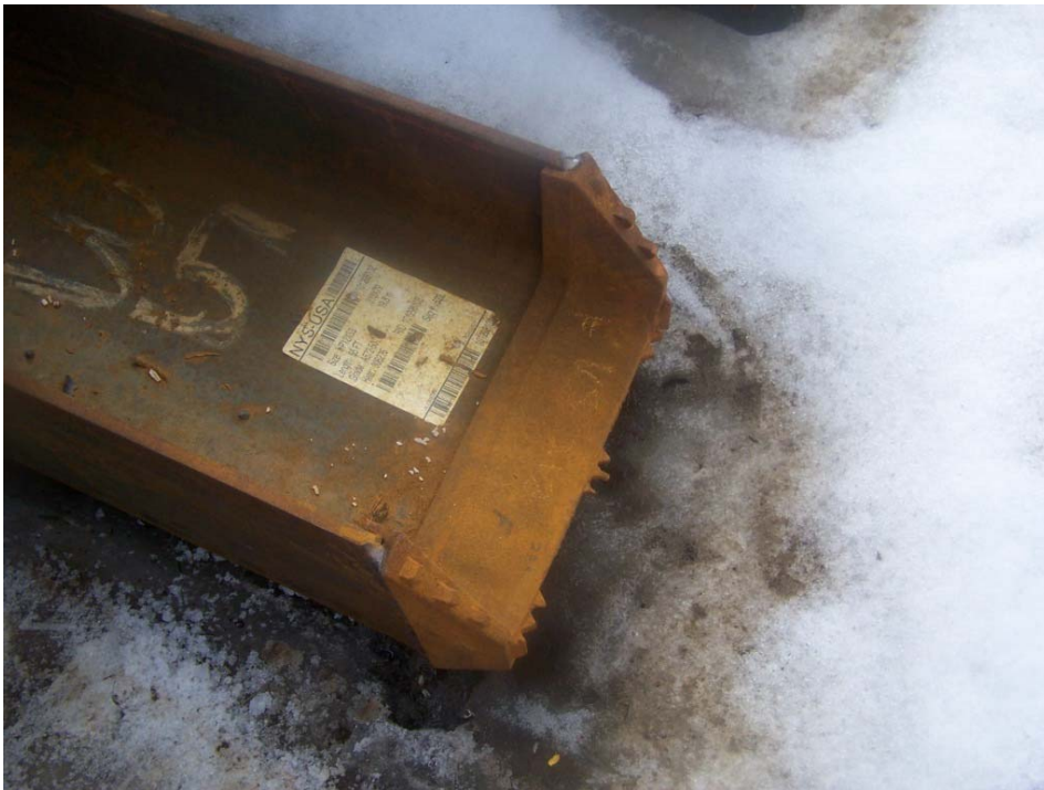
Pile Point F before driving – Note the position of teeth on the web portion
