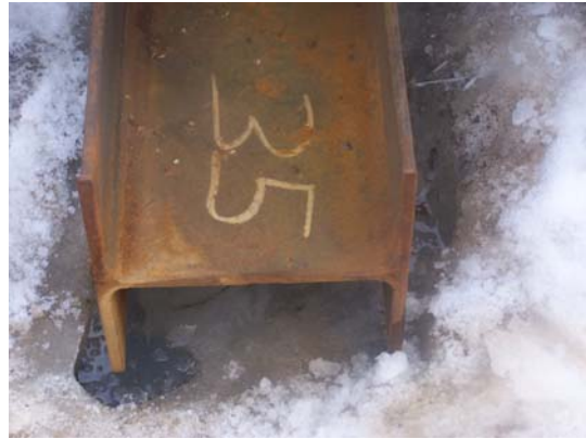
Control Pile Before Damage
