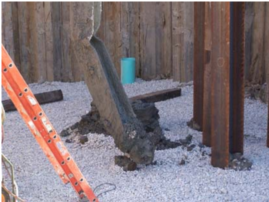
Pile F upon extraction
