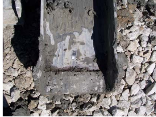
Pile Point E
