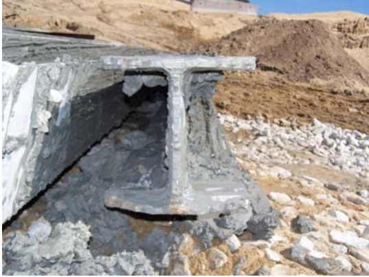
Pile Point D
