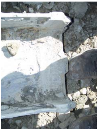
Pile Point I
