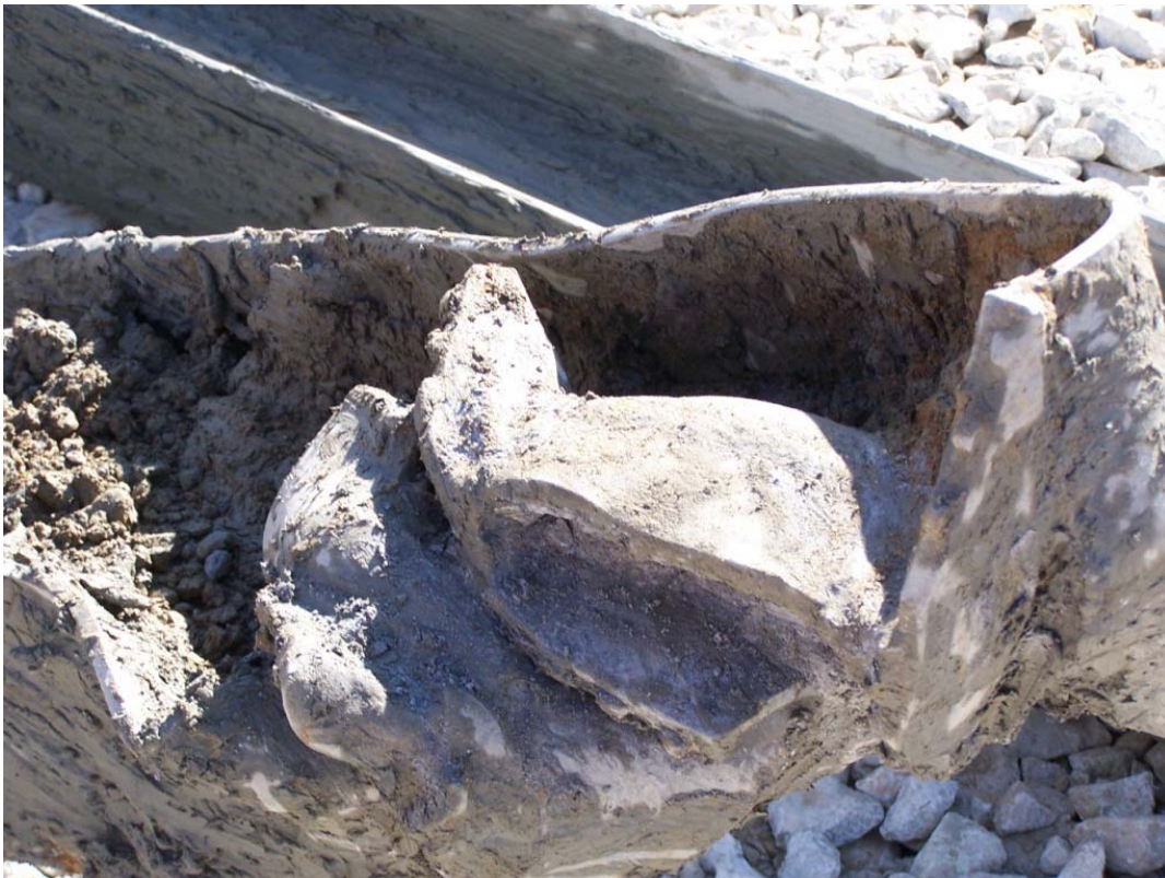
Pile Point F – Note pulverized rock particles on point
