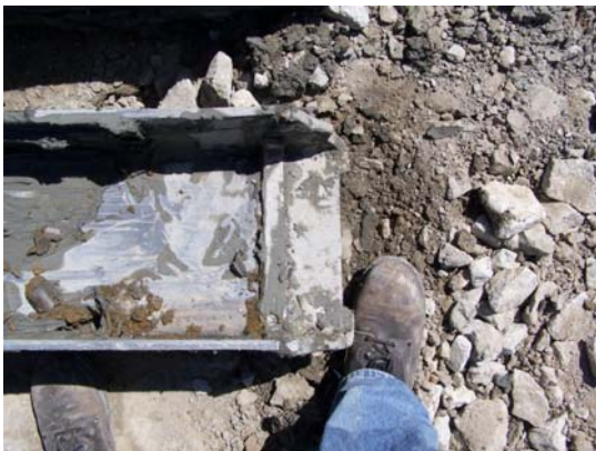
Pile Point C
