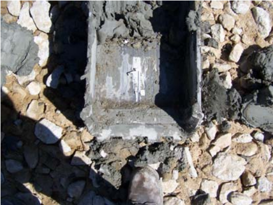
Pile Point L
