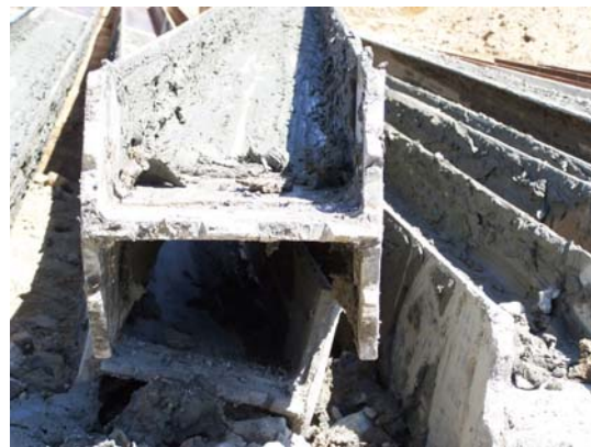
Pile Point B
