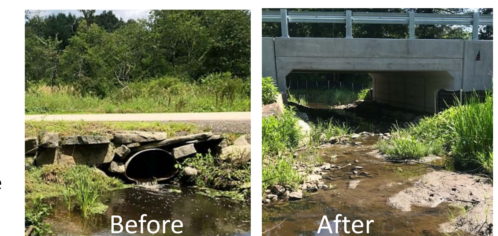
Fig. 10 Retrofitted road crossing to support aquatic and terrestrial wildlife passage 5
