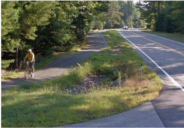
Sidepath along the roadway
