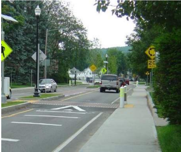
Sidewalks with no buffer
