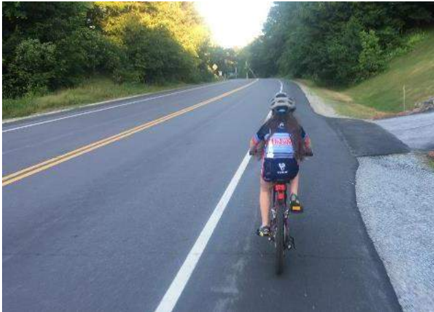
Wider paved shoulders
