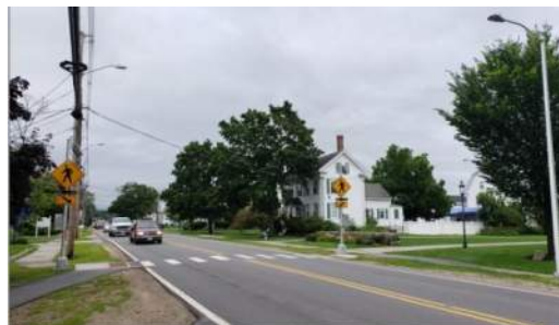
A crosswalk with a Rectangular Rapid Flashing Beacon (RRFB) in Windham, NH (photo: Rebecca Harris)
