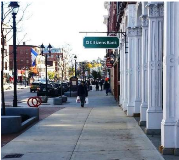
Wide sidewalks with streetscape elements
