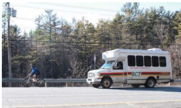
Lebanon Street/NH 120 in Hanover is a multimodal corridor with provisions for active transportation.
