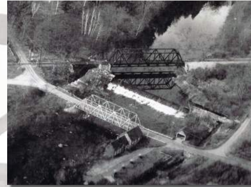
This mid-20th century view shows the dam and canals that powered North Newport's industries. The canal on the left bank first powered a saw mill and then the bobbin blank factory, while the right bank canal powered the Sibley Scythe Factory. By this time, the bridges over the Sugar River were now metal trusses.
