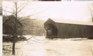
The Flood of 1936 damaged the Oak Street covered bridge's eastern abutment. The damage required the bridge's closure to all but pedestrians, who used the improvised walkway shown above.
