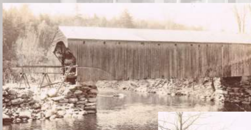
The Flood of 1936 damaged the Oak Street covered bridge's eastern abutment. The damage required the bridge's closure to all but pedestrians, who used the improvised walkway shown above.
