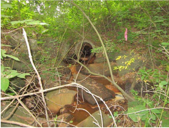
Photo 51: Stream 13 (S-13) – Outlet from PUB wetland/Start of Stream
