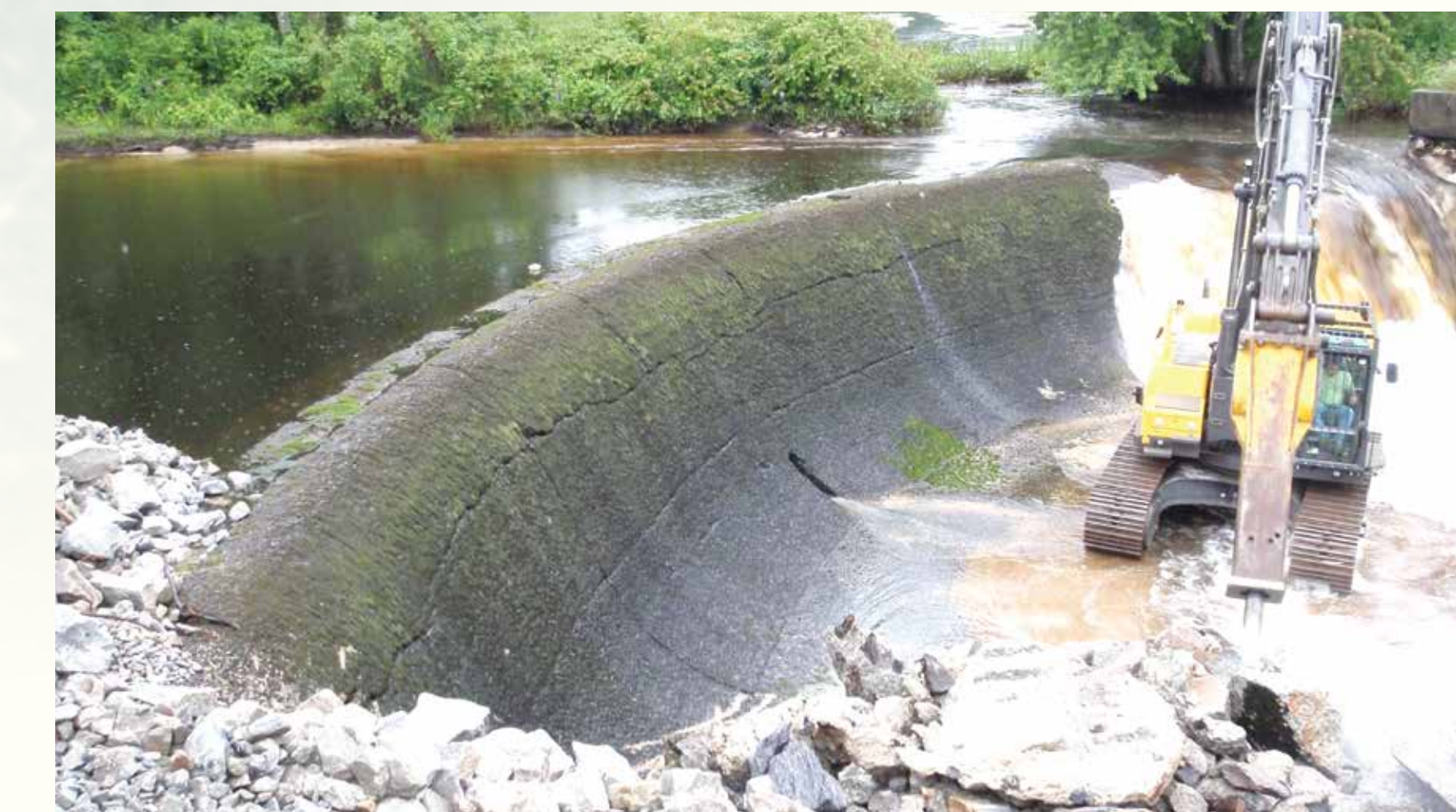
August 2008, Removal of Dam. The machinery removed the upper portions of the north end of the dam first, to release the impounded water. This shows the ogee spillway and one of the outflows. Mark Wamser
