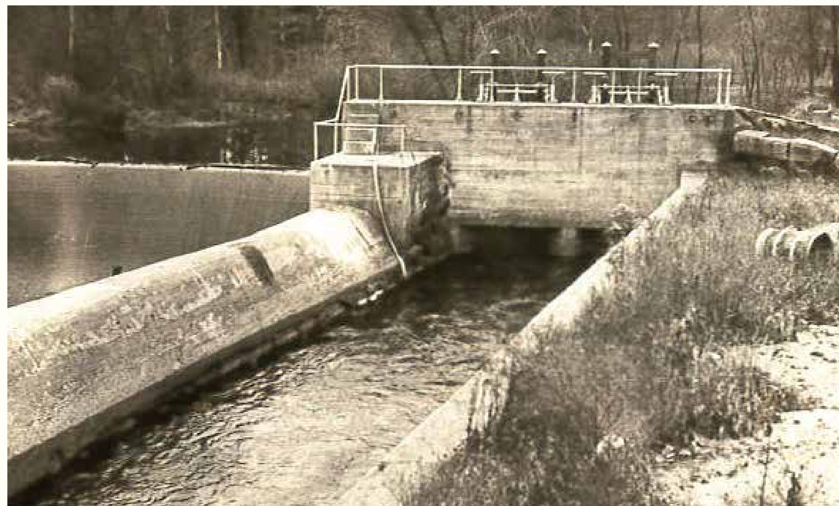
1935 photo of concrete covered power canal and headgate. NH Dam Bureau.
