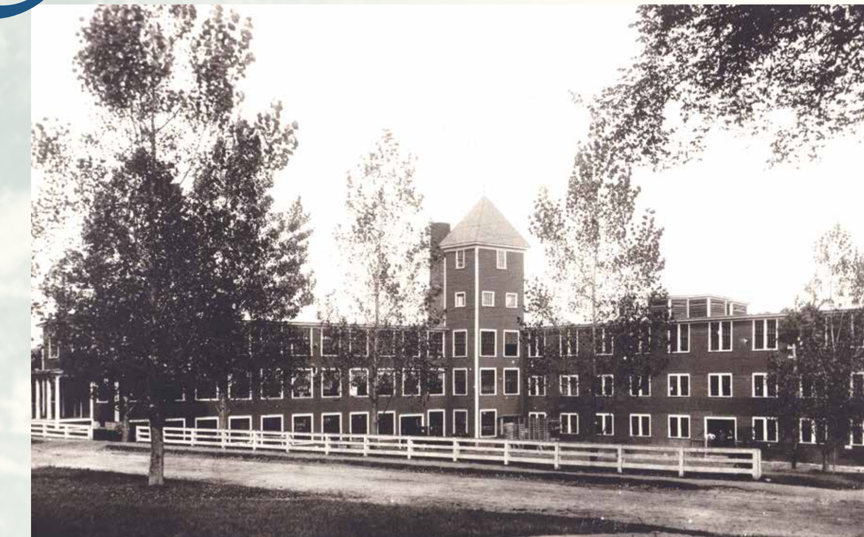
Undated photograph of Shoe Factory, with later alterations including added tower and new power plant to rear made by the McElwain Company. Merrimack Historical Society
