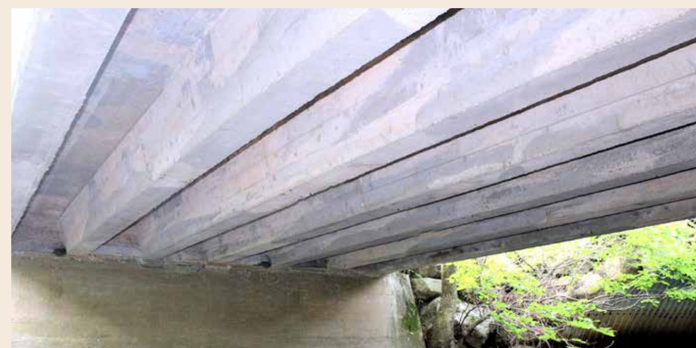
Darrah Bridge underside with concrete encasing the metal girders
