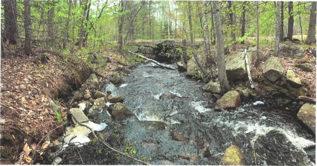
Reference Reach Data collected upstream the next structure upstream of the DOT structure and before reaching beaver dam and large pond upstream of both crossings
