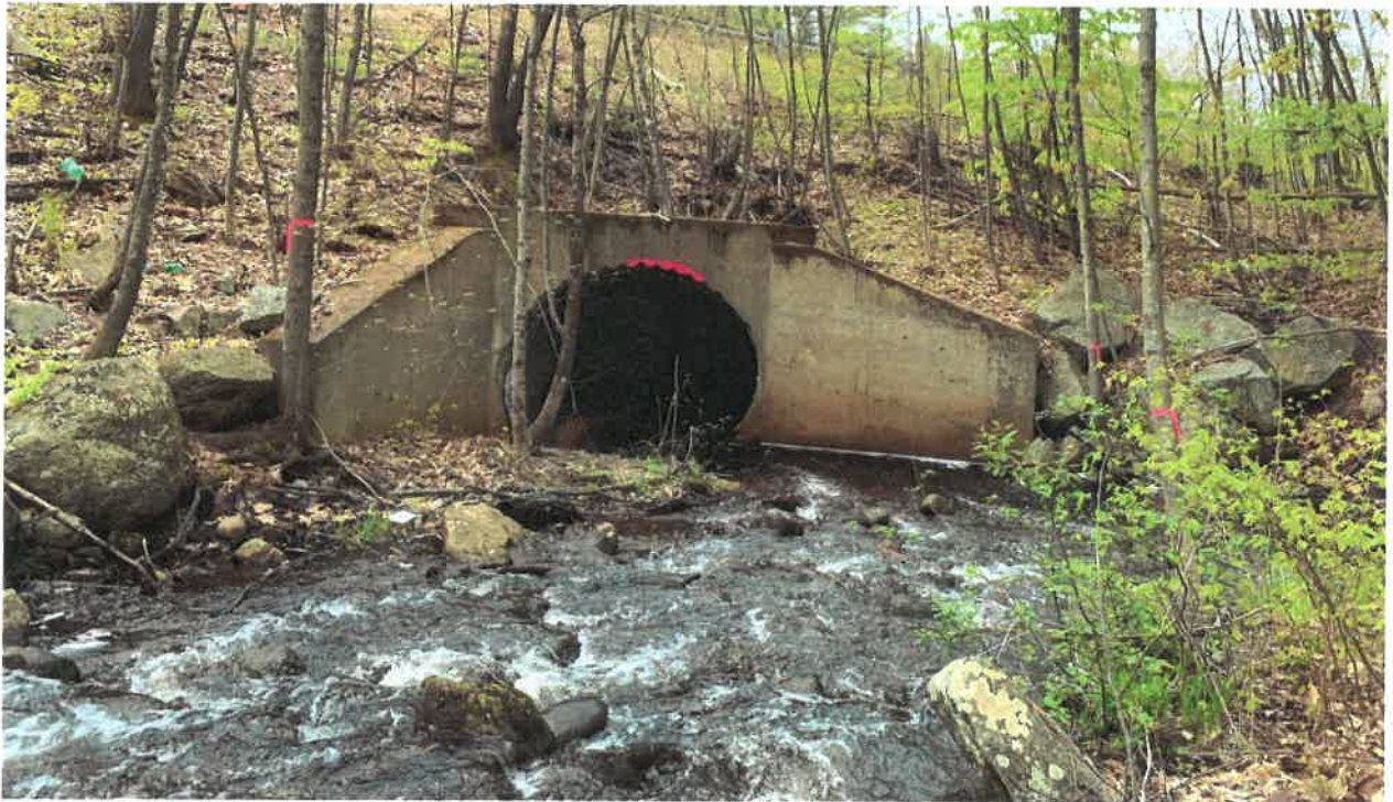
Inlet Cross Section- Facing downstream towards the inlet of the culvert
