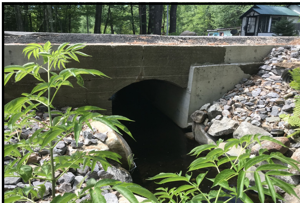
PHOTO 2: A view looking into the inlet of the existing concrete box culvert from the north side of Meredith Neck Road. Both the culvert and headwall have been damaged over time.
