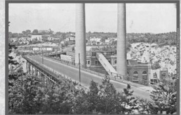
Kelly's Falls Bridge and PSNH power plant, 1940. Harold E Langley, noted Highway Department engineer, designed major repairs in 1940. The bridge was replaced in 1973 when PSNH demolished their power plant, allowing the new bridge to follow a straight alignment.
