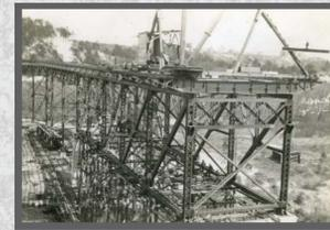
Kelly's Falls Bridge construction, May 1914. Designed by noted engineer John W. Storrs, it was one of the largest bridges in the state at the time. Storrs designed hundred of bridges in NH during the early 20th century.
