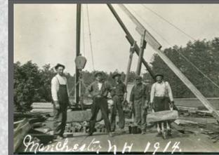
Kelly's Falls Bridge masonry workers posing, 1914. Note timber derrick behind them, used to raise and lower construction materials.
