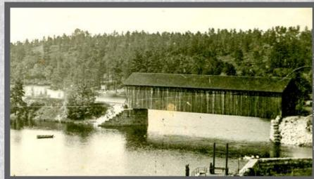
The Boston & Maine Railroad Covered Bridge at Kelly's Falls was a 150'-span lattice truss with a reinforcing arch, built c. 1901. When destroyed by fire in 1941, the roof and siding had already been removed by the railroad to help prevent such a disaster.
