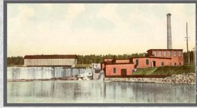
Kelly's Falls Hydroelectric plant, c. 1915, with new concrete dam and coal-fired steam generator plant. More capacity was added in 1925 and 1927 to meet the demand of newly electrified appliances like stoves, toasters and irons.
