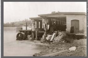
Kelly's Falls Hydroelectric Plant, March 1, 1896, after 36 hours of rain caused the stone dam to burst, collapsing the generator house and dumping equipment into the river. The plant was quickly rebuilt to maintain its share of the competitive and growing electric lighting market.
