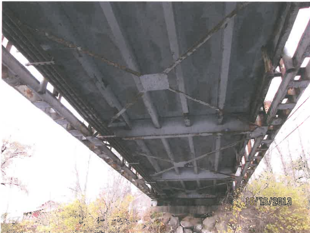
Photo 6 – View from VT shoreline looking westerly at existing river bank and bridge abutment to be temporary impacted to temporarily relocate bridge during pier replacement.
