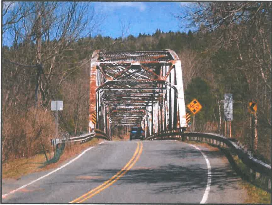
Figure 3: Existing bridge crossing, view to the east (MAC report, 5-12-16)
