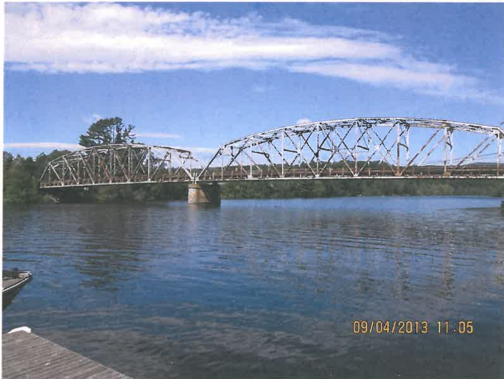
Photo 1 – View from NH shoreline downstream of bridge looking northwesterly and upstream at areas of proposed temporary trestles during reconstruction.
