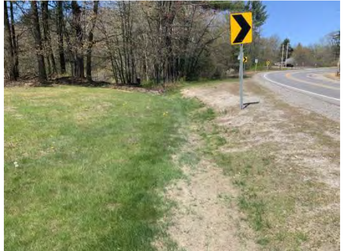
Photo 6. NJDA-3 is a grass swale that conveys stormwater to Stream 1 and Wetland B (* Photo taken 17 May 2022).
