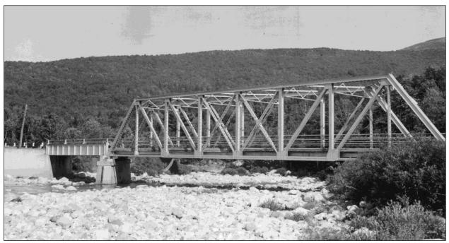
FIGURE 30: Gorham 092/058, NH 16 over Peabody River. Built 1912 by United Construction Co., Replaced in 1950. One high Pratt truss span and one thru-plate-girder span. The truss had eight panels, 16'-0" long, for a total length between the bearing pins of 128'-0". Photo August 29, 1940 (NHHD Bridge Inventory Card).
