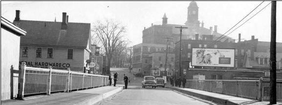
FIGURE 51: Claremont 132-097, Broad St. Bridge over Sugar River. This 2 span deck plate girder bridge was designed by Storrs and built by United Construction Co. in 1915. It had an overall length of 138 feet. Replaced in 1981 with a single-span I-beam bridge. Photos taken during inspection of the bridge by NHHD engineers on November 19, 1940 (NHHD Bridge Inventory Card).
