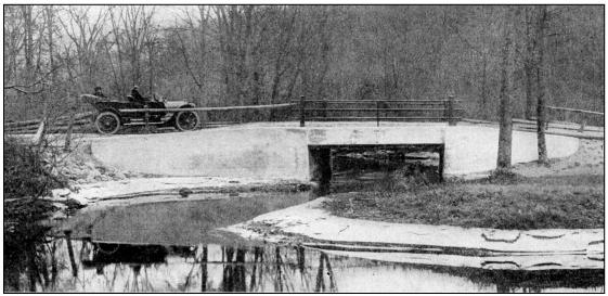
FIGURE 25: Bow 135/160 Turkey River Bridge, an 18' span jack arch built 1911 by Boston Bridge Works. Upstream side, pictured in Storrs & Storrs bridge construction handbook (Storrs & Storrs, 1918, p. 11). Demolished and replaced in 1959 with I-89 Ramp.
