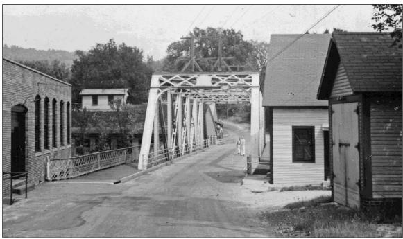
FIGURE 1: Claremont 091/118, Plains Road over Sugar River. This single 131' span high Pratt truss was designed by John Storrs and built by United Construction Co. in 1906. Replaced in 1974. Photo August 26, 1942 (NHHD Bridge Inventory Card).
