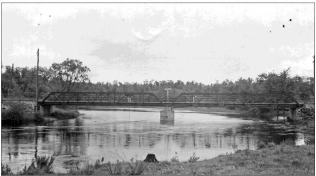
FIGURE 23: Tilton-Northfield 128/158 (now 109/062), a two span Warren pony truss carrying NH 140 over Winnipesaukee River. Designed by John Storrs and built by Canton Bridge Co. in 1910. Replaced in 1968. Each truss measured 67'-7" between bearings. Photo June 17, 1942 (NHHD Bridge Inventory Card).
