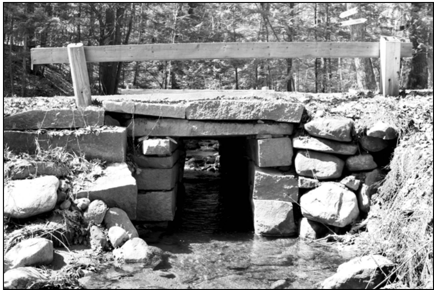
Photo No. 10: This is an example of a typical cut-stone (ashlar) box culvert located in Marlborough, NH (MAR0015). It is of average size (4'-0" opening width), built with split lintel spans, ashlar channel walls and mixed cut and field stone facewalls.
