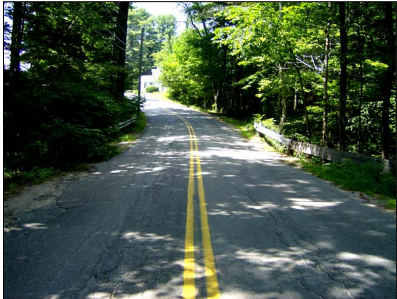
Photo No 19: Repair cracked, broken pavement to stop water infiltration. Repair or install curbing to direct runoff away from culvert and embankments.
