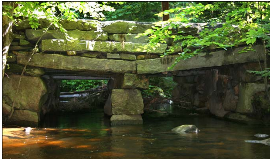
Photo No. 15: The center wall of this double box culvert has settled and shifted dramatically at the outlet end due to scour undermining and is now in danger of collapse. Scour is most severe on the downstream side of piers and abutments.
