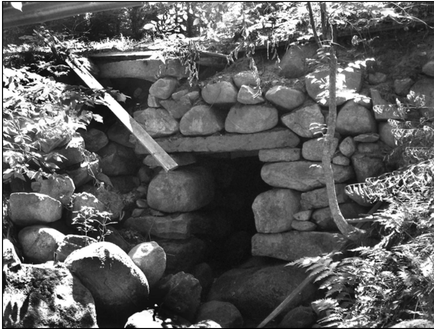
Photo No. 16: This 3.5' box culvert in Wolfeboro, NH, WOL0026 has split lintel spans and fieldstone walls. The dry-laid masonry is "loosely built," with poorly fitted joints, due to the use of rounded boulders that offer limited bearing surface. Rough work like this is normally chinked and mortared. It stands due to the weight of the overlying fill pressing the stones tightly together from all sides. If the fill is lost, the stones will follow. In this case roadway runoff has washed out and collapsed the facewall on the left.
