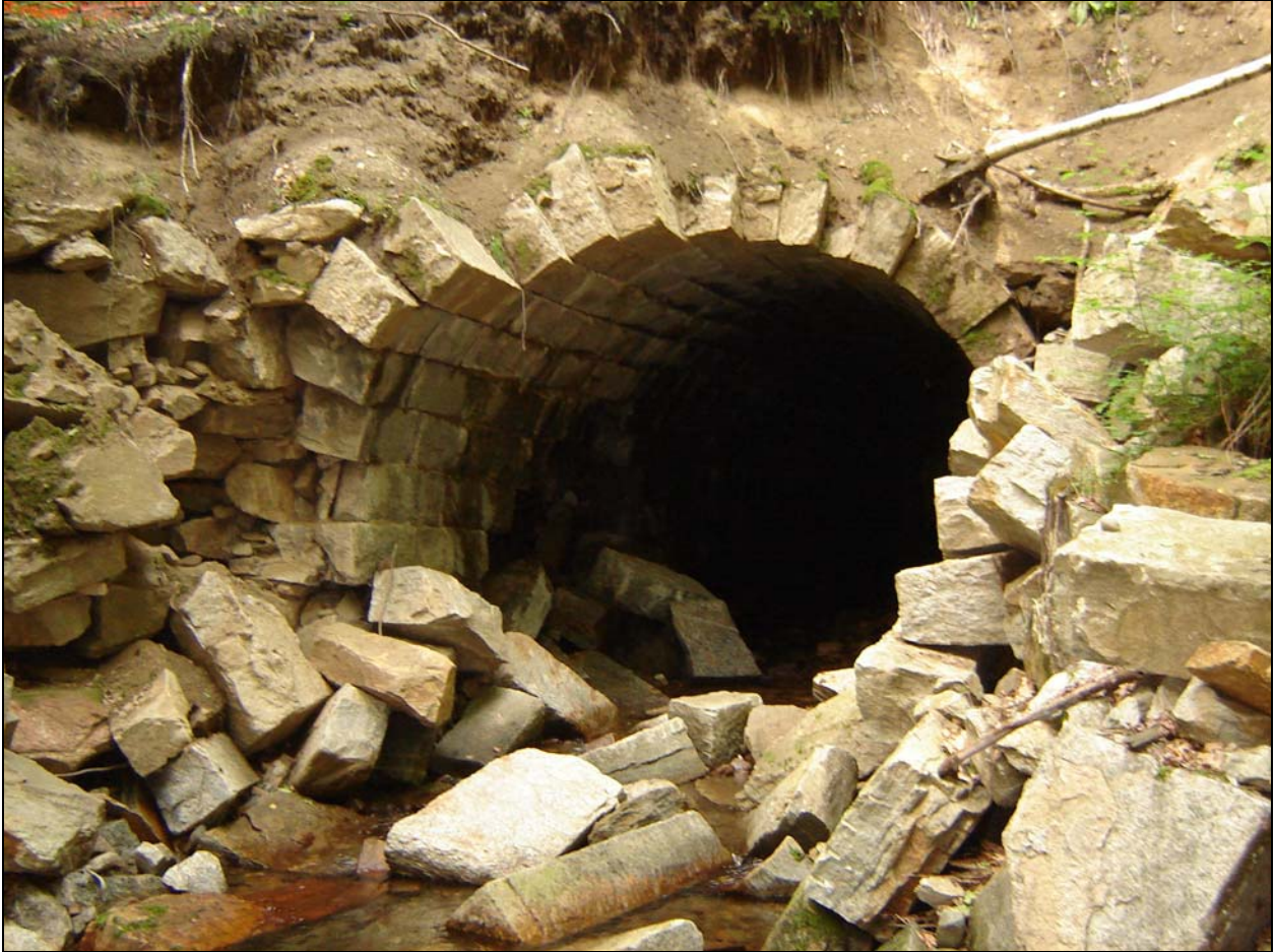
Photo No. 23: Remarkable workmanship exposed by the partial collapse of this stone arch culvert on the former Cheshire Railroad line in Westmoreland NH (Photo courtesy of James Garvin, NHDHR).
