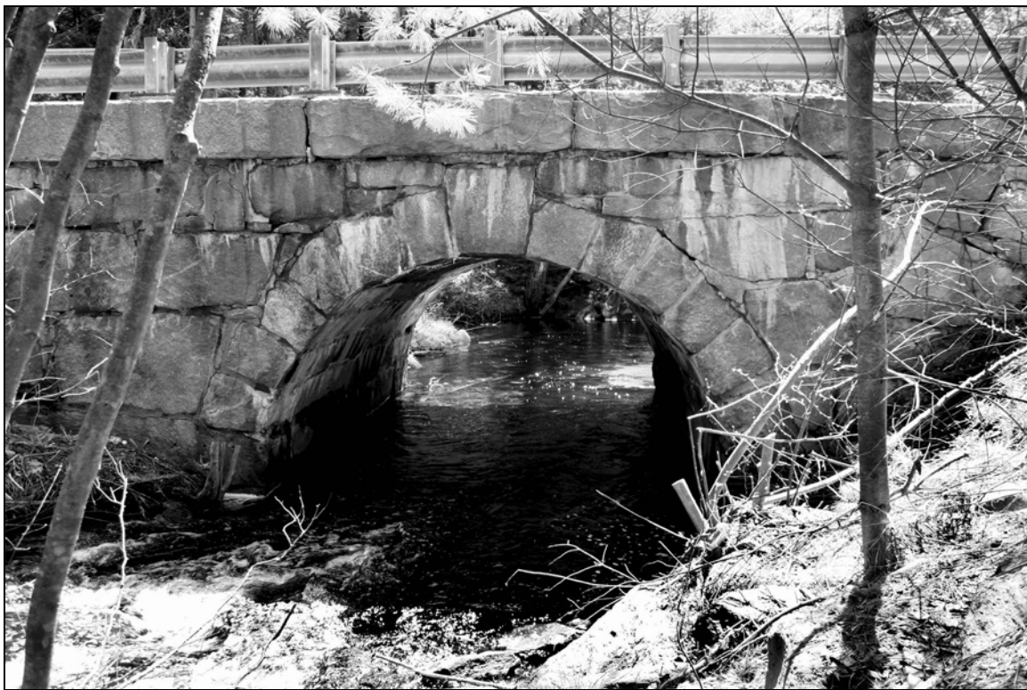
Photo No. 11: This is an outstanding "textbook" example of a semi-circular cut-stone arch culvert located in Jaffrey, NH (JAF0464). It displays a very high degree of skilled masonry craftsmanship in the tightly fitted arch stones, enlarged keystone and massive cut facewall stones.
