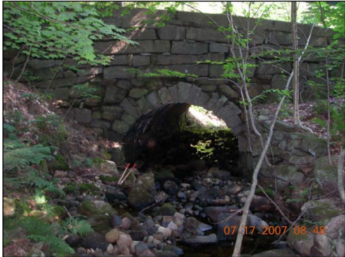
Photo No. 18: Regularly remove small trees and vegetation growing in stonework before it becomes a big problem.
