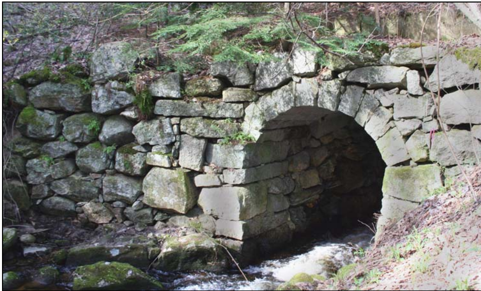
Photo No. 12: This culvert is located in Litchfield, NH (LIT0010). The 7' span arch is a segment of a circle springing from tall sidewalls. The type is sometimes called a horseshoe arch, but is more correctly known as a stilted segmental arch
