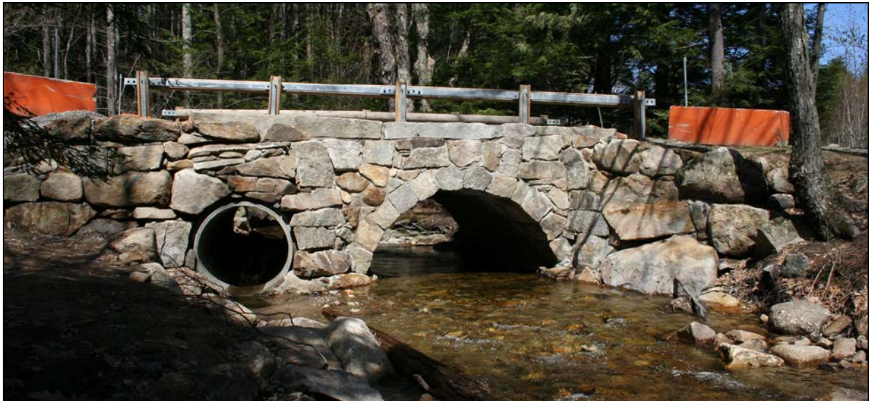
Photo No. 24: This arch culvert in Temple NH (TEM0002) was washed out by flood waters and reconstructed using the original stone. A pipe bypass culvert was installed to the side of the arch to increase the flow capacity. Bypassing causes some loss of integrity of setting, feeling and association but may not substantially diminish the culvert's most important characteristics providing the majority of its functional stonework is left undisturbed and unaltered.
