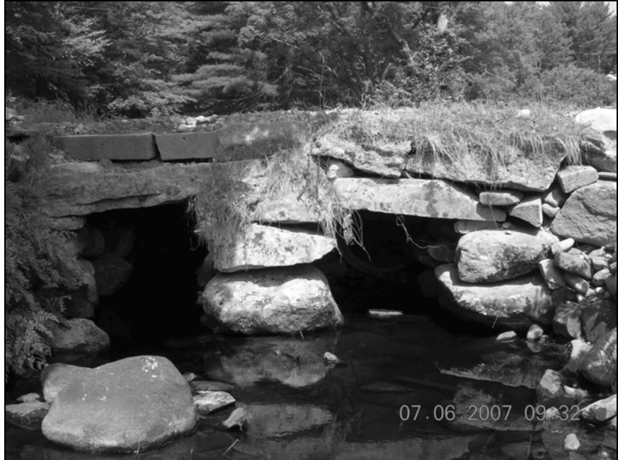
Photo No. 9: A double box culvert in Canterbury, NH, (CNT0007) with two 3'-6" wide openings, split stone slab spans and a center wall built with large-dimension fieldstone.
