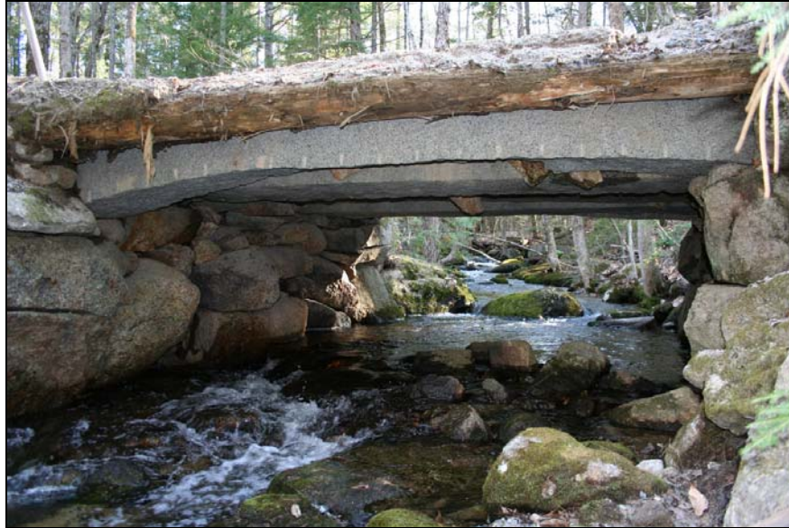
Photo No. 5: This box culvert in Hillsborough, NH (Culvert HIL0019) is of exceptional span with a 10'-6" opening width. It is built with split granite lintel spans and fieldstone walls. The outside lintel seen in the picture is particularly interesting in that it was cut from a quarry face with a slight curve to it, giving the lintel a slight arch shape with thickened ends. While unsuitable for many purposes the builder perhaps saw the structural advantage of such a stone beam for use in this culvert project.
