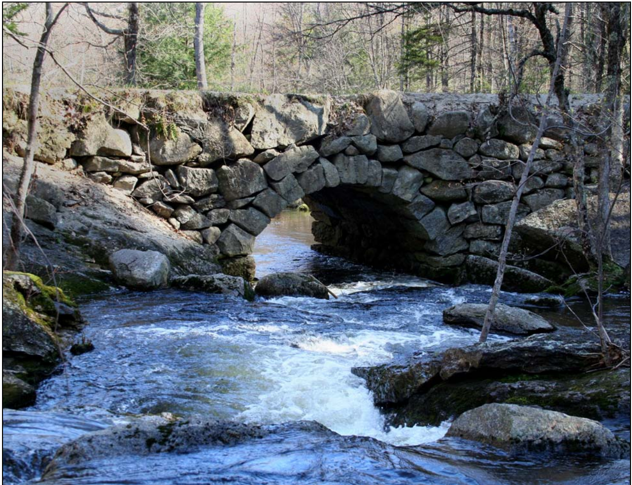
Photo No. 2: This stone arch culvert (HIL0022) and another similar but larger one only 100 feet away (HIL0023) carry Beard Brook under Gleason Falls Road in Hillsborough, NH. This is a segmental arch – nearly semi-circular – spanning 12 feet. Twelve stone arch bridges and culvert-size bridges (see Photo No. 4) were built in Hillsborough during the 19 th century.
