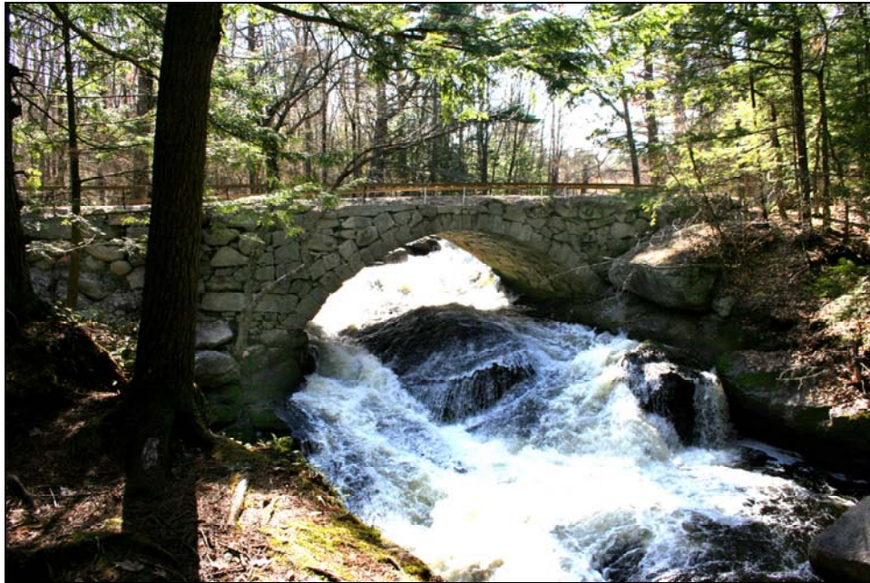
Photo No. 4: This stone arch bridge in Hillborough (HIL023), the companion arch to the one in Photo No. 2, was built with the same materials and techniques but with a longer span and a flatter segmental arch, illustrating the similar characteristics of arch bridges and culverts.
