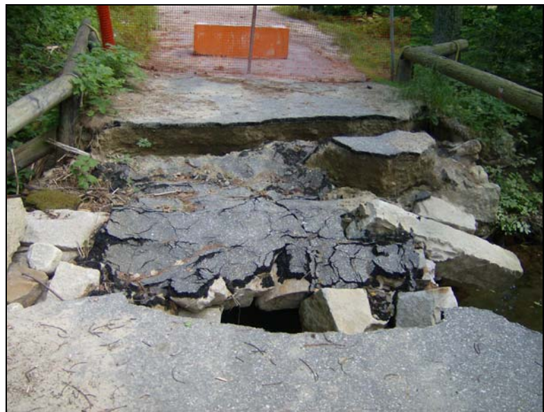
Photo No. 17: Collapsed roadway over stone arch culvert in Temple, NH caused by overtopping. (Photo courtesy of James Garvin, NHDHR).
