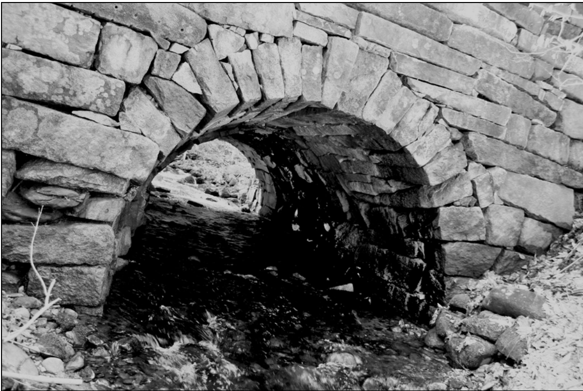
Photo No. 14: This culvert is also located in Hillsborough County, in the town of Wilton (WIL0006) and is an exceptional example of an entirely dry-laid segmental arch (nearly semi-circular) built with split and cut stone. Much of the stone was thinly bedded and split readily into thin manageable slabs that could then be easily squared and tightly fitted with a minimum of chinking required. An occasional untrimmed fieldstone is mixed in for economy and speed. Not visible are concrete roadway curbs that support railing posts, a visual but necessary detriment that does not significantly diminish the integrity of the resource.
