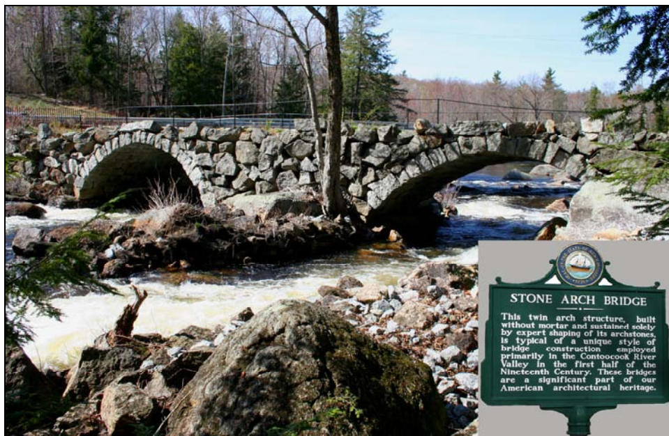
Photo No. 26. This Twin Stone Arch Bridge with segmental arches, cut arch stones and fieldstone facewalls is located in Stoddard, NH, spans the North Branch of the Contoocook River near the Antrim town line. It is now bypassed by a new bridge and preserved in a small public roadside park visible from Route 9. A historical marker (inset) commemorates this important historic artifact.
