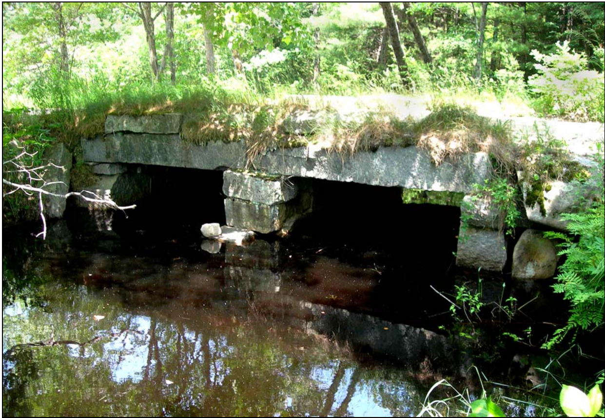
Photo No. 7: This is a double box culvert in Fitzwilliam, NH, (FIT0017) with two 6-foot channel openings. It is built with cut lintels and mortared cut-stone channel walls. Culvert channels are sometimes referred to as cells or barrels.
