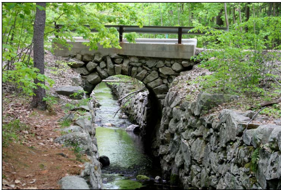
Photo No. 25: A heavy reinforced concrete curb/parapet has been cast-in-place across the top of the facewall of this culvert in Wakefield (WAK0010) with the dual purpose of providing a strong anchorage for the railing and a curb capable of redirecting tire impacts back into the travel lane. By eliminating the need to anchor the railing posts into the facewall, the culvert is protected from damage that could result from a forceful impact. The curb or cap beam helps consolidate and protect the top of the facewall from loosening due to erosion and vibration and could be an acceptable alteration in situations such as this.
