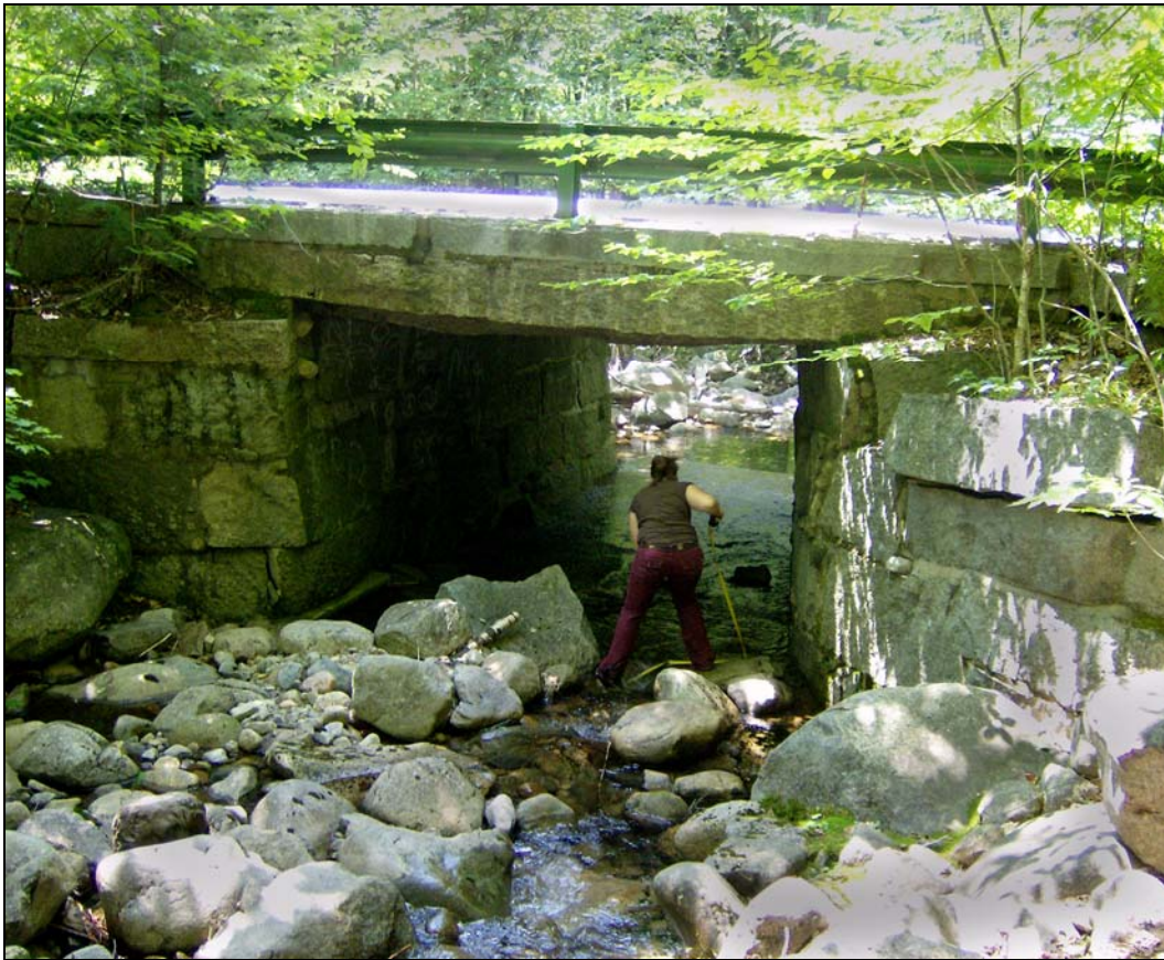
Photo No. 8: This box culvert in Albany, NH (ALB0045) has an unusually large area of waterway opening, with a 9'-4" opening width (span) and 8'-0" opening height. The channel walls are built with very large dimension cut stones bedded in mortar, notable for both their length at 25'-9" and their craftsmanship. Note the massive lintel.
