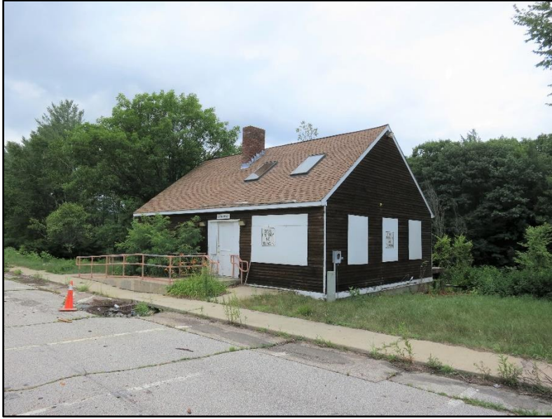
Rumney Rest Area Building constructed in 1986
