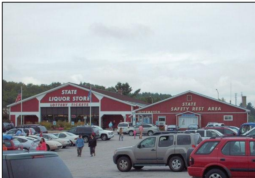
Hooksett State Liquor Store and Safety Rest Area Building, constructed 1979
