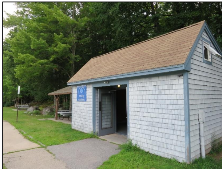
Vending machine shelter at Sutton Rest Area
