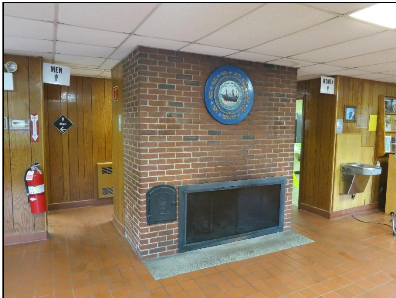
Fireplace, Canterbury Rest Area
