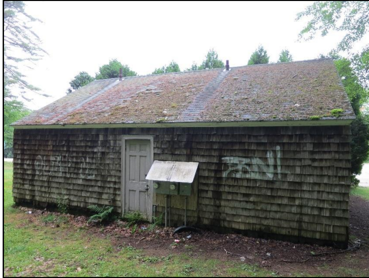
Rear elevation of original Sanbornton Rest Area (now storage)
