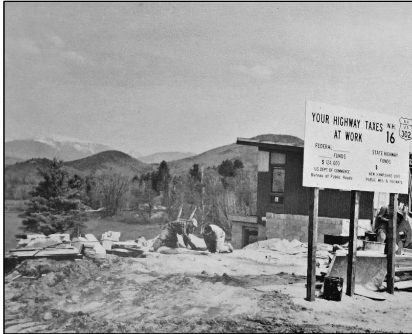
Intervale/North Conway Rest Area under construction Source: New Hampshire Highways , October 1967
