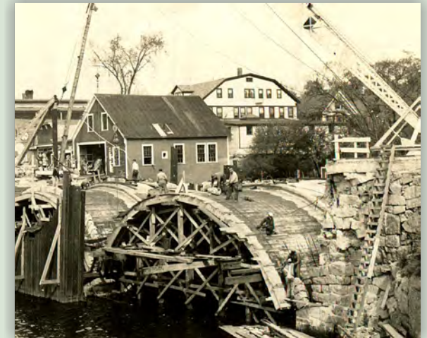
Rebuilding Henniker's 18th-century double stone arch bridge in 1938. Photo courtesy Henniker Historical Society.
