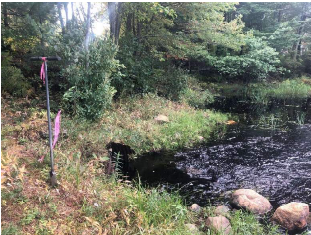
Wetland A—Downstream side of Johnson's Pond at culvert outlet
