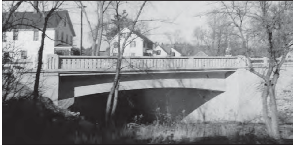
Figure 8. T-beam Bridge Carrying Dartmouth College Road/N.H. Route 10 over Croydon Branch River in Croydon (State Bridge No. 112/069). Circa 1935. Designed by Gordon Whittum (NH DOT Bridge Card).
