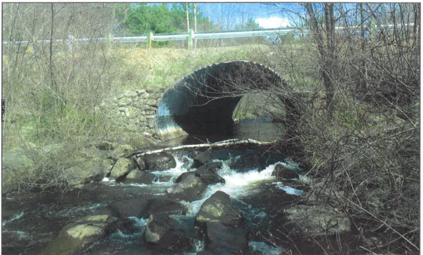
Photo 6: Looking North (upstream) at bridge outlet
