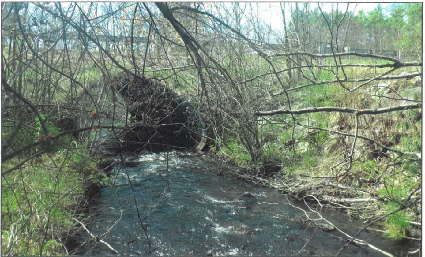
Photo 4: Looking South (downstream) at bridge inlet
