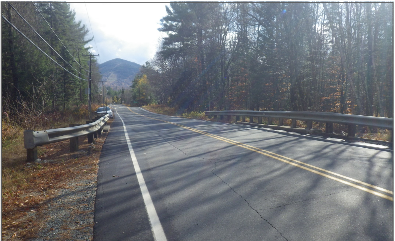
Photo 2: Looking south along NH18
