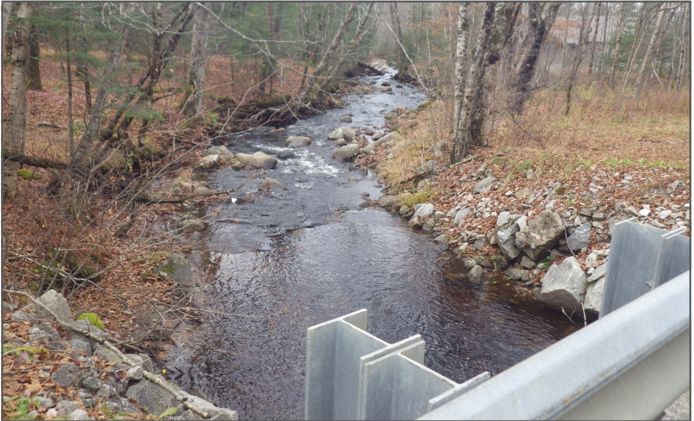
Photo 5: Looking east (downstream) from NH 18
