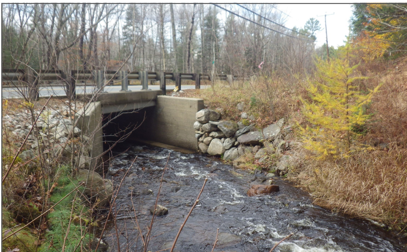
Photo 4: Looking east (downstream) at inlet
