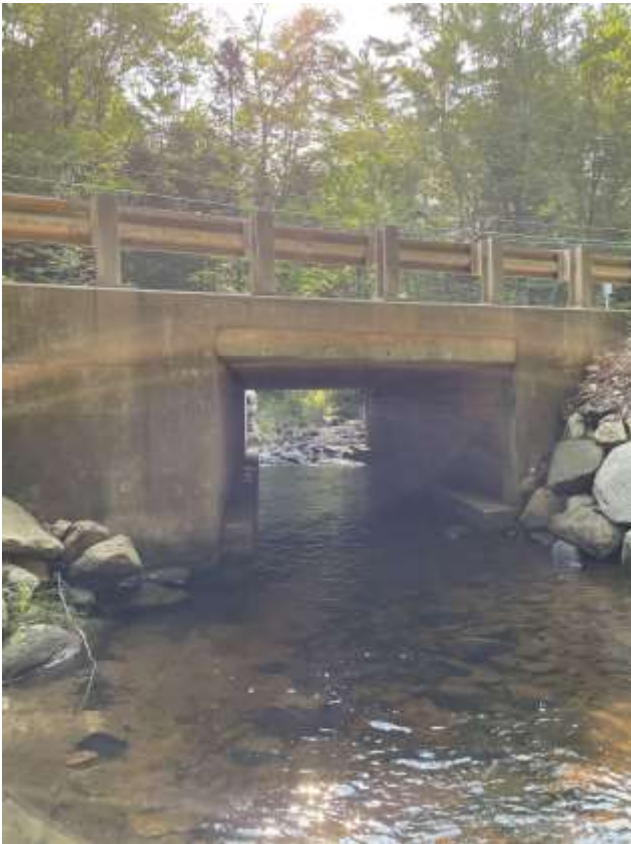
Outlet Looking Upstream
