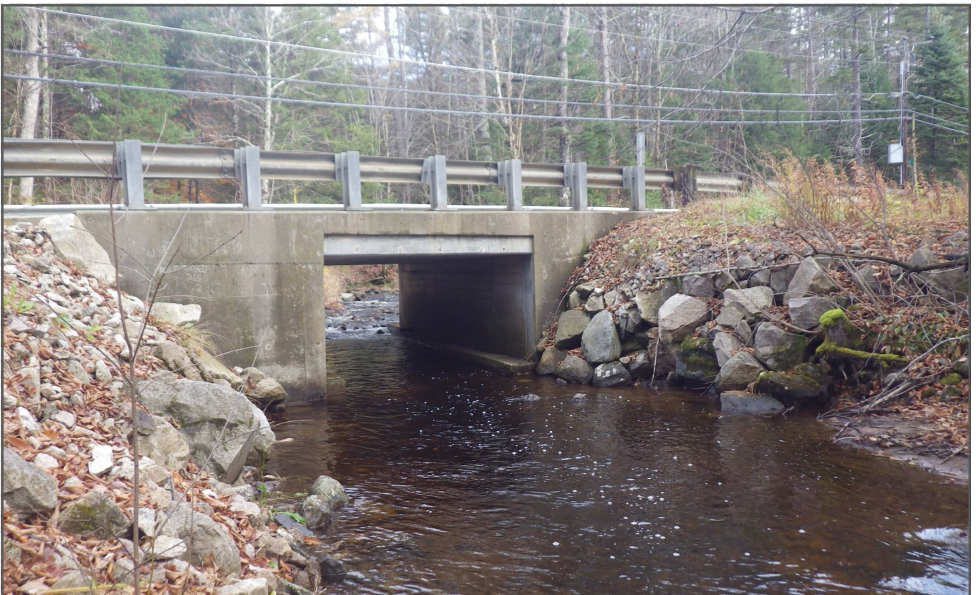
Photo 6: Looking west (upstream) at outlet
