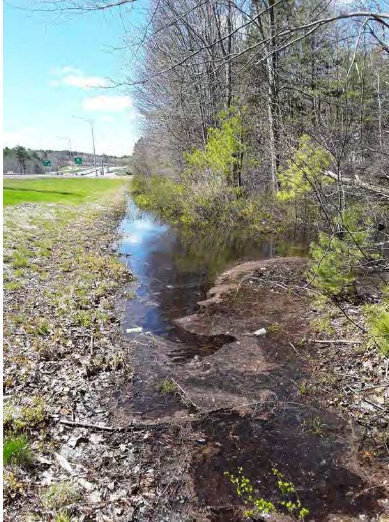
Facing northwest along western wetland and VP boundary
