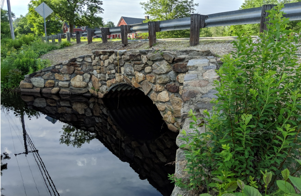
Photo 11: View northeast of the downstream side of the corrugated steel pipe arch bridge (6/27/19).
