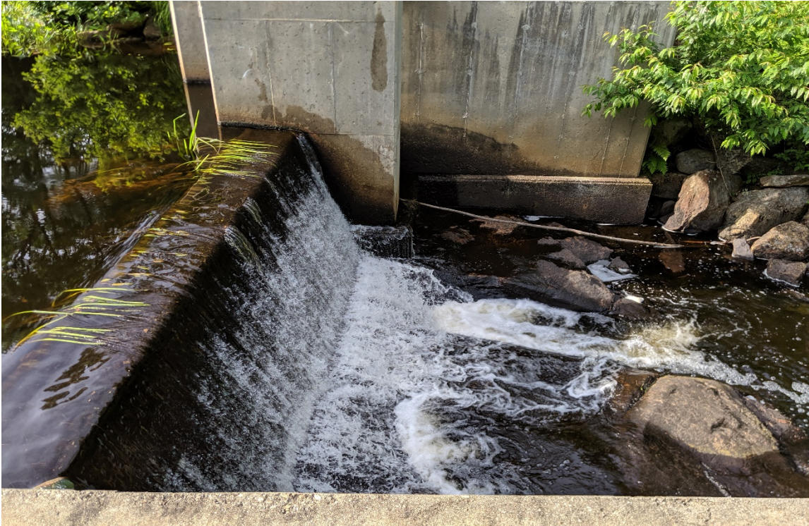
Photo 14: View north of the Freeses Pond Dam spillway (6/27/19).
