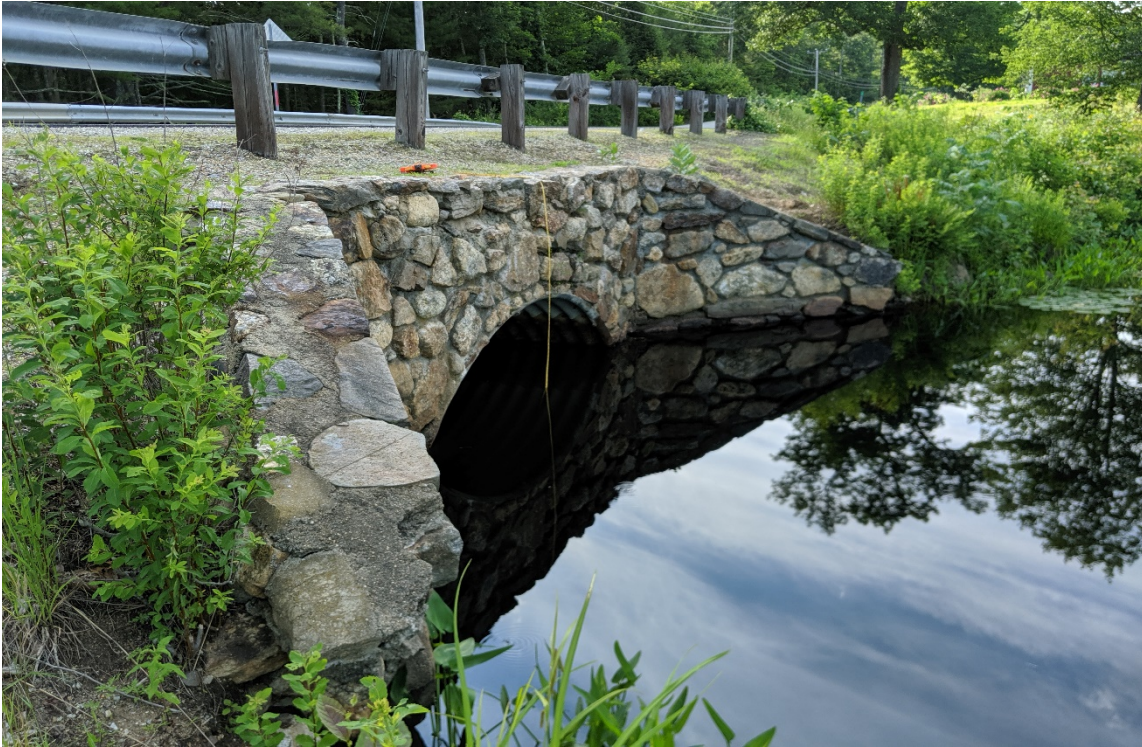
Photo 3: View northwest of the upstream side of the corrugated steel pipe arch bridge (6/27/19).
