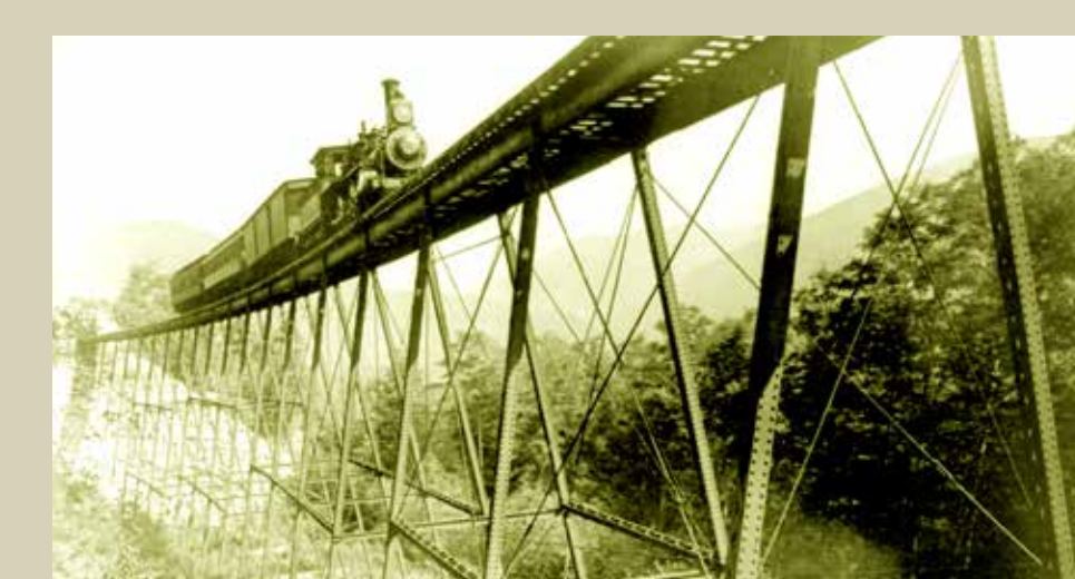
1885 photograph of the first (wrought iron) Frankenstein Trestle, built by the Portland & Ogdensburg Railroad in 1875. In 1892 it was replaced with the current steel trestle which still carries excursion trains through Crawford Notch. Library of Congress
