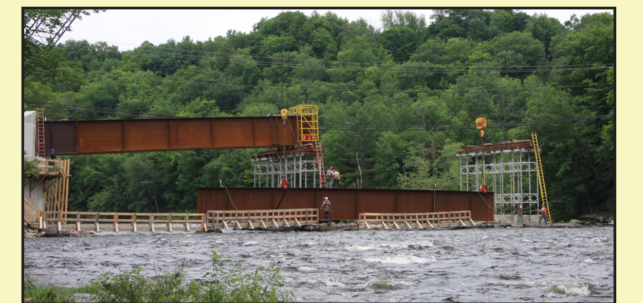
Erecting new bridge, July 2009. Preparing plate girder lift.
