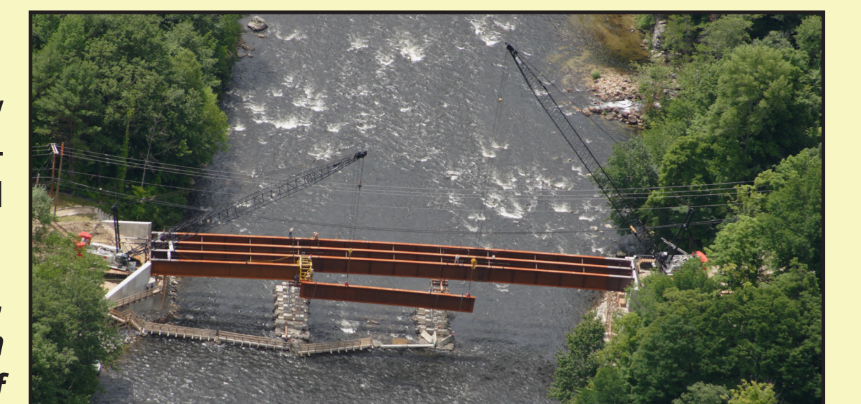
Lifting and setting the plate girder with two cranes.
