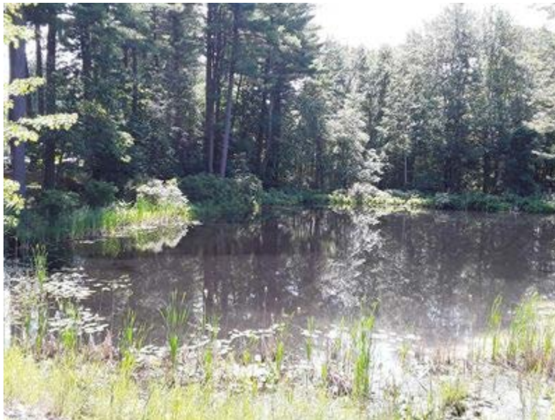
From road culvert facing open (7/30/2020)
