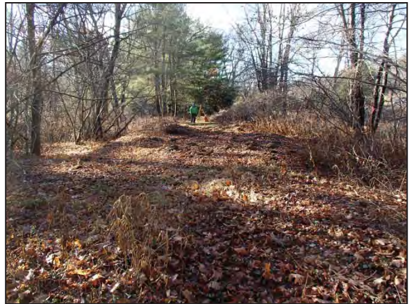
View southwest along abandoned road toward abandoned bridge. Photo date: 12-01-16
