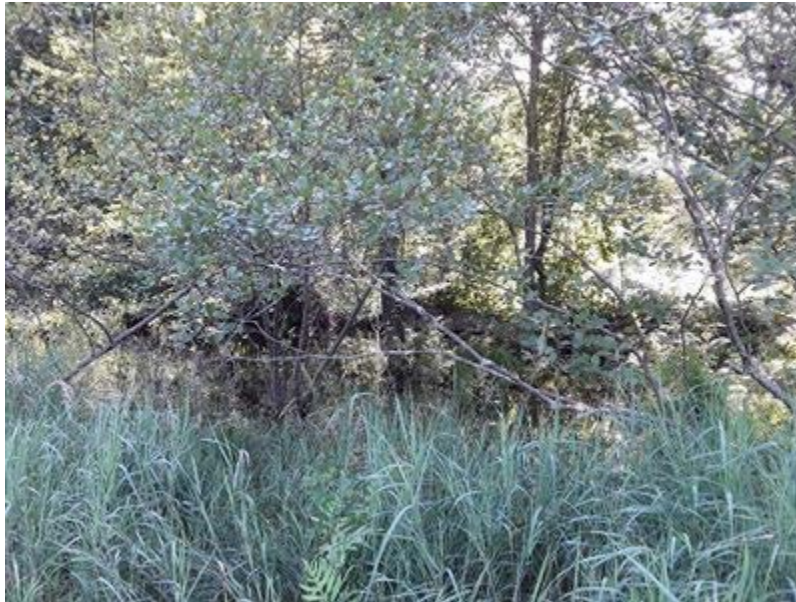
Between flags 7 and 8 facing headwall (7/30/2020)
