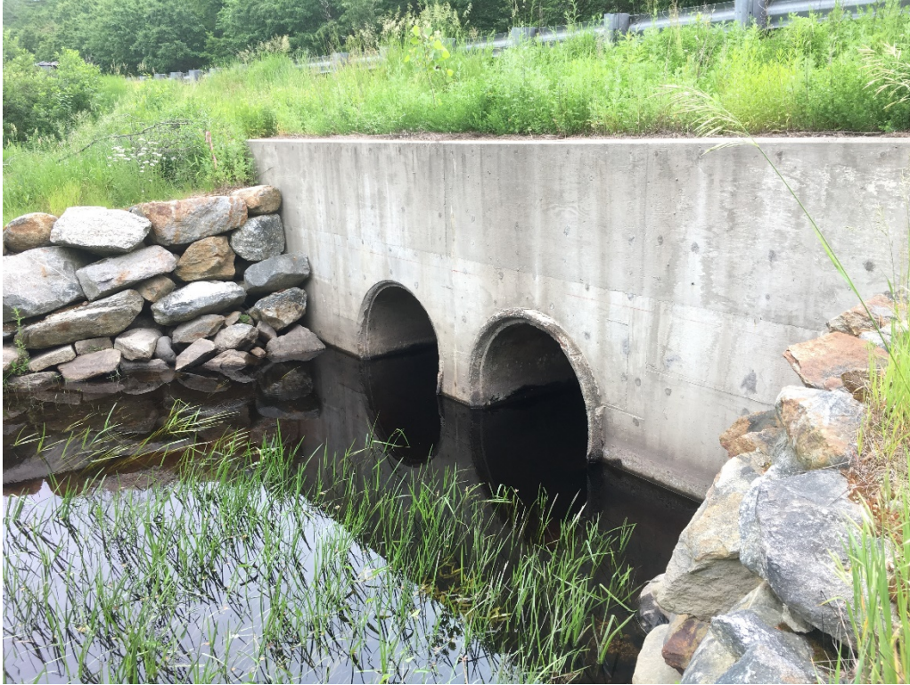
Facing headwall and NH Route 101 from W8 (6/16/2017)
