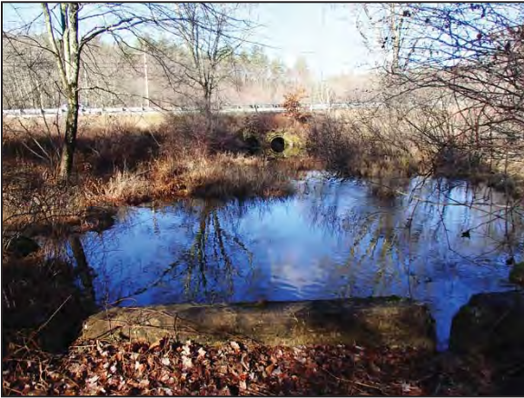
View upstream from abandoned bridge toward Route 101. Photo date: 12-01-16
