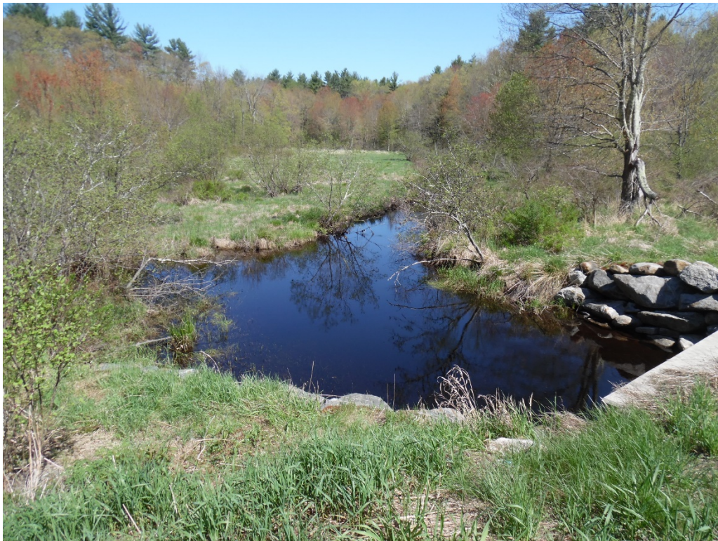
Facing north from culvert headwall (5/9/2018)
