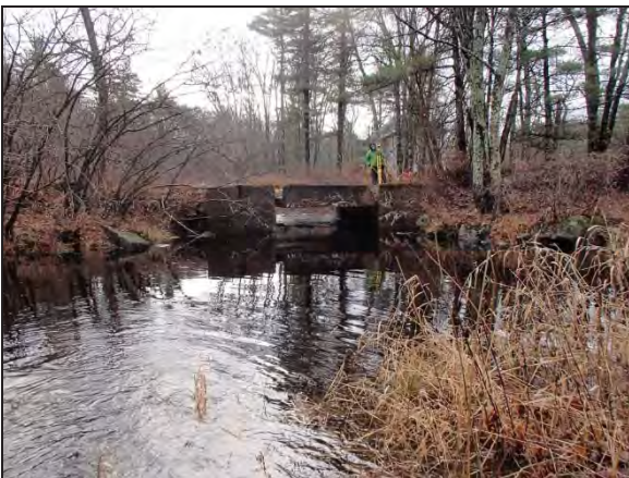
View downstream toward inlet of abandoned Bridge. Photo date: 12-01-16
