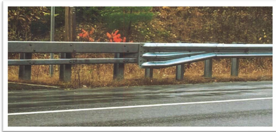
Asymmetrical Transition Rail Section
