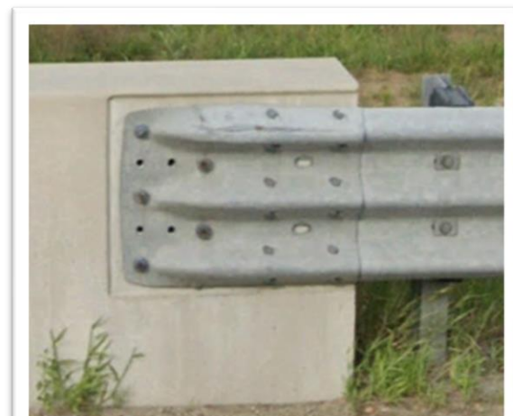
Connection Plate and Thrie-Beam Terminal Connector
