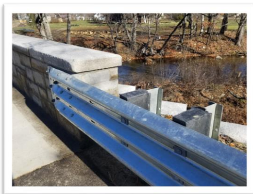
Connection Plate and Thrie-Beam Terminal Connector
