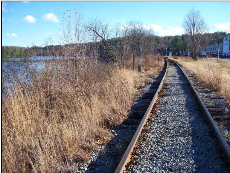
View south of the existing rail line and the Merrimack River near Hall Street in Concord
