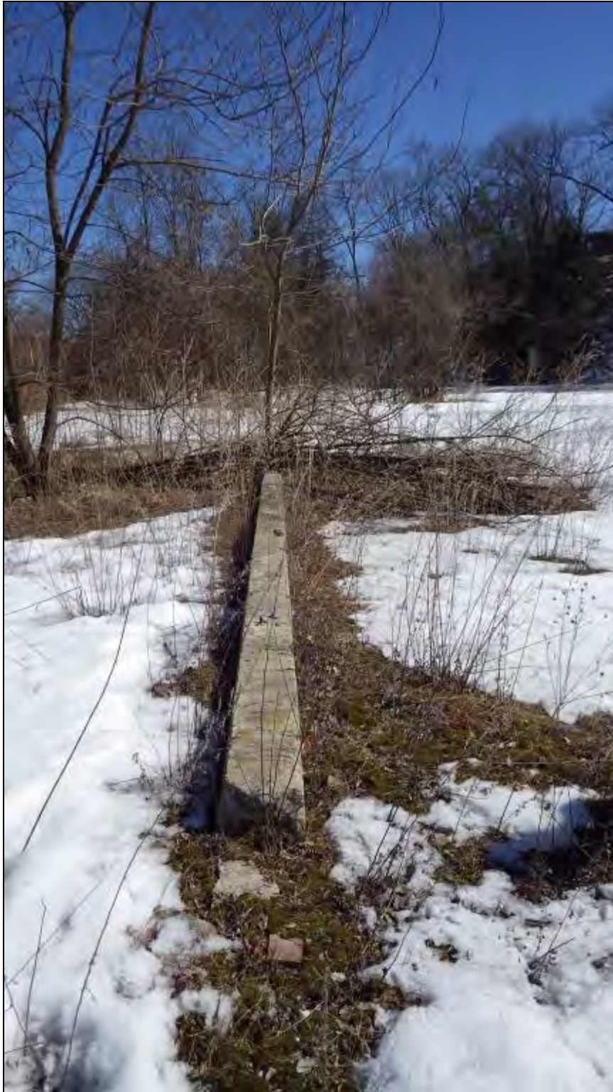
Figure 86 - Eastern wall of a large structure in the upper area of the proposed Crown Street parking area, facing south.
