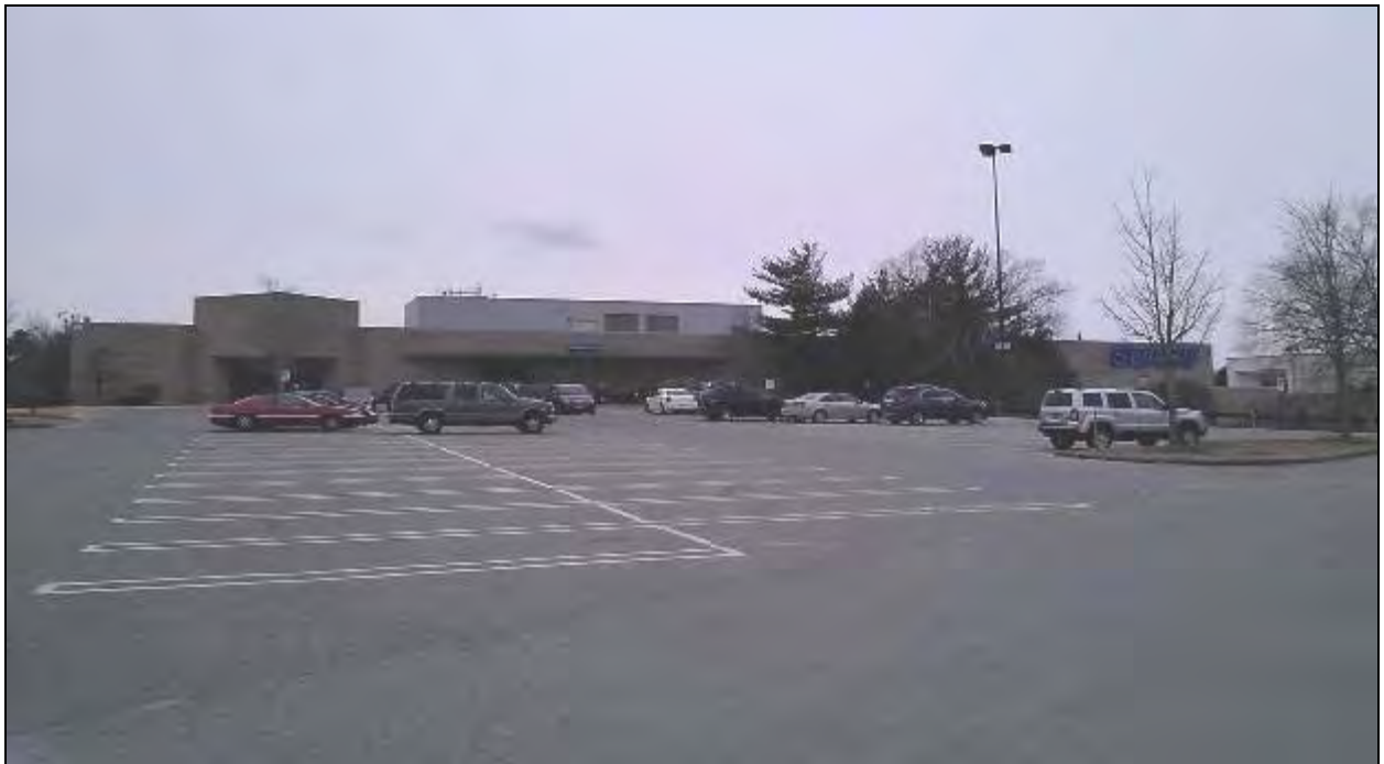
Figure 105 - Location of the Pheasant Lane Mall Station parking structure. This location is currently overflow-parking for Sears.
