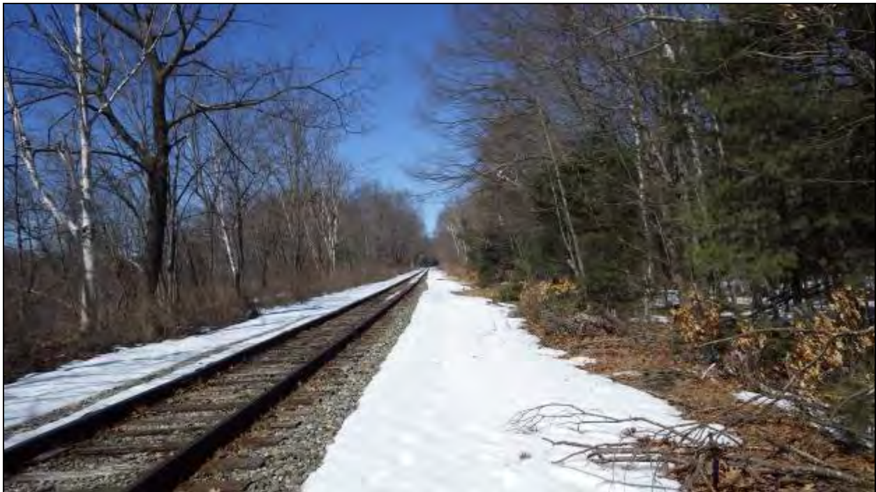
Figure 63 - View of the proposed railroad siding, facing north.
