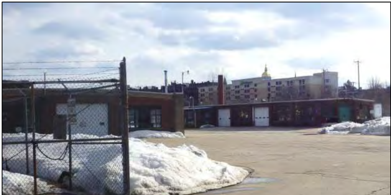
Photo 46. Rear of C-5 in the Direct APE for Stickney Avenue Station and Layover Facility; view southwest from driveway
