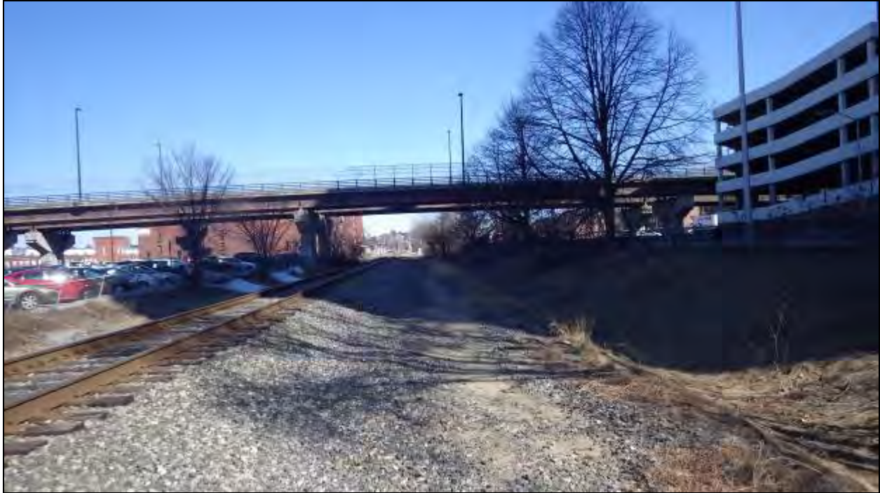
Figure 39 - Spring Street Station APE facing north. The right of frame shows a drainage ditch that separates the rail bed from Canal Street. In the background is the Bridge Street overpass, under which part of the proposed platform will reside.
