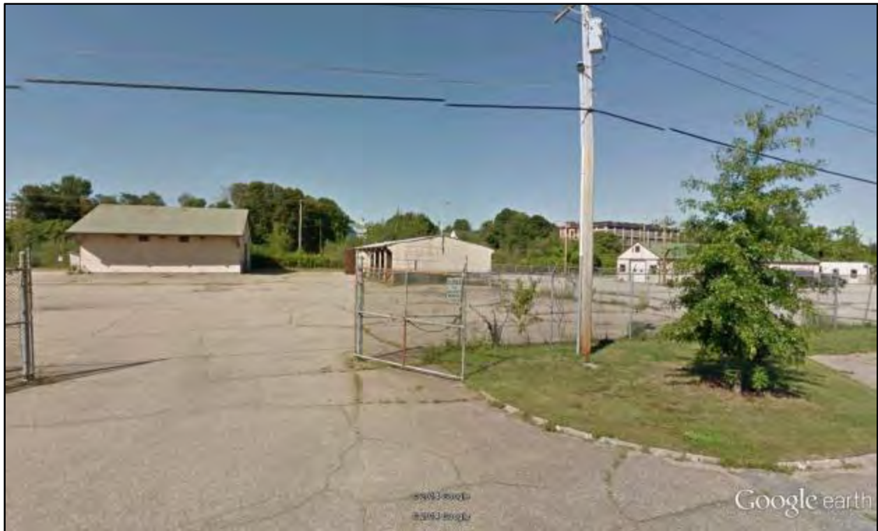
Photo 47. C-6 (left), C-7 (center), and C-8 (right) in the Direct APE for Stickney Avenue Station and Layover Facility; view west from driveway (Google Earth August 2011)
