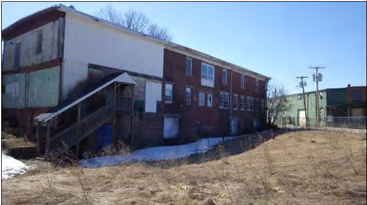
Figure 88 - East wall of an old building, facing northwest.
