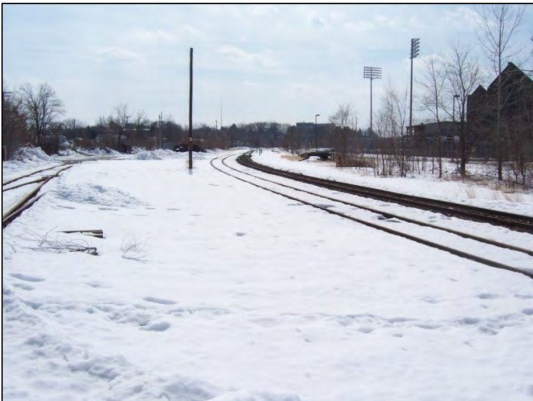
View south along existing rail line at Riverwalk Way Layover Site in Manchester
