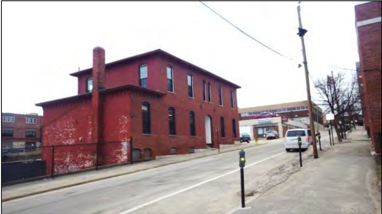
Photo 55. Indirect APE for Spring Street Station, view east on Hollis Street showing a late 19 th century industrial building
