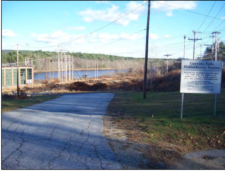
View toward the existing rail line near the Garvins Falls Dam in Bow
