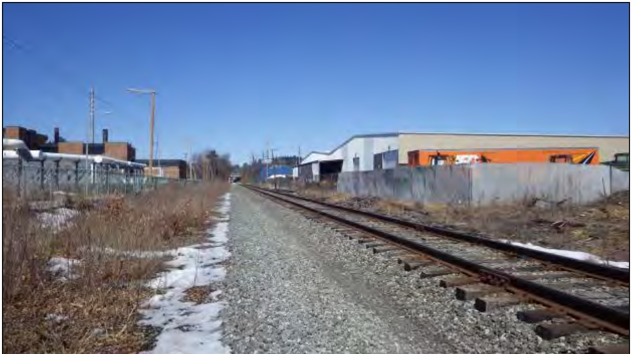
Figure 73 - Wastewater Treatment Plant Layover APE, facing north. The Wastewater Treatment Plant is located in the left of frame and a warehouse complex is located in the right of frame.
