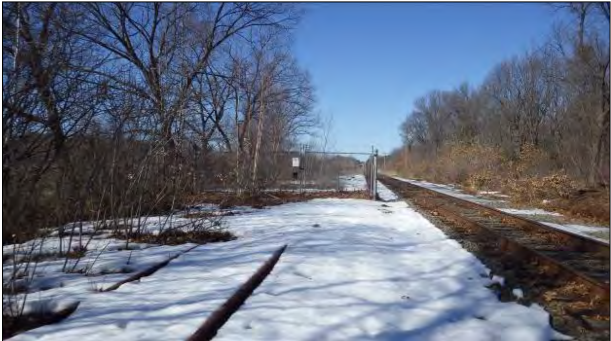
Figure 98 - A disused rail siding leading into the exclusion zone where the proposed Spit Brook Layover is situated, facing north.
