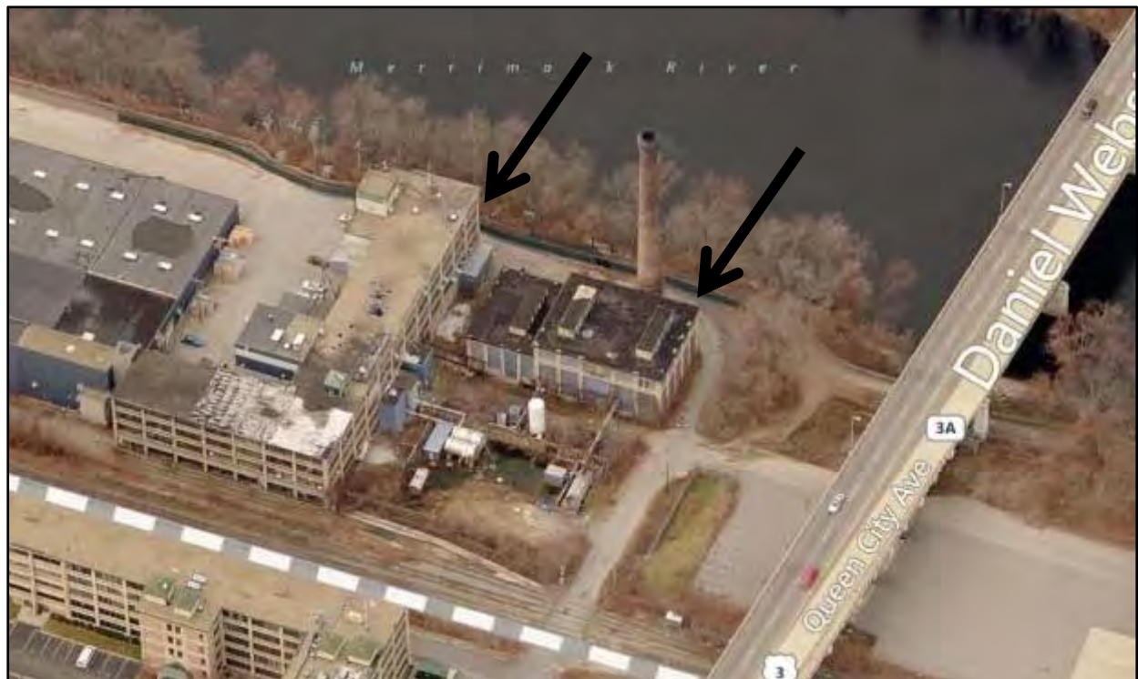
Photo 60. Indirect APE for Manchester Layover Facility, view west (on the south side of Queen City Bridge) showing two buildings over 50 years of age (Bing Maps)
