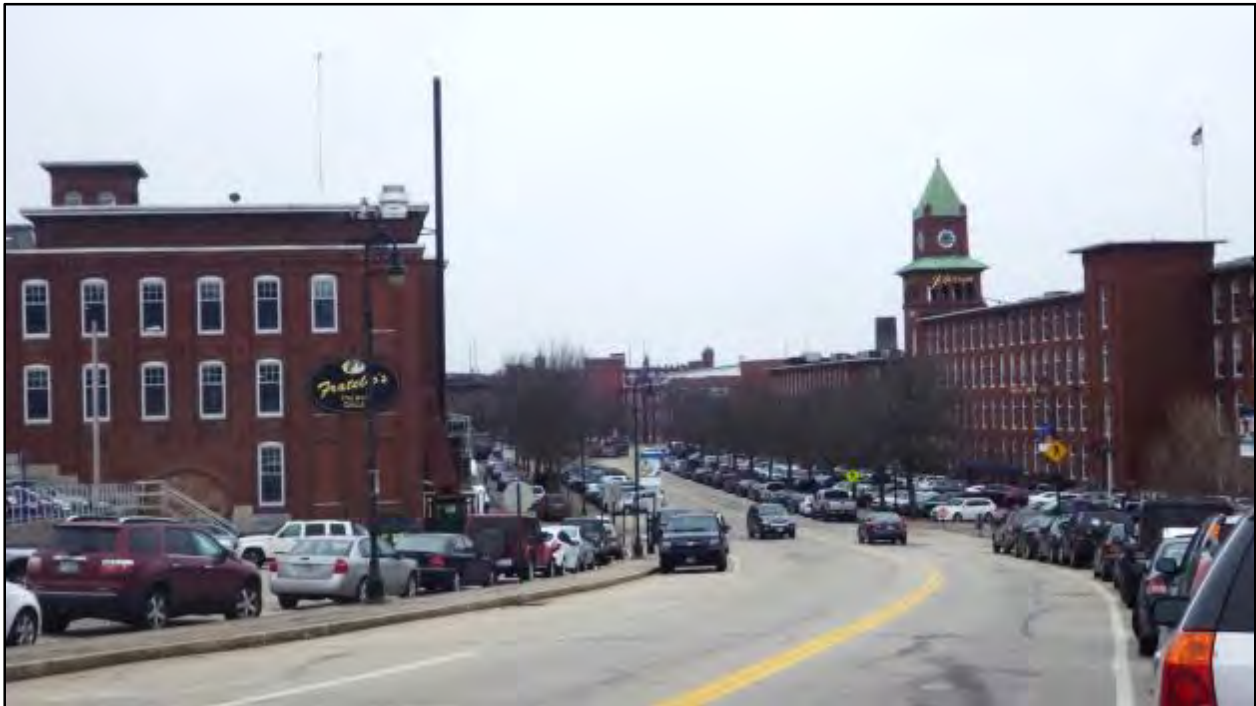
Photo 34. Amoskeag Millyard Historic District in Manchester (NRHP-eligible); view south on N. Commercial Street showing the Jefferson Mill (right), MAN1144.
