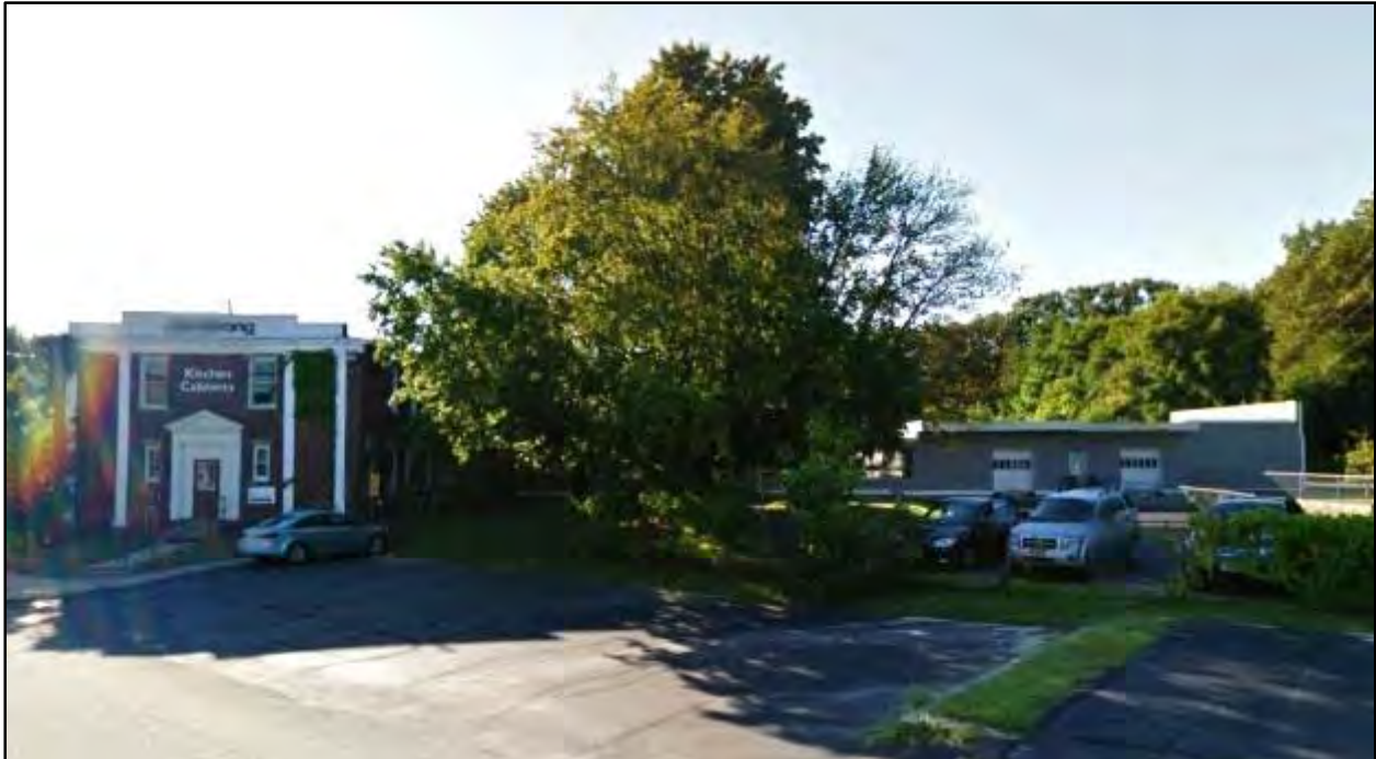
Photo 49. N-9 (left) and N-10 (right) in the Direct APE for Crown Street Station; view south from Crown Street (Google Earth August 2011)
