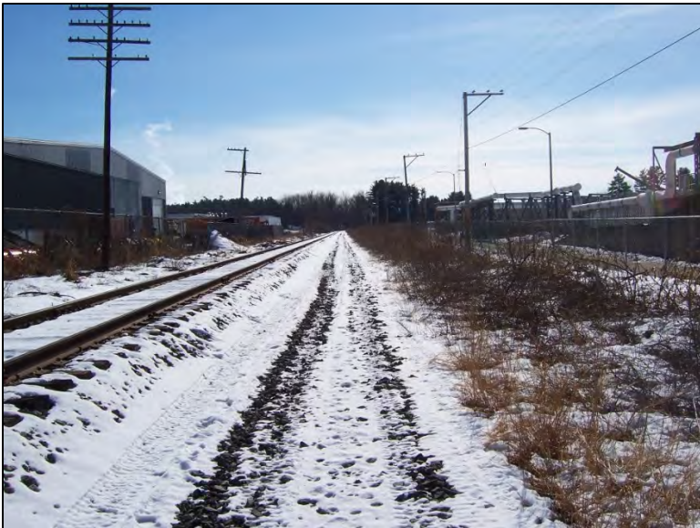
View north along existing rail line at Brown Avenue Layover Site in Manchester
