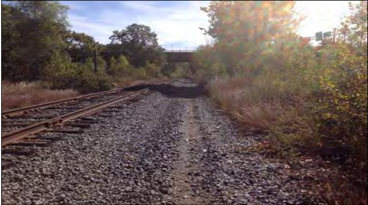
Figure 79 - MHT: Ray Wiczorek Drive Bridge Station APE, facing north toward the Ray Wiczorek Drive Bridge. The right-hand side of frame is a continuation of the railroad bed.
