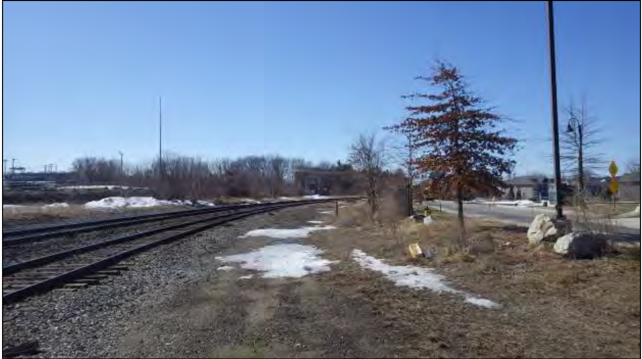
Figure 55 - View of the proposed Granite Street siding, facing south. The whole area is a former railroad siding, completely graded and covered in crushed stone ballast.
