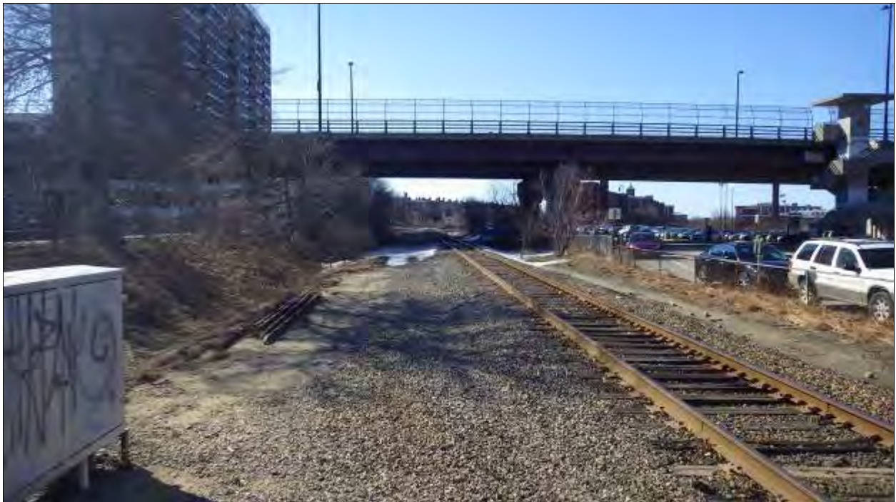
Figure 40 - Looking south from the Dow Street Rail crossing at the end of the Spring Street Station APE. In the background is the Bridge Street overpass, to the right is the parking area, and to the left is the drainage ditch that separates Canal Street from the railroad bed.
