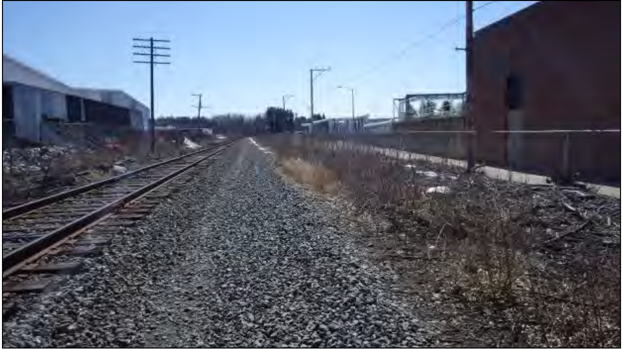
Figure 72 - View of the wide existing railroad bed, facing south. The Wastewater Treatment Plant is located along the right of frame.
