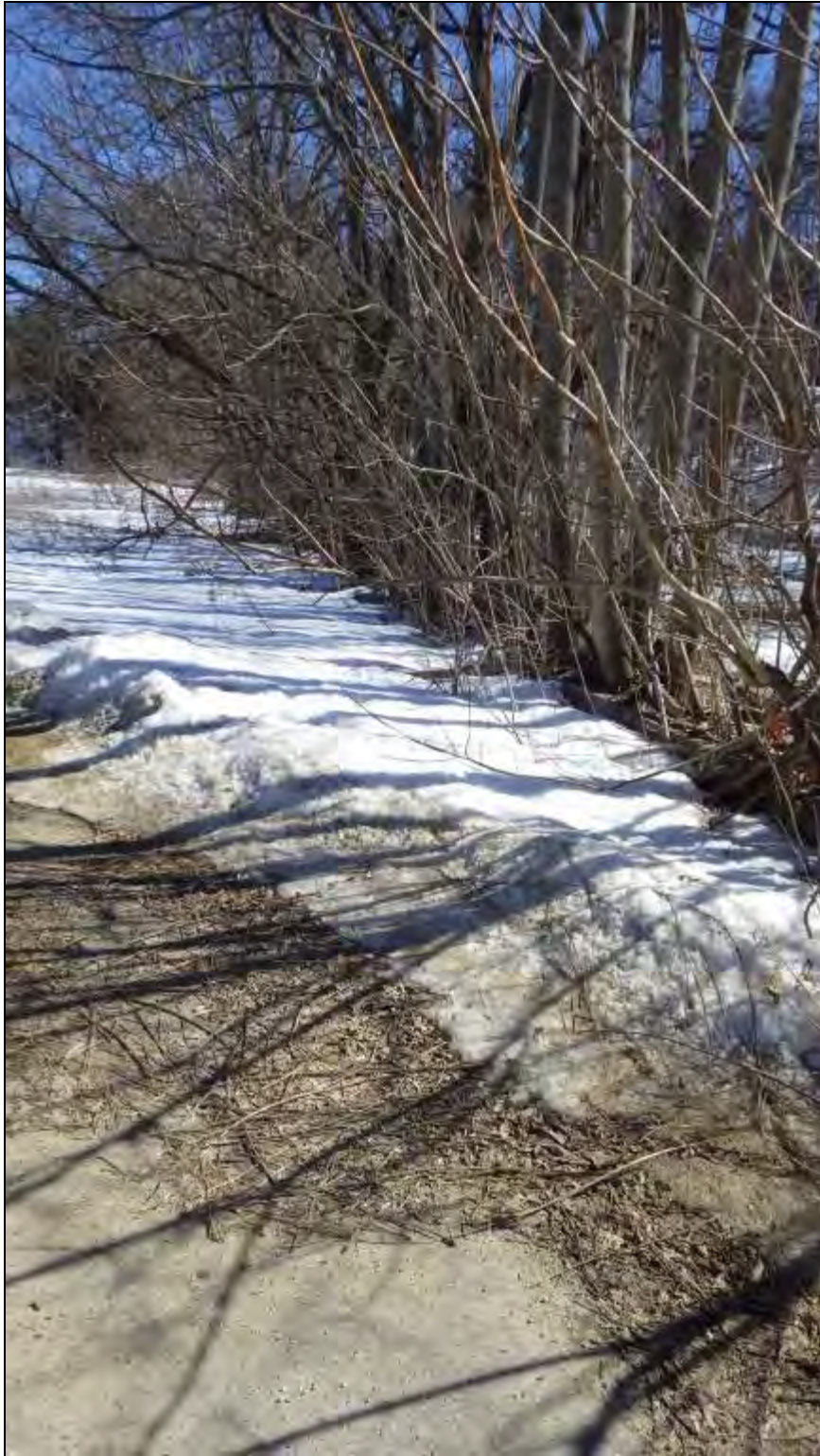
Figure 85 - Western foundation wall situated in the upper section of the proposed Crown Street parking area, facing south.
