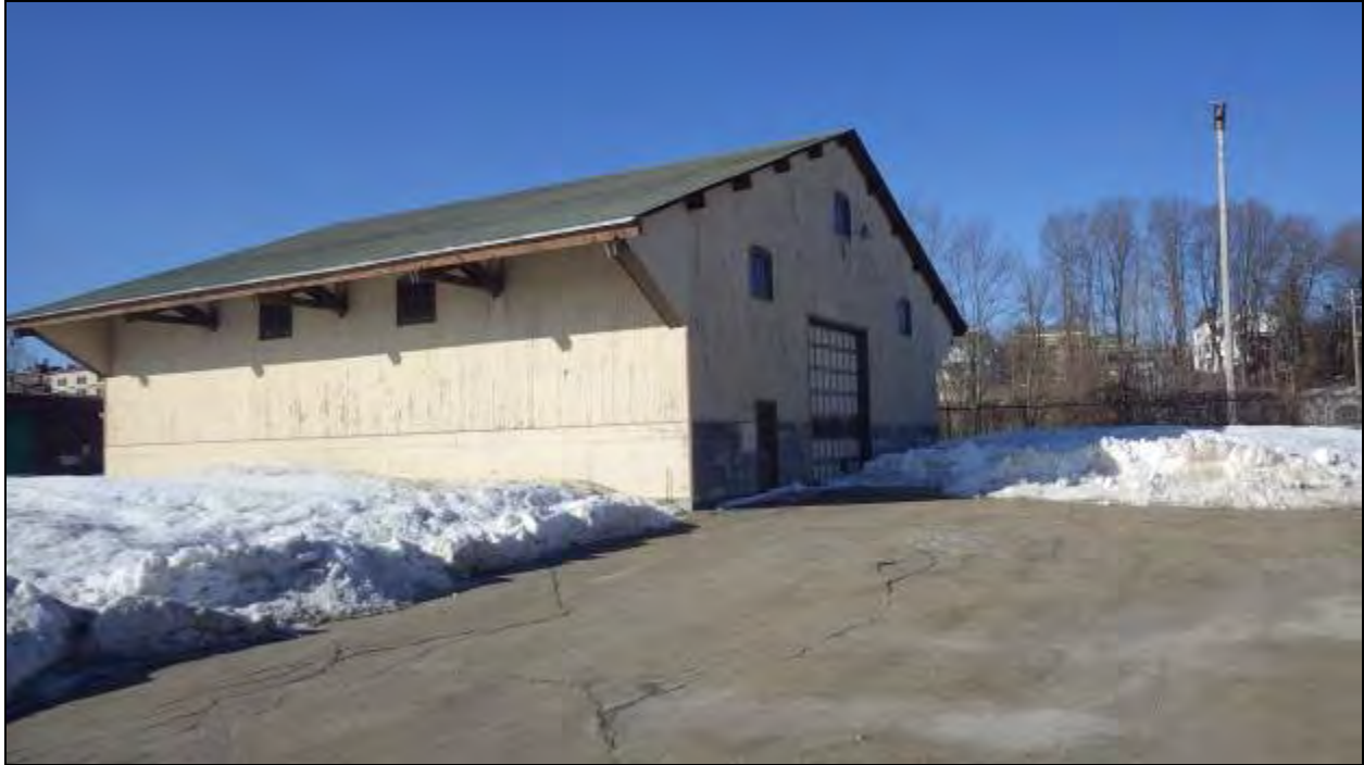
Figure 25 - Disused NH DOT garage, view facing west.
