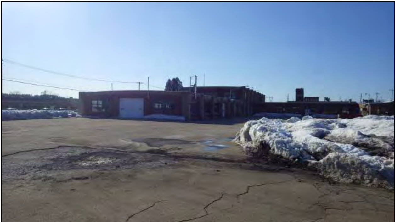
Figure 26 - View south toward a former NH DOT headquarters.
