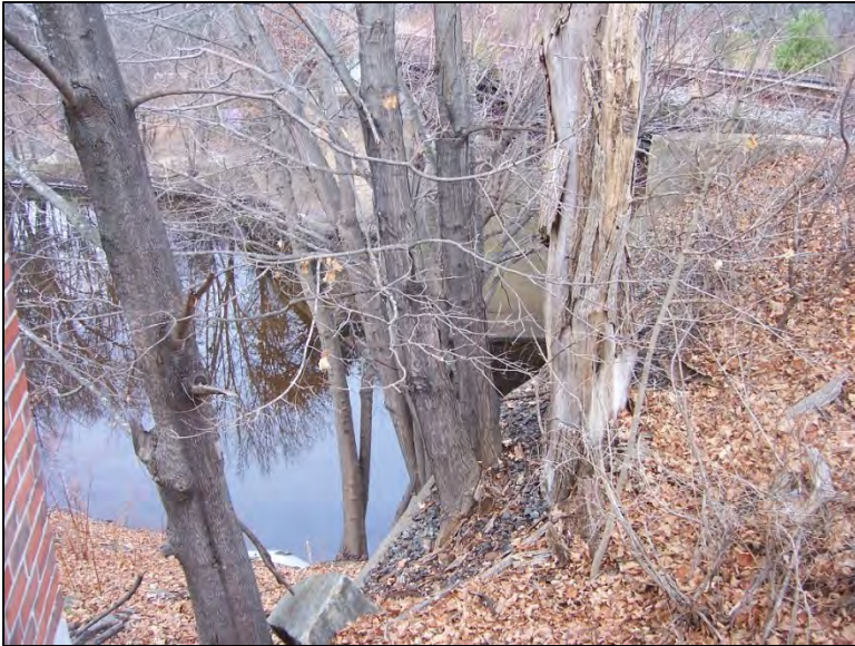
View of the Souhegan River crossing in Merrimack
