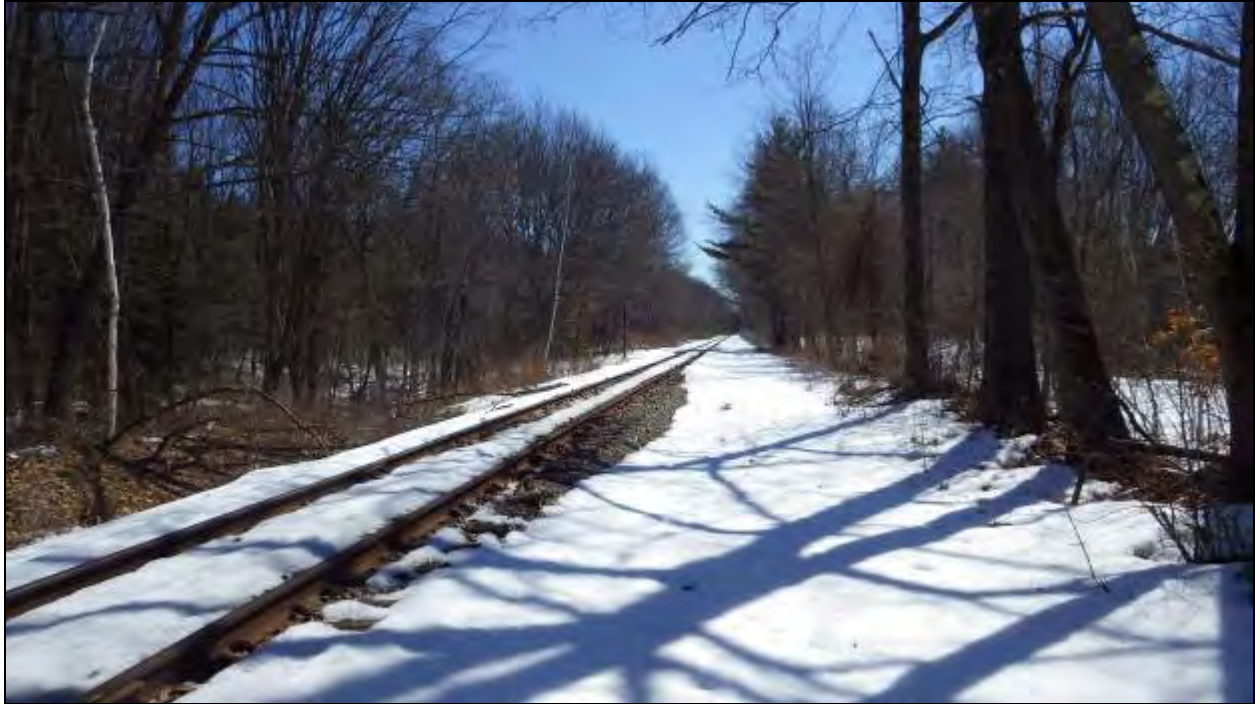
Figure 62 - View south from the northwestern edge of the APE, part of extant railroad bed.
