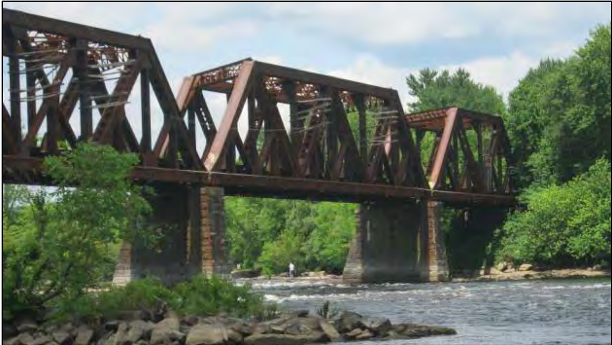
Photo 51. Goffs Falls Railroad Bridge (B-12); view south from the northern shore ( http://kayakthemerrimack.blogspot.com/ )
