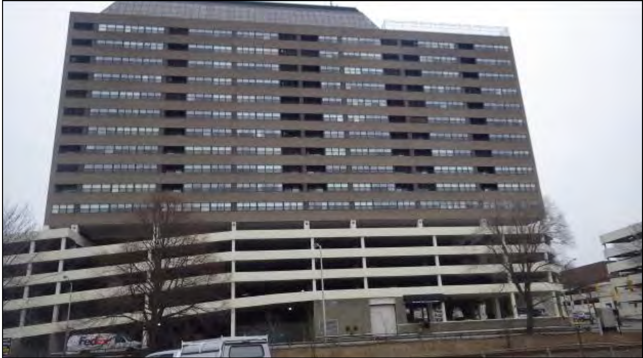
Figure 37 - View of the parking structure opposite the Spring Street end of the proposed station.
