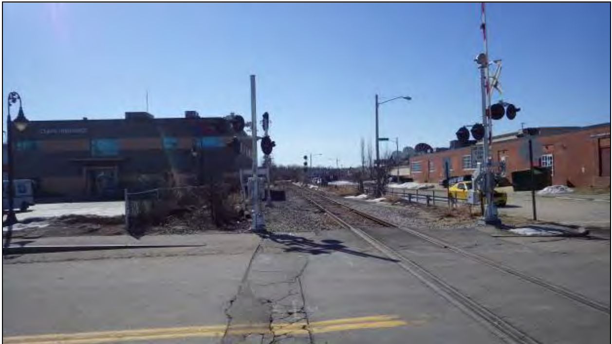
Figure 46 - View of the Granite Street Station APE, facing south from the Depot Street railroad crossing.
