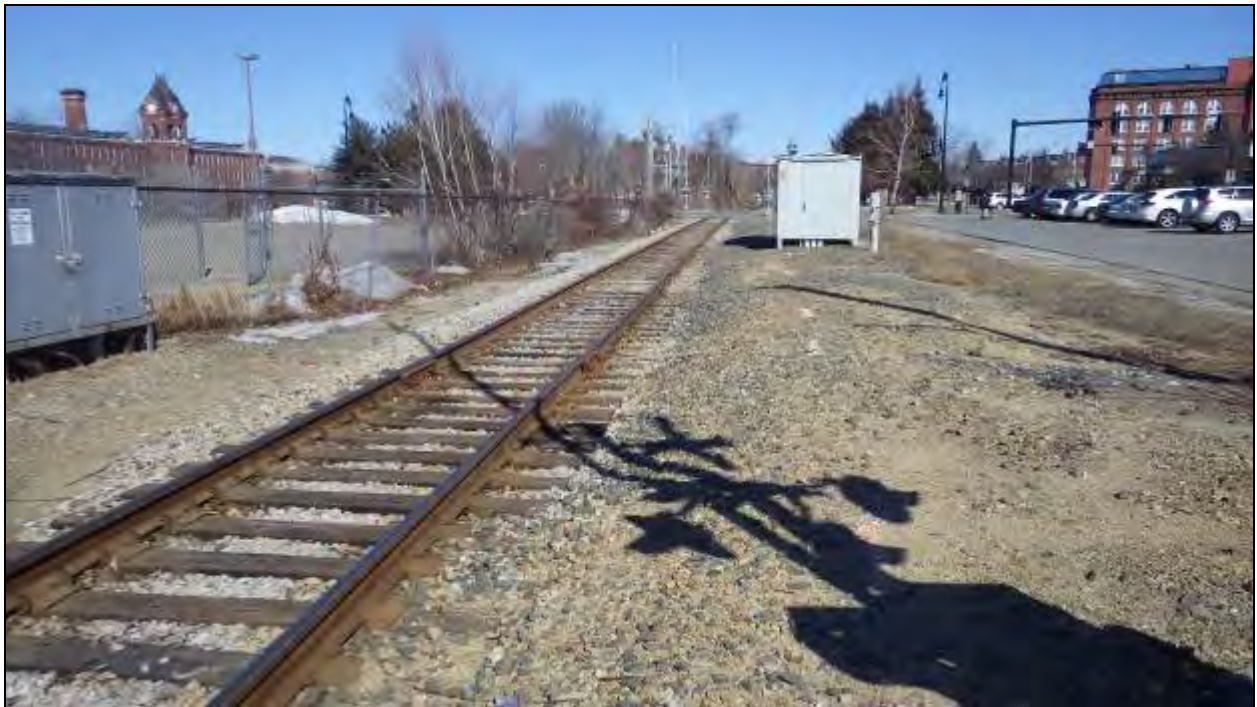
Figure 47 - View north from above the Granite Street road crossing.
