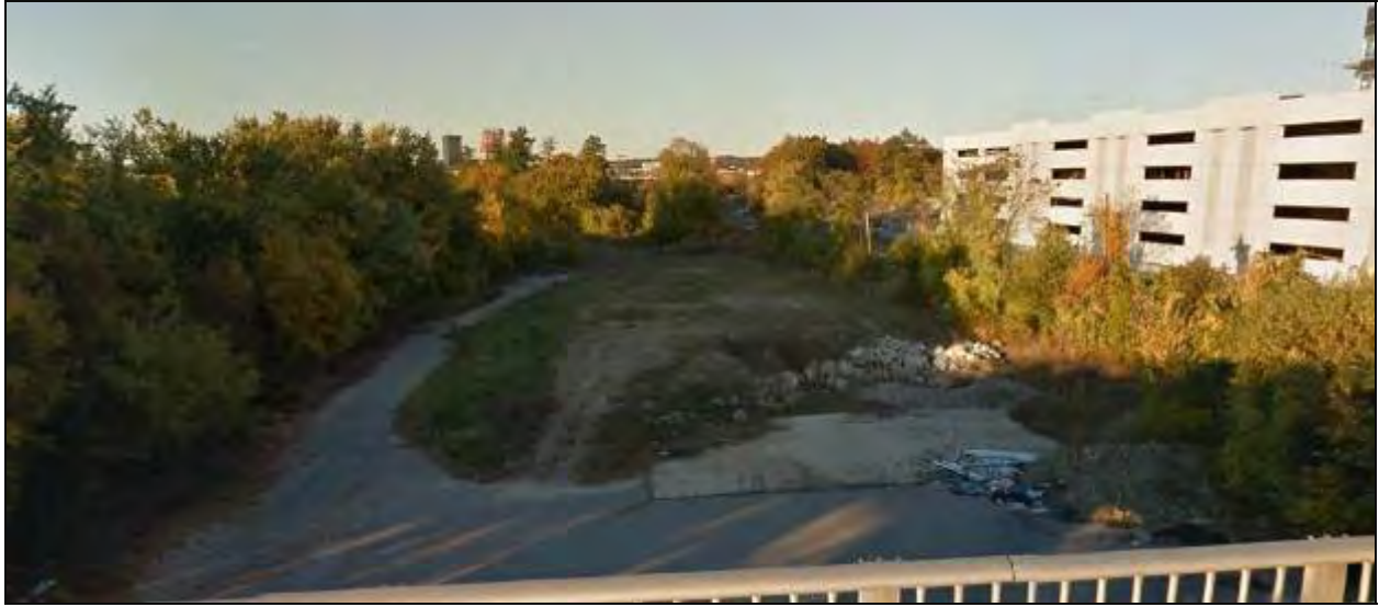
Figure 69 - View of the Queen City Bridge Layover APE, facing north.
