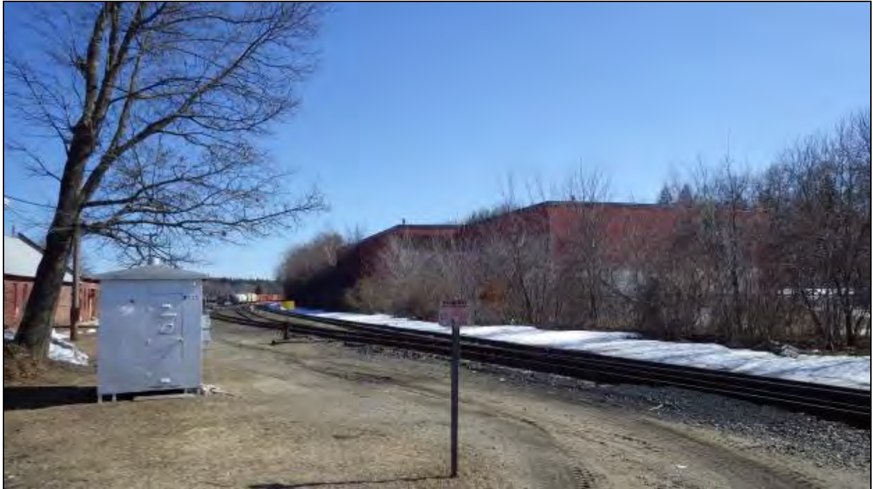
Figure 82 – Crown Street Station APE facing the location of the proposed station from the opposite side of the tracks. A disused warehouse occupies the right of frame and the far background contains the Pan America rail yard.
