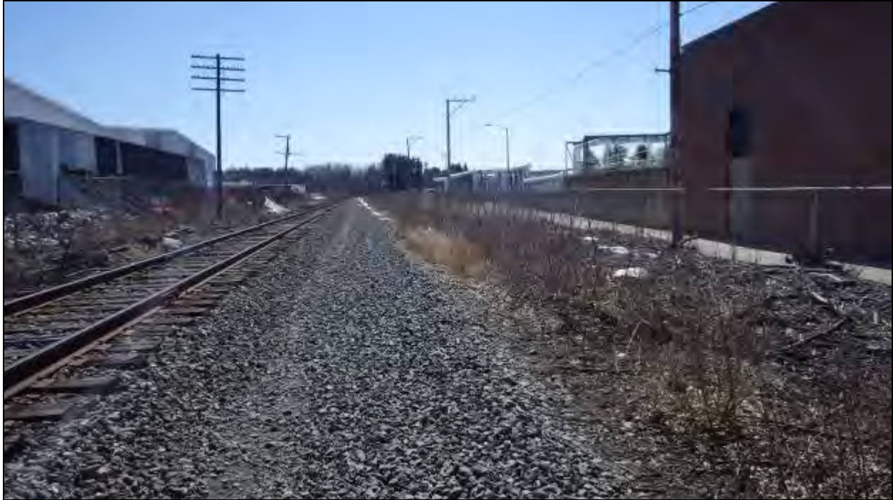
Figure 72 - View of the wide existing railroad bed, facing south. The Wastewater Treatment Plant is located along the right of frame.
