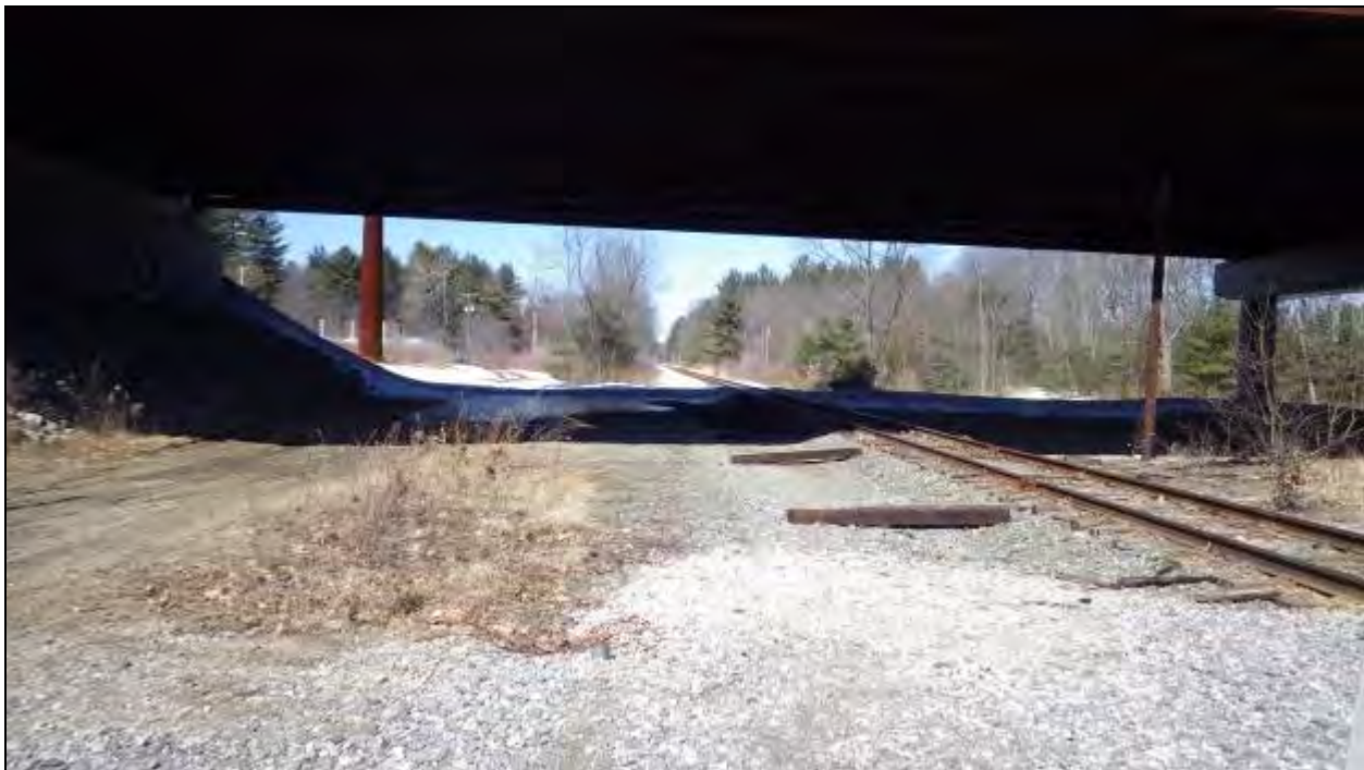
Figure 80 - MHT: Ray Wiczorek Drive Bridge Station APE, looking south under the bridge. The APE is comprised of the railroad bed and the area to the left of frame was disturbed by the recent bridge construction.
