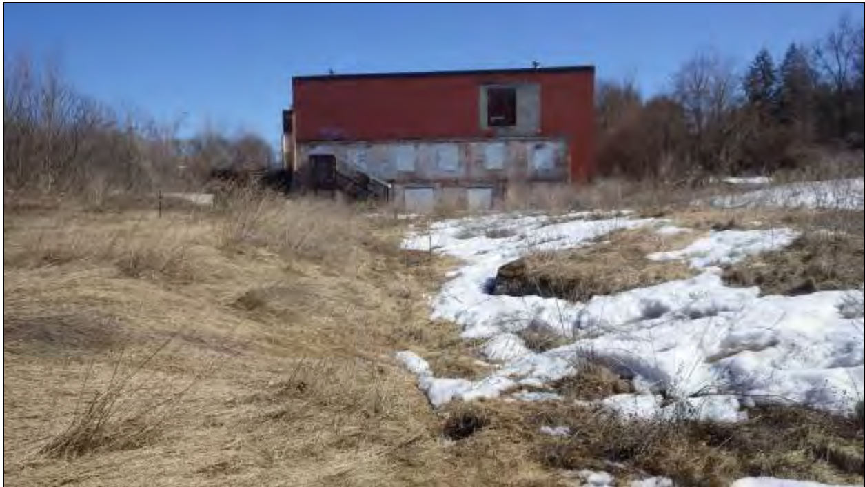
Figure 93 - A drainage ditch in the middle of an old building foundation, facing south.
