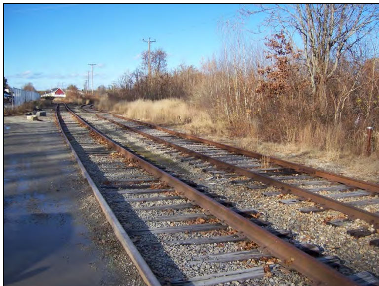
View north along existing rail line at Stickney Avenue Station/Layover Site in Concord
