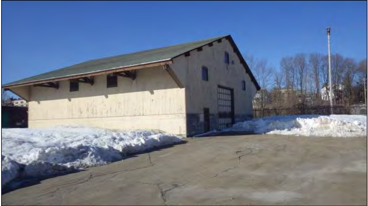
Figure 25 - Disused NH DOT garage, view facing west.
