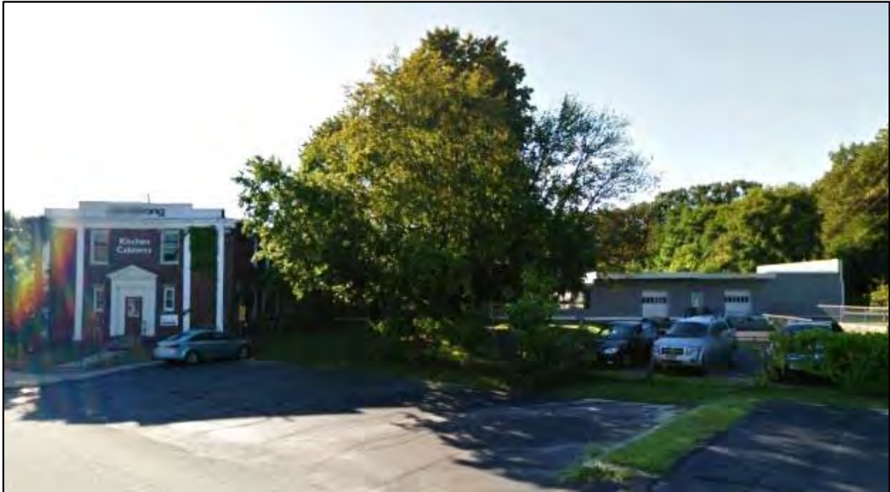
Photo 49. N-9 (left) and N-10 (right) in the Direct APE for Crown Street Station; view south from Crown Street (Google Earth August 2011)
