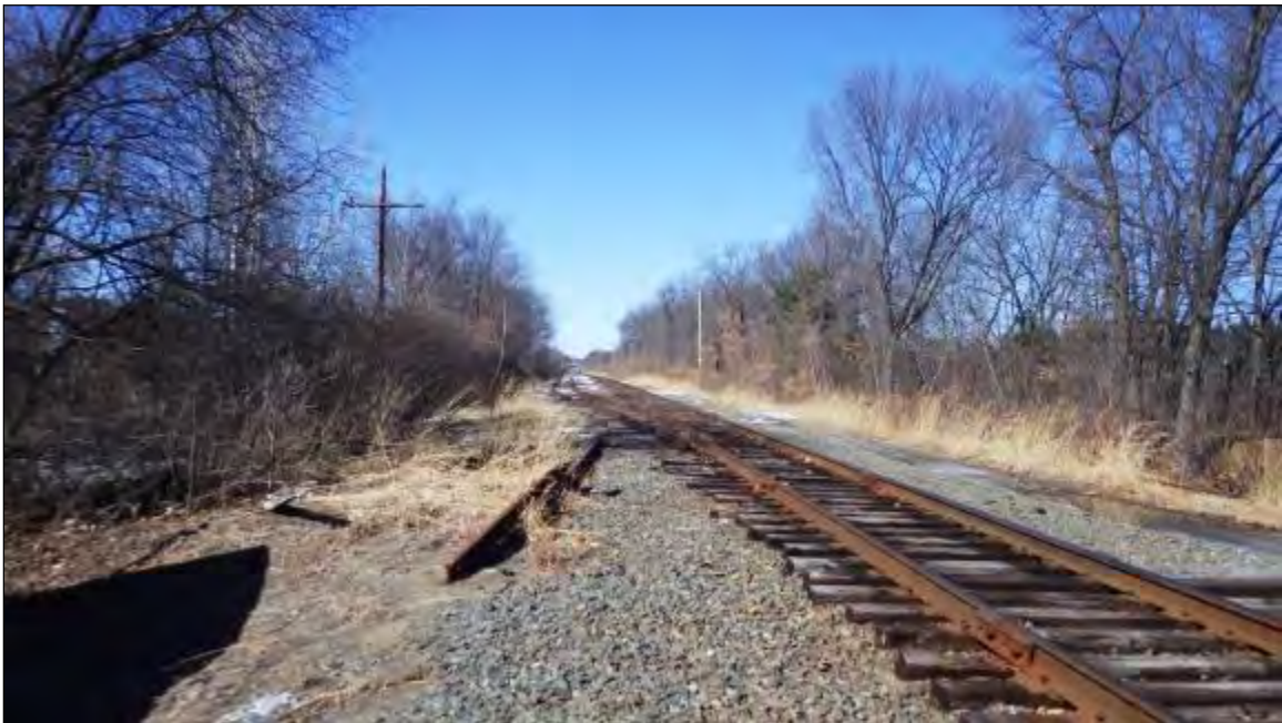
Photo 22. Proposed Spit Brook station/layover location; view north along the right-of-way from Spit Brook Road
