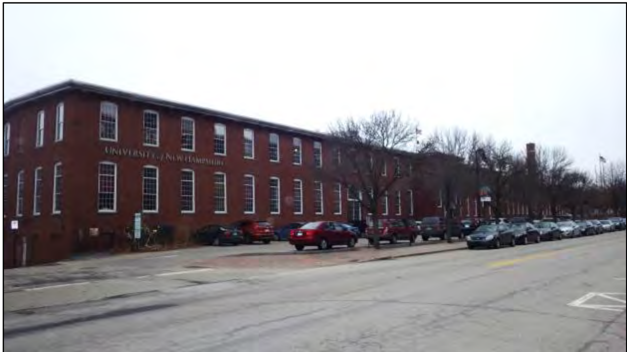
Photo 36. Amoskeag Millyard Historic District in Manchester (NRHP-eligible); view north on Commercial Street showing the Amoskeag Machine Shop (MAN1059)
