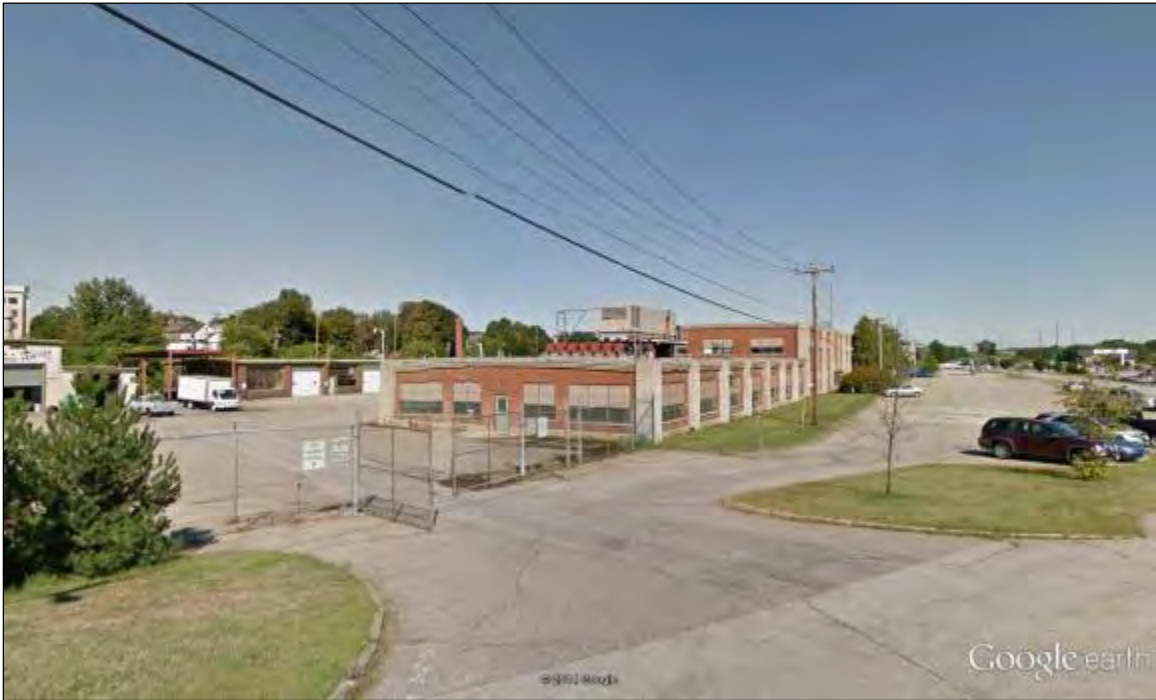
Photo 1. Proposed Stickney Avenue station location; view north showing existing buildings on parcel (Google Earth, August 2011)
