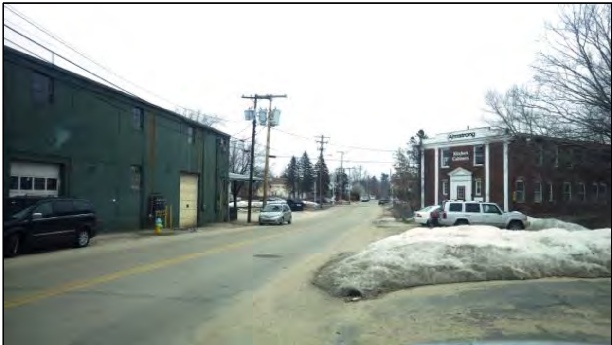
Photo 48. N-9 (right) in the Direct APE for Crown Street Station; view south from Crown Street.
