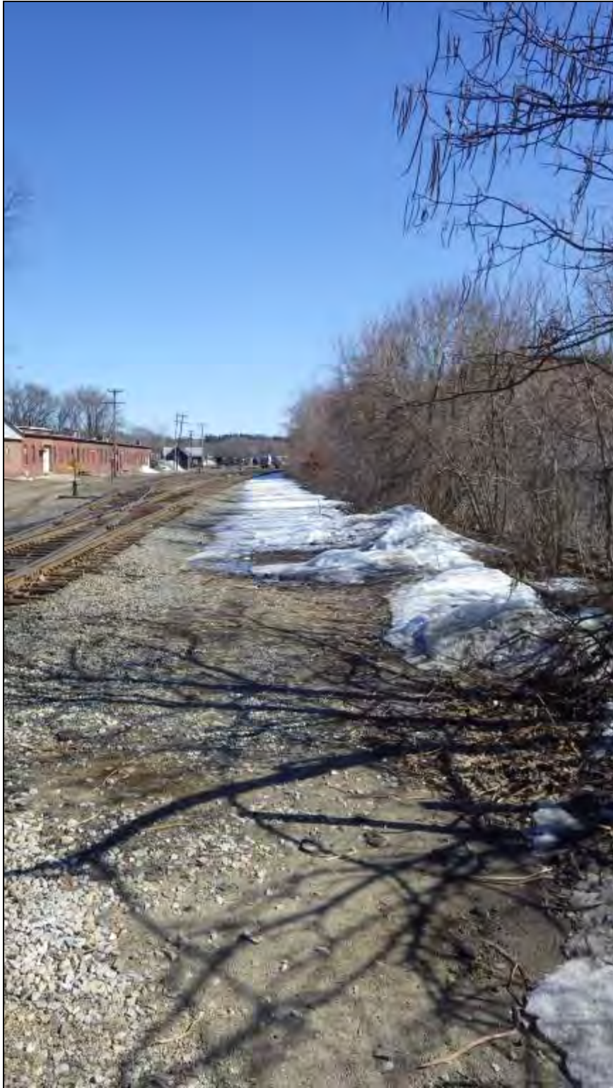
Figure 83 – The location of Crown Street Station platform, facing south. The platform location is a road bed made of crushed stone ballast.
