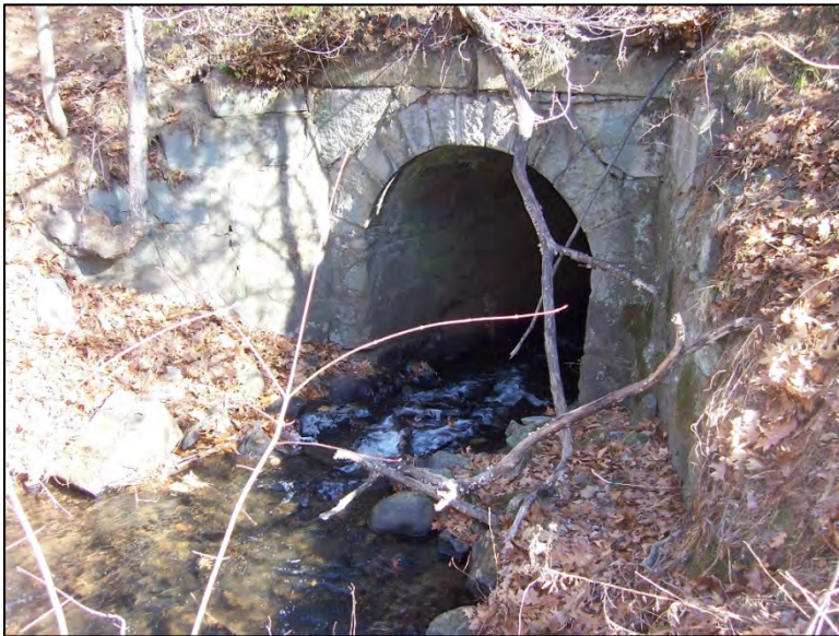
View of Sebbins Brook crossing under existing rail line at Raymond Wieczorek Drive (MHT) Station Site in Bedford
