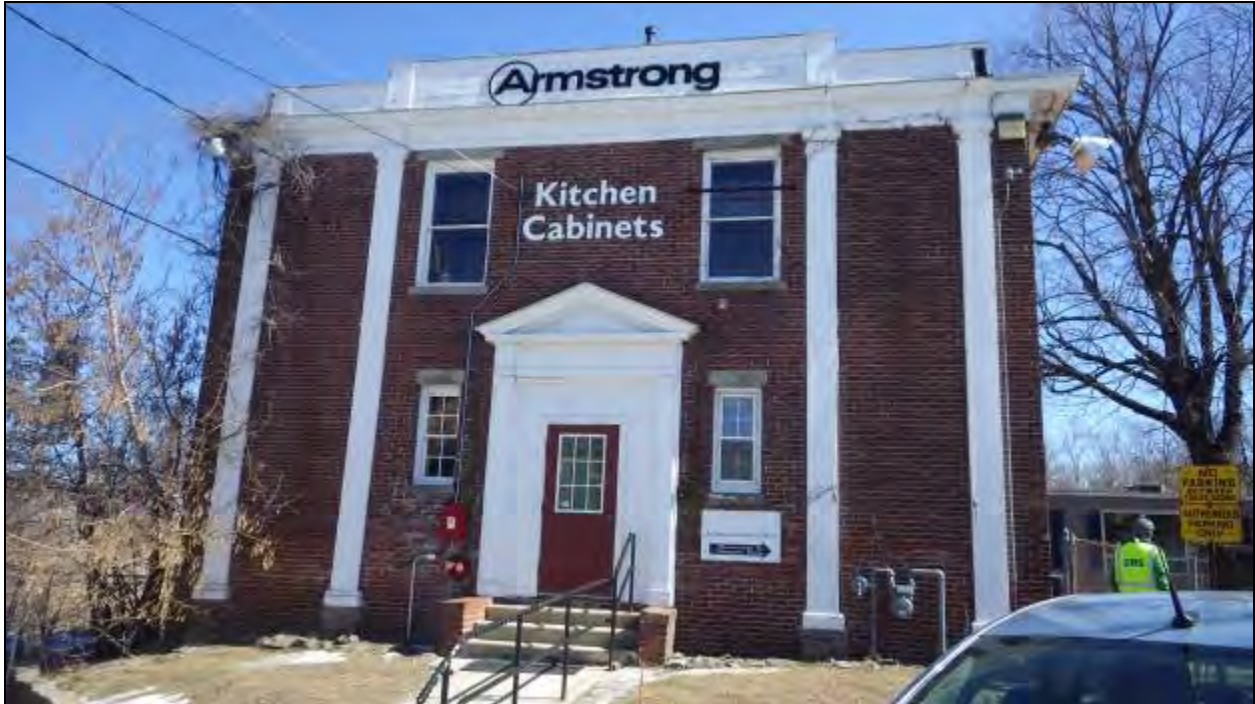
Figure 94 - Front of a structure to the west of rail line on Crown Street, facing southeast.
