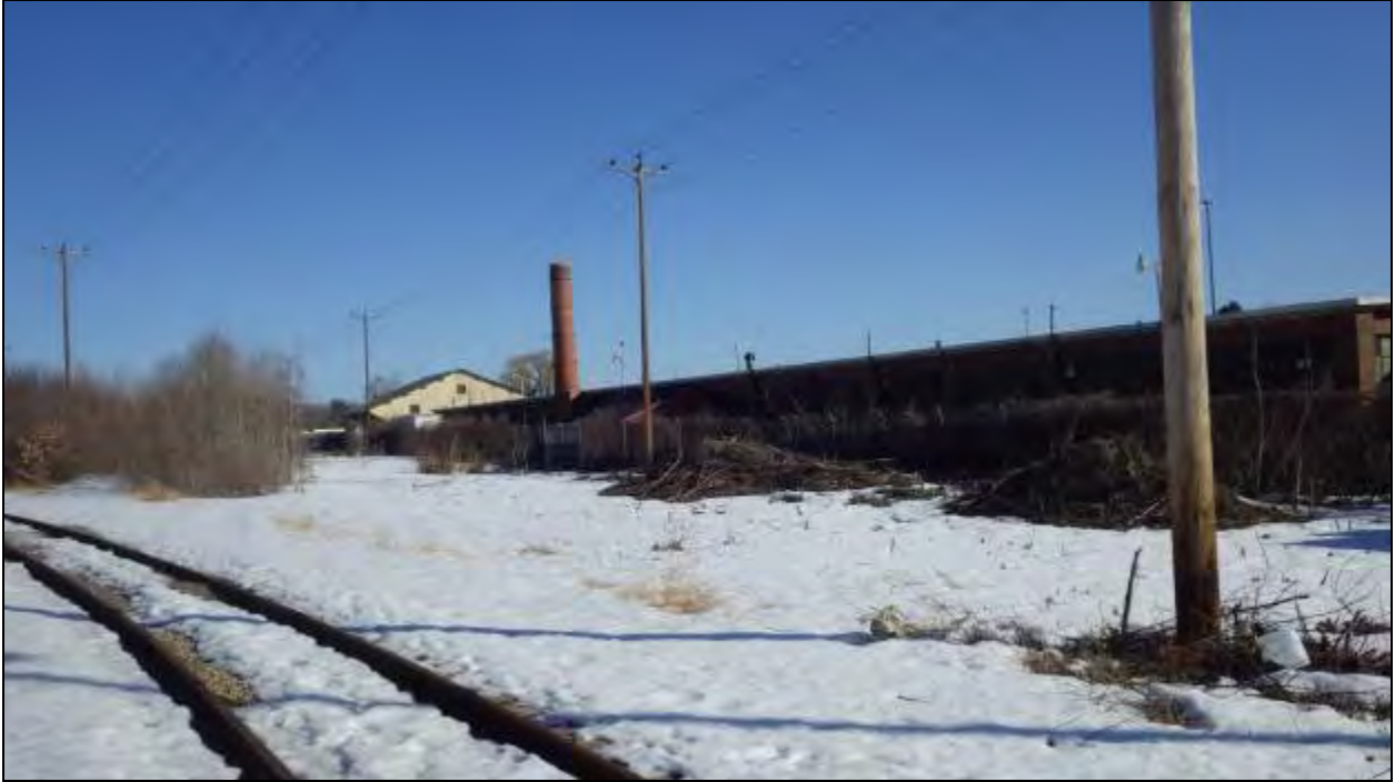
Figure 35- View of the APE, facing northeast.
