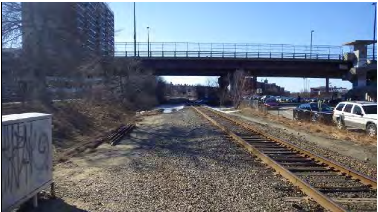
Figure 40 - Looking south from the Dow Street Rail crossing at the end of the Spring Street Station APE. In the background is the Bridge Street overpass, to the right is the parking area, and to the left is the drainage ditch that separates Canal Street from the railroad bed.
