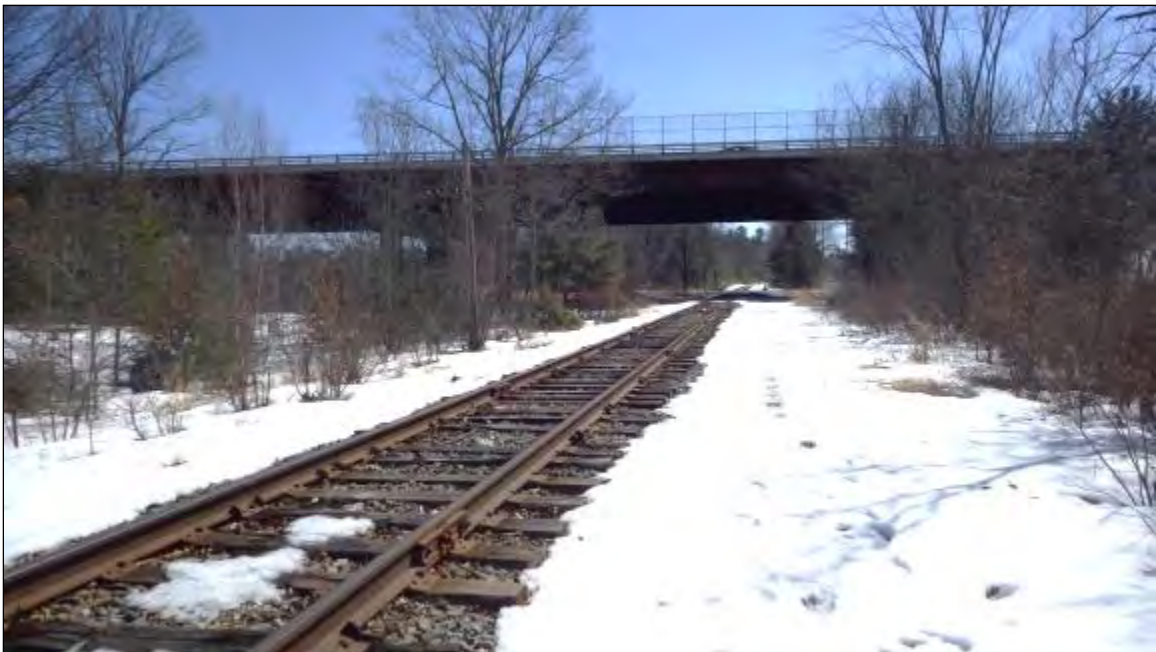
Photo 16. Proposed Ray Wieczorek Drive station location; view north along the right-of-way from the south side of the Ray Wieczorek Drive bridge
