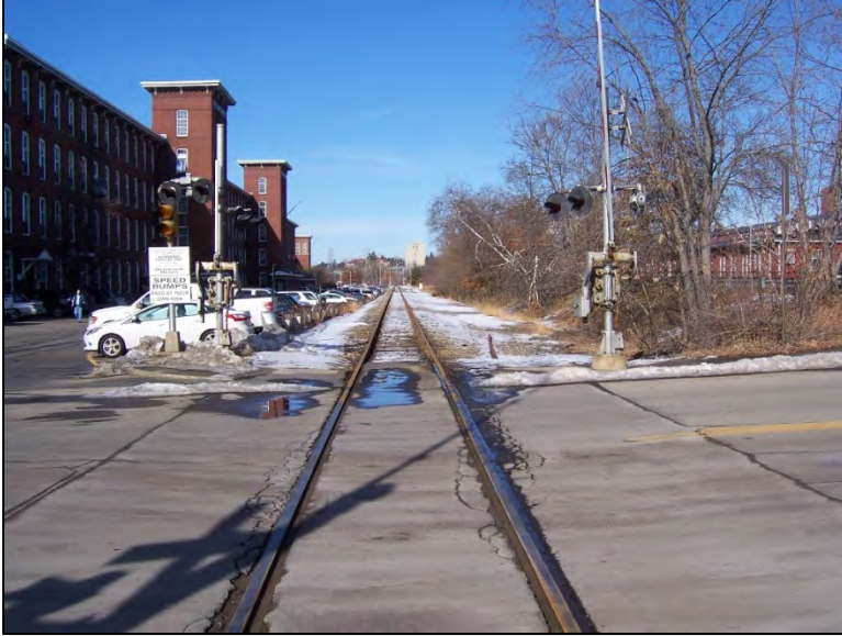
View north along existing rail line at Bridge Street Station Site in Manchester
