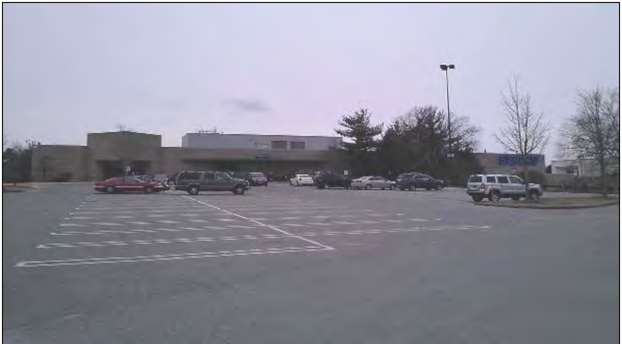
Figure 105 - Location of the Pheasant Lane Mall Station parking structure. This location is currently overflow-parking for Sears.
