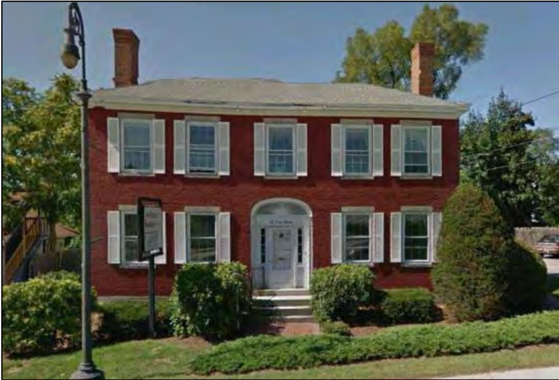
Photo 31. French-Thompson House, Concord (NRHP-eligible); view west from Water Street (Photo credit: Google Earth August 2011)
