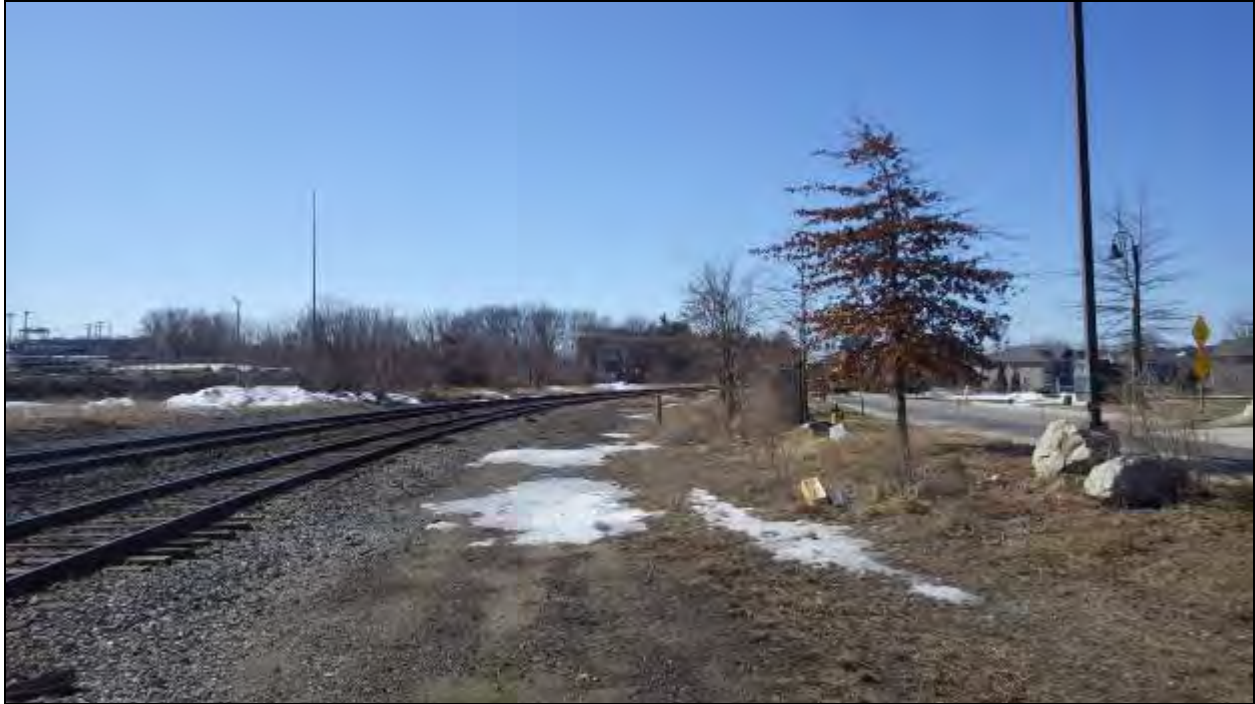
Figure 55 - View of the proposed Granite Street siding, facing south. The whole area is a former railroad siding, completely graded and covered in crushed stone ballast.
