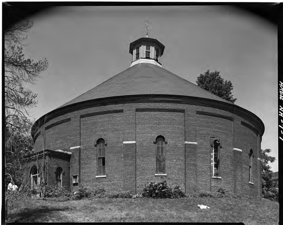
Photo 30. NRHP-eligible Gasholder House, Concord Gas Co. (Photo credit: Gary Samson 1982)
