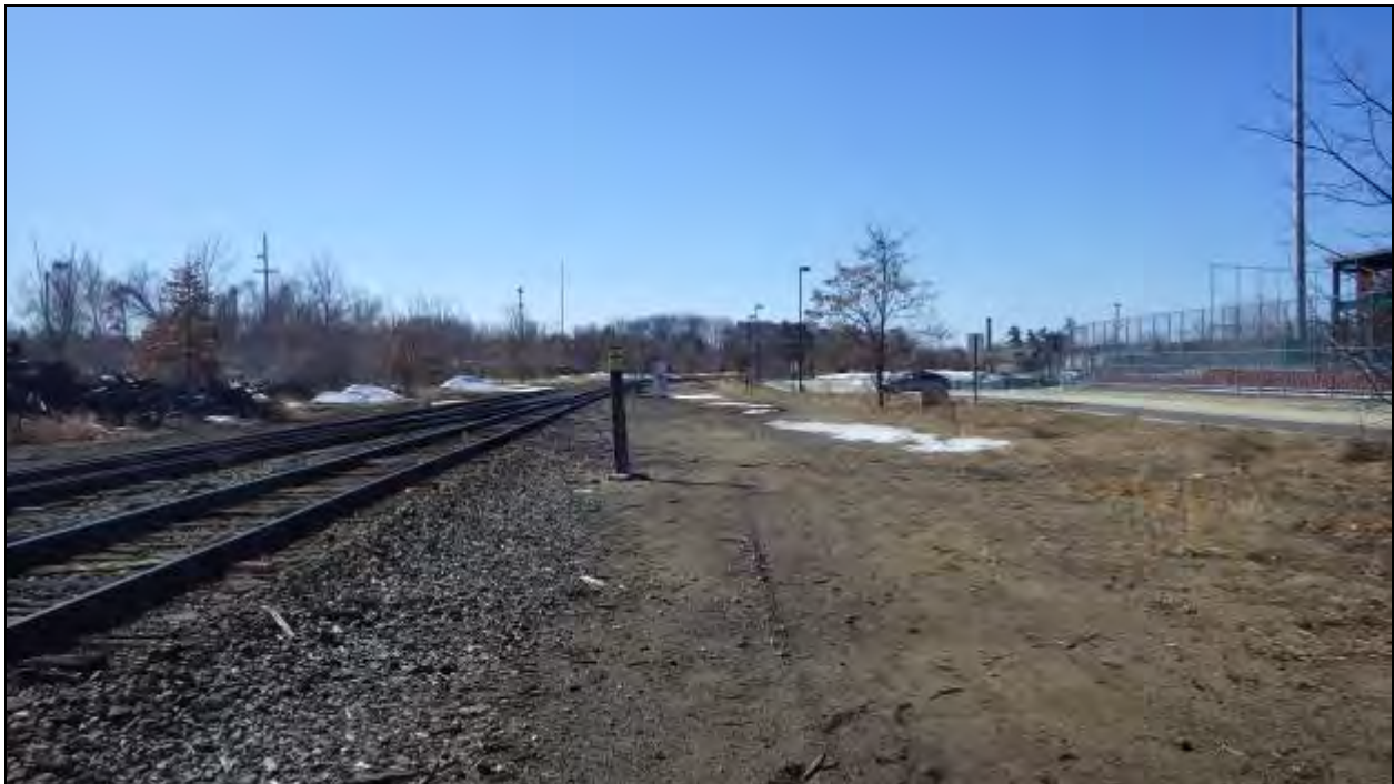
Figure 56 - View of the proposed Granite Street siding, facing south.
