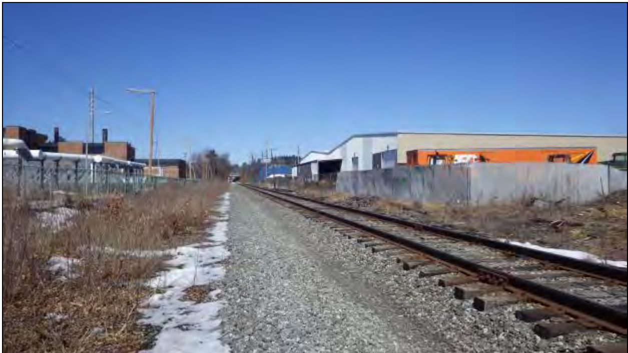
Figure 73 - Wastewater Treatment Plant Layover APE, facing north. The Wastewater Treatment Plant is located in the left of frame and a warehouse complex is located in the right of frame.
