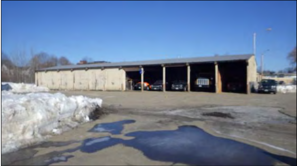
Figure 27 - View of NH DOT garage facing north.
