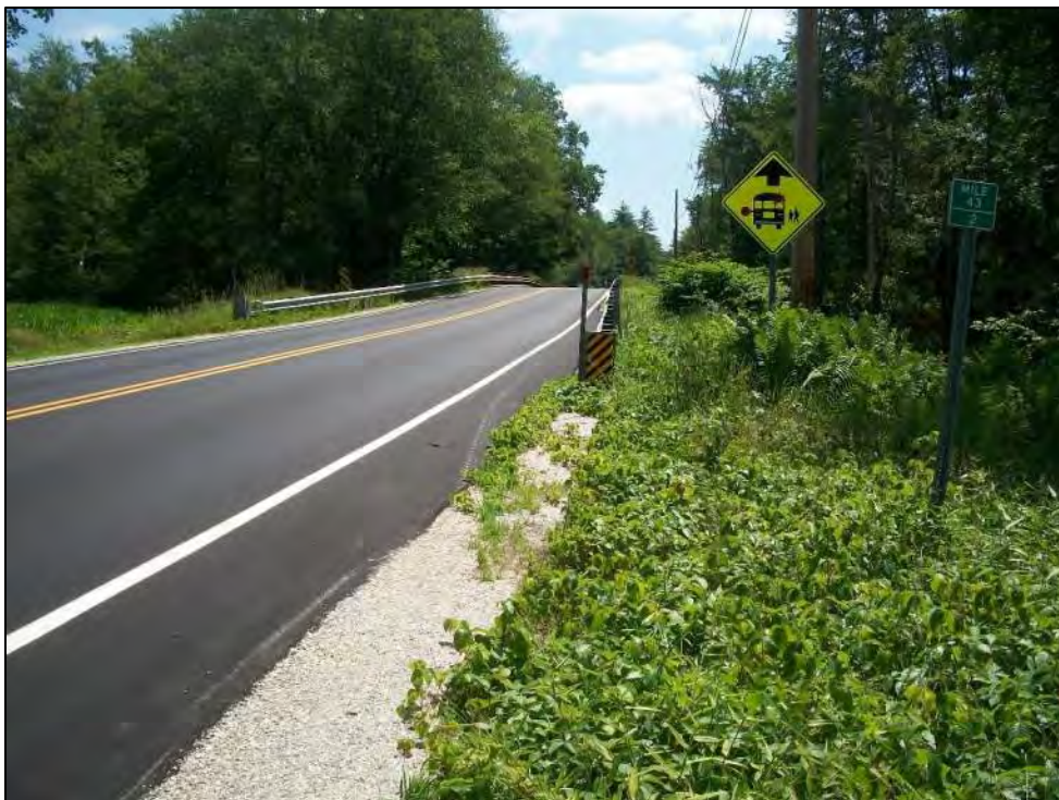
Photo 10. View southeast toward Bridge No. 143/077. Photo taken on 7/19/2019.
