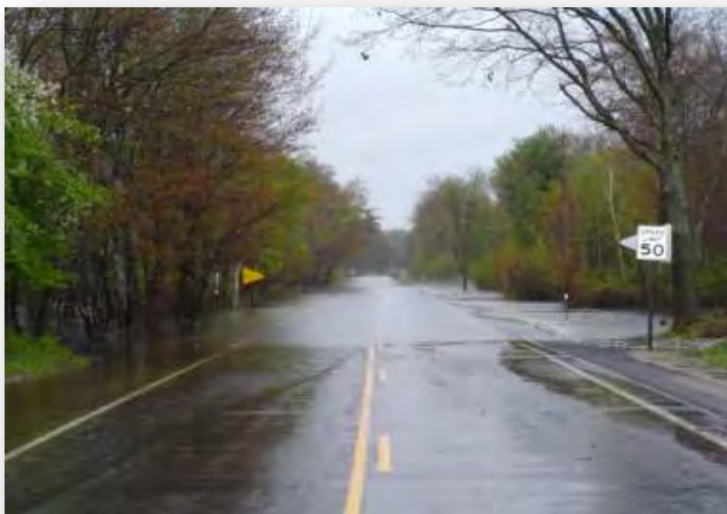
US Route 4 Looking Southeast: Water Over Roadway – Road Closed and Barricaded (May 16, 2006)
