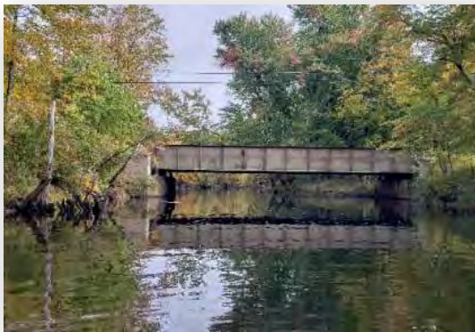
Downstream (South) Elevation
