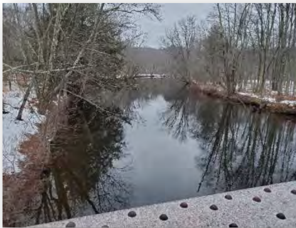
Blackwater River Downstream of US Route 4 Bridge
