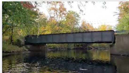
Upstream (North) Elevation
