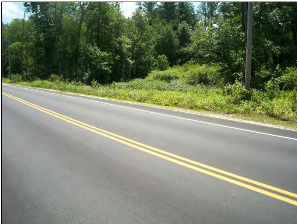
Photo 6. View south toward Prime Wetland Impact Areas T and U (Wetland 7), located in the southeast bridge quadrant. Photo taken on 7/19/2019.
