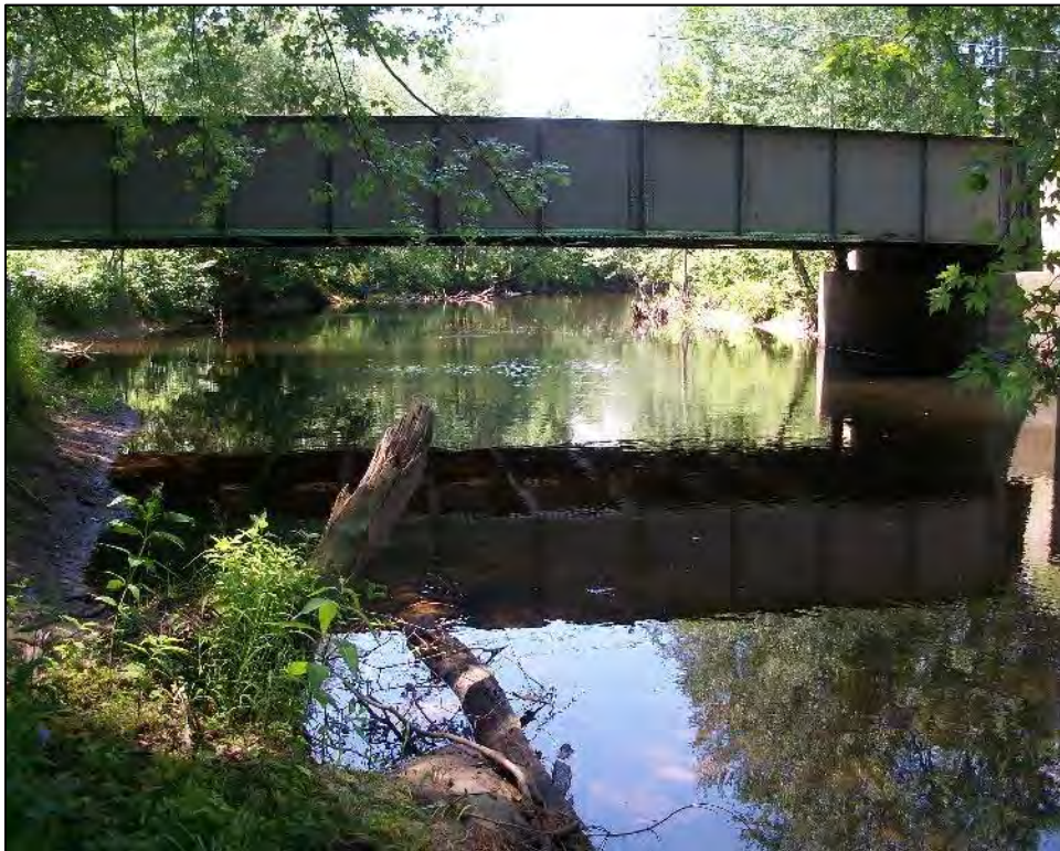
Blackwater River, view downstream toward bridge Photo taken 7/19/19
