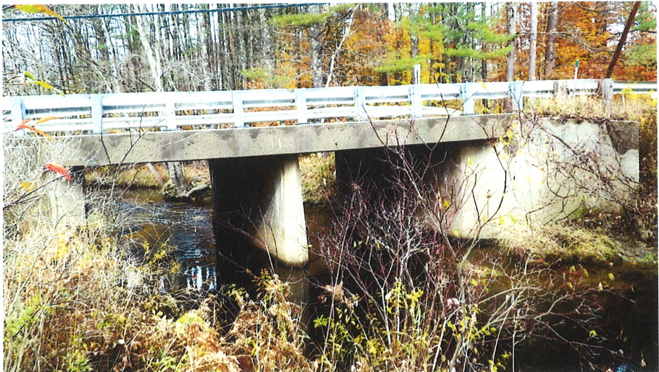
Figure 8: Elevation of structure (10/2014).
