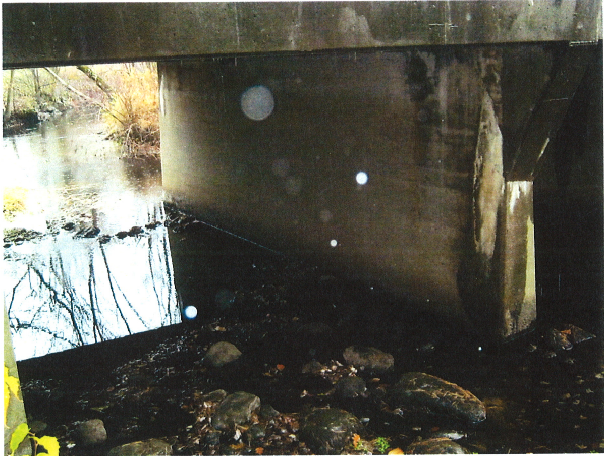
Figure 7: Pier to be removed (10/2013).
