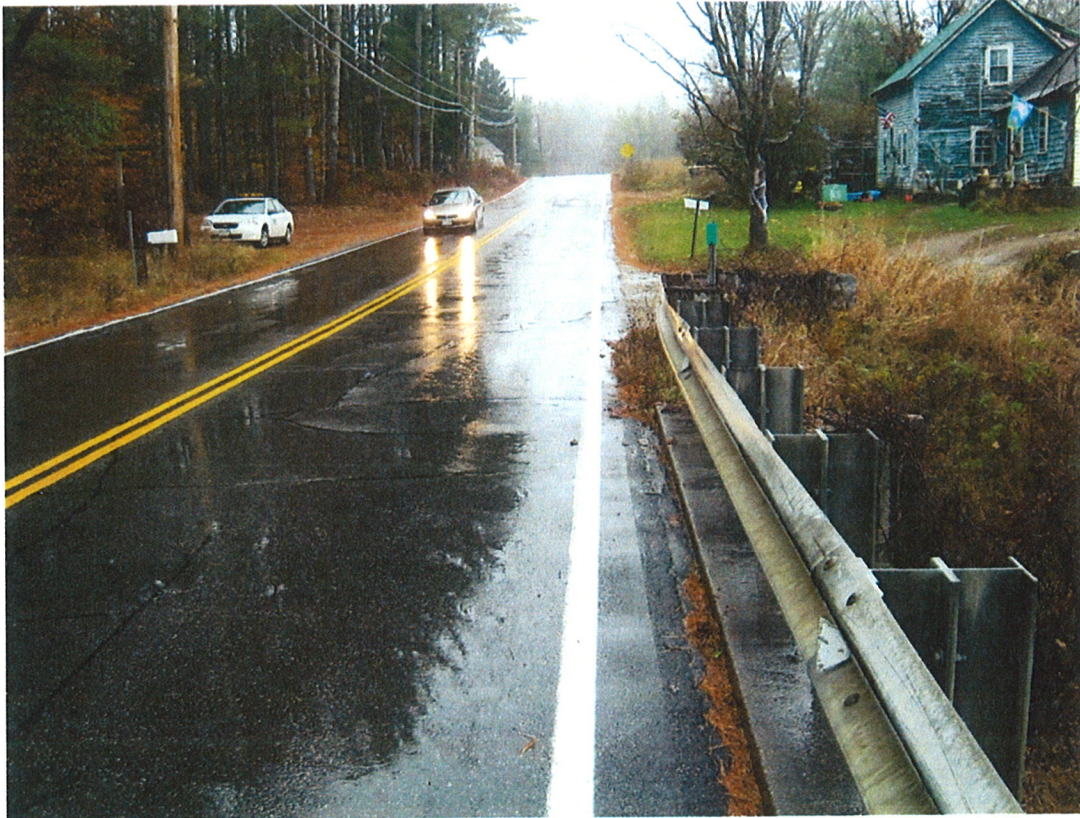
Figure 1: Fowler River Road over structure looking towards Bristol (10/2013).
