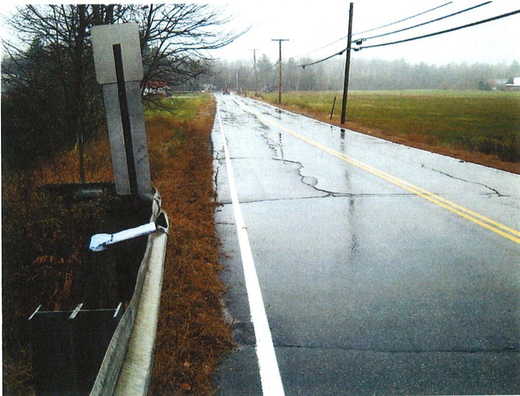
Figure 2: Fowler River Road over structure looking towards Alexandria (10/2013).
