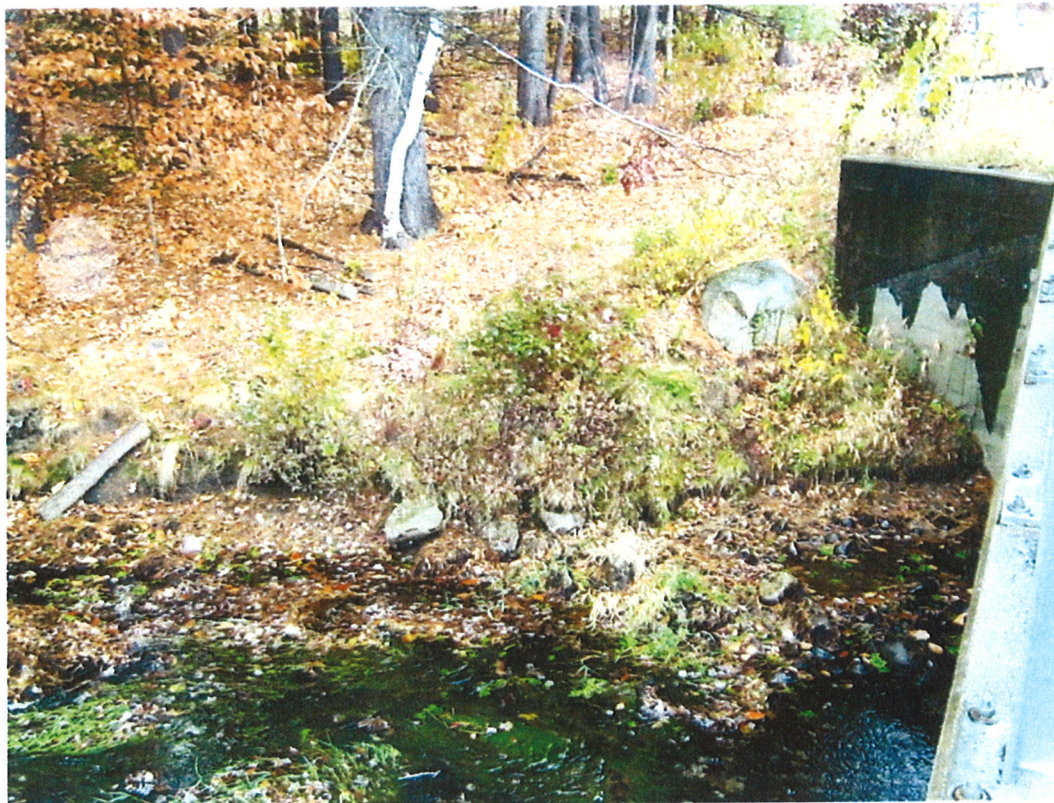
Figure 3: NE side to be widened (10/2013).
