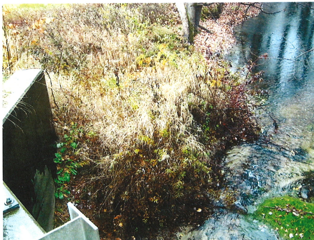
Figure 4: NW side to be widened (10/2013).
