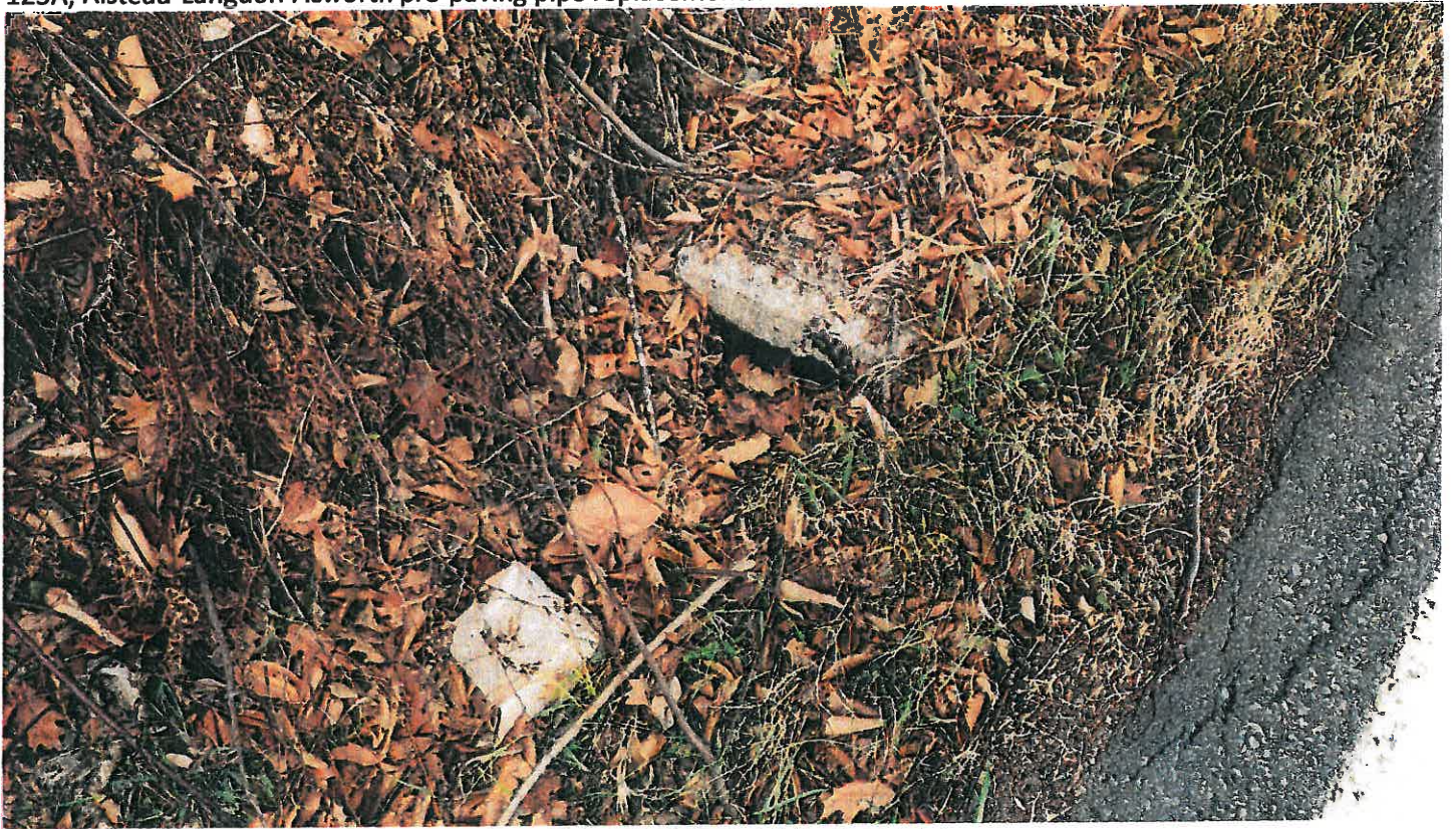
Pipe #21, 12" CMP, Catch basin at inlet.
