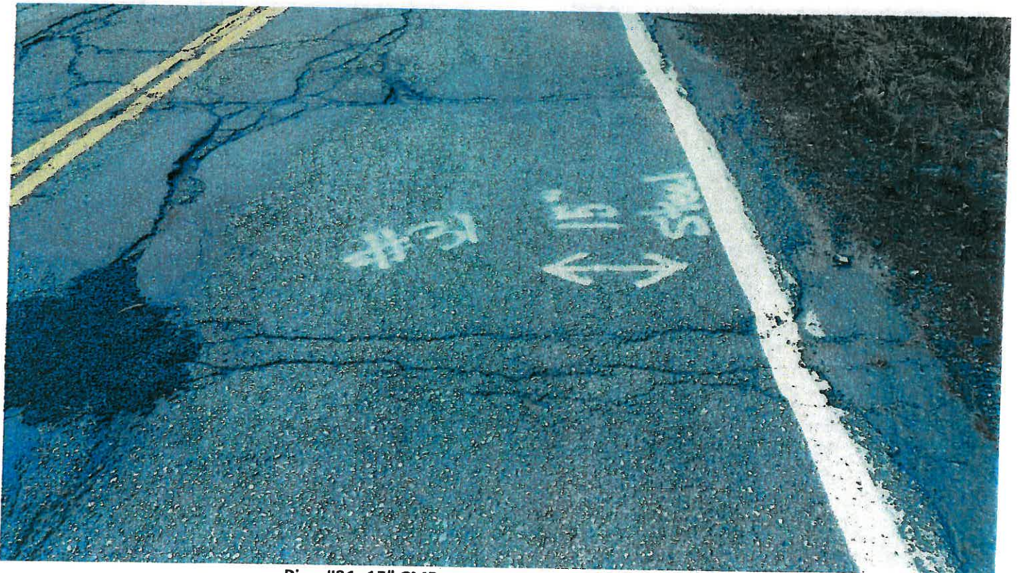
Pipe #31, 15" CMP, pavement condition at crossing.
