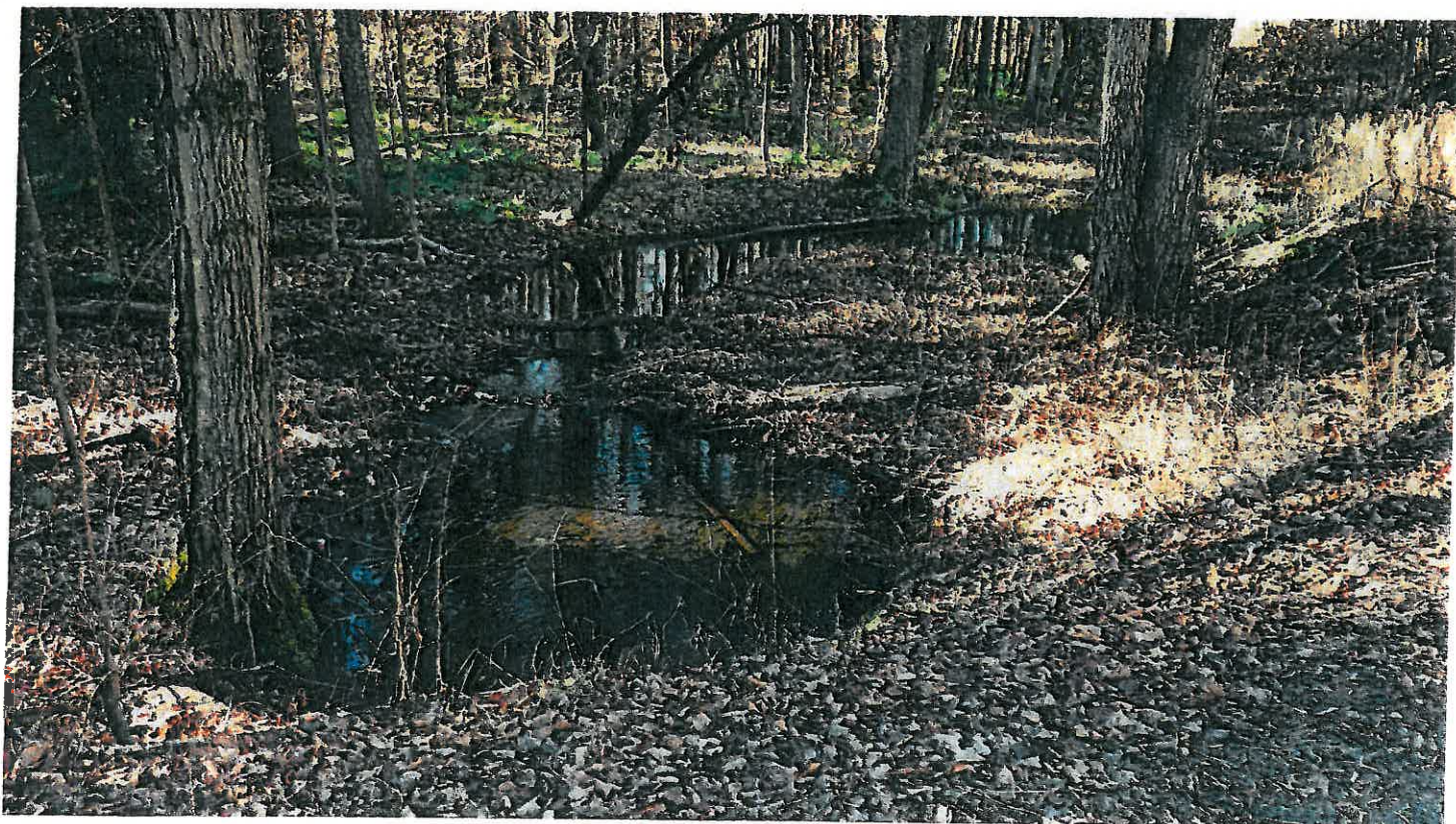
Pipe #27, 18" CMP, Looking at outlet.
