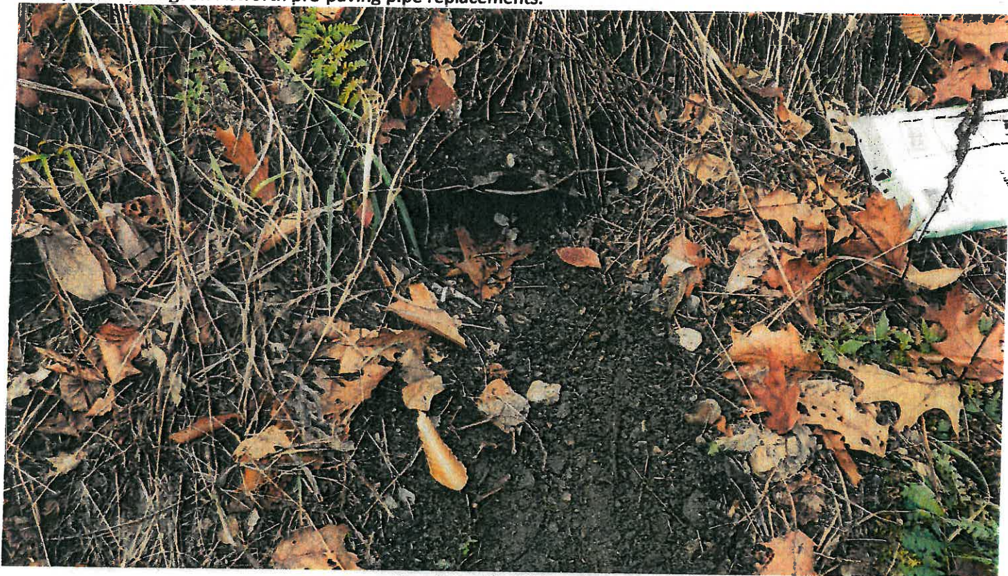
Pipe #21, 12" CMP, outlet.
