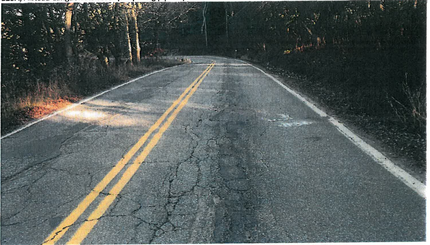
Pipe #36, 15" CMP, Looking East on 123A.
