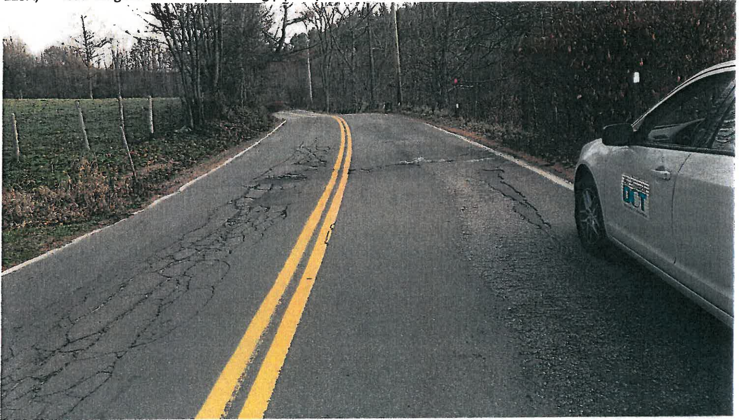
Pipe #13, 15" CMP, Looking East on 123A.
