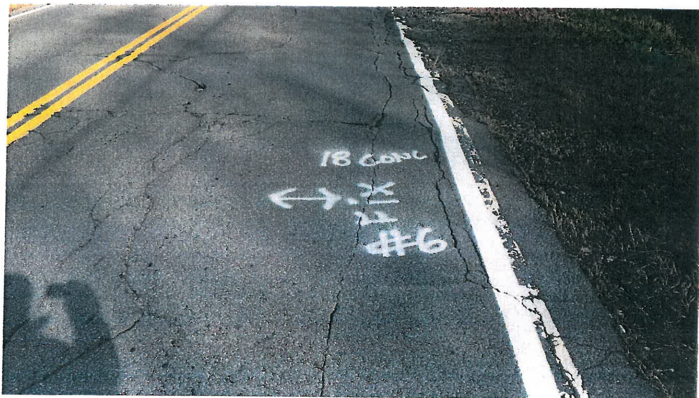
Pipe #6, 18" Concrete, Pavement Condition at Crossing.
