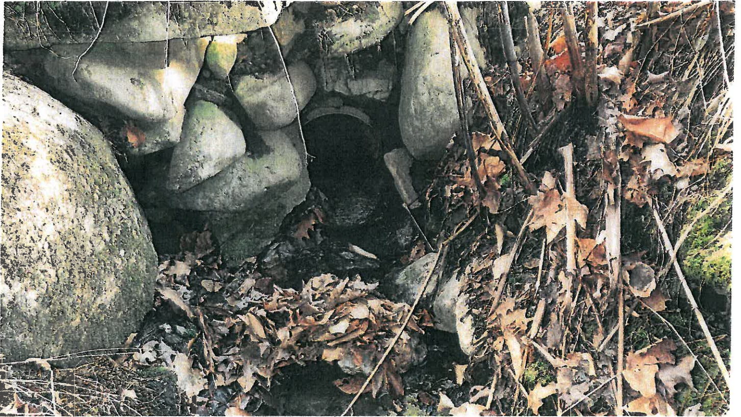
Pipe #34, 12" CMP, outlet.
