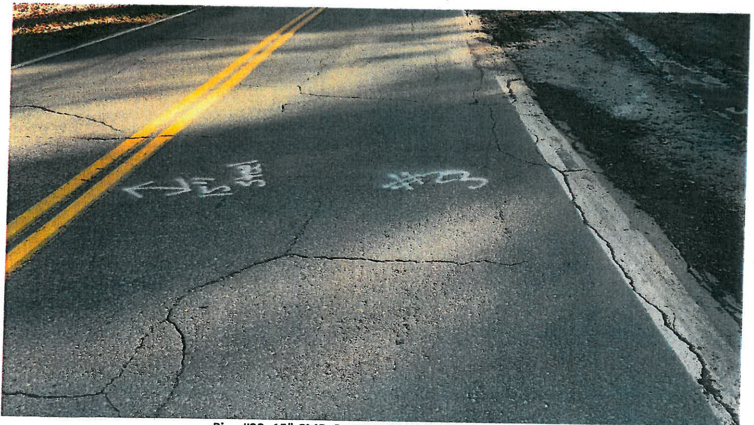
Pipe #23, 15" CMP, Pavement Condition at crossing.
