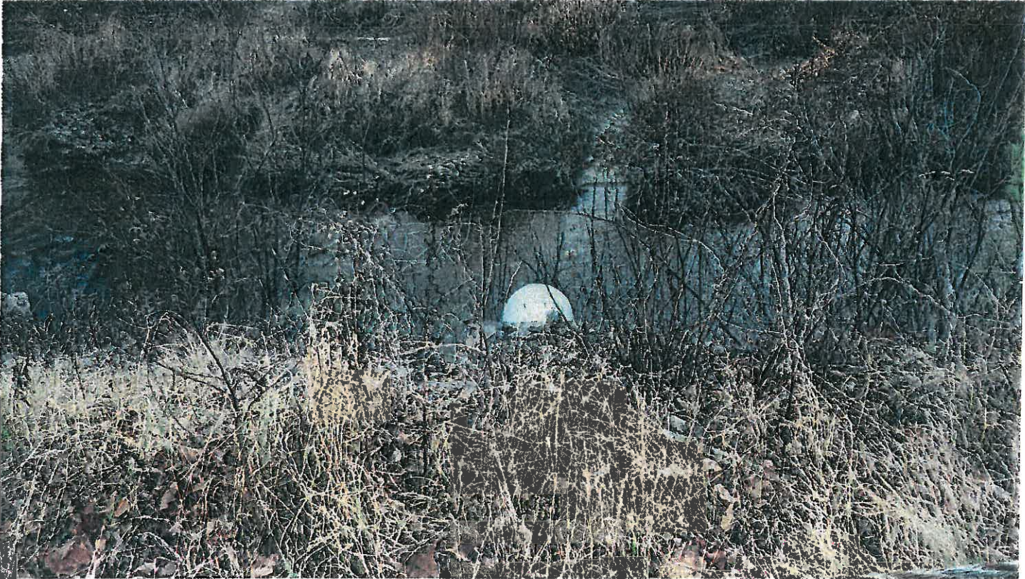
Pipe #38, 15" CMP outlet.
