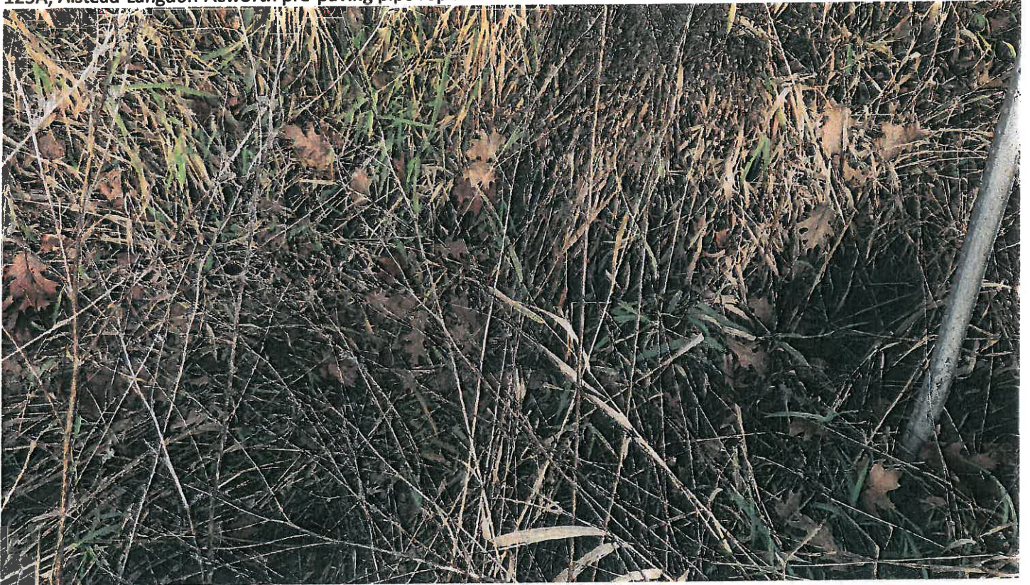
Pipe #15, 15" CMP, Inlet.
