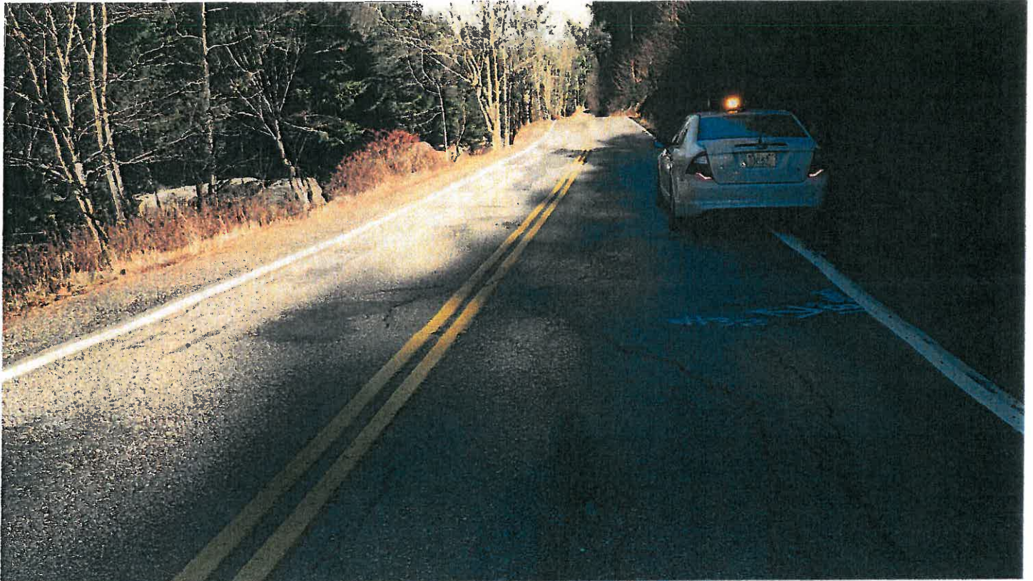
Pipe #32, 18" CMP, Looking East on 123A.
