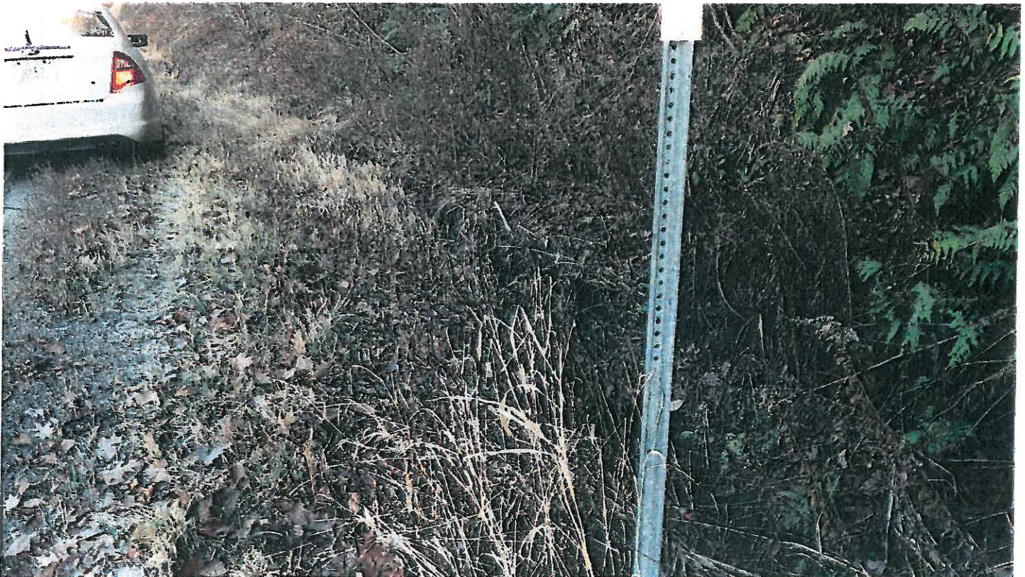
Pipe #31, 15" CMP, looking at inlet.
