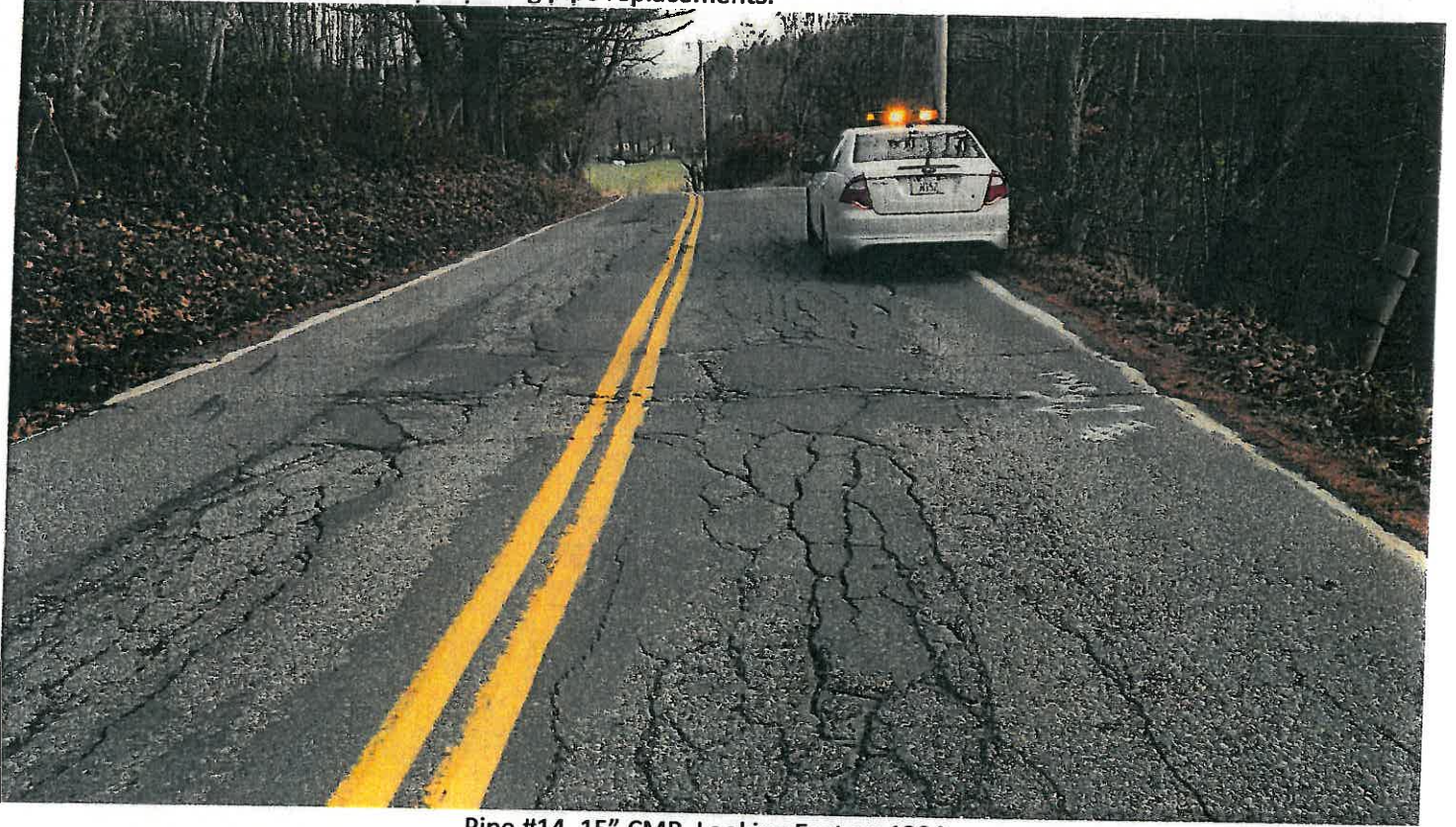
Pipe #14, 15" CMP, Looking East on 123A.
