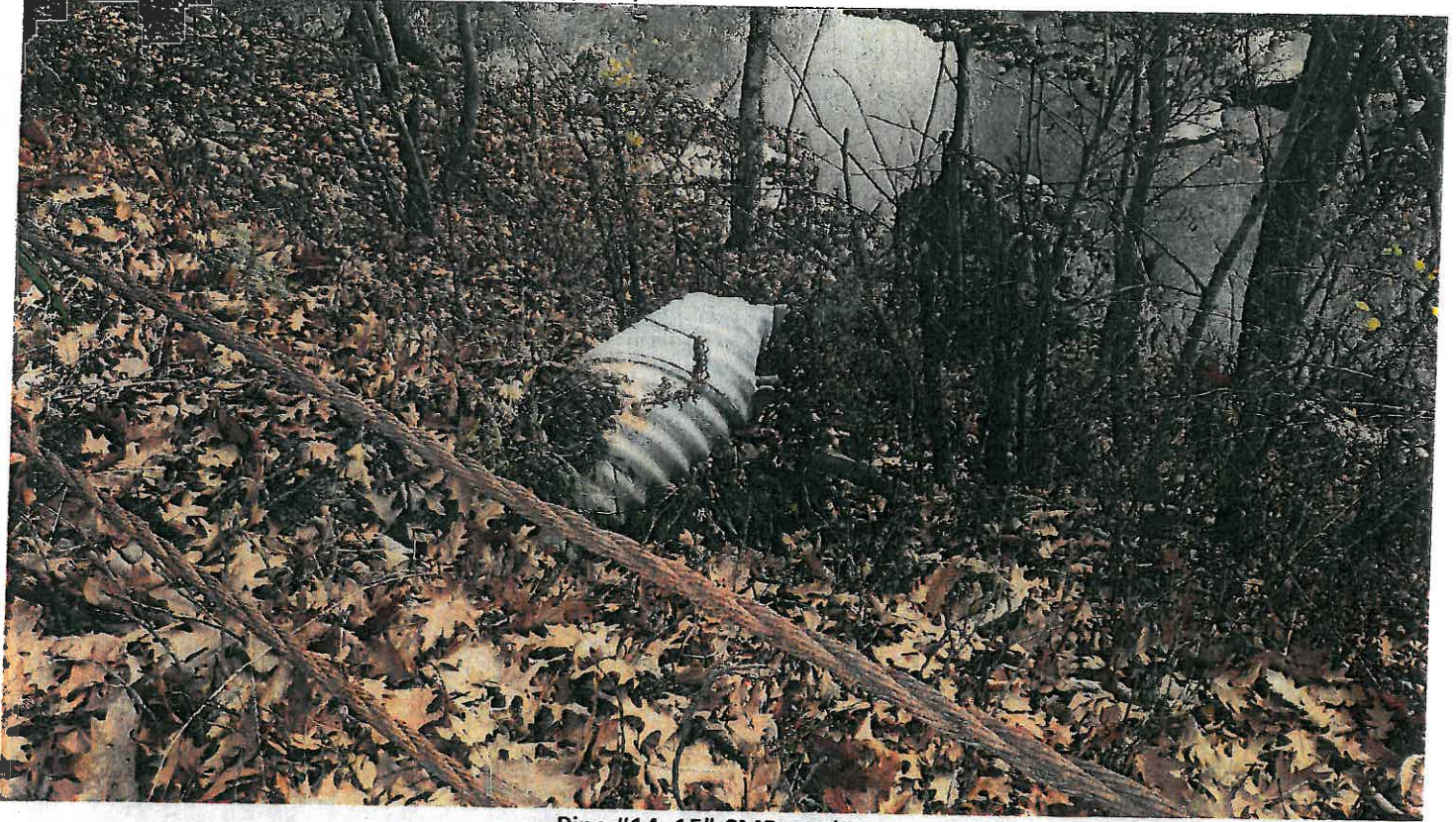
Pipe #14, 15" CMP, outlet.
