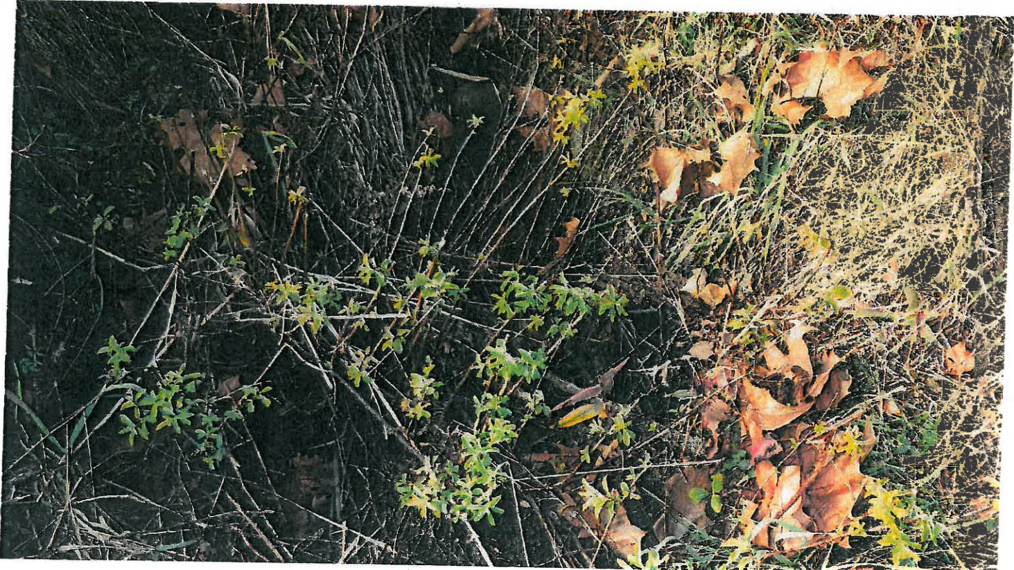
Pipe #10, 12" CMP, Inlet.
