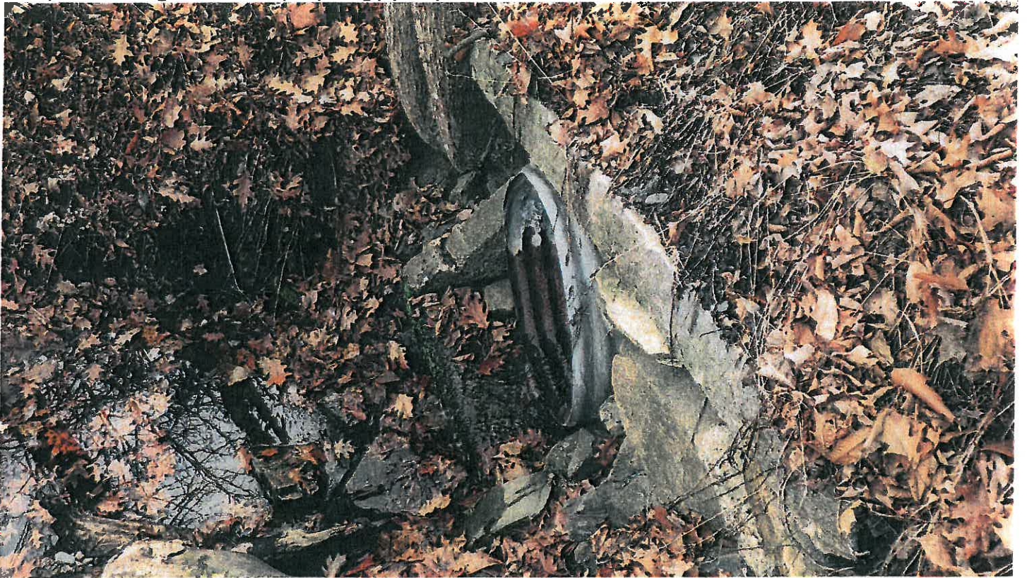
Pipe #19, 2x3 box 30" CMP, Outlet.
