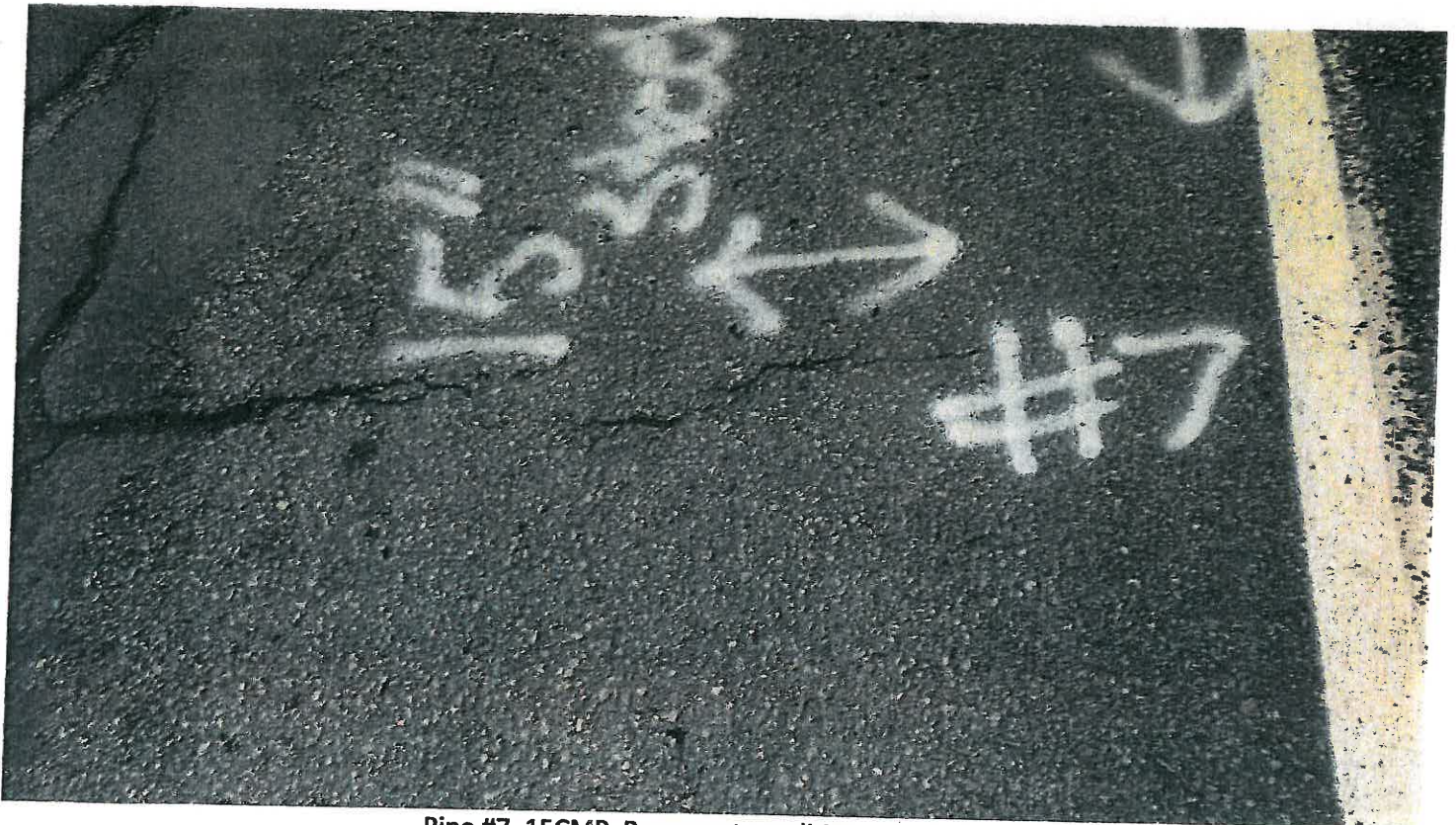
Pipe #7, 15CMP, Pavement condition at crossing.
