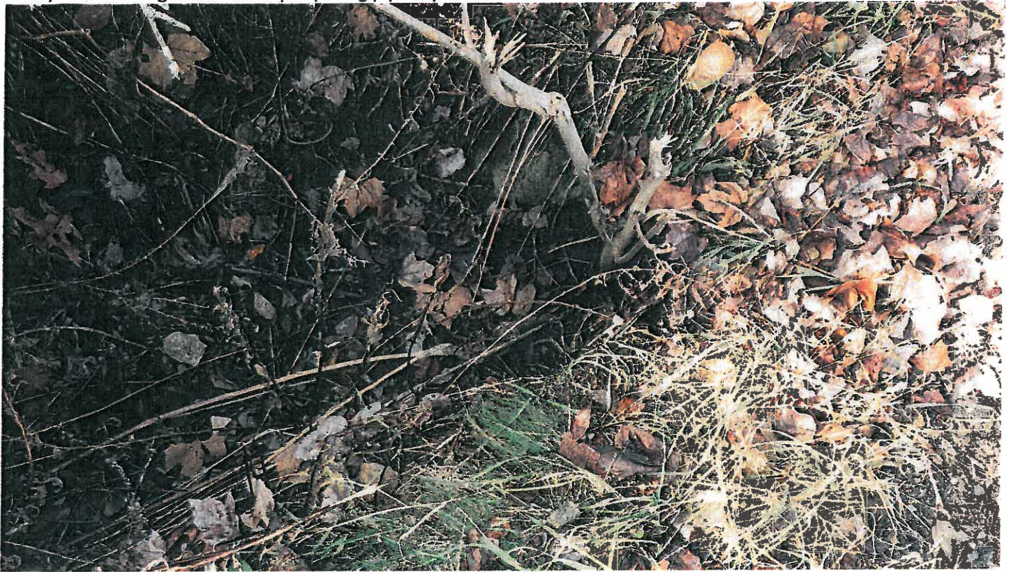
Pipe #9, 15" CMP, inlet.
