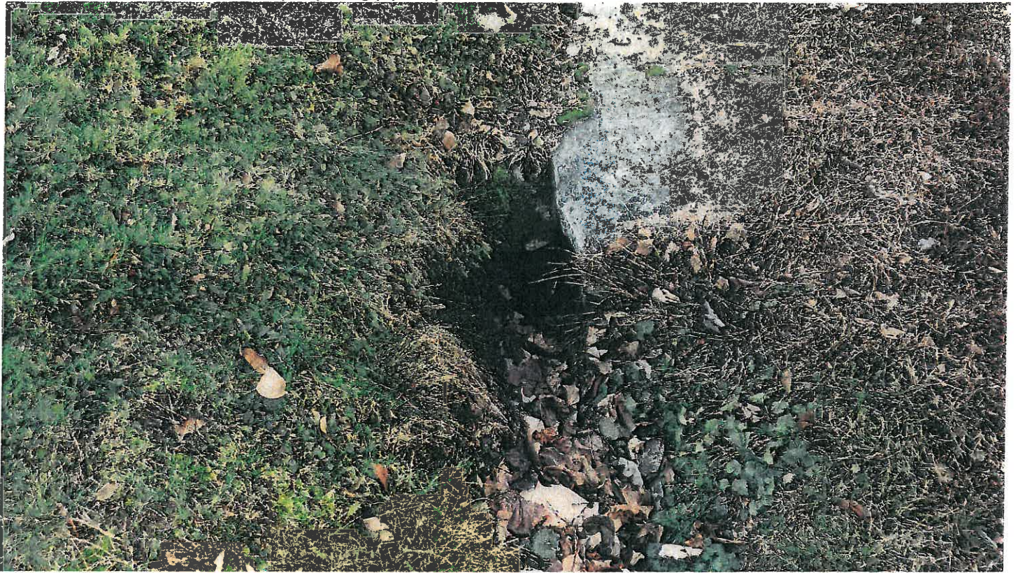
Pipe #35, 15" CMP, inlet.
