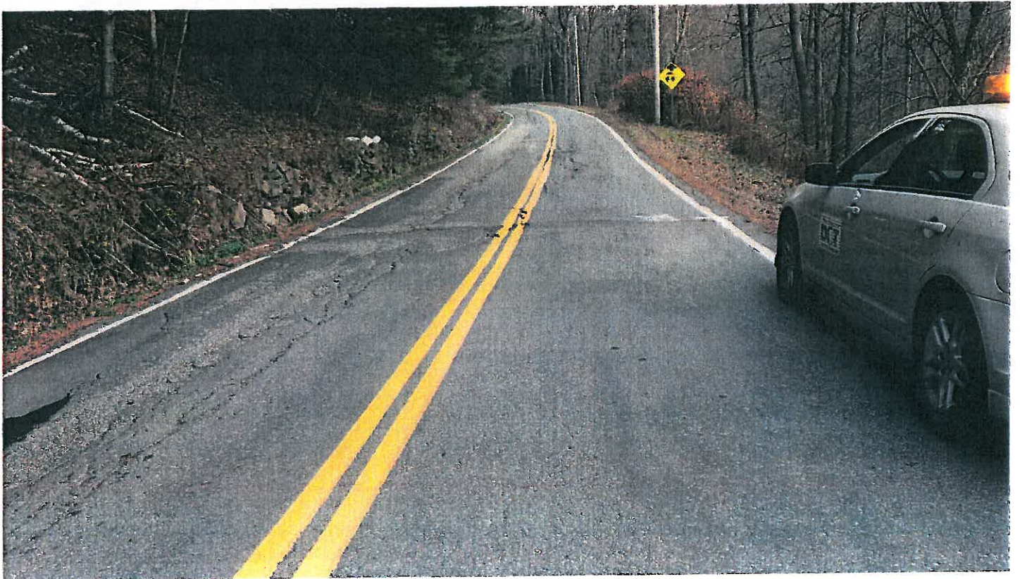
Pipe #16, 15" CMP, Looking East on 123A.
