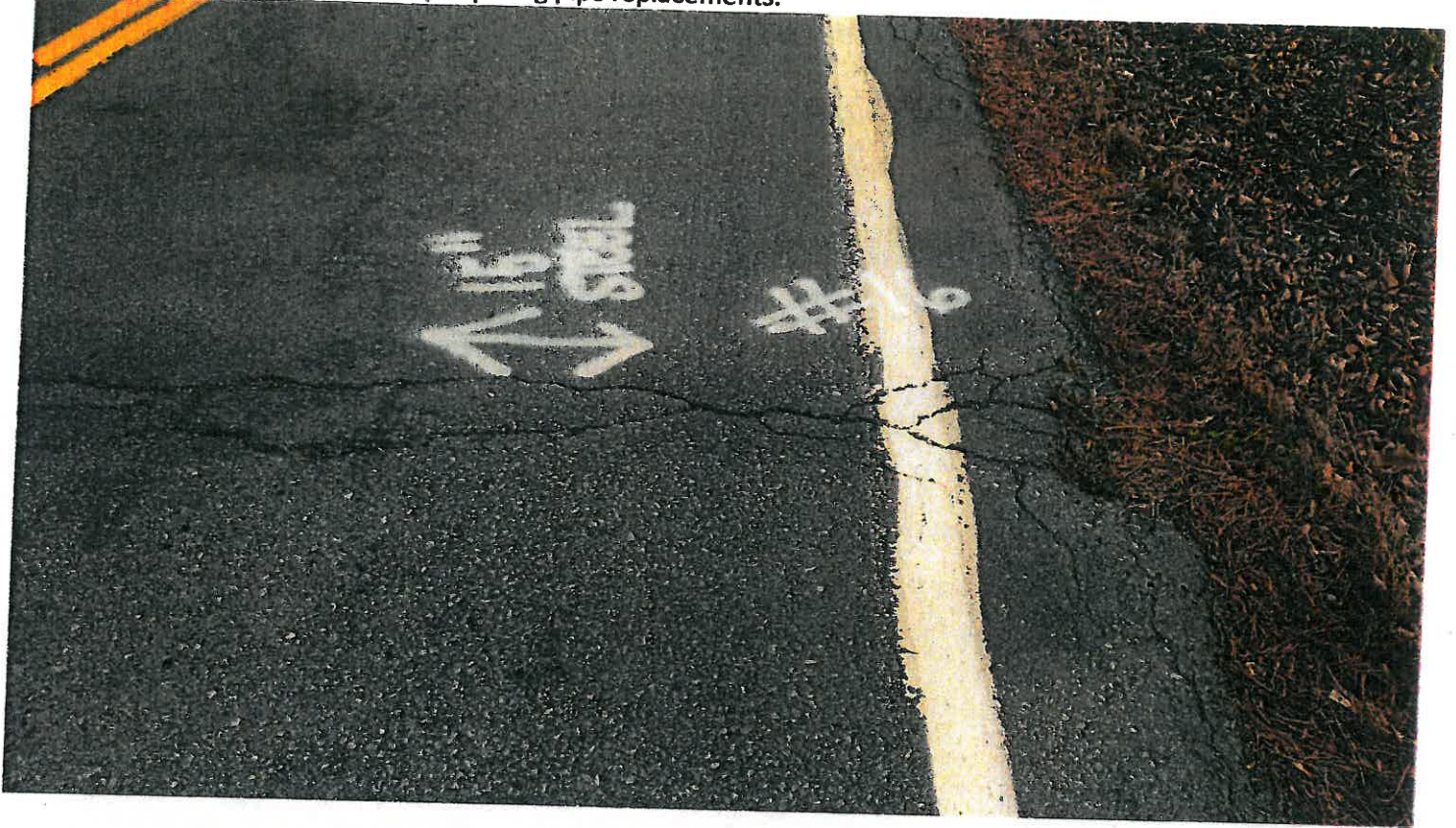
Pipe #16, 15" CMP pavement condition at crossing.
