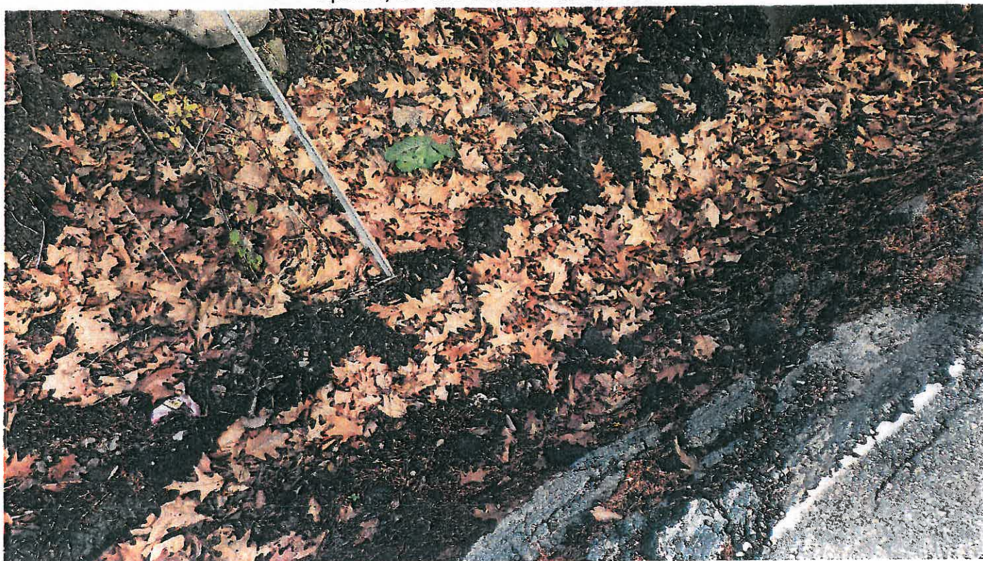
Pipe # 14, 15" CMP inlet ditch.
