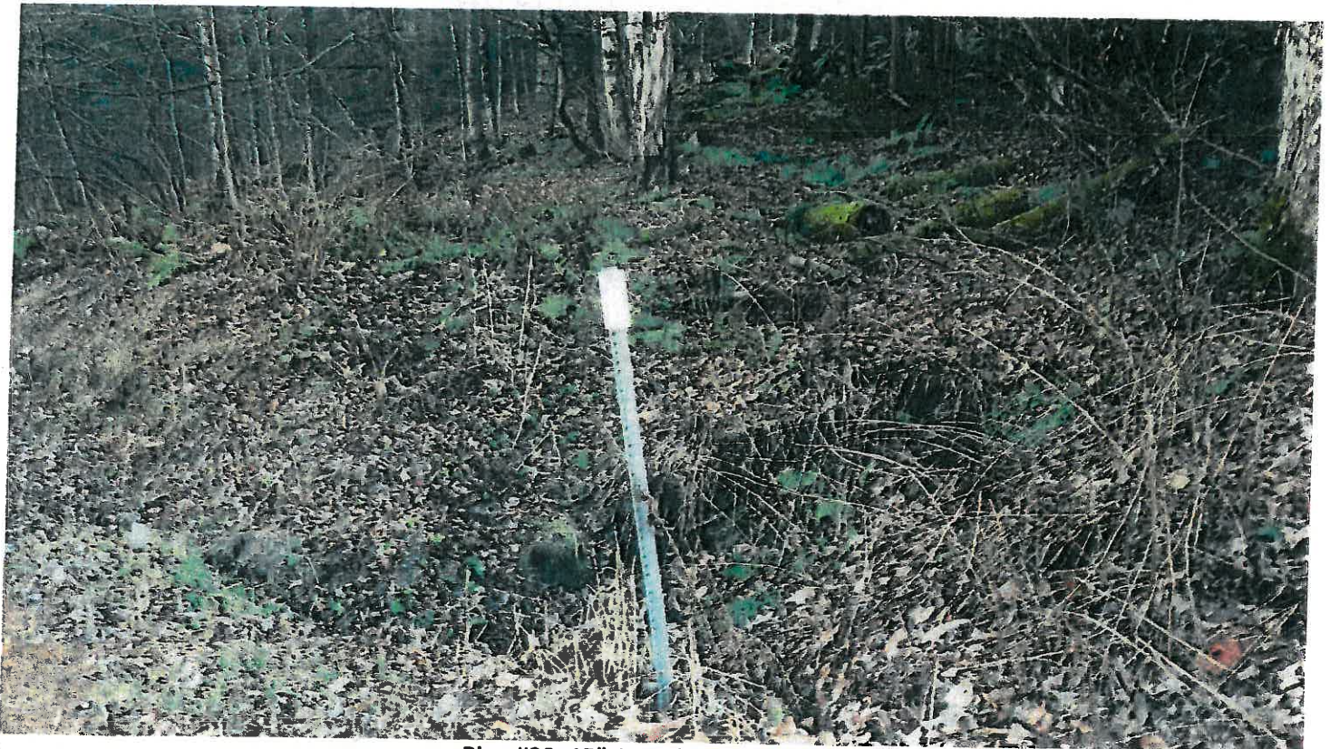
Pipe #30, 15" CMP, looking at inlet.
