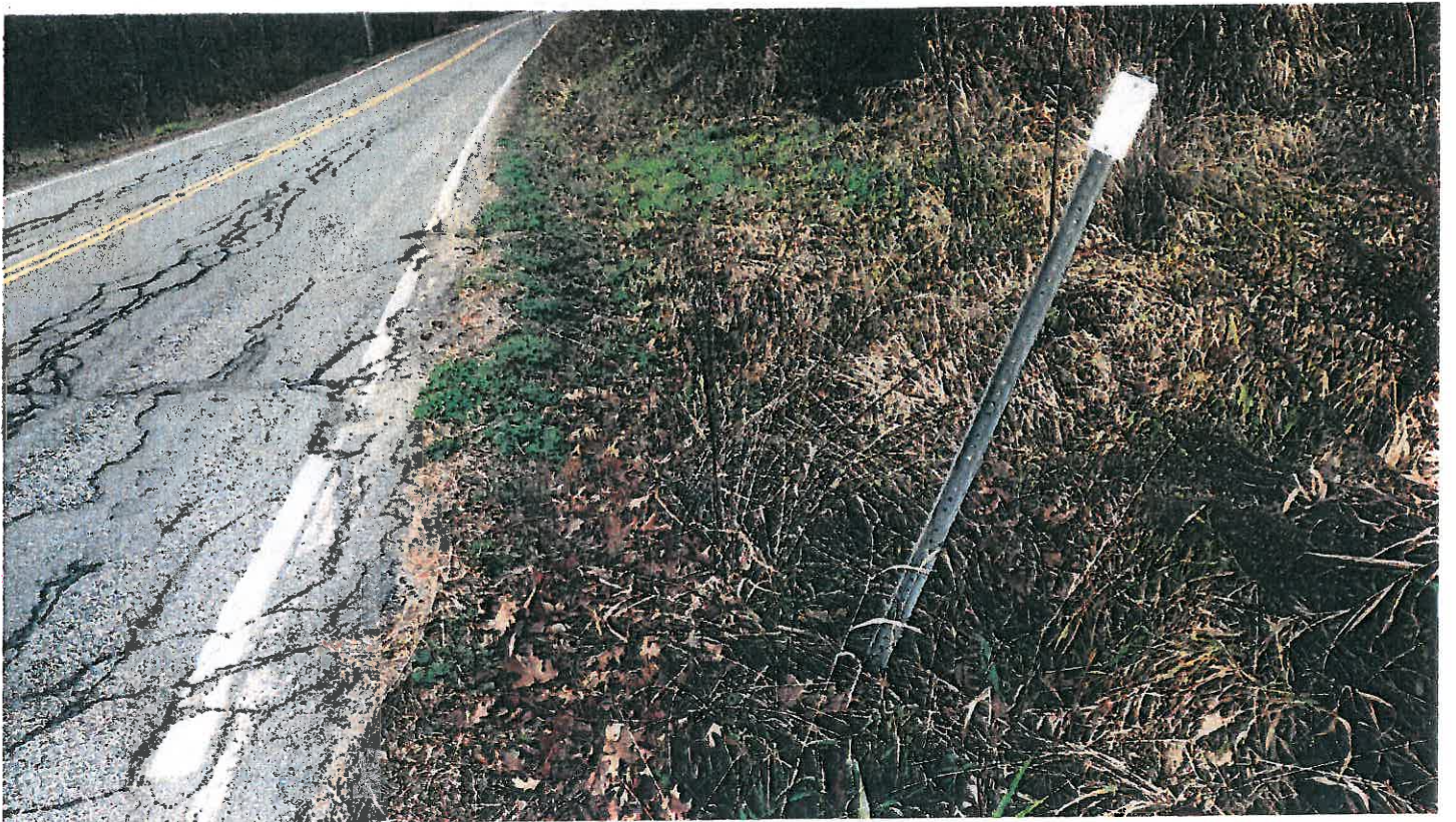
Pipe #15, 15" CMP, Inlet ditch.
