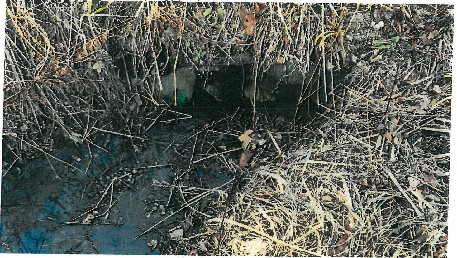
Pipe #35, 15" CMP, outlet.
