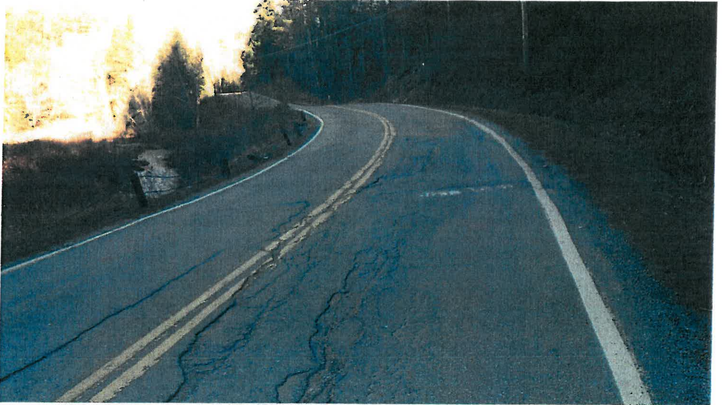
Pipe #38, 15" CMP, Looking East on 123A.
