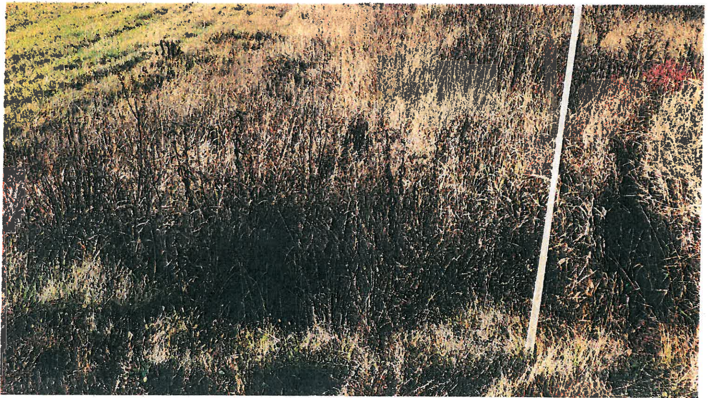
Pipe#3, 15" CMP, Looking at outlet
