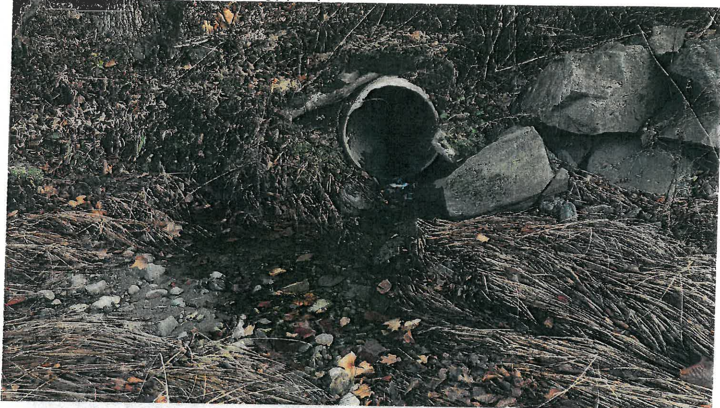
Pipe #11, 24" CMP outlet.
