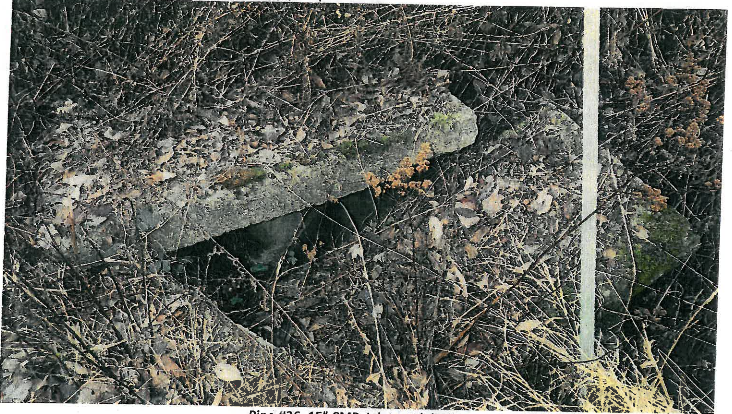
Pipe #36, 15" CMP, Inlet catch basin.
