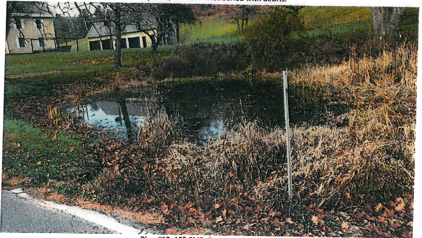
Pipe #13, 15" CMP, Farm pond at inlet.
