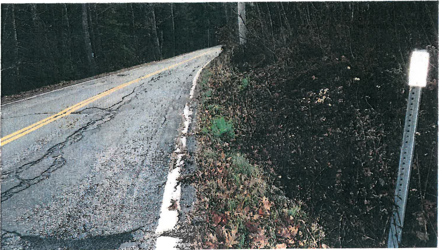
Pipe #18, 15" CMP inlet ditch.
