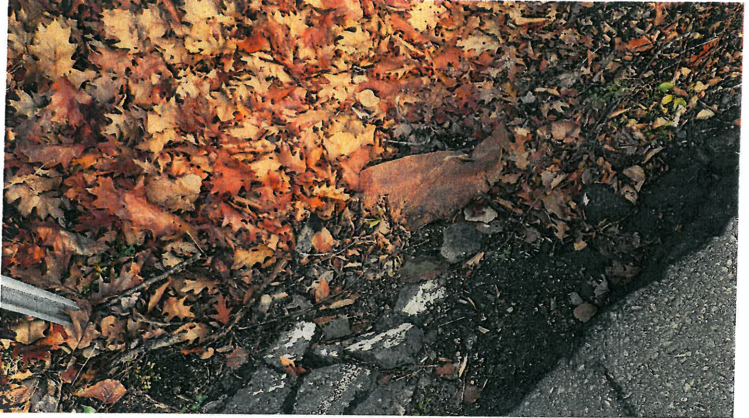
Pipe #17, 15" CMP Inlet.
