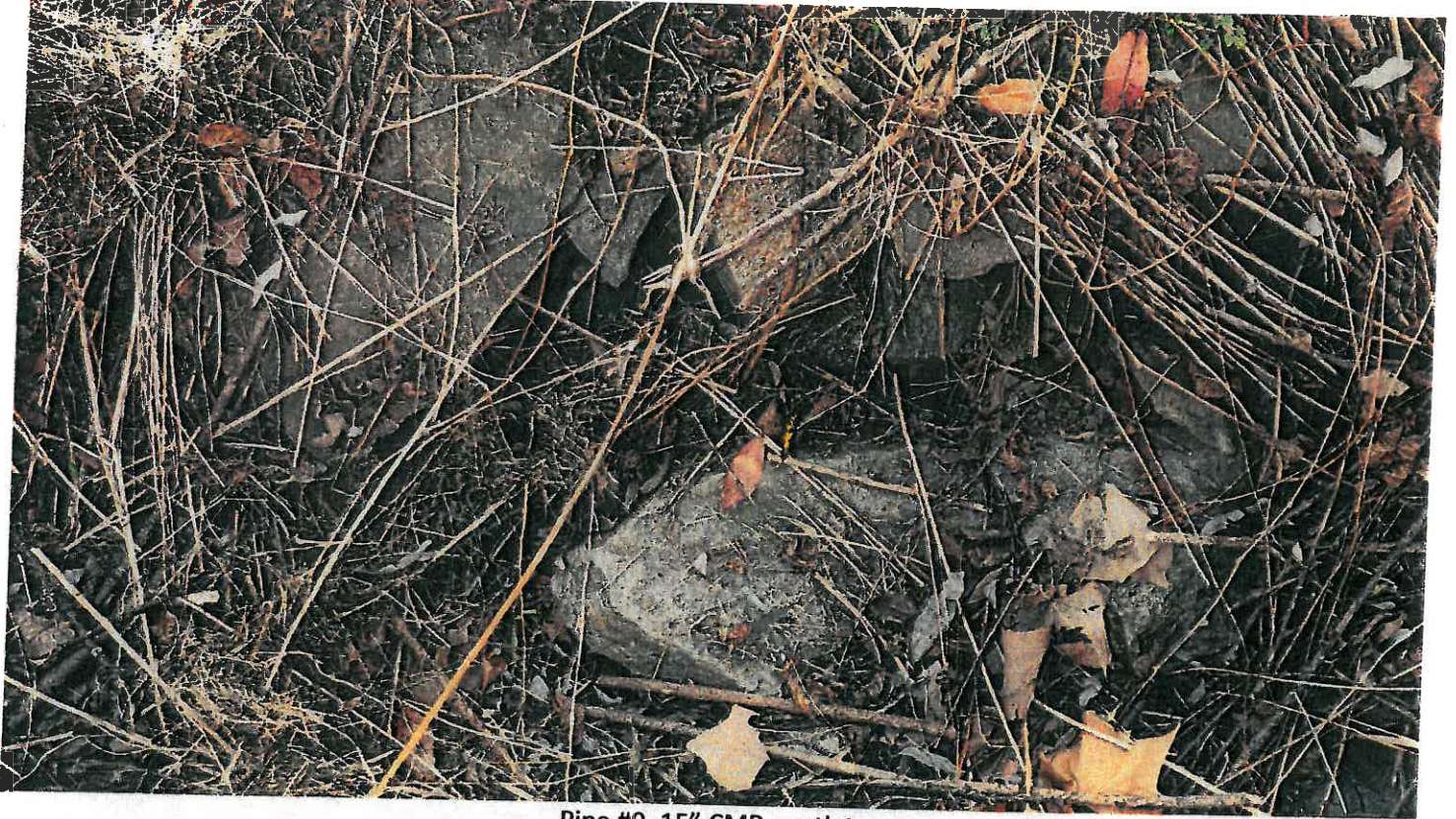
Pipe #9, 15" CMP, outlet.
