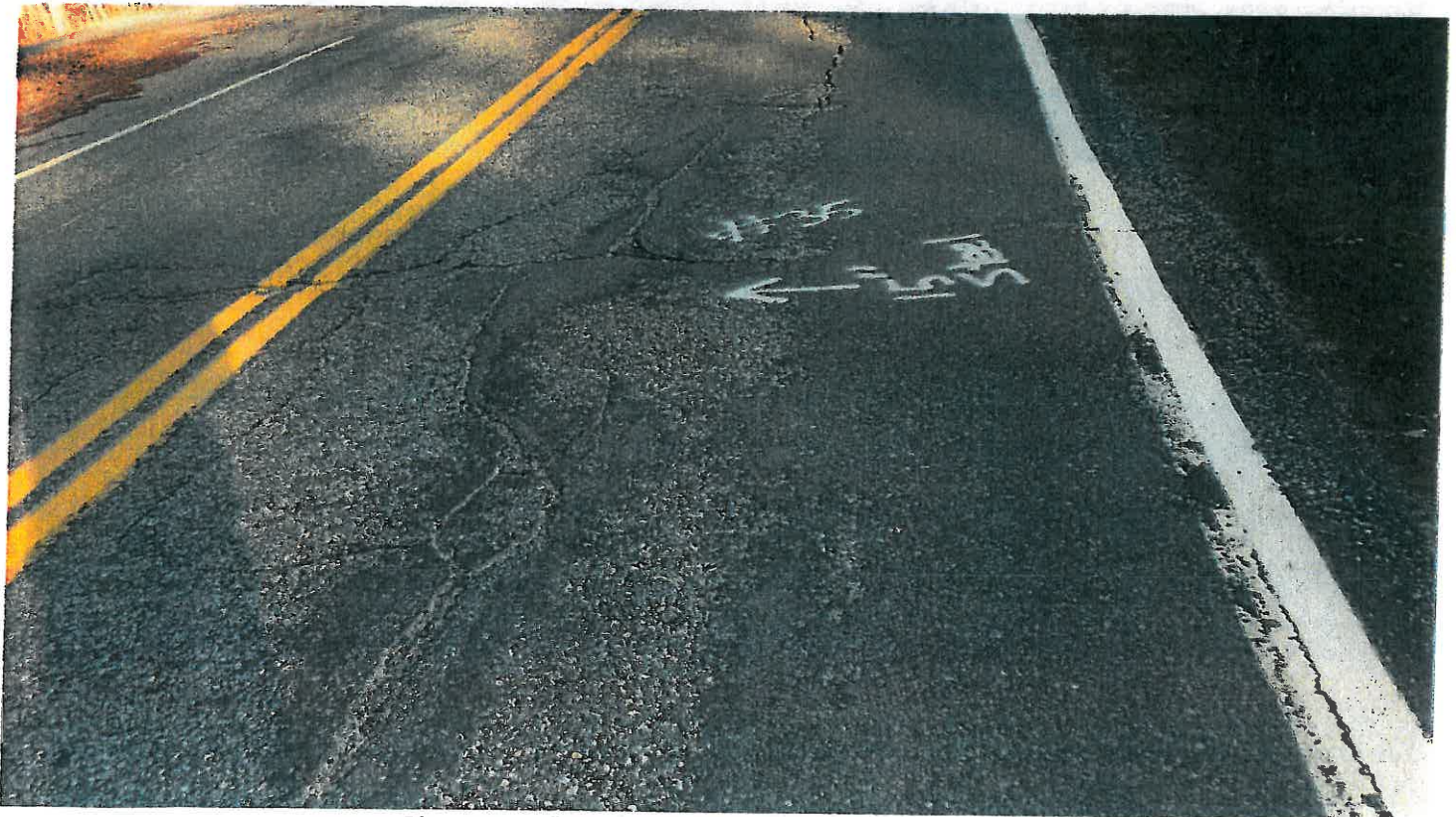
Pipe #35, 15" CMP, pavement conditions at crossing.
