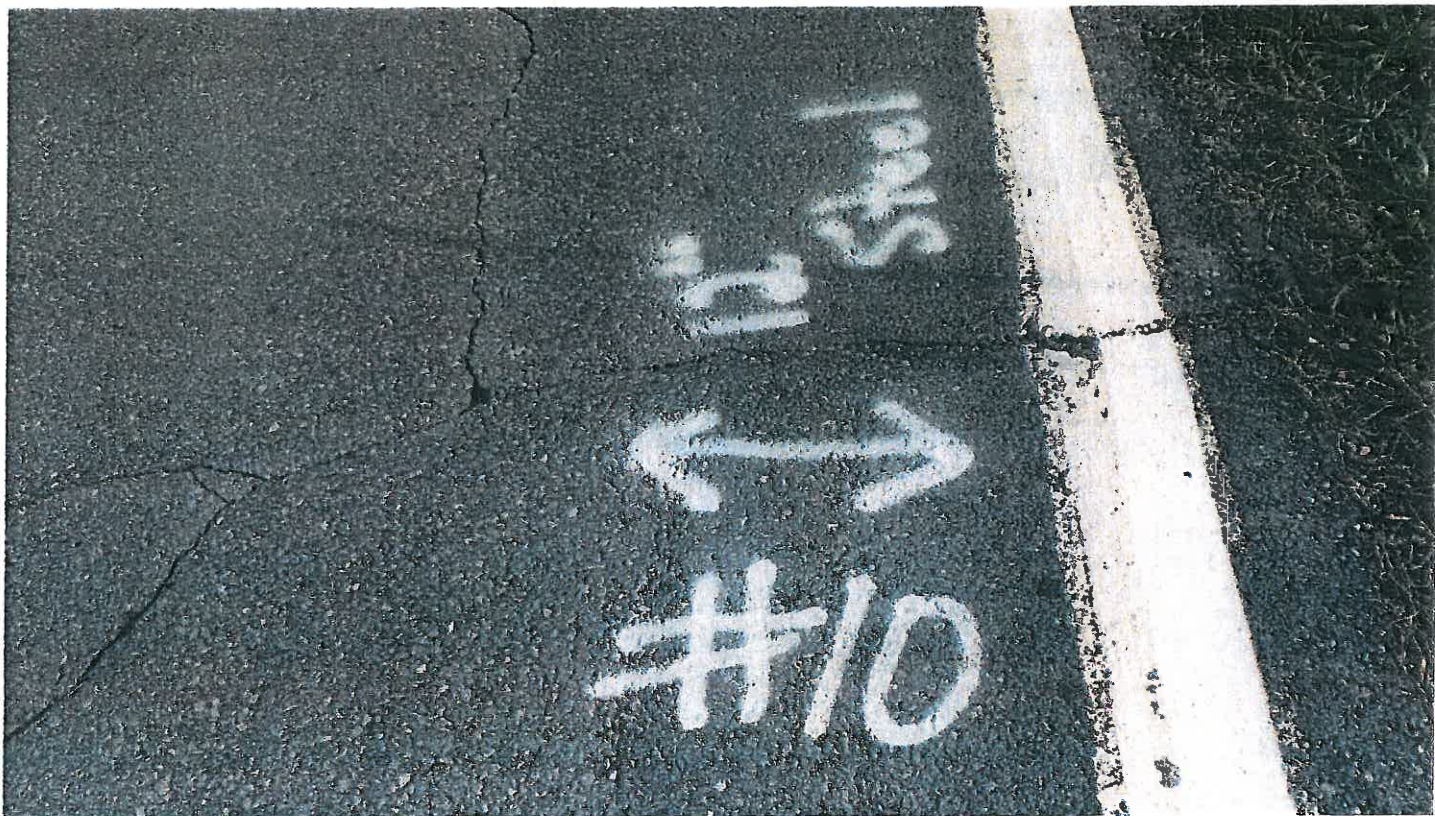
Pipe #10, 12" CMP pavement condition at crossing.
