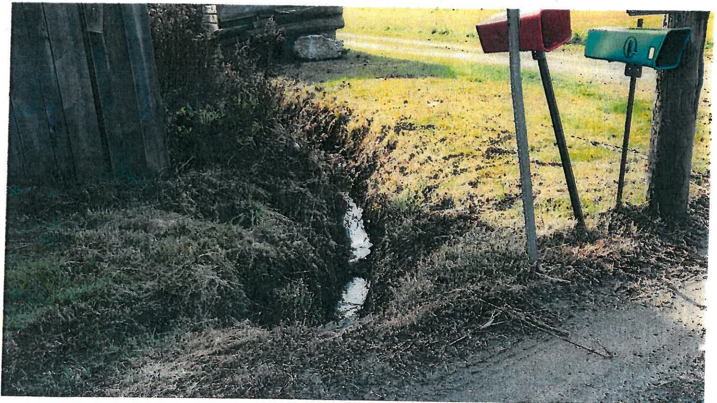
Pipe #8, 15" CMP inlet.
