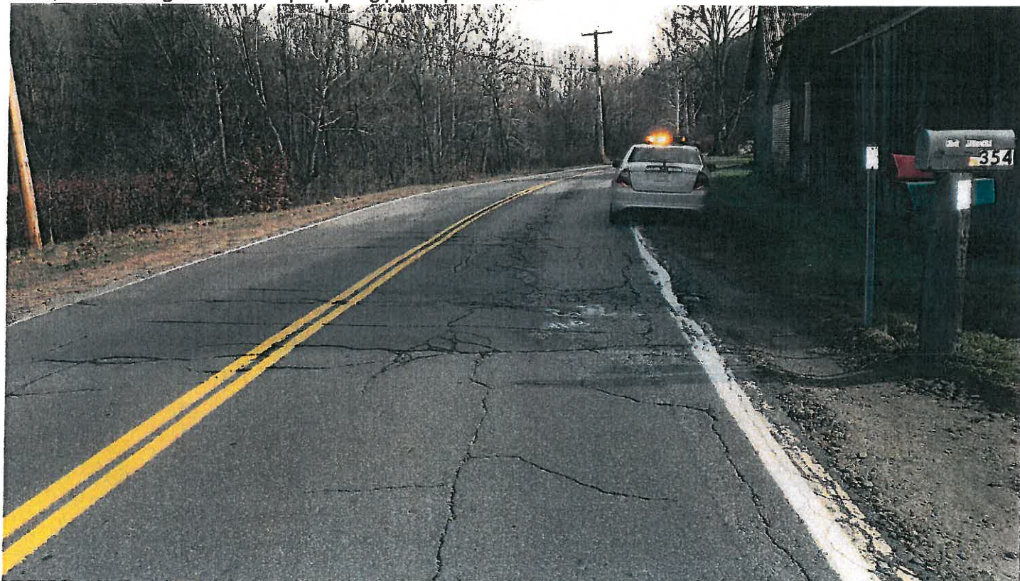
123A, Alstead-Langdon-Acworth pre-paving pipe replacements.
