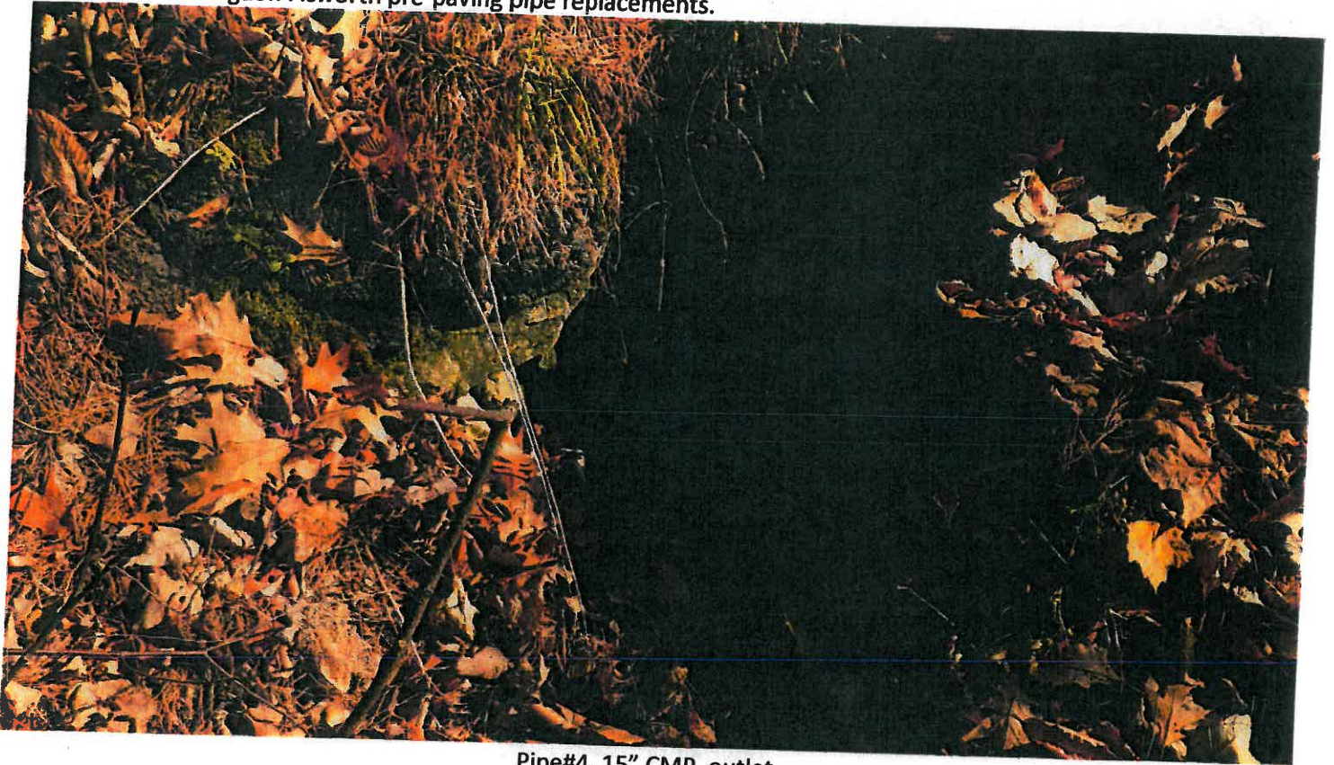
Pipe#4, 15" CMP, outlet.
