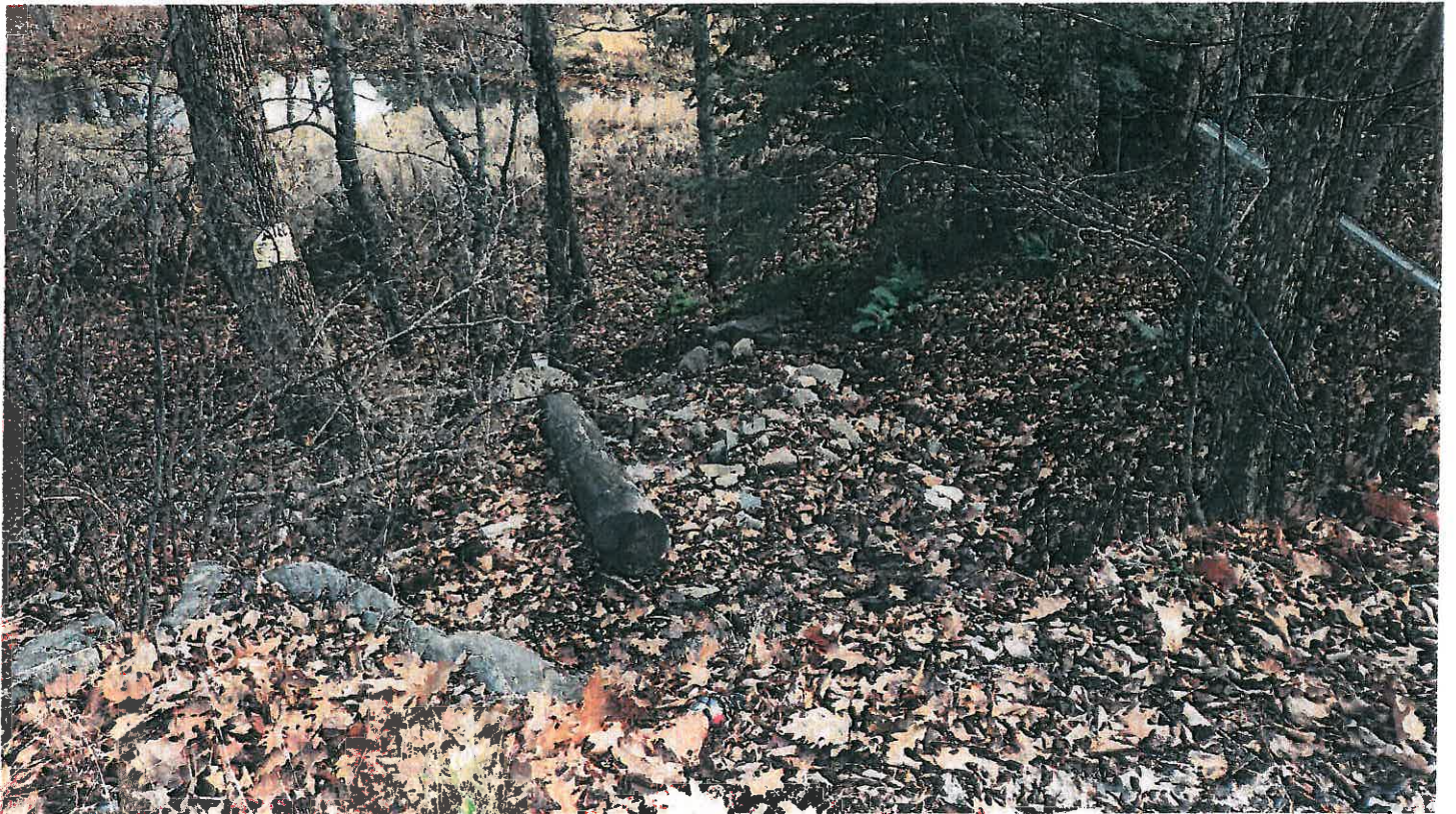
Pipe #19, 2x3 Box 30" CMP, Looking at outlet.
