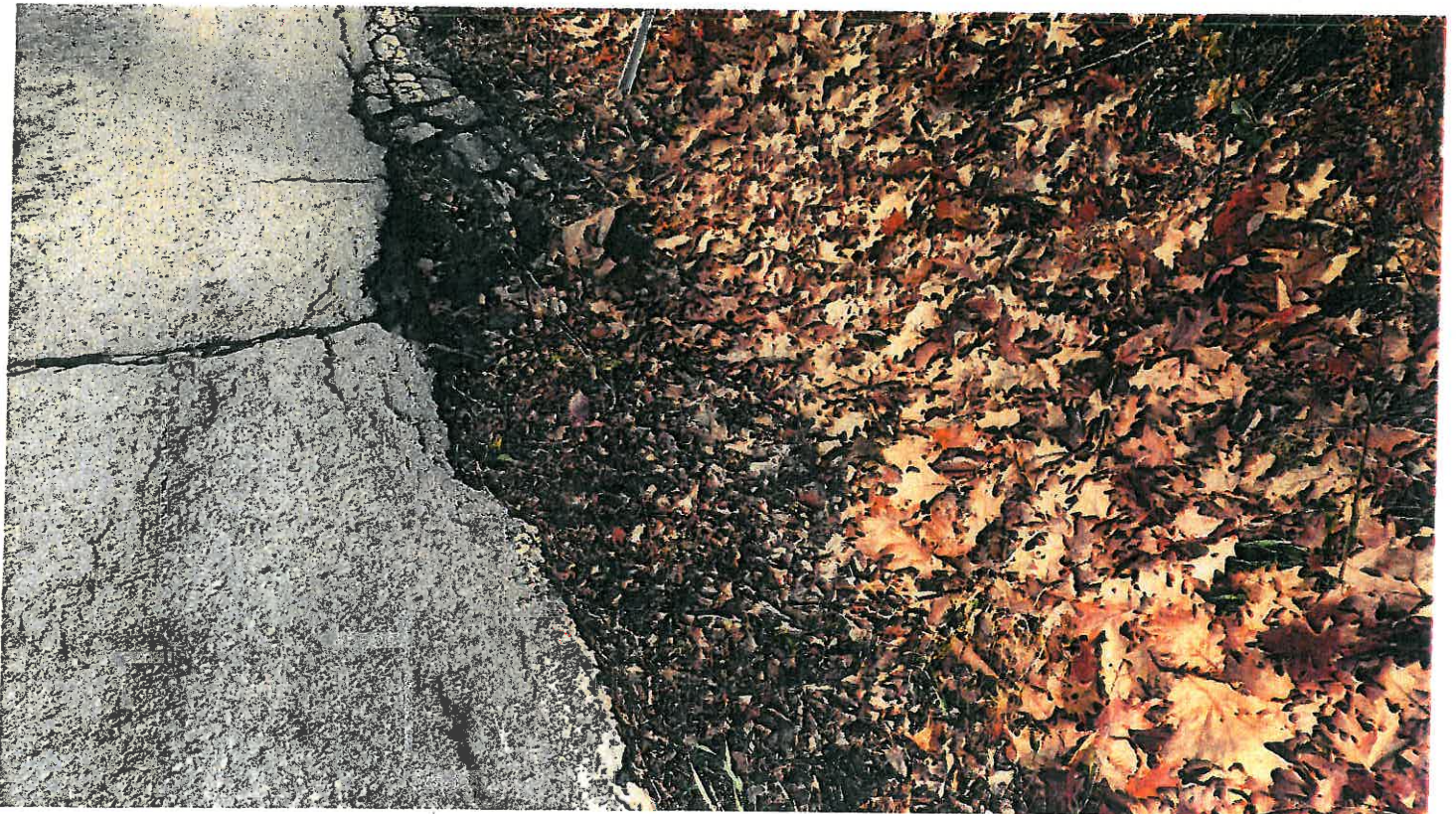
Pipe #17, 15" CMP inlet ditch.
