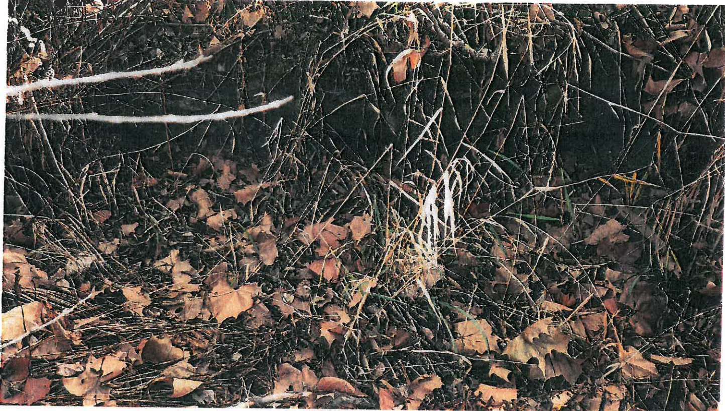
Pipe #10, 12" CMP, Outlet
