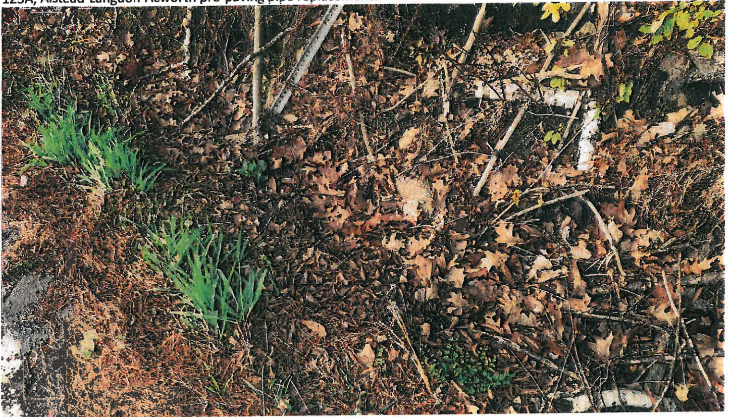
Pipe #16, Inlet ditch.
