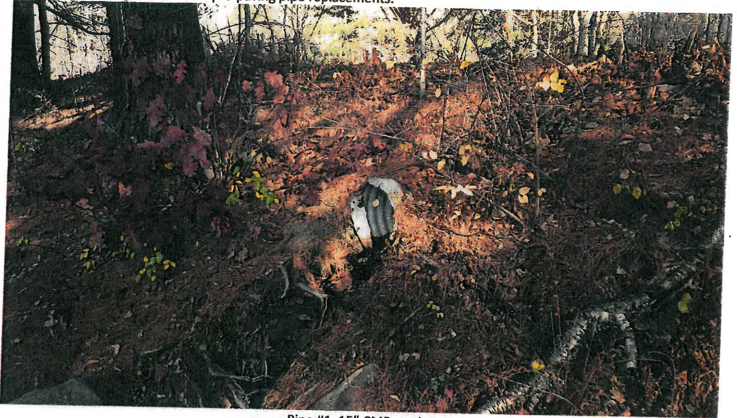
Pipe #1, 15" CMP, outlet
