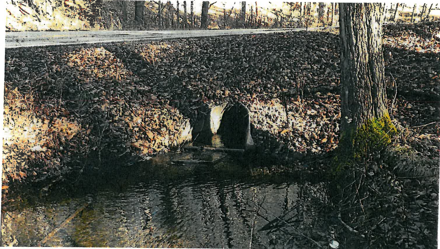
Pipe #27, 18" CMP, outlet.
