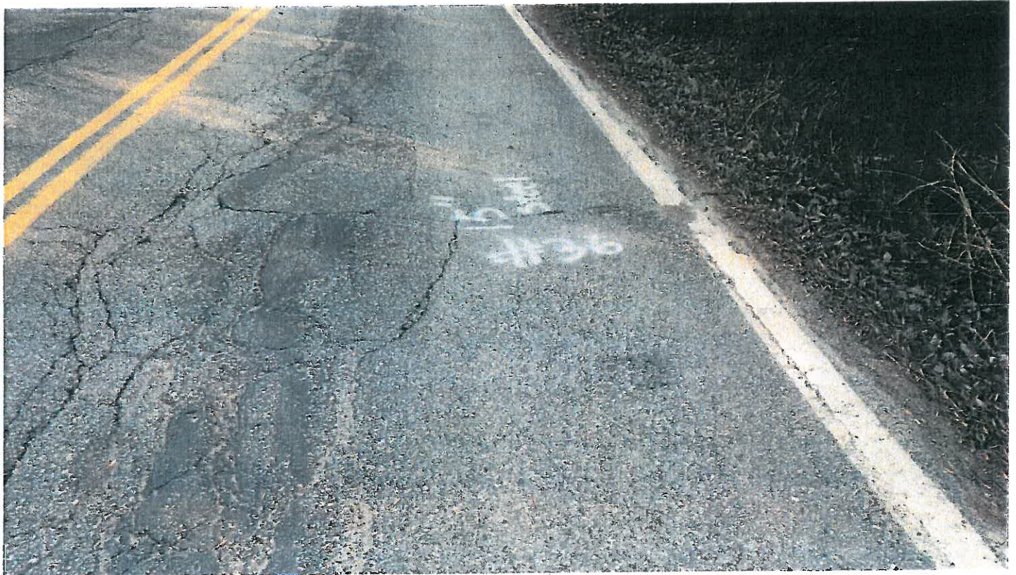
Pipe #36, 15" CMP, pavement conditions at crossing.
