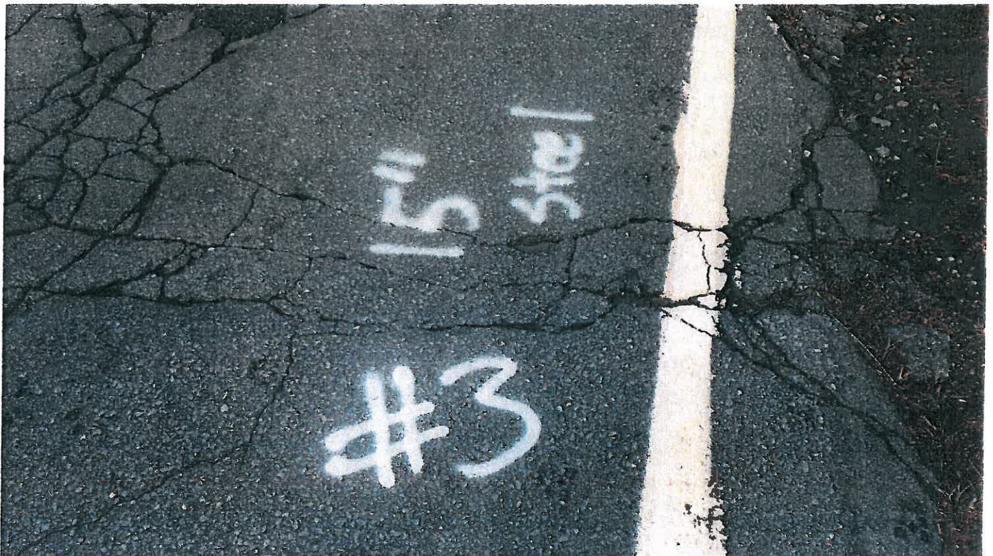
Pipe#3, 15" CMP, Pavement Condition at pipe.
