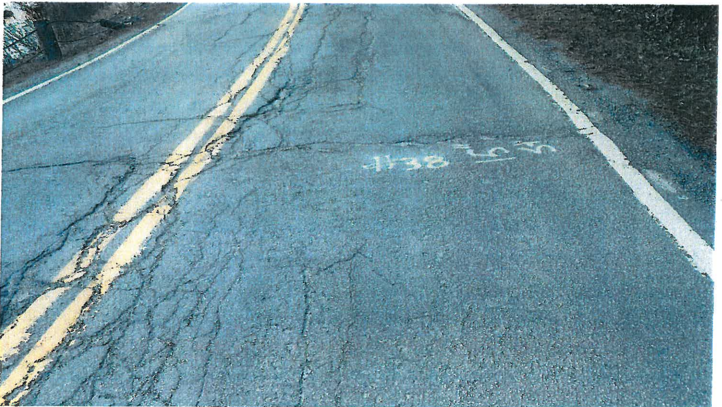
Pipe #38, 15" CMP, Pavement condition at crossing.
