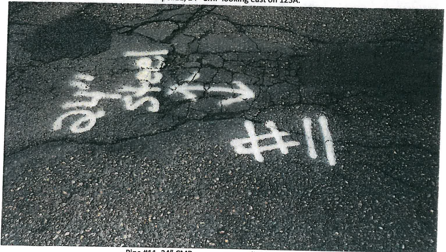
Pipe #11, 24" CMP, pavement condition at crossing.
