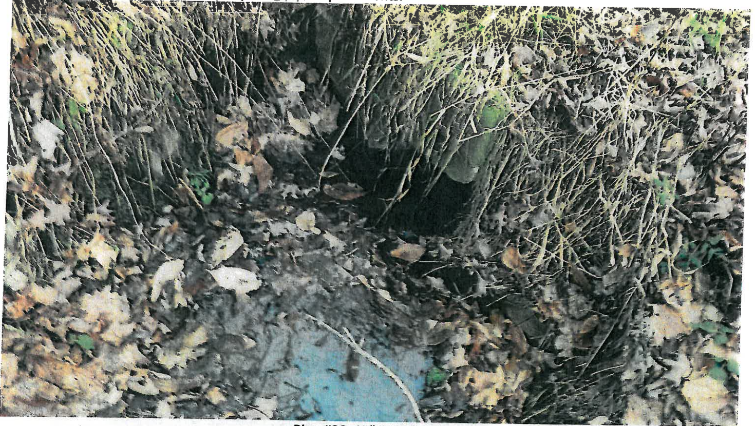
Pipe #30, 15" CMP, Inlet.
