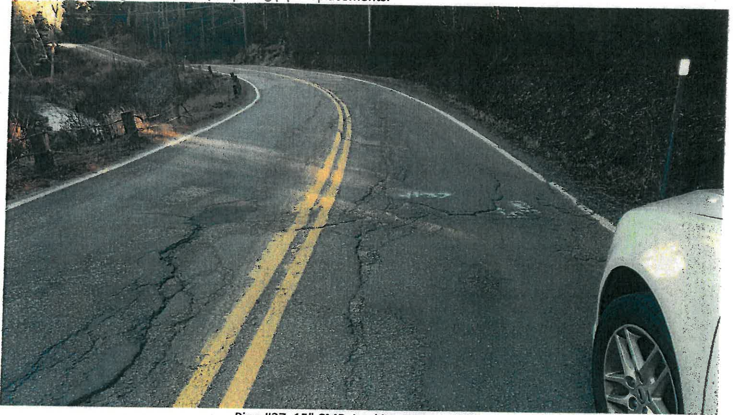
Pipe #37, 15" CMP, Looking East on 123A.
