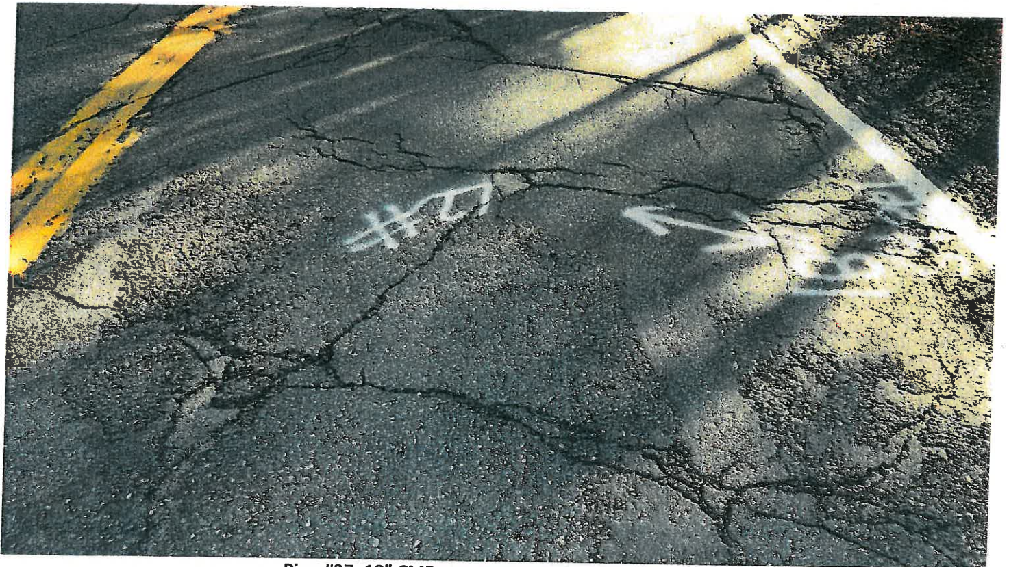
Pipe #27, 18" CMP, pavement condition at crossing.
