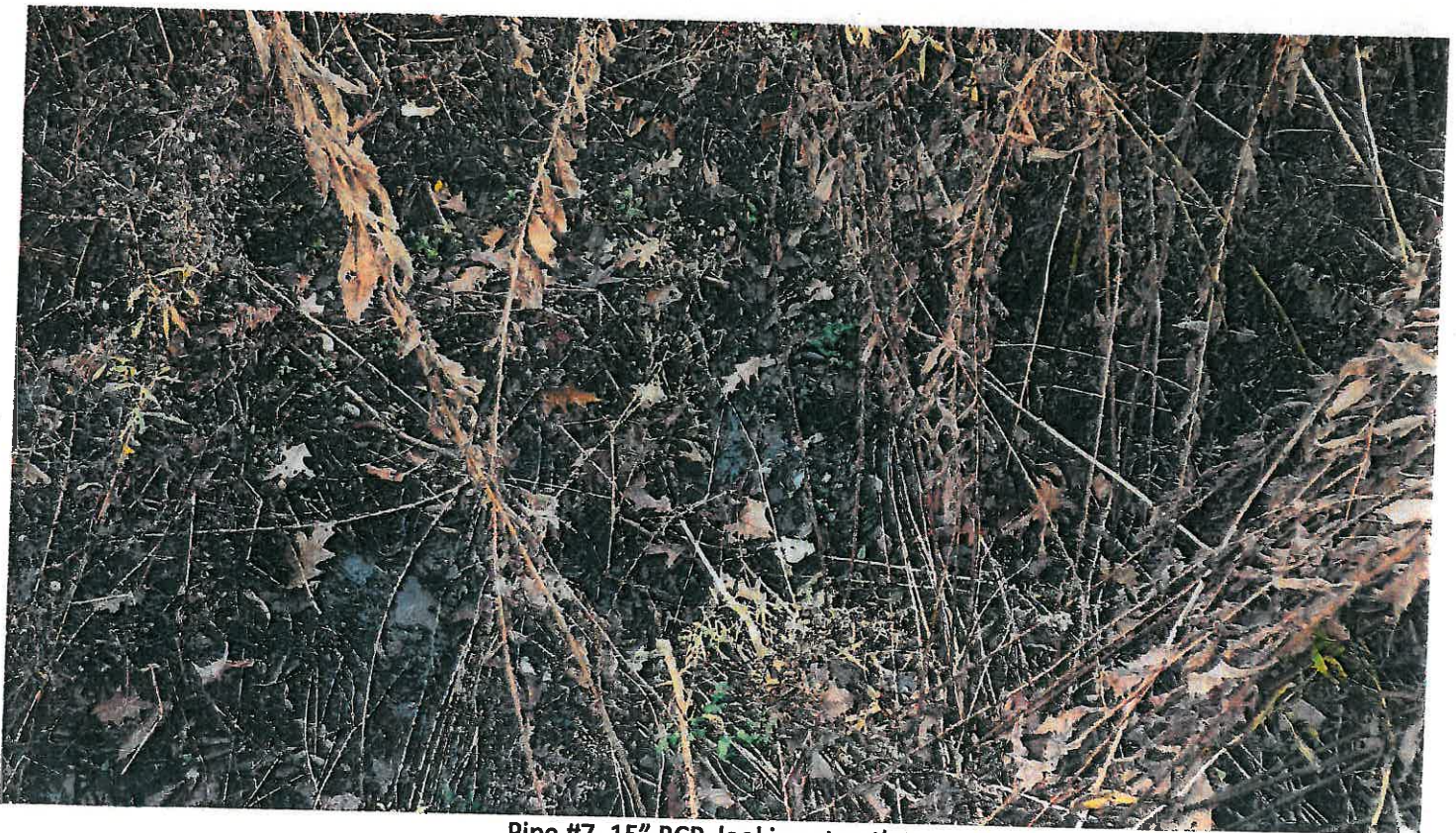
Pipe #7, 15" RCP, looking at outlet.
