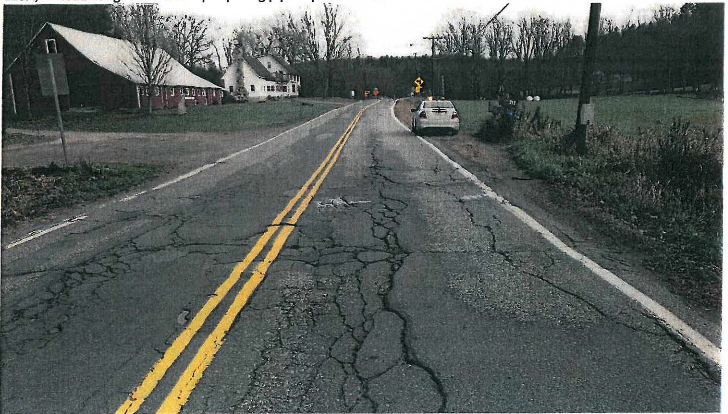
Pipe #15, 15" CMP, Looking East on 123A.
