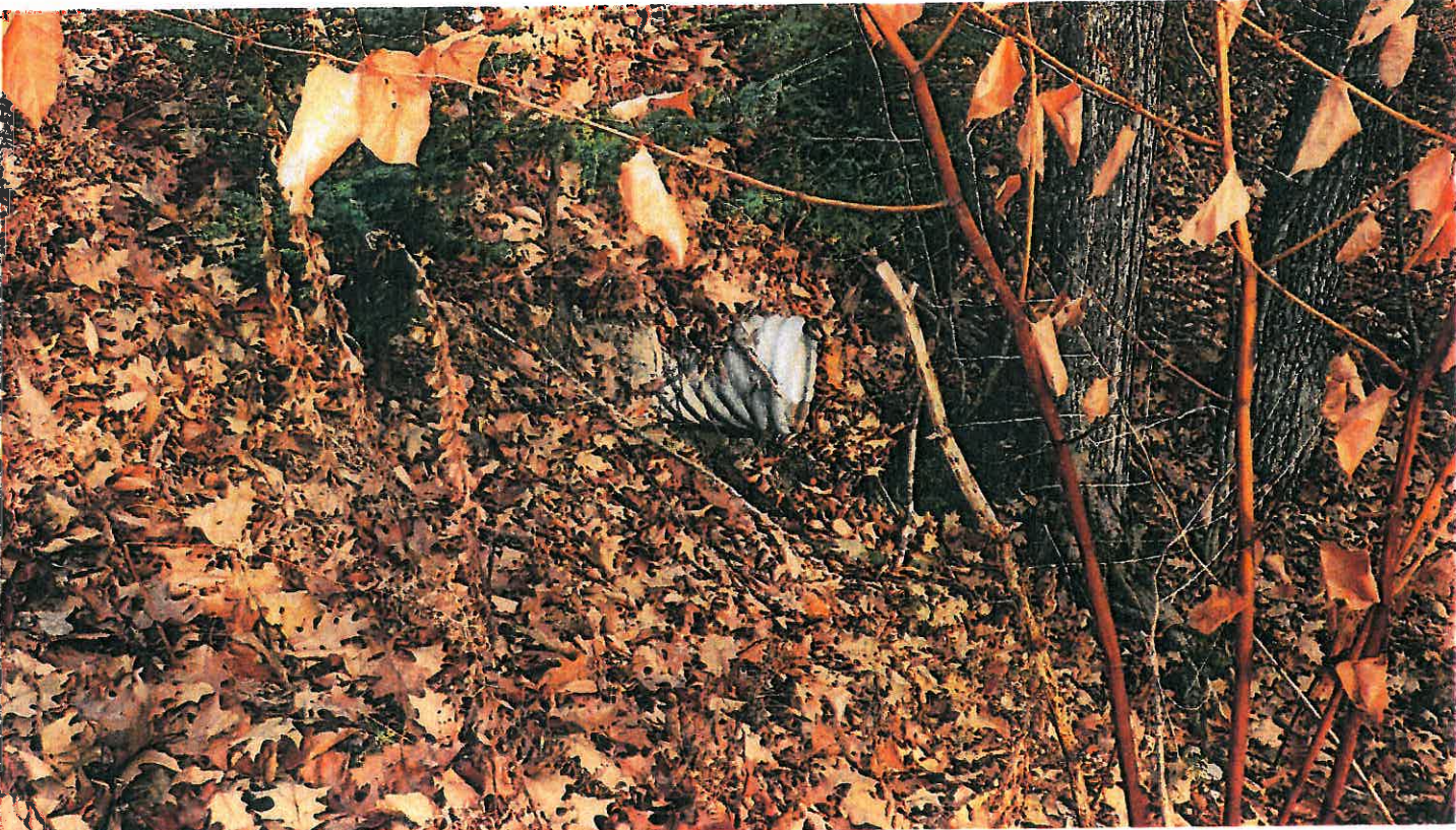
Pipe #17, 15" CMP, outlet.
