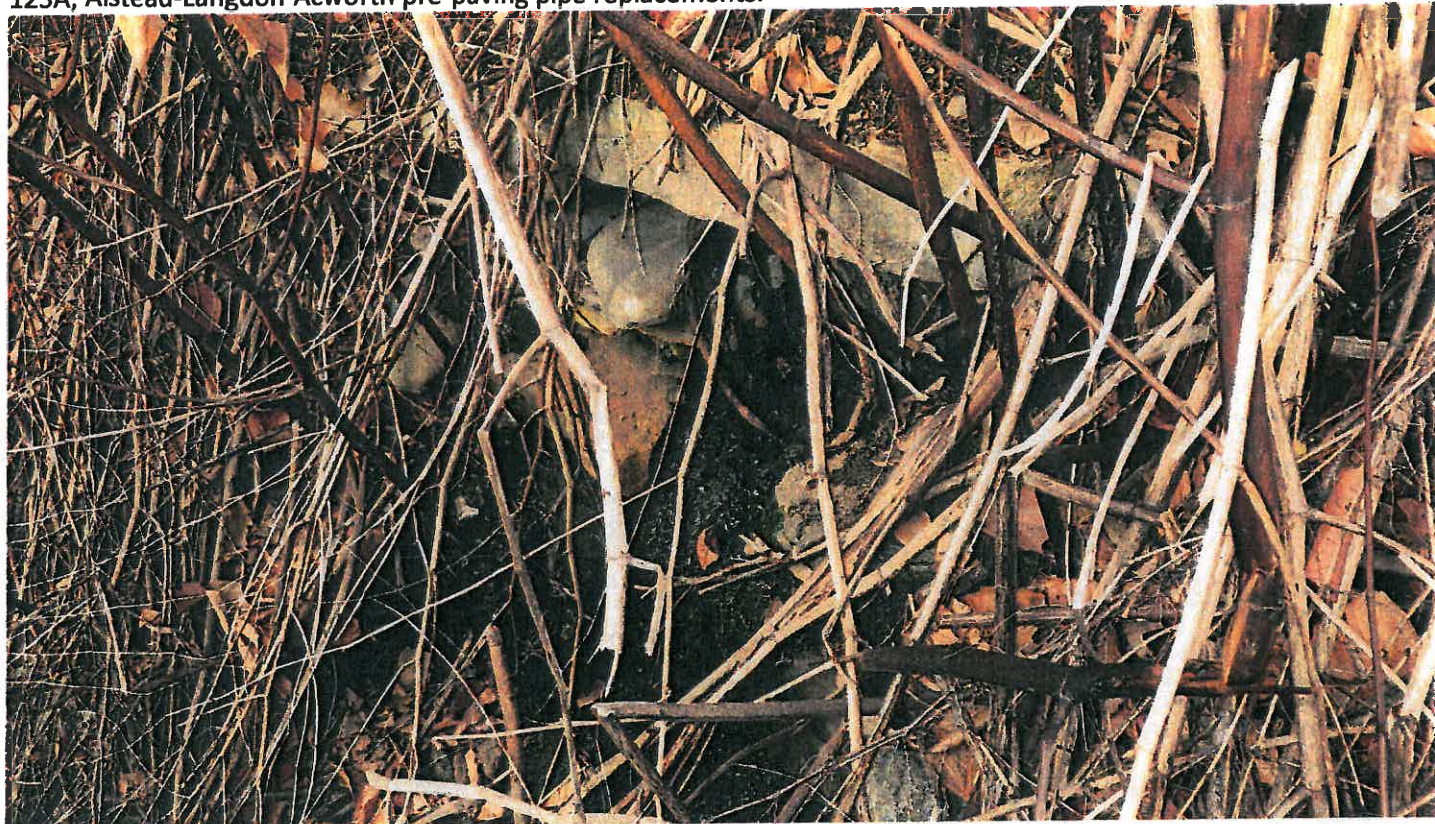
Pipe #13, 15" CMP, outlet
