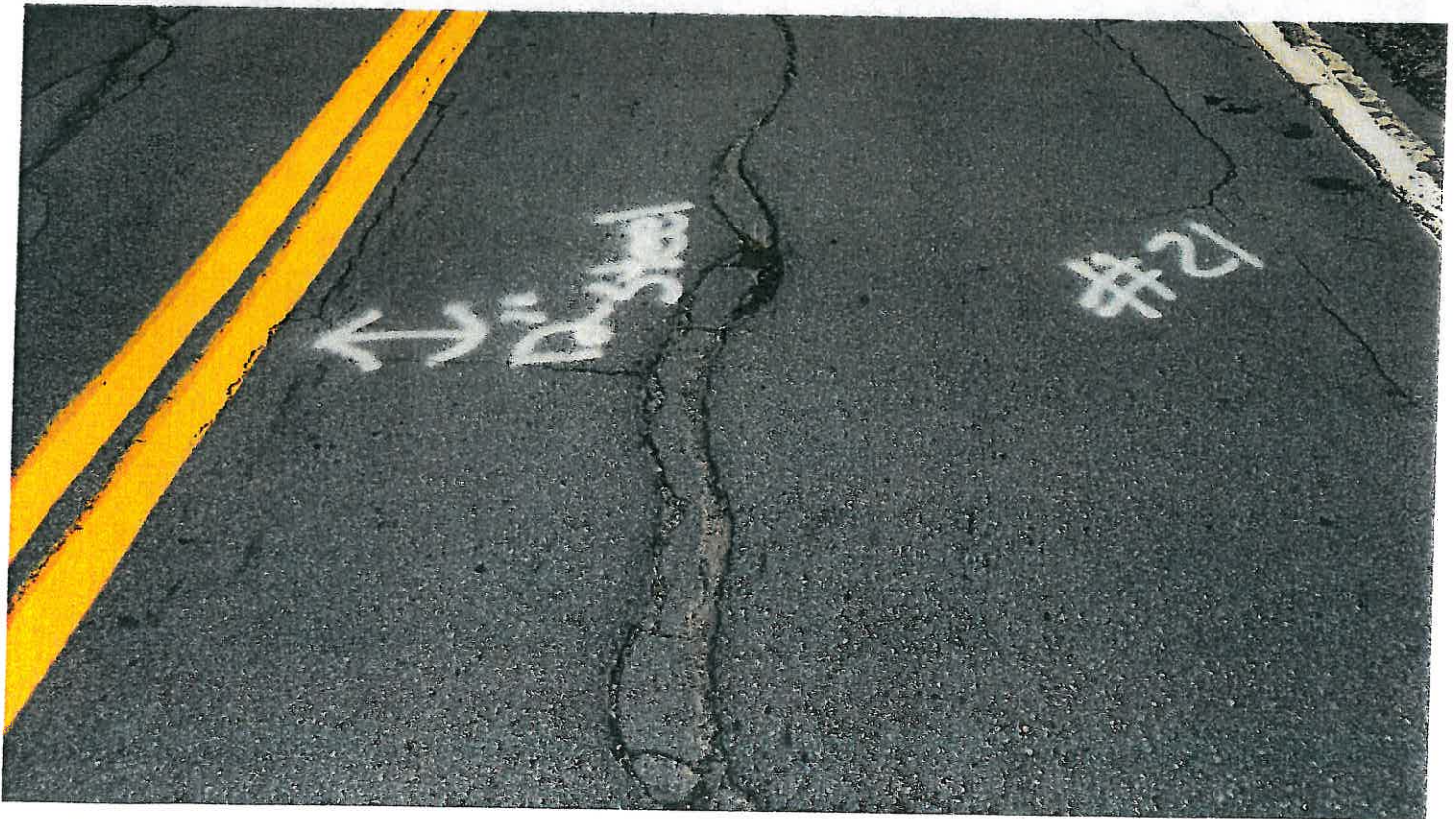
Pipe #21, 12" CMP, pavement conditions at crossing.
