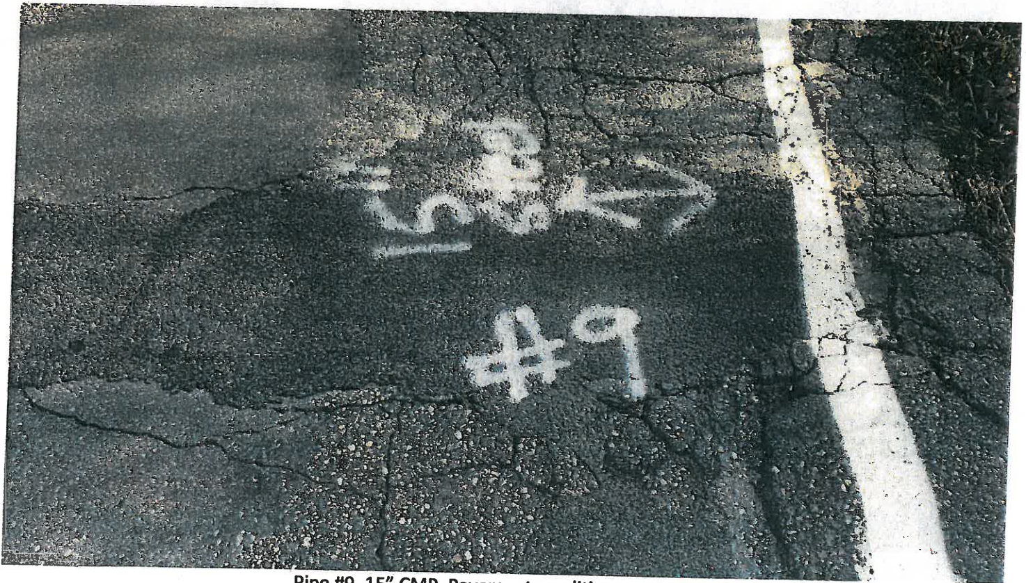
Pipe #9, 15" CMP, Pavement condition at crossing.
