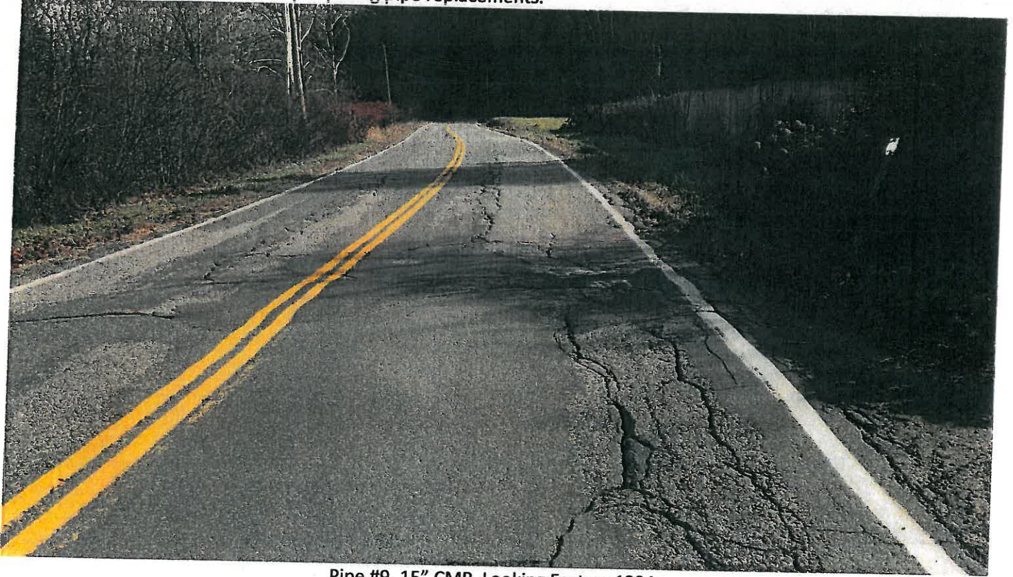
Pipe #9, 15" CMP, Looking East on 123A.
