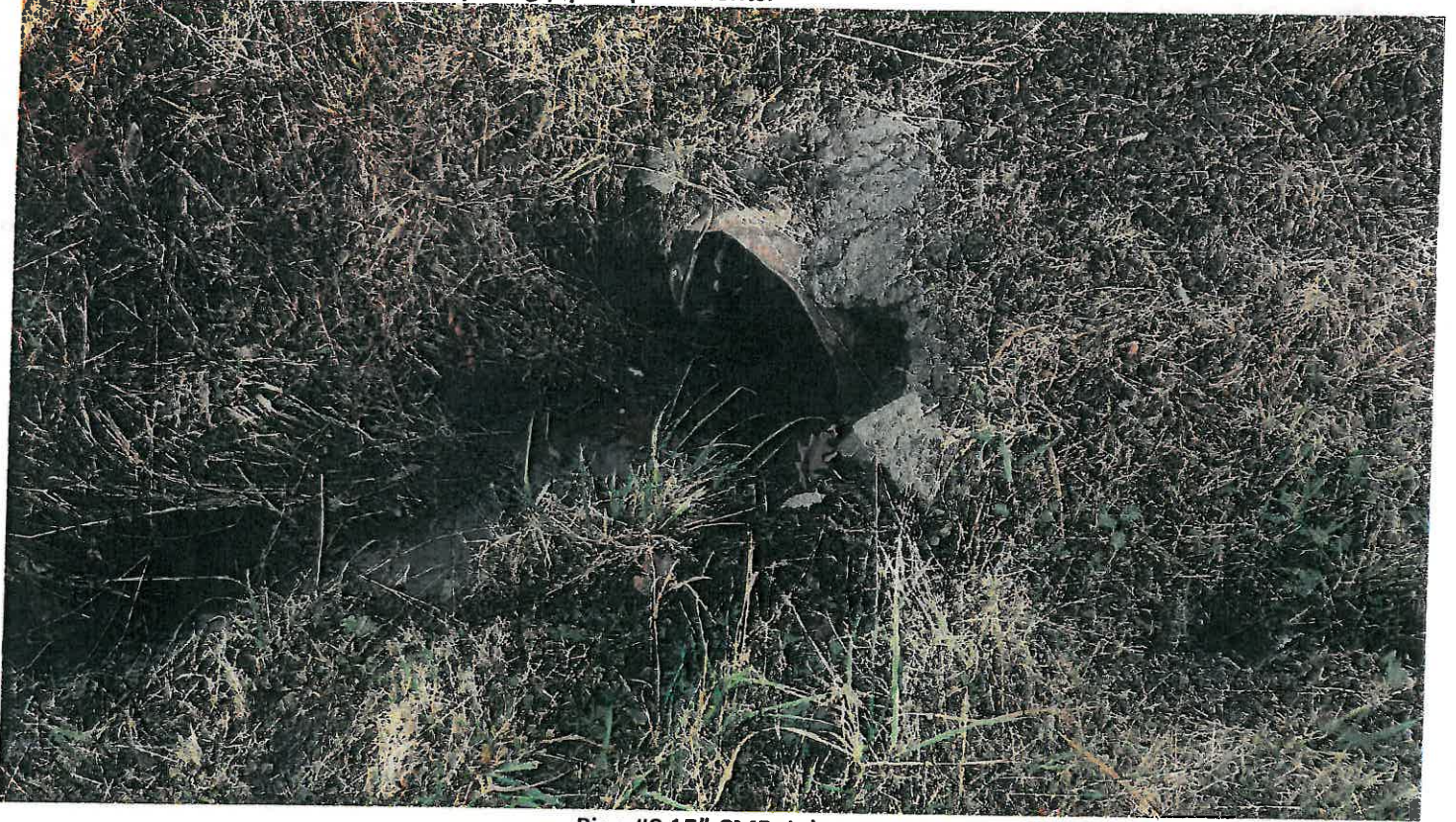
Pipe #8 15" CMP, Inlet.
