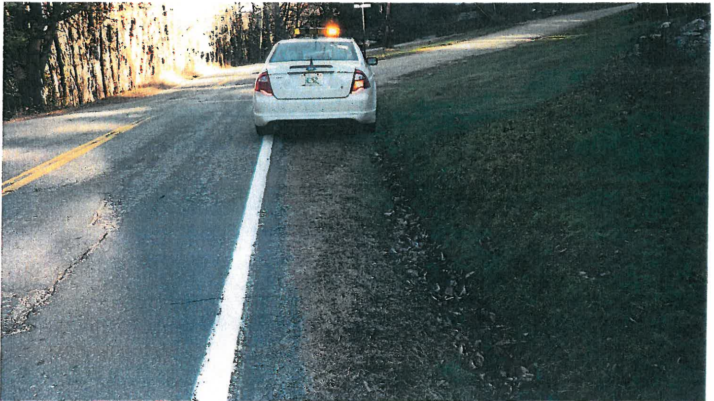
Pipe #35, 15" CMP, inlet ditch.
