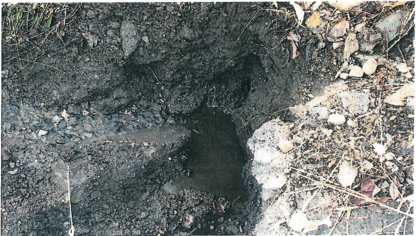
Pipe #36, 15" CMP, outlet.
