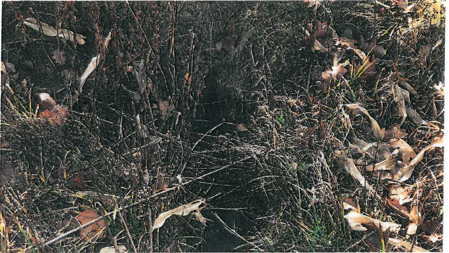
Pipe #8, 15" CMP, outlet.
