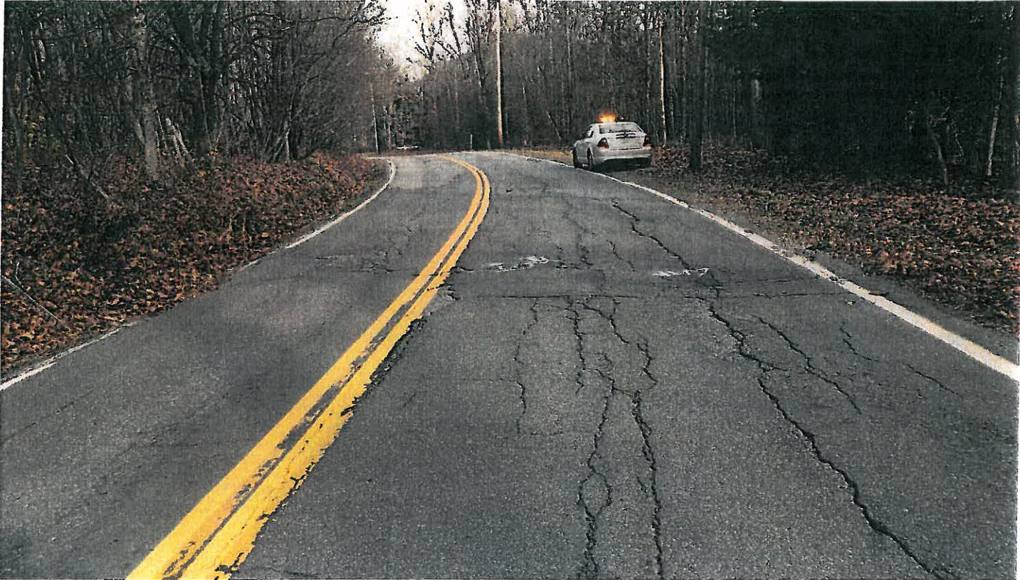
Pipe #17, 15" CMP, Looking East on 123A.
