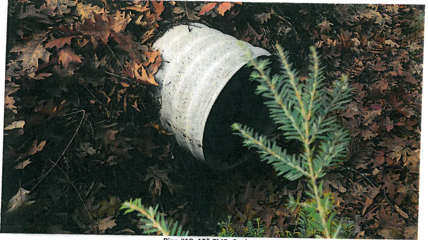
Pipe #18, 15" CMP, Outlet.
