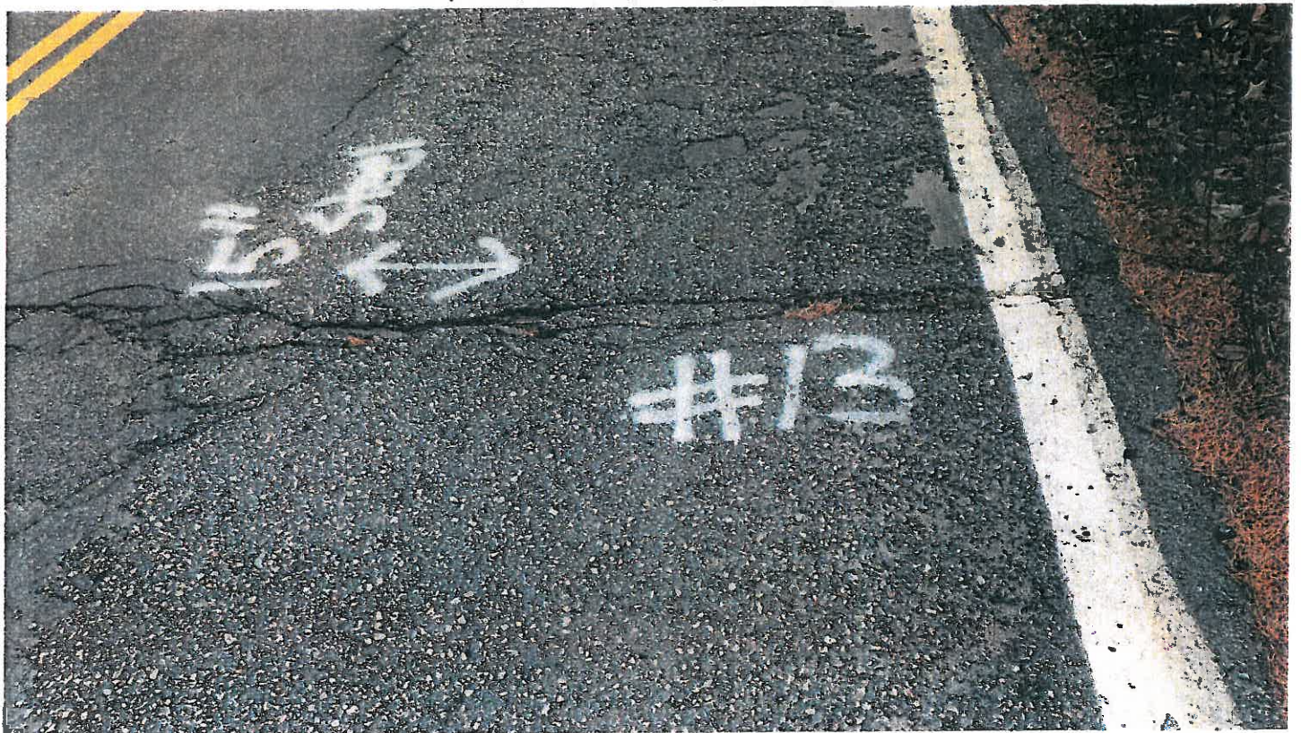
Pipe #13, Pavment Condition at Crossing.
