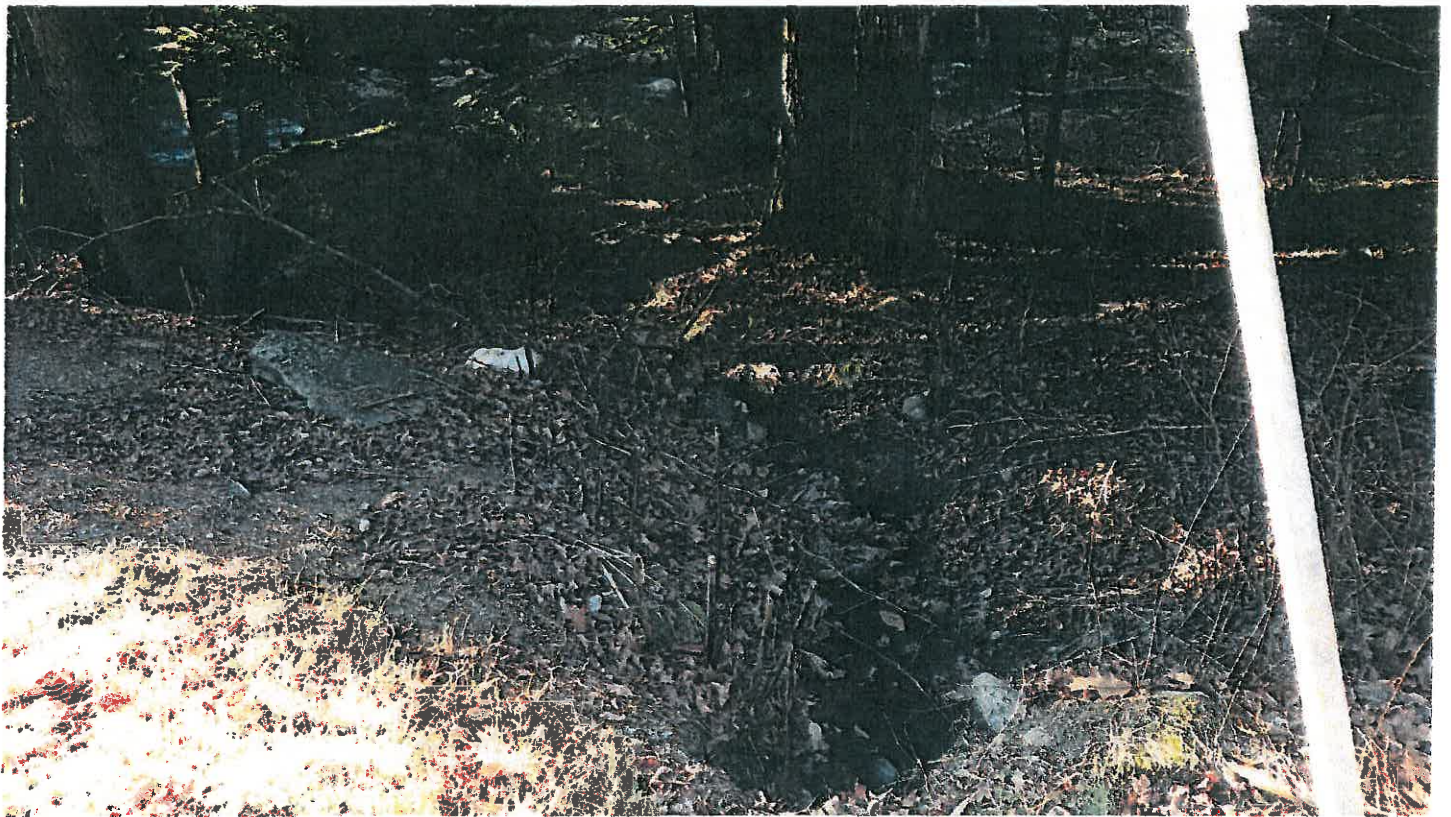
Pipe #34, 12" CMP looking at outlet.
