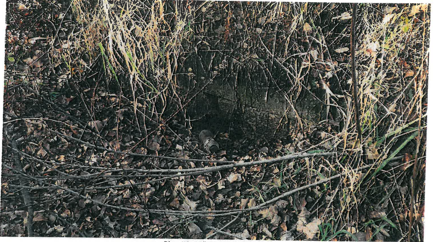
Pipe #6, 18" Concrete Inlet.
