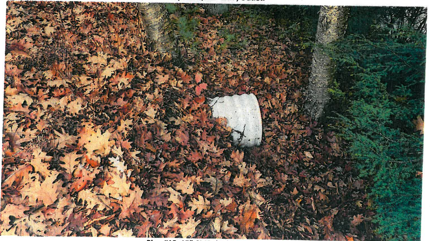
Pipe #18, 15" CMP, looking at outlet.
