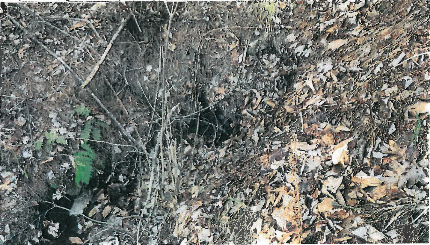
Pipe #30, 15" CMP, outlet.
