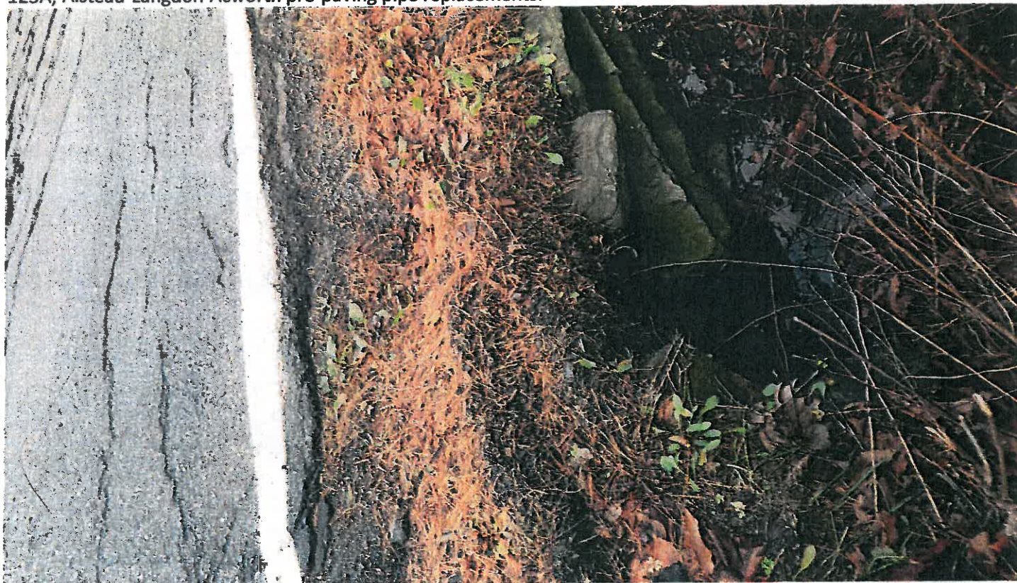
Pipe#11, 24" CMP, inlet.
