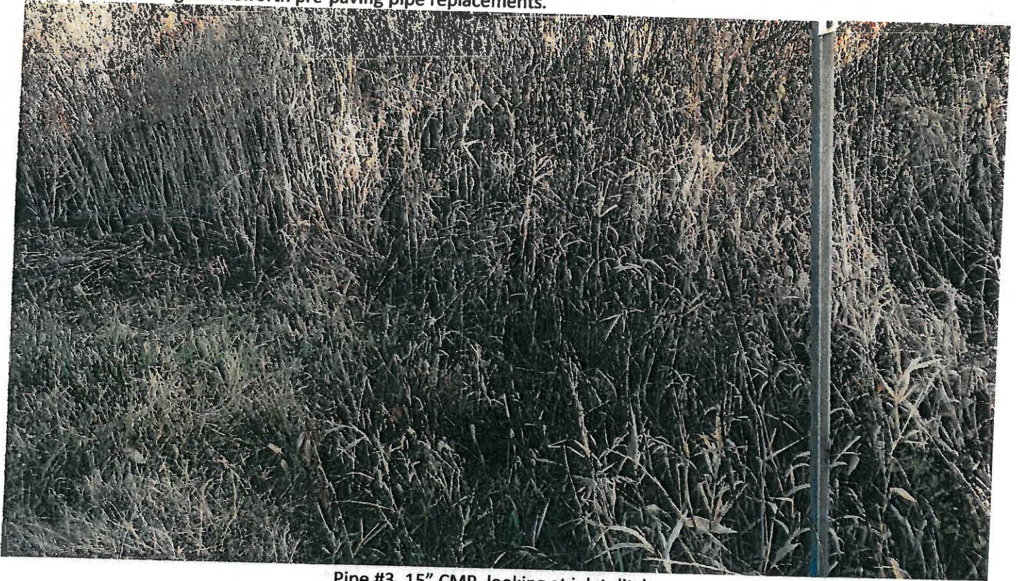
Pipe #3, 15" CMP, looking at inlet ditch.
