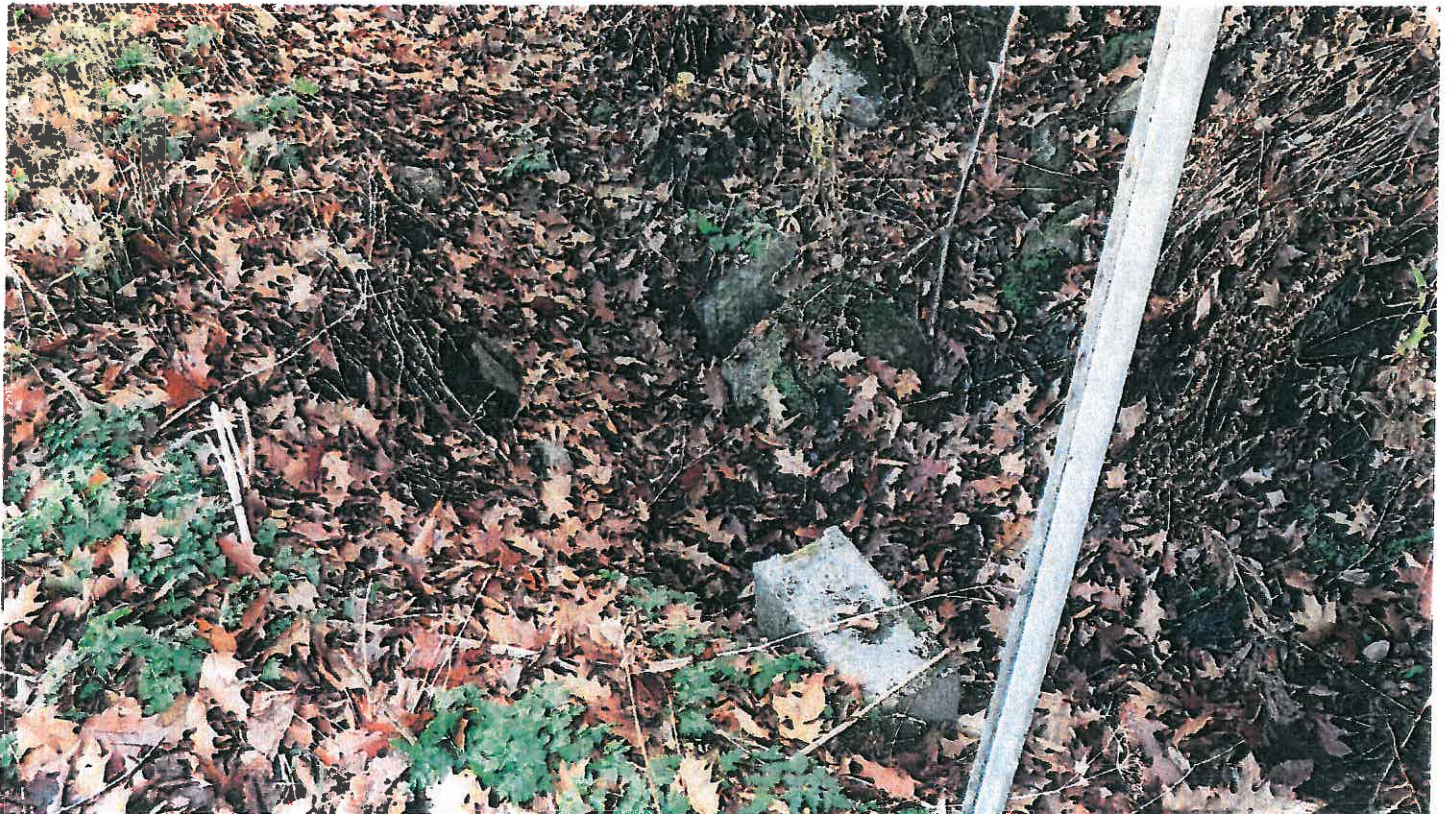
Pipe #7, 15" RCP, looking at inlet.
