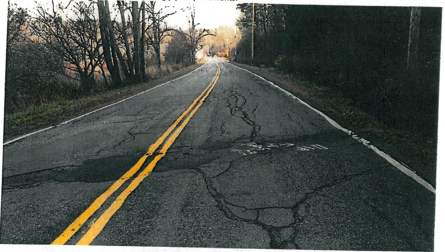
Pipe#11, 24" CMP looking east on 123A.
