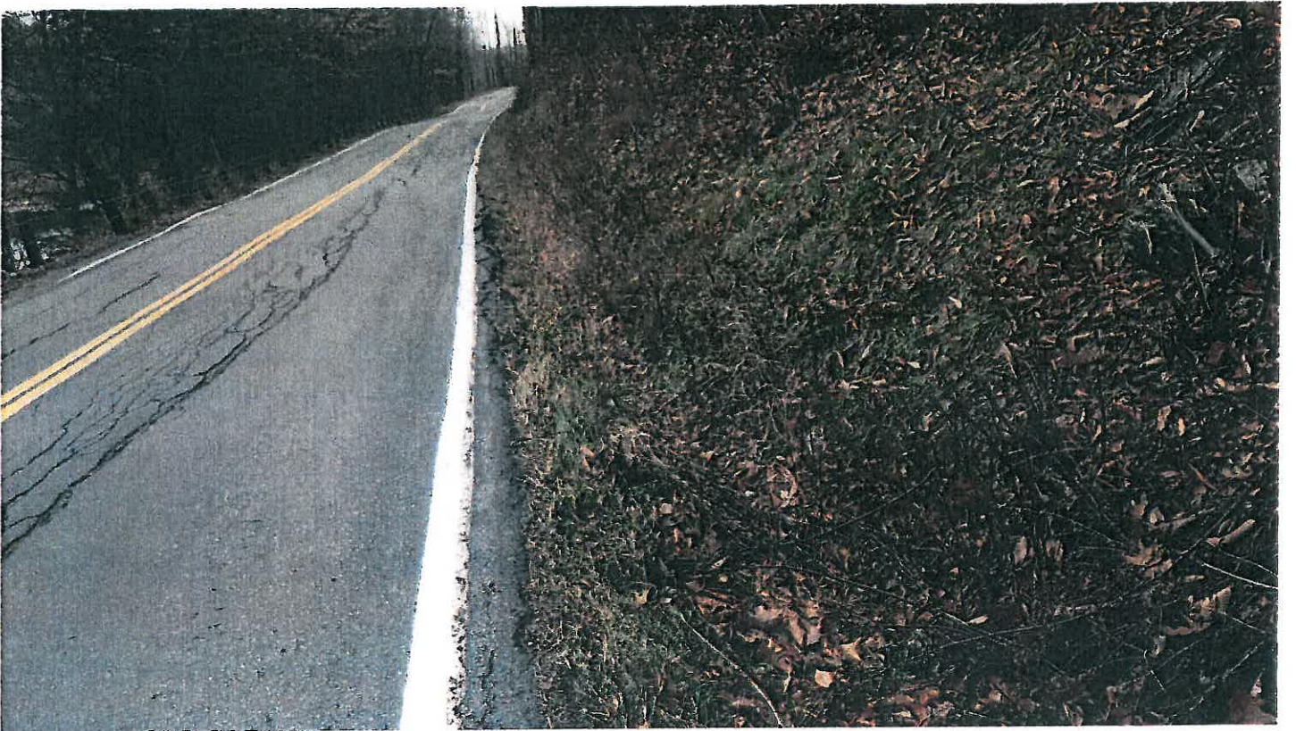
Pipe #21, 12" CMP, Pipe inlet roadside ditch.
