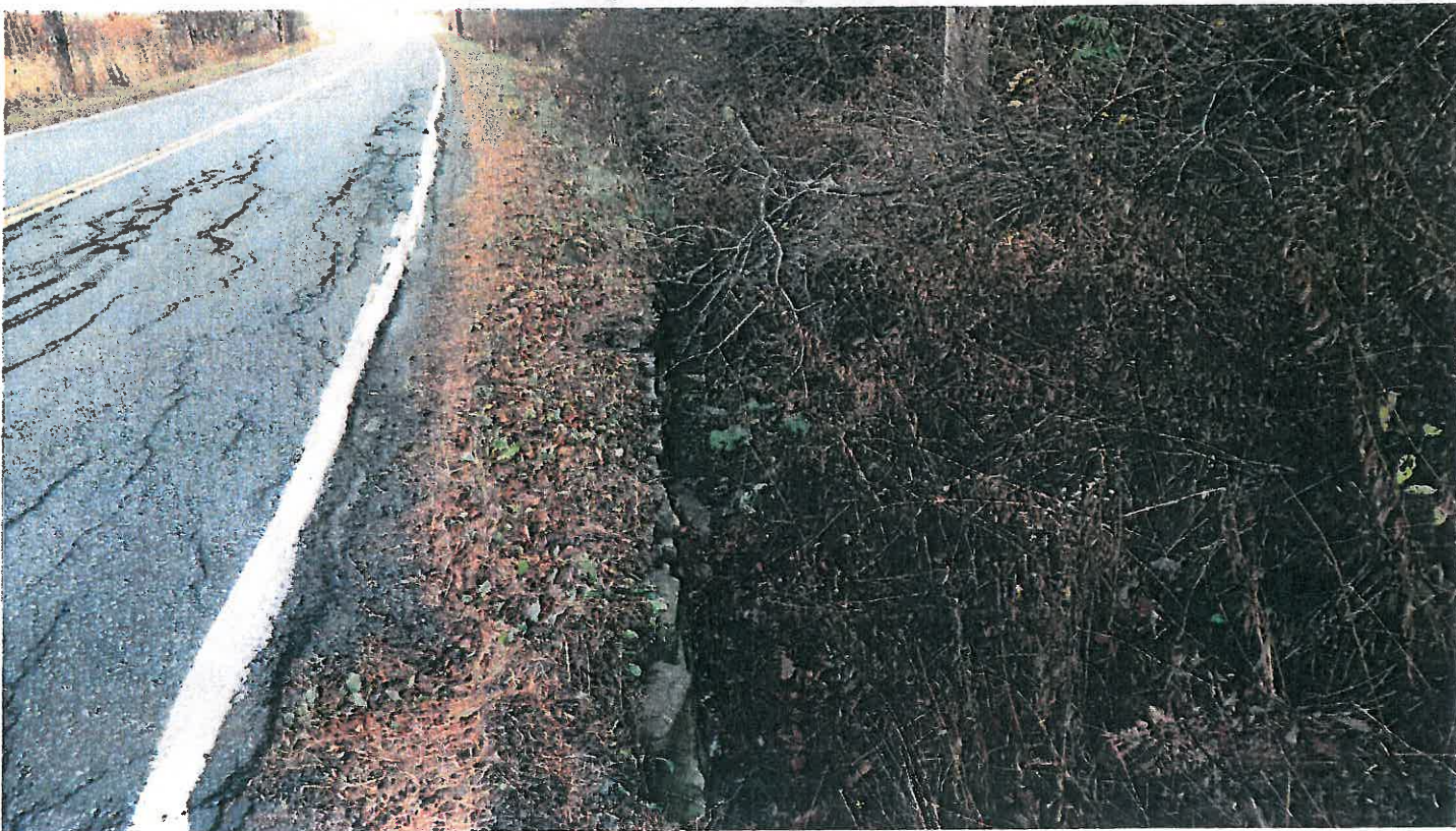
Pipe #11, 24" CMP inlet.
