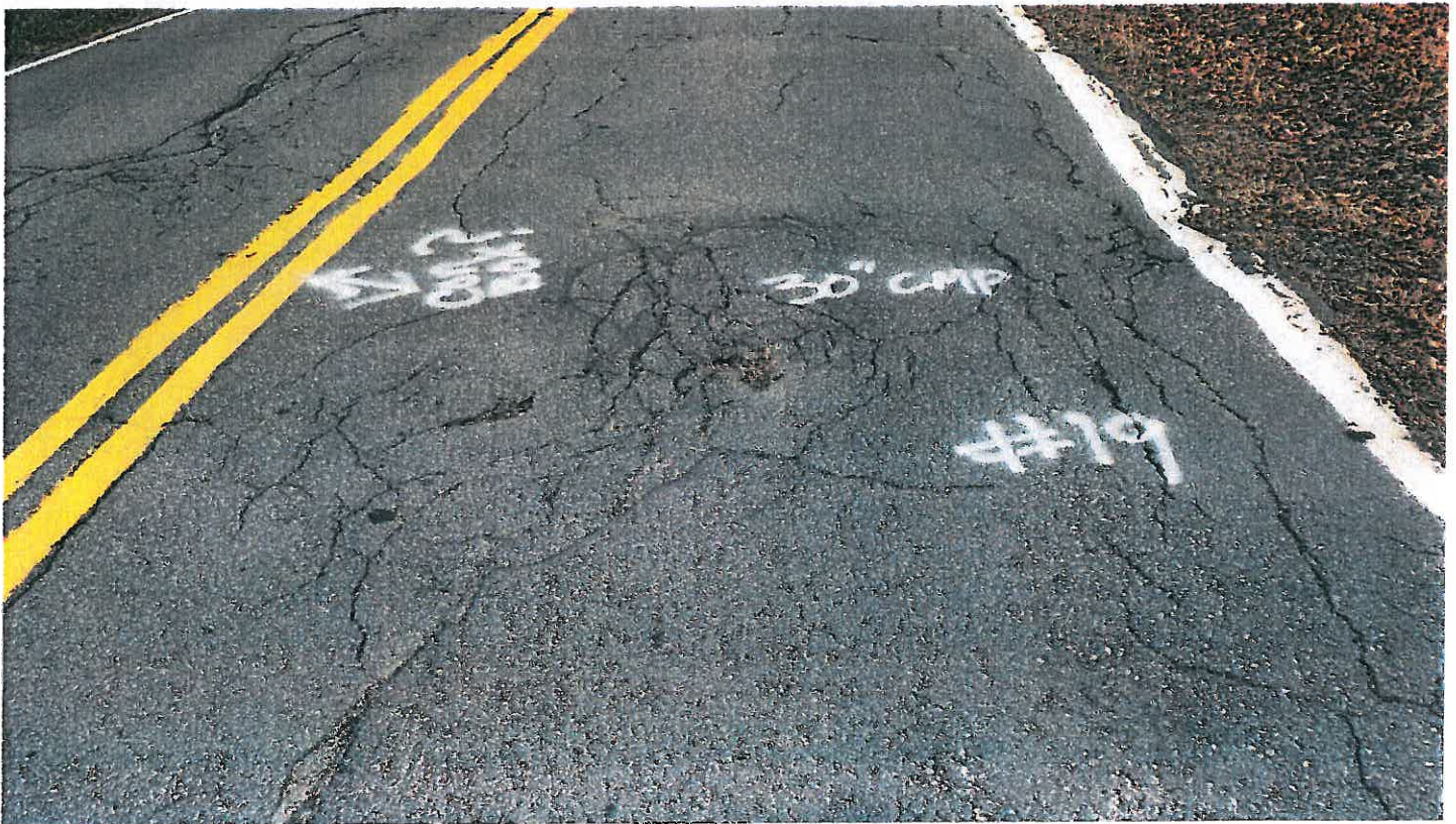
Pipe #19, 2x3 box 30" CMP, pavement condition at crossing.
