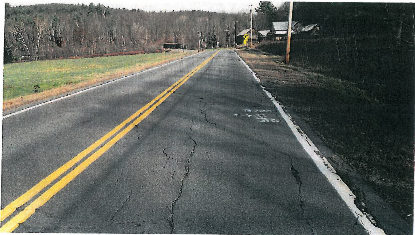
Pipe #6, 18" Concrete, Looking East on 123A.
