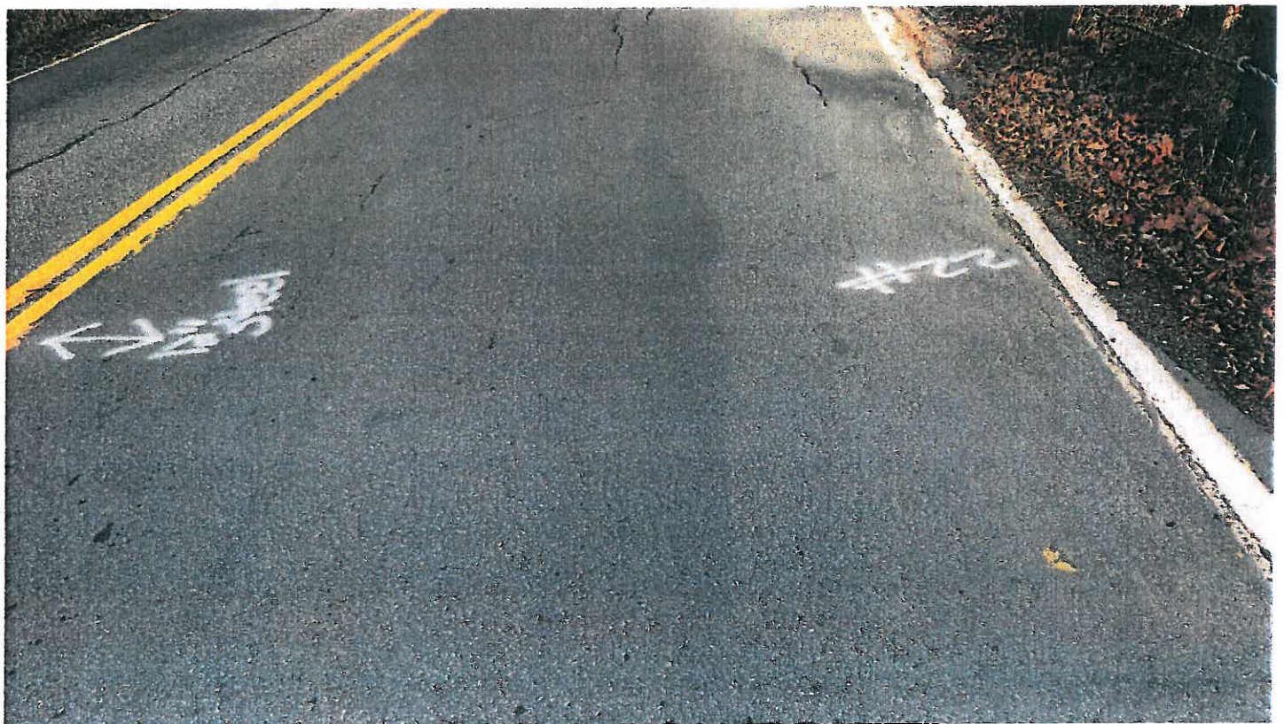
Pipe #22, 12" CMP, pavement condition at crossing.
