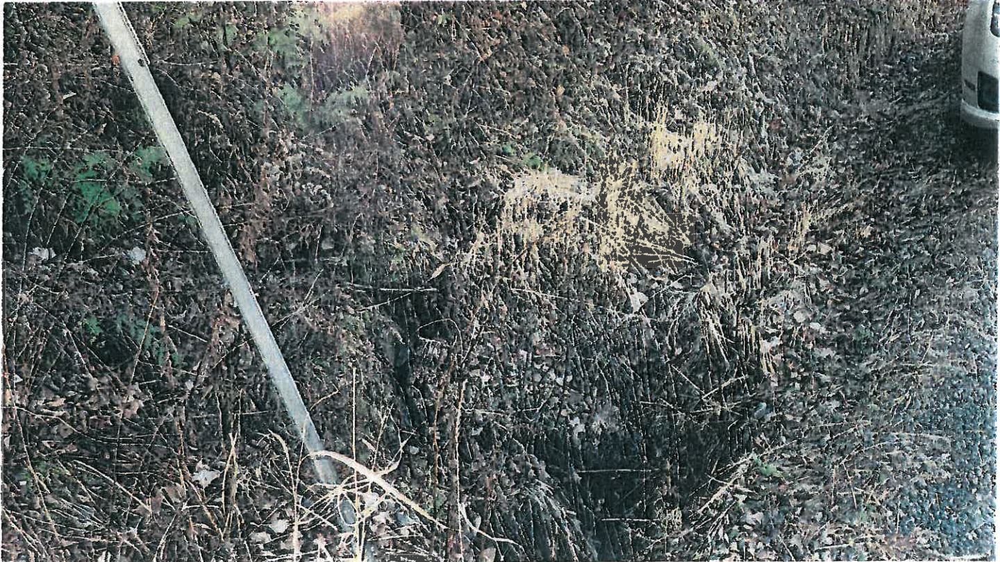
Pipe #37, 15" CMP inlet ditch.
