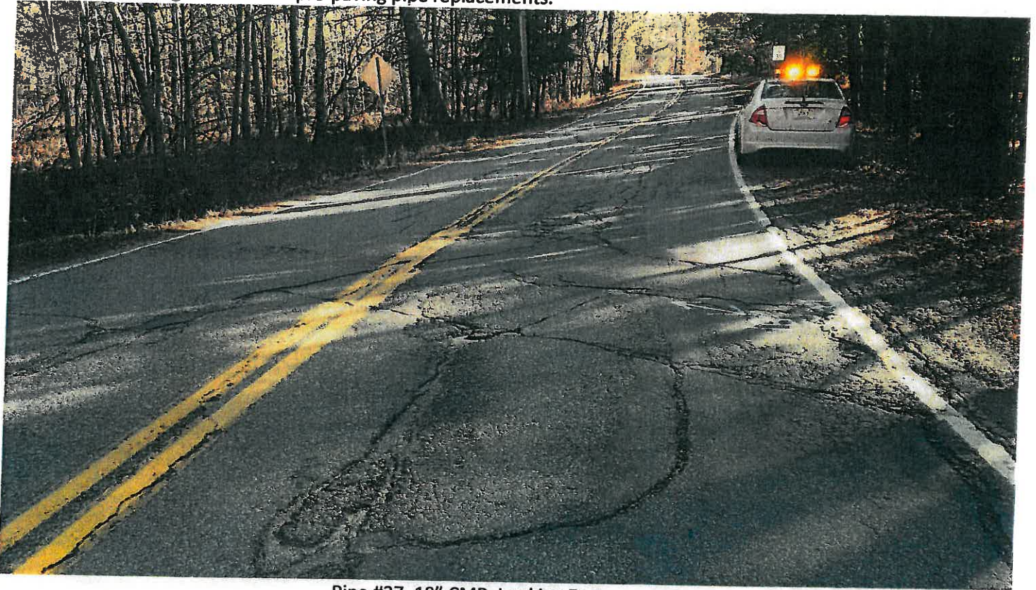
Pipe #27, 18" CMP, Looking East on 123A.
