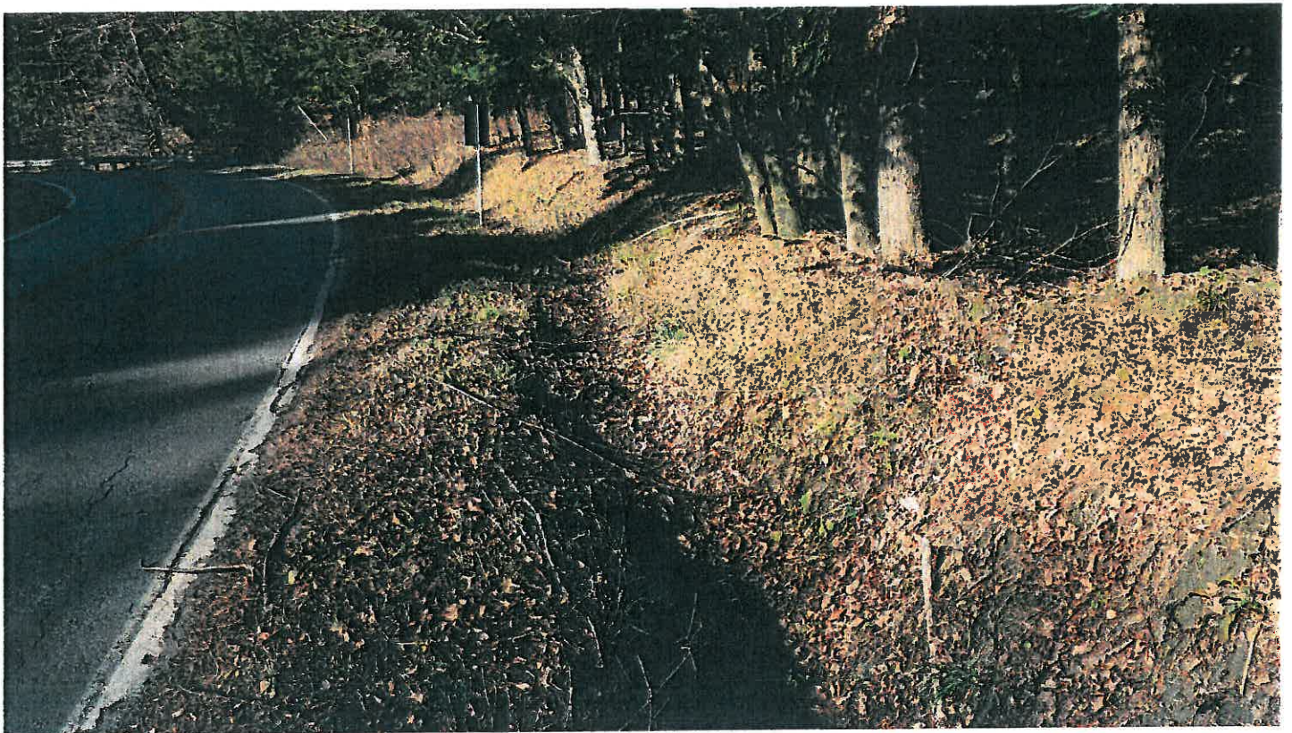
Pipe #23, 15" CMP, Roadside Ditch at inlet.
