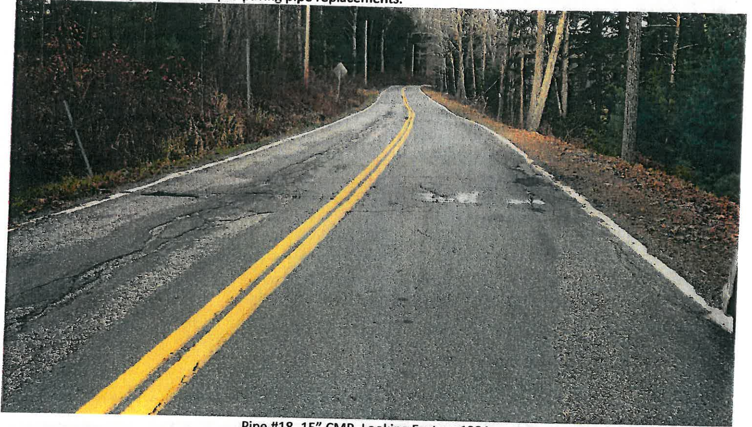
Pipe #18, 15" CMP, Looking East on 123A.
