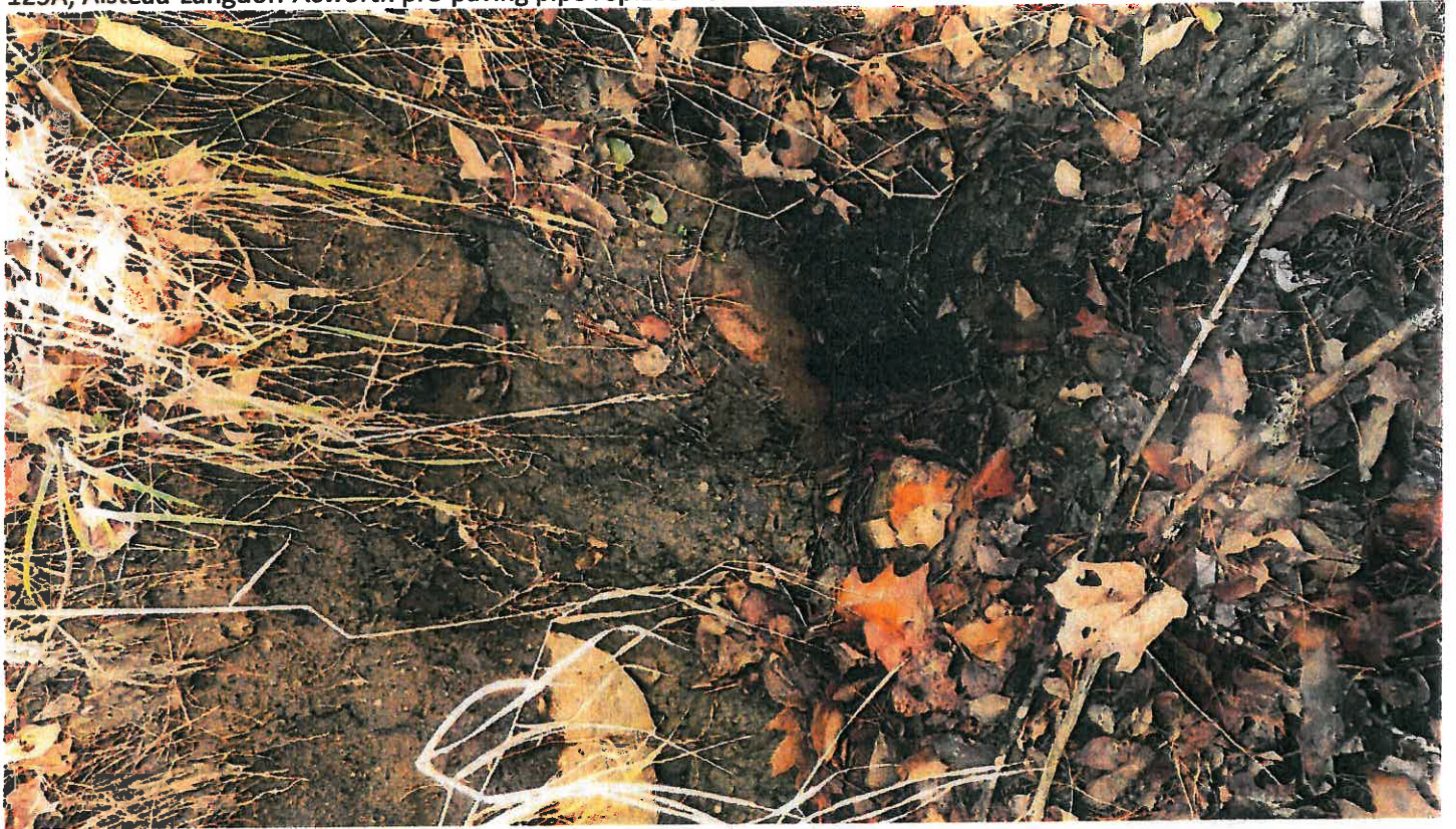
Pipe #23, 15" CMP, inlet.
