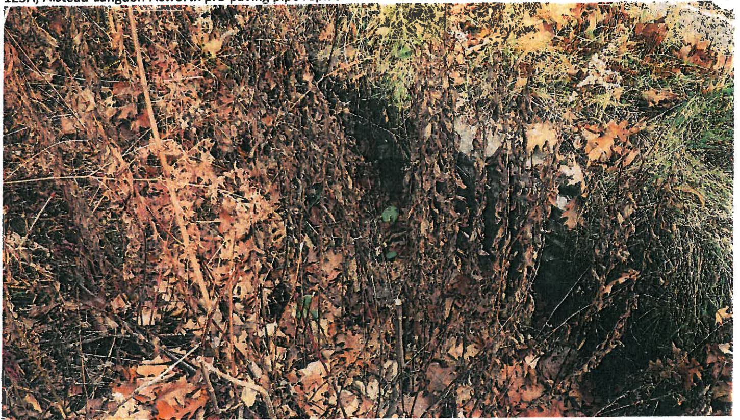
Pipe #18, 15" CMP, Inlet.
