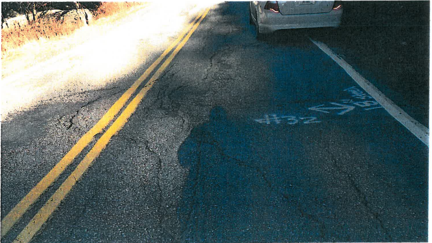
Pipe #32, 18" CMP, pavement condition at crossing.
