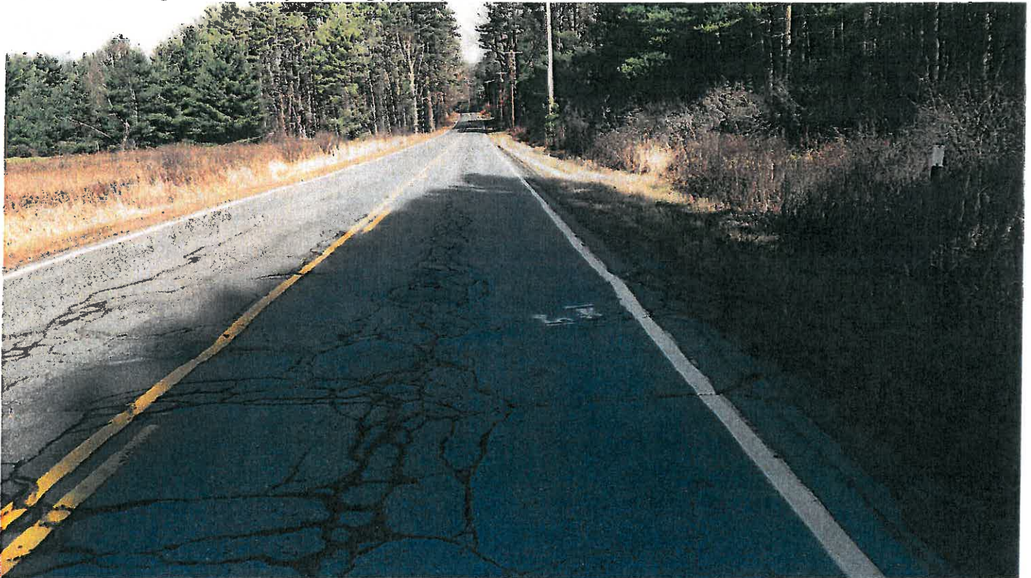
Pipe #3, 15" CMP, Looking East on 123A.
