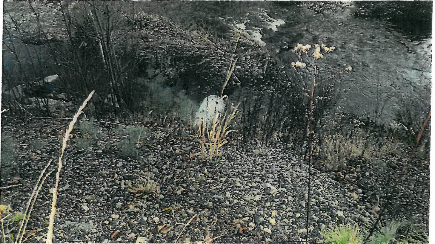
Pipe #37, 15" CMP, outlet.
