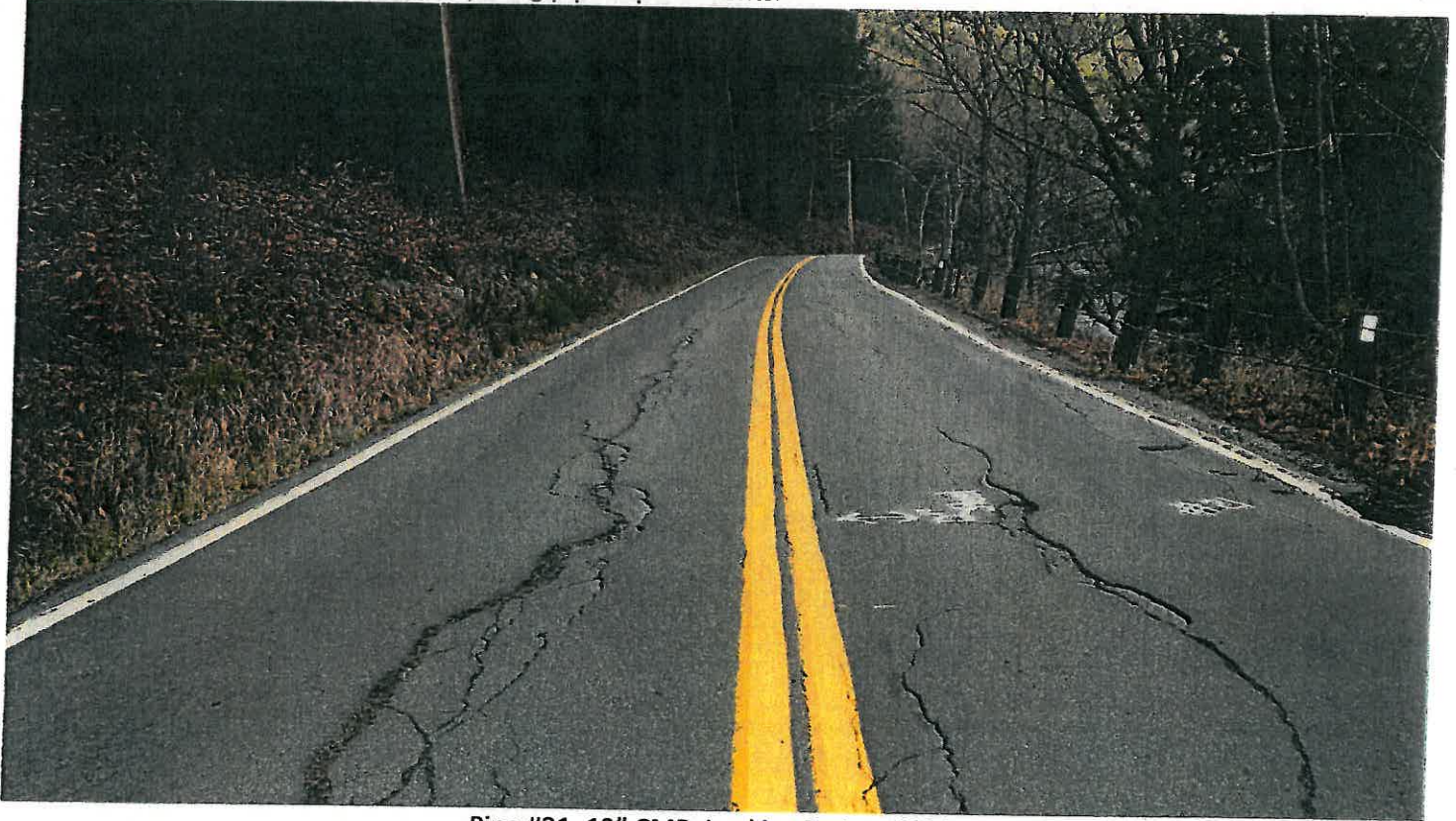
Pipe #21, 12" CMP, Looking East on 123A.
