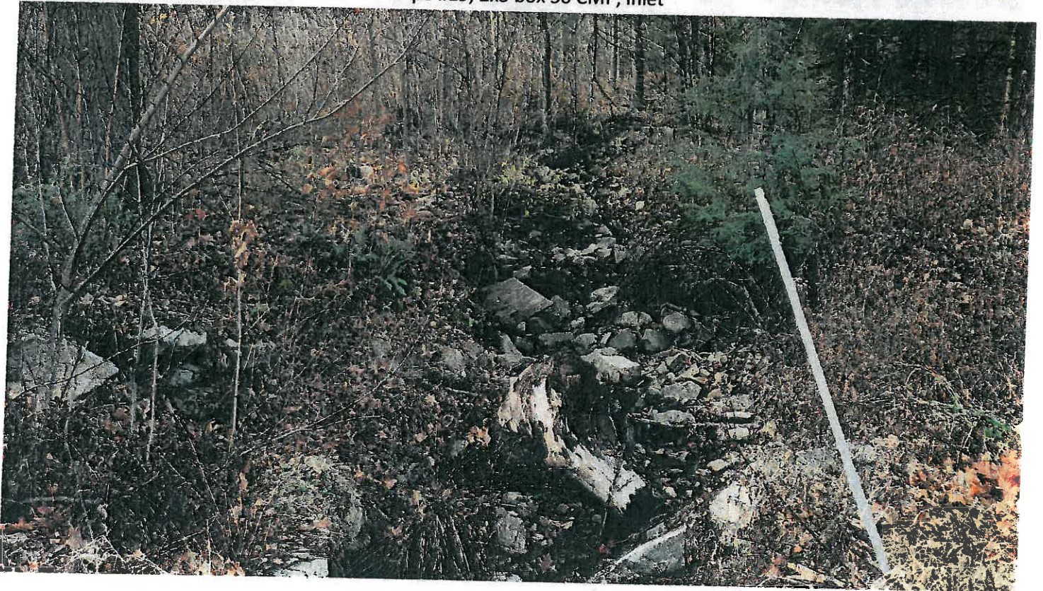
Pipe #19, 2x3 box 30 CMP, Looking at inlet.
