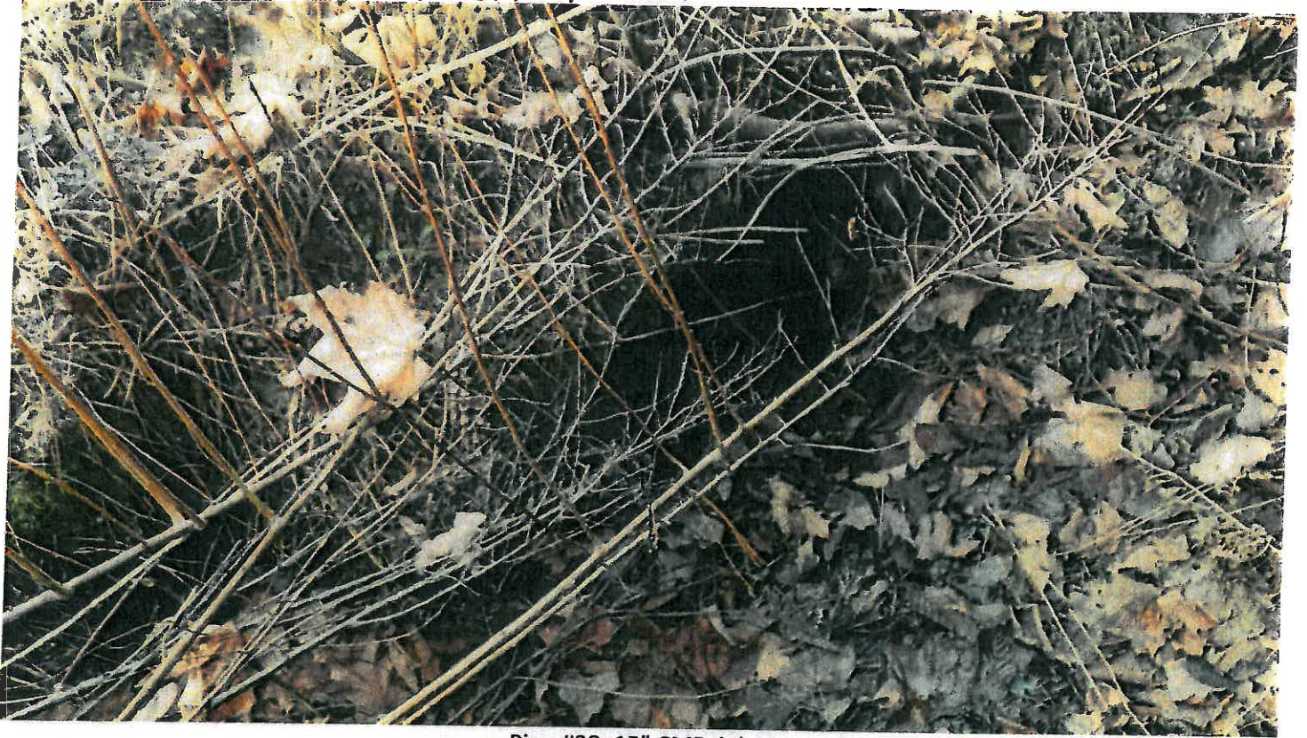
Pipe #38, 15" CMP, inlet.
