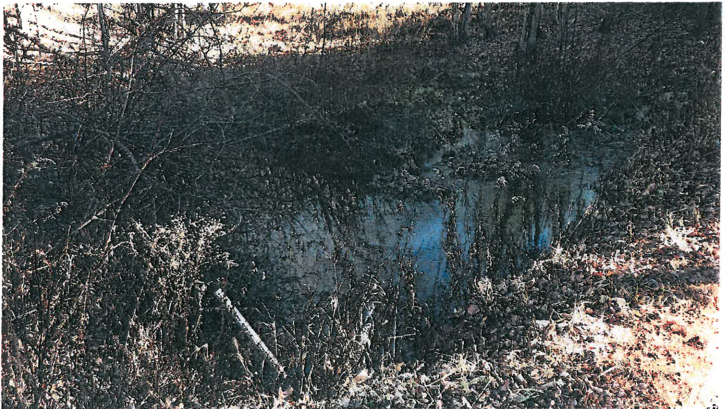
Pipe #27, 18" CMP, Looking at inlet.
