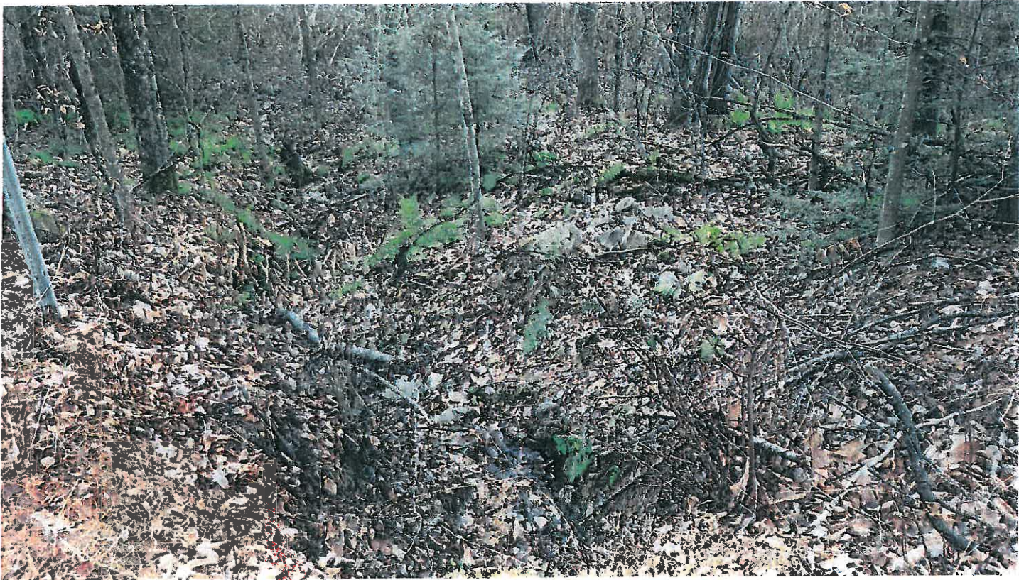
Pipe #30, 15" CMP, looking at outlet.
