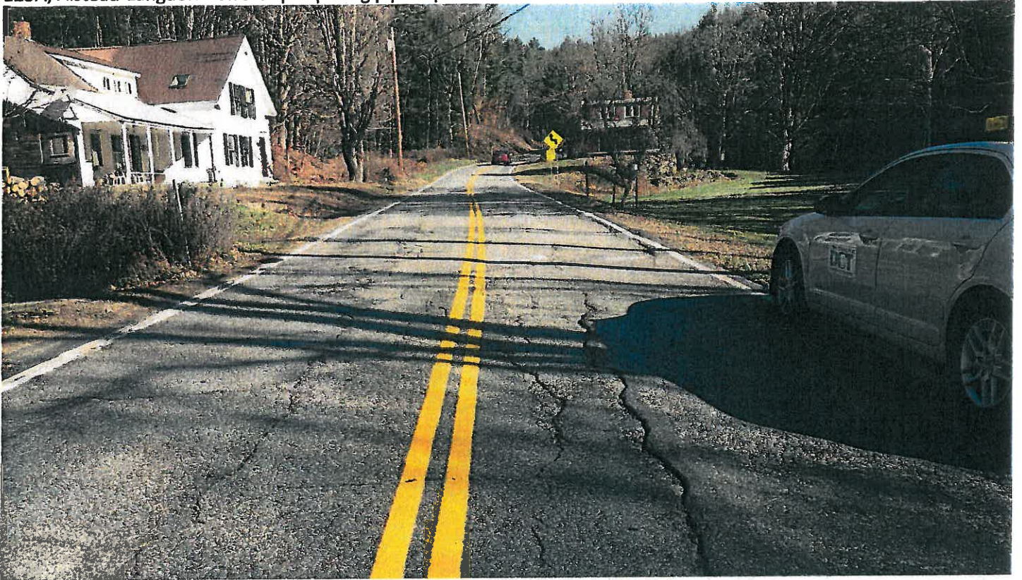
Pipe #24, 12" CMP, Looking East on 123A.
