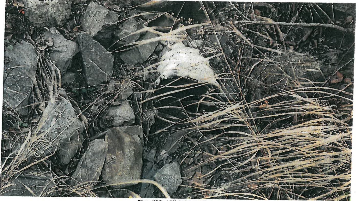
Pipe #23, 15" CMP, outlet.
