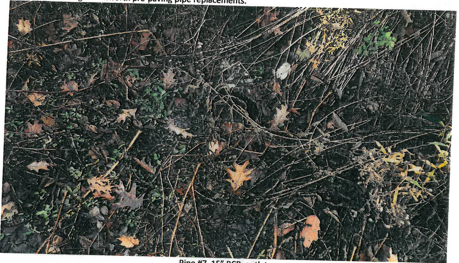
Pipe #7, 15" RCP, outlet.
