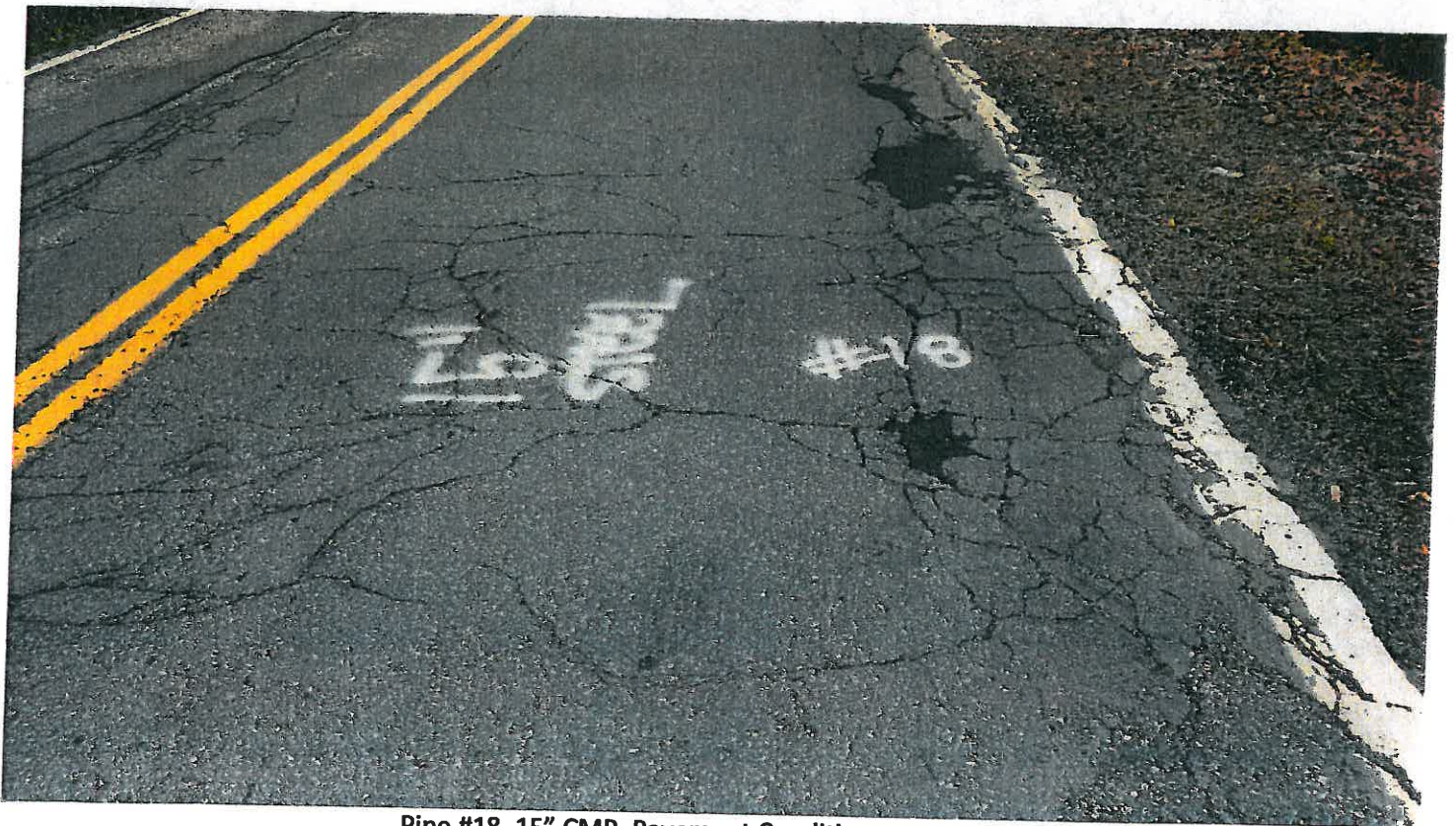
Pipe #18, 15" CMP, Pavement Conditions at crossing.
