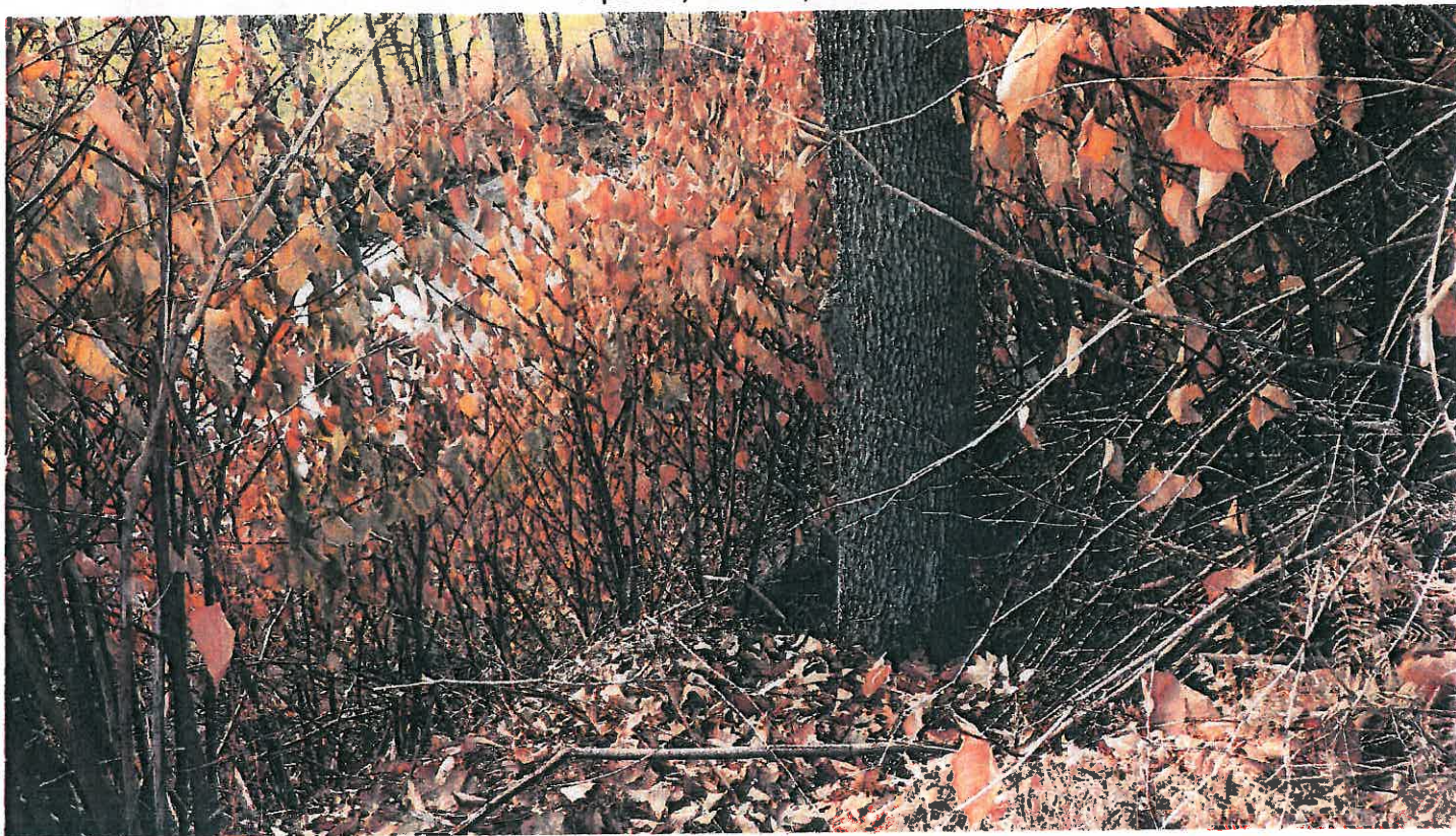
Pipe #13, 15" CMP, looking at outlet.
