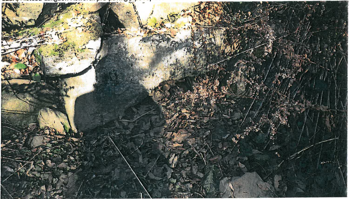
Pipe #24, 12" CMP, outlet.
