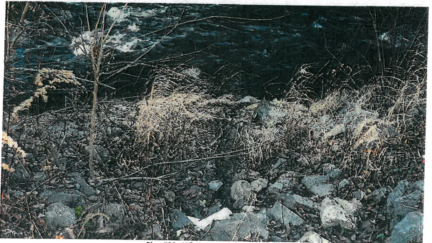
Pipe #23, 15" CMP, Looking at outlet.
