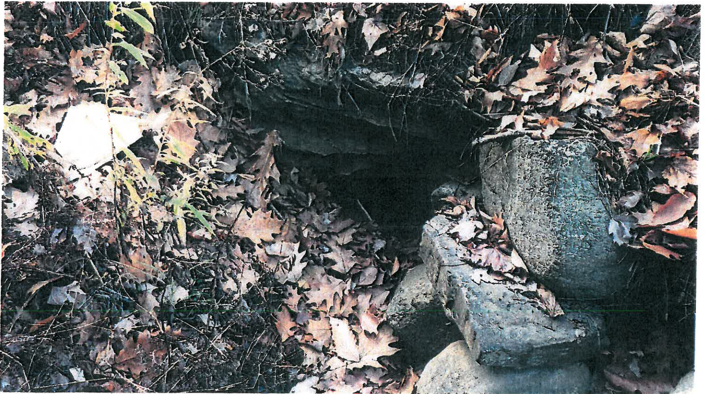
Pipe#1, 15" CMP inlet
