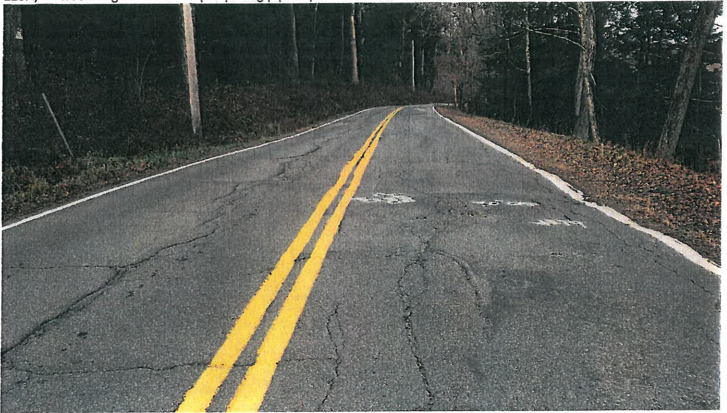
Pipe #19, 2x3 box 30" CMP, Looking East on 123A.
