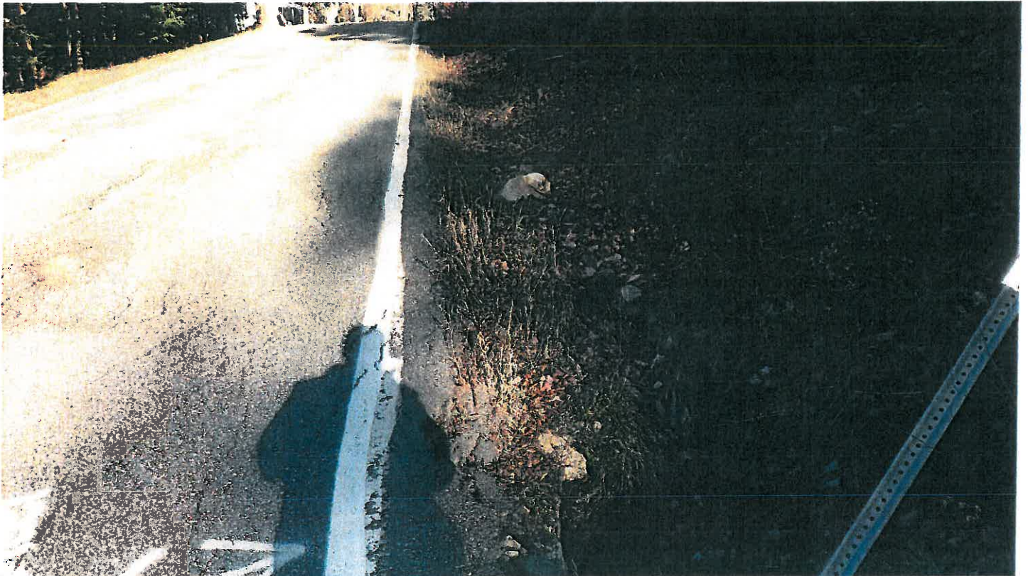
Pipe #33, 15" CMP, inlet ditch.
