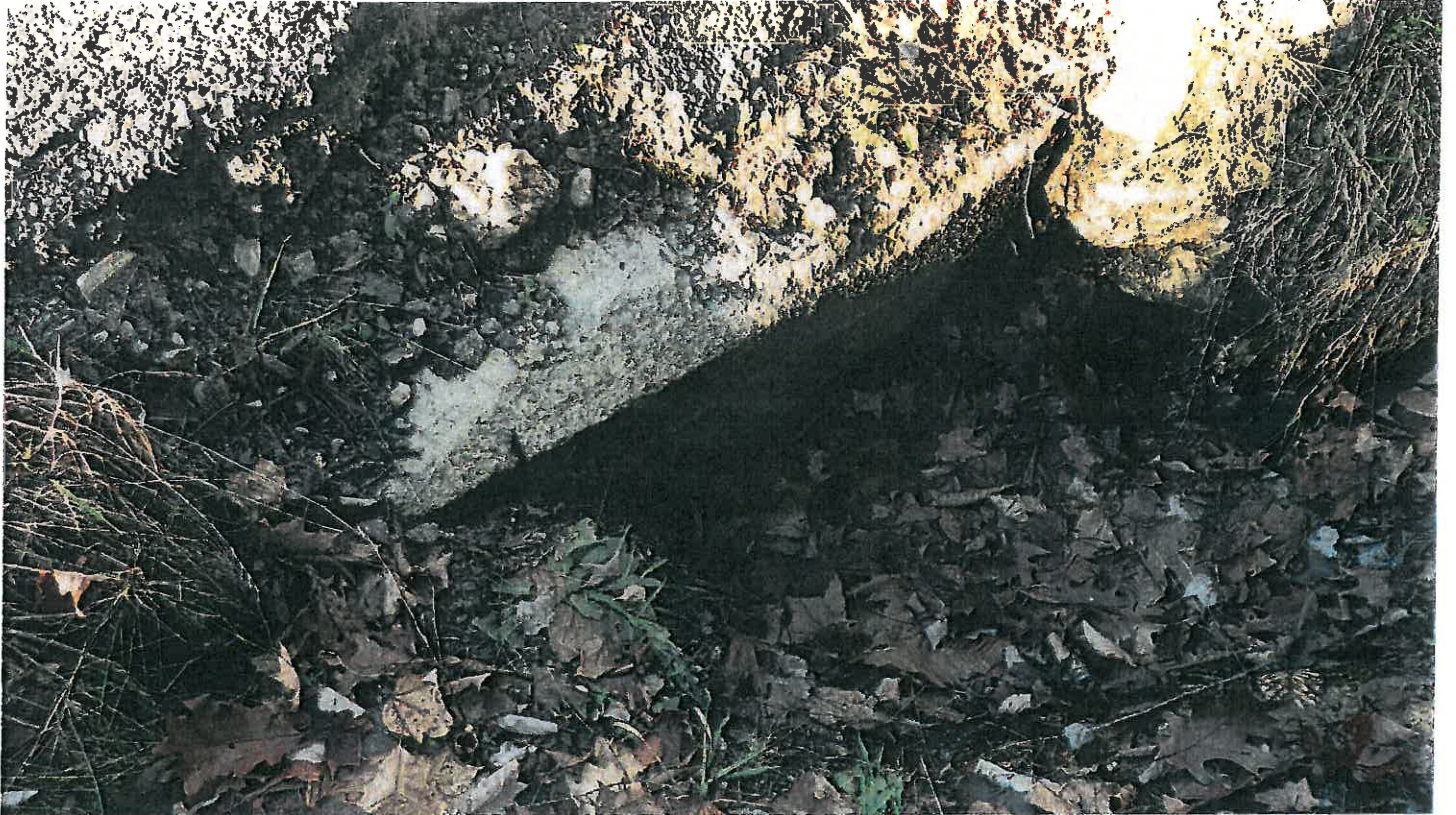
Pipe #33, 15" CMP, Inlet.
