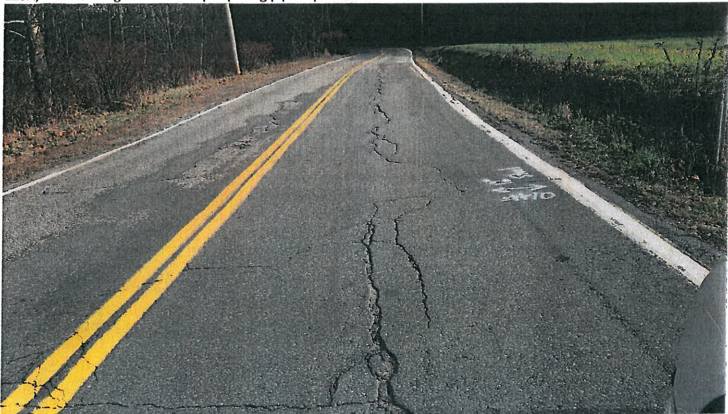
Pipe #10, 12" CMP, Looking East on 123A.
