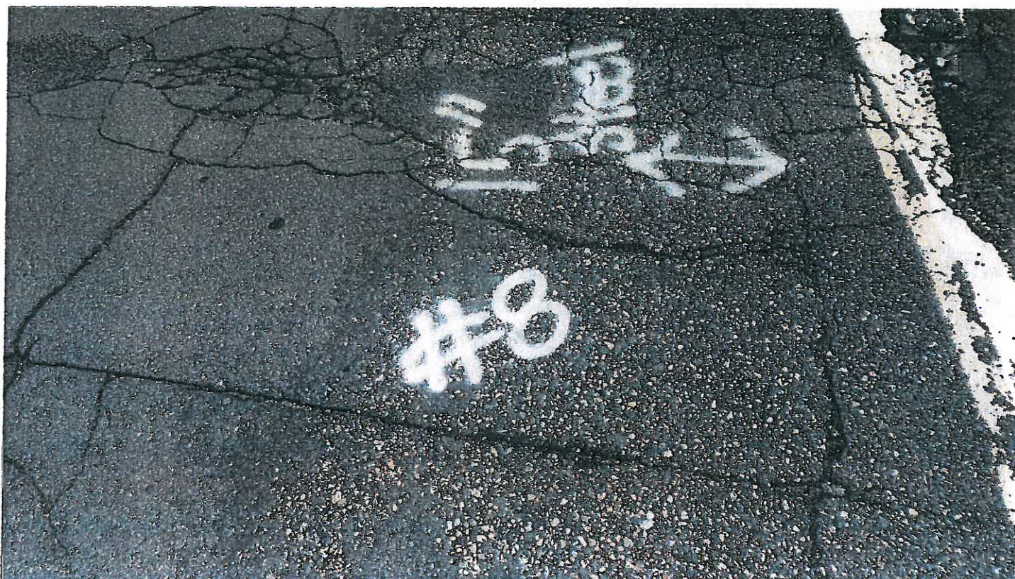
Pipe #8, 15" CMP, Pavment condition at crossing.
