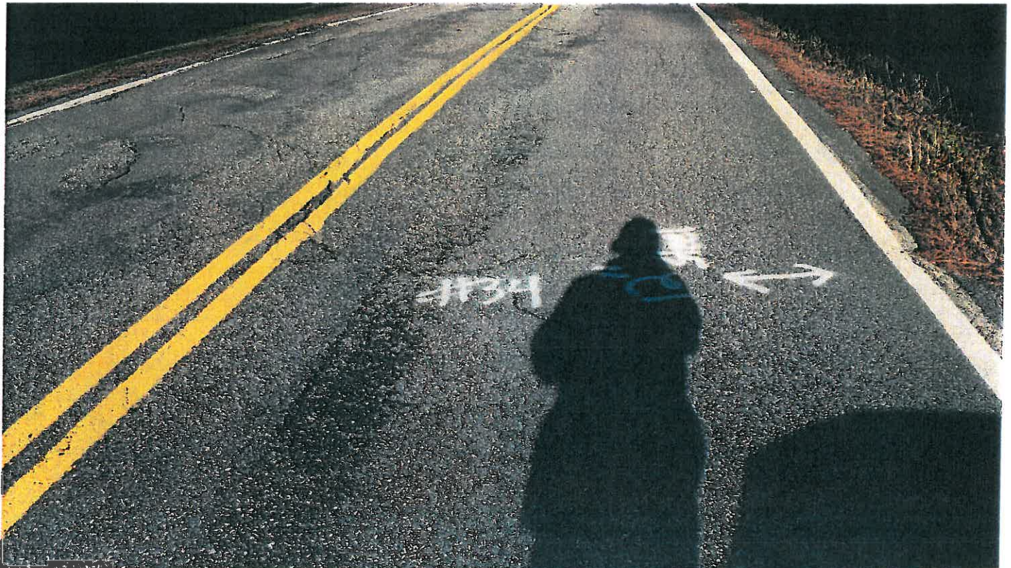
Pipe #34, 12" CMP, pavement condition at crossing.
