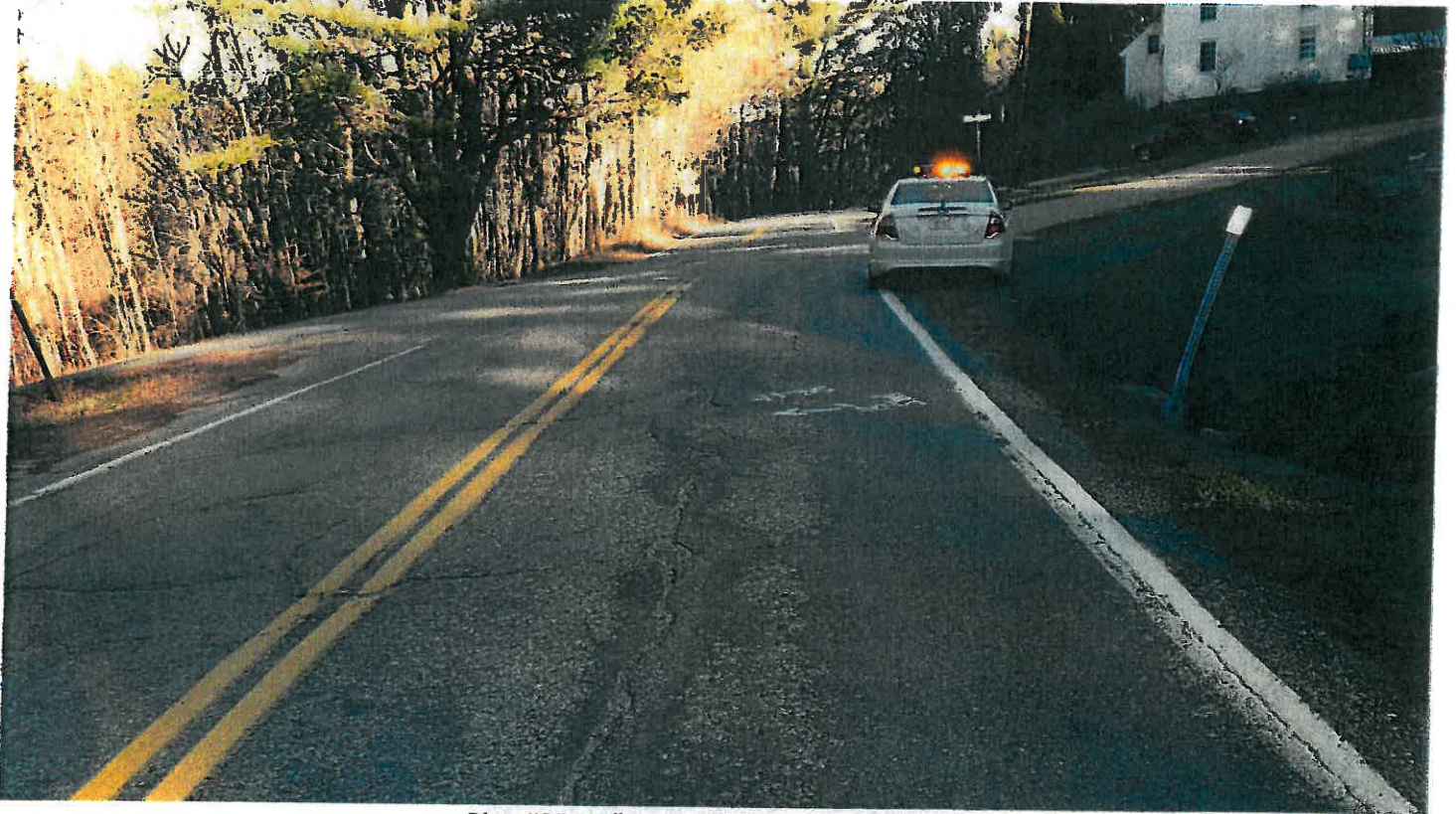
Pipe #35, 15" CMP, Looking East on 123A.
