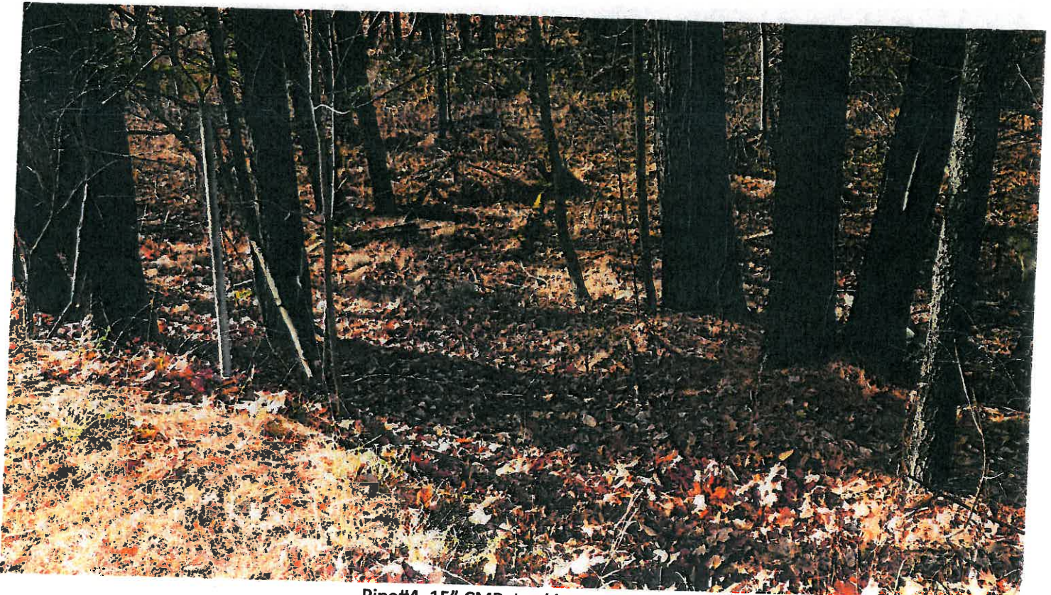
Pipe#4, 15" CMP, Looking at outlet.
