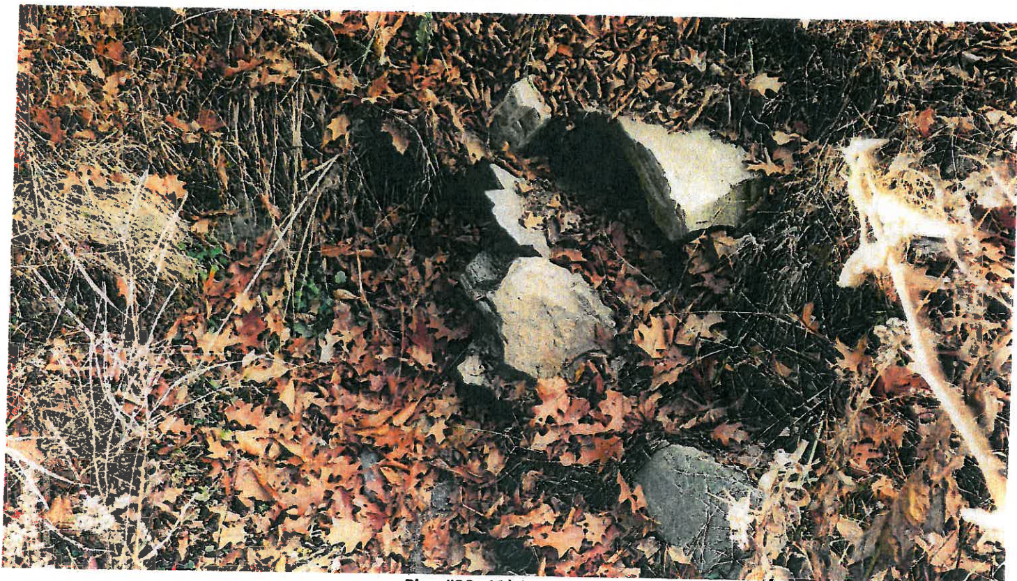
Pipe #22, 12' CMP, Inlet
