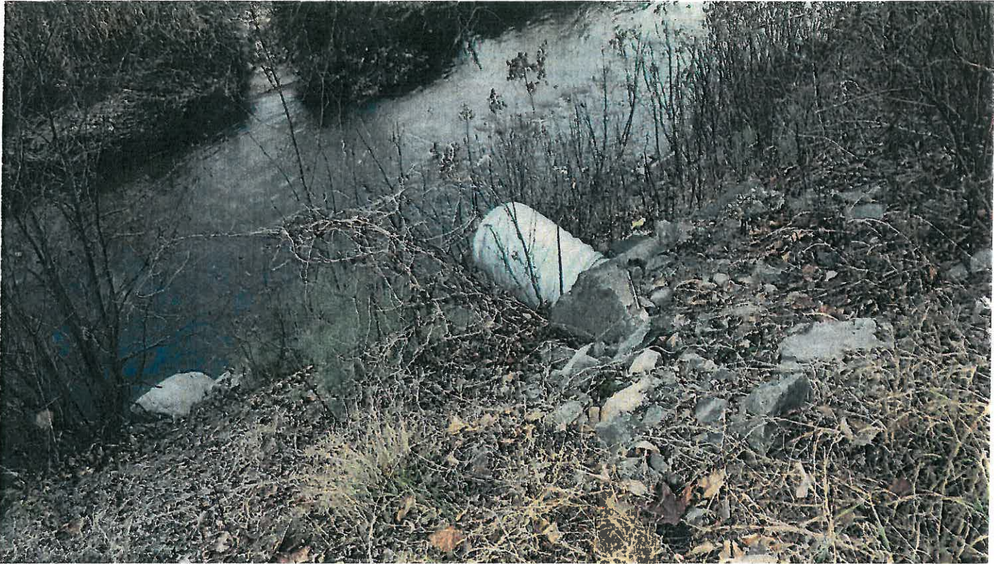
Pipe #38, 15" CMP, outlet.
