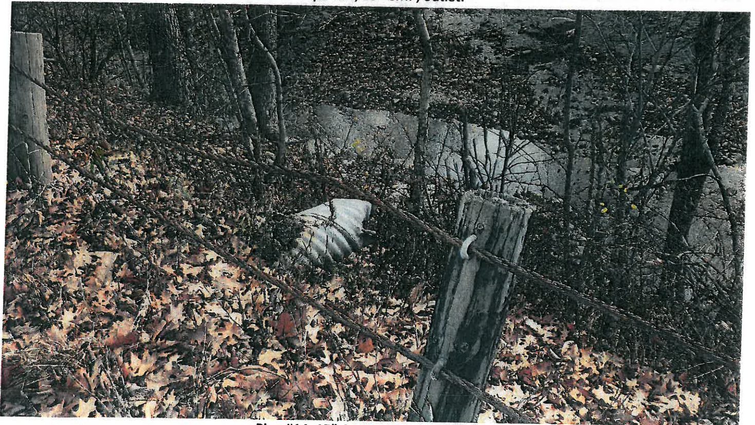
Pipe #14, 15" CMP, Looking at outlet.
