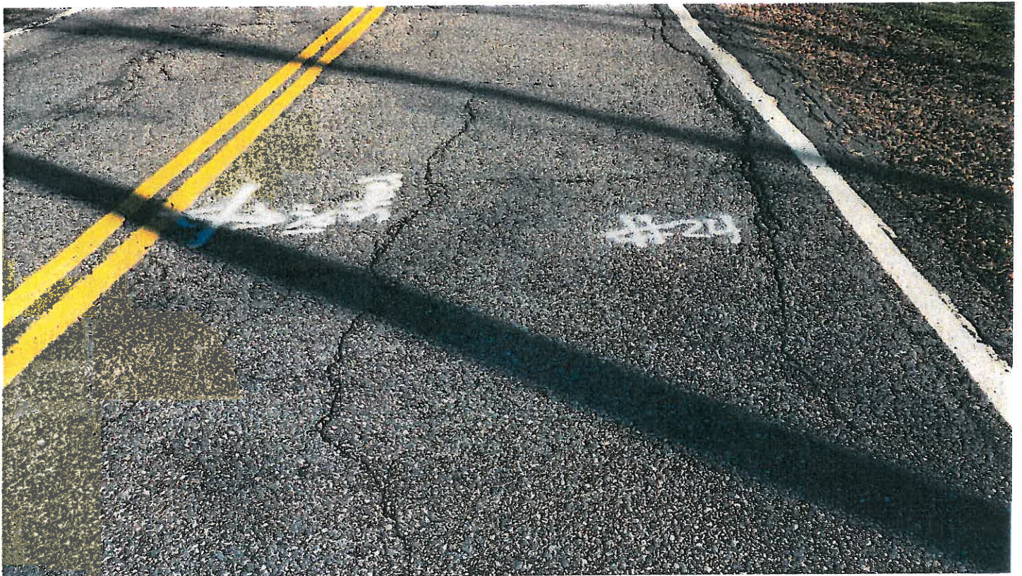
Pipe #24, 12" CMP, pavement condition at crossing.
