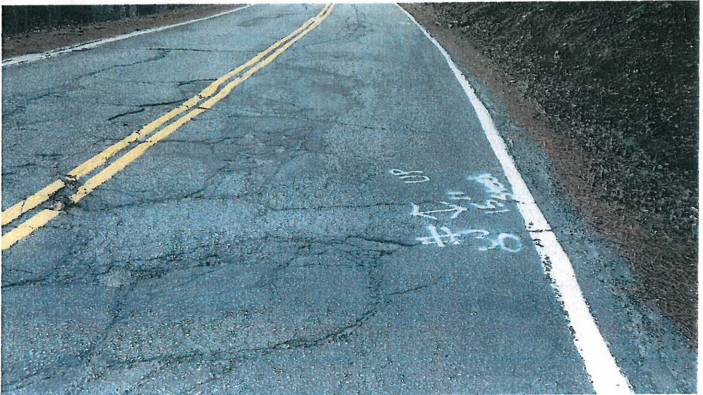
Pipe #30, 15" CMP, Pavement condition at crossing.
