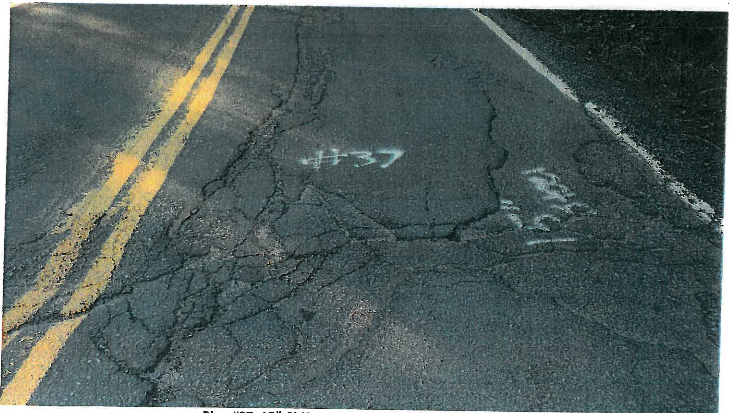
Pipe #37, 15" CMP, Pavement conditions at crossing.
