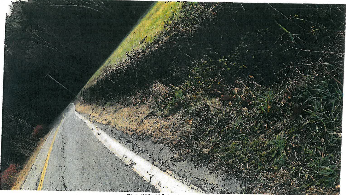
Pipe #10, 12" CMP, Inlet Ditch.
