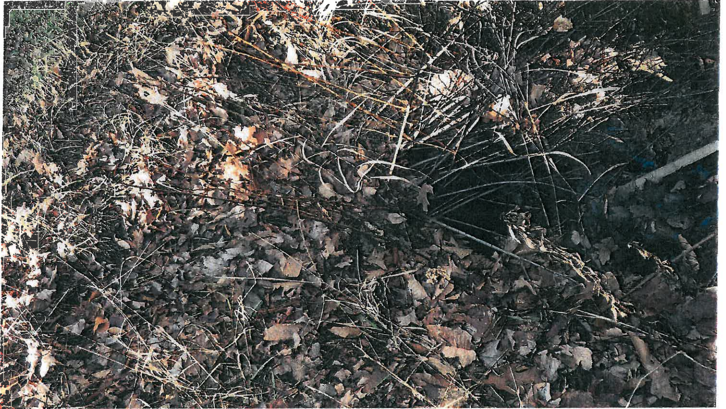
Pipe #27, 18" CMP, inlet.
