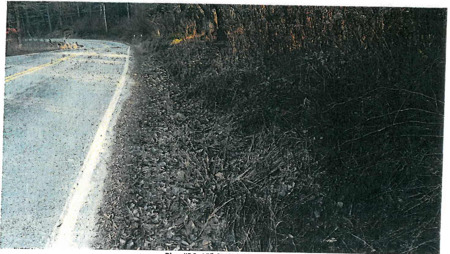
Pipe #36, 15" CMP, inlet ditch.
