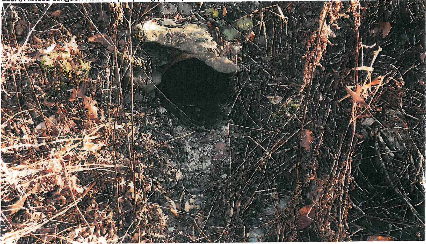
Pipe #32, 18" CMP, outlet.
