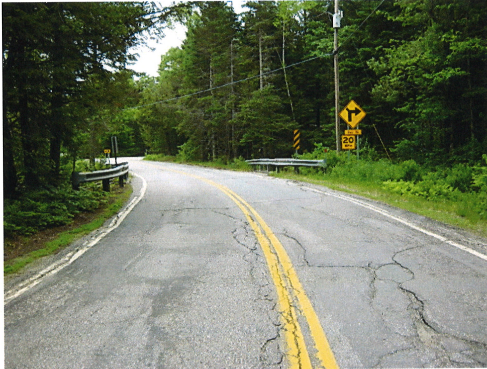
Figure 1: West approach. Rte. 123A over Honey Brook (7/2014).
