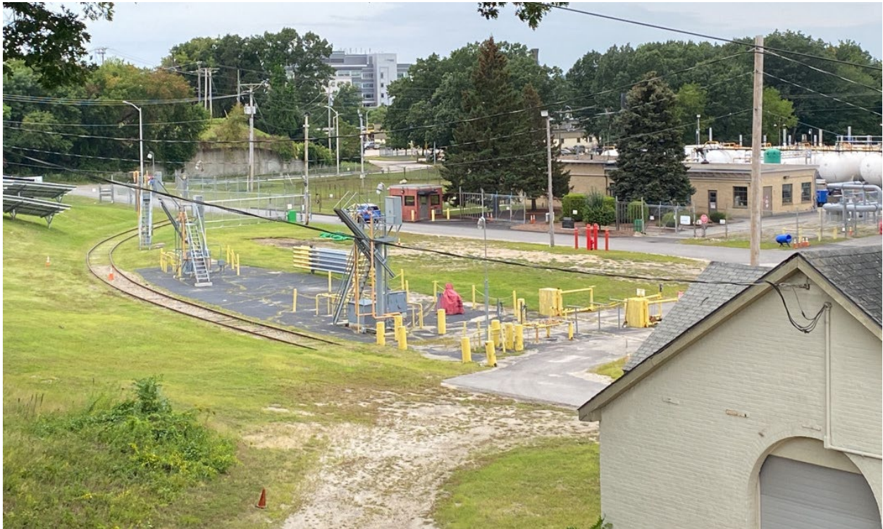
Photo 13. A view looking southwest from Elm Street in Manchester providing a view of the gas plant and former tracks on the Manchester Gas Light Co./Peoples Gas Light Co. Complex (CCP-008) property.
