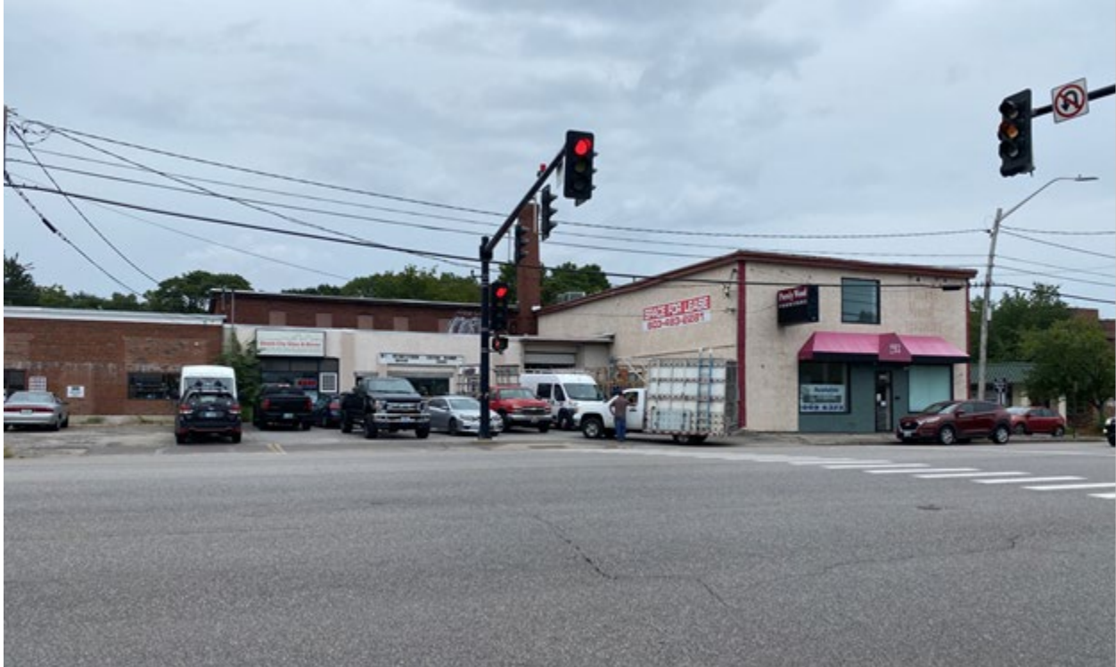
Photo 7. View looking east across Elm Street in Manchester at the façade of a pre-1947 building (CCP-004).
