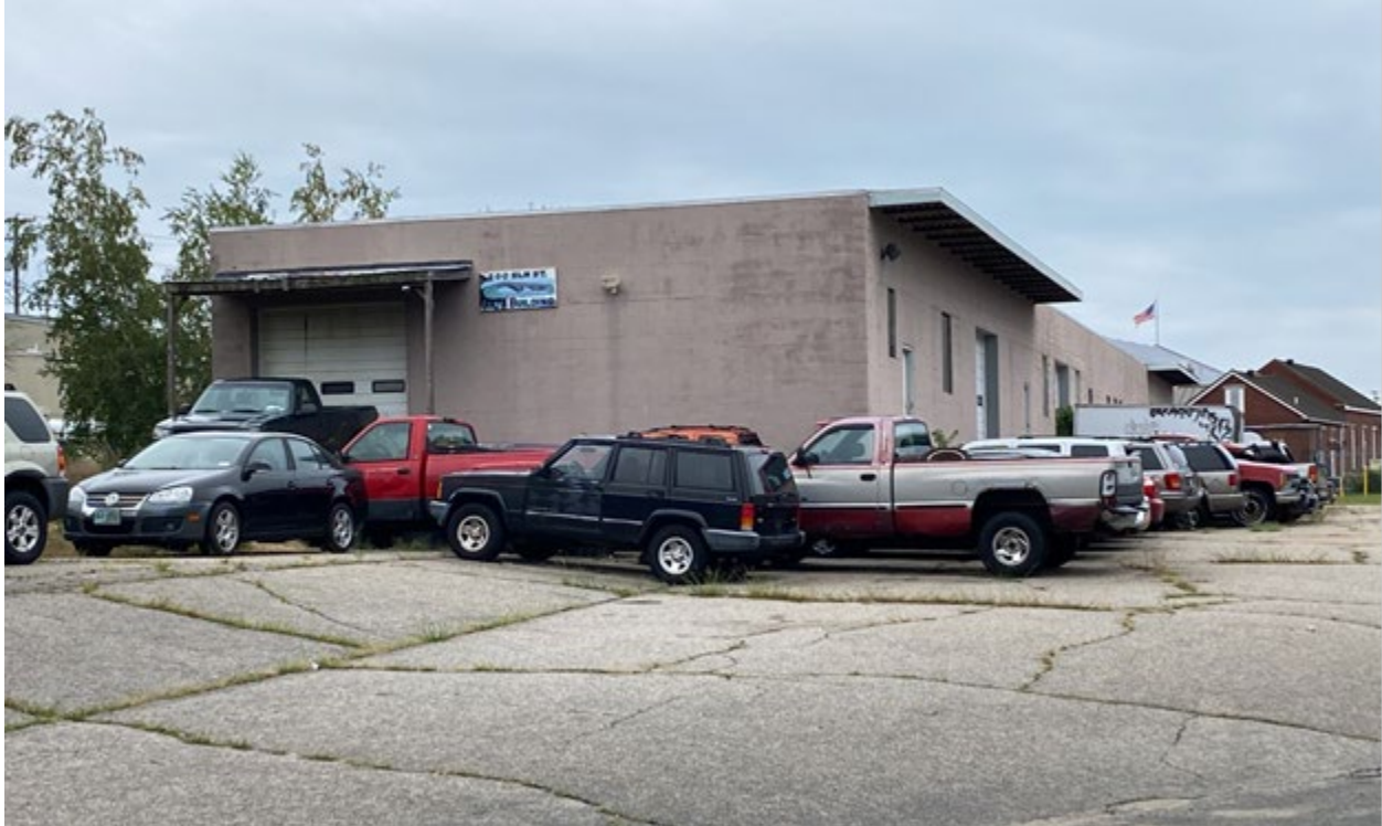
Photo 9. A view looking southeast at CCP-007, a building constructed ca. 1960.
