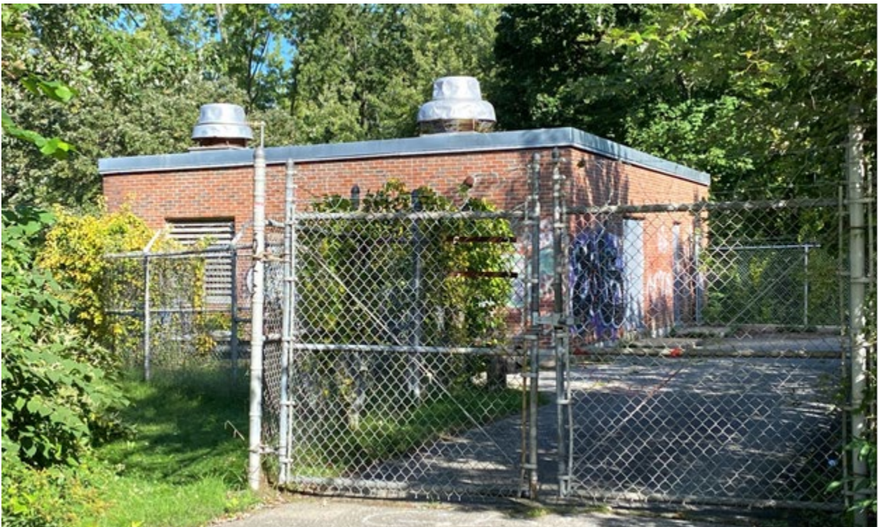
Photo 18. View looking northwest at a pumping station south of the Souhegan River in Merrimack part of the Merrimack Wastewater Treatment Facility historic district (MER0168).
