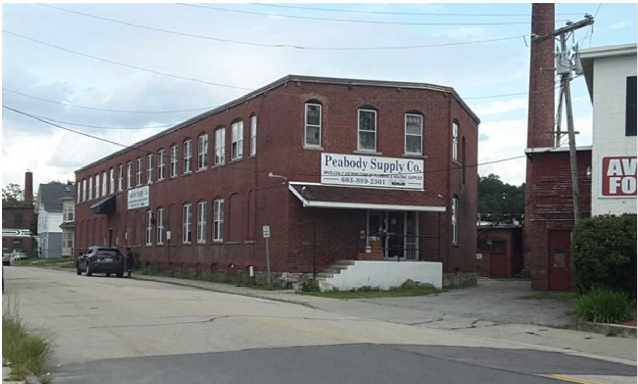
Photo 30. A view facing southeast along Crown Street opposite the intersection of Chase and Crown Streets in Nashua showing the façade and north side of the Peabody Supply Co. (CCP-018). This ca. 1900 building is located to the northeast of the proposed Crown Street station.
