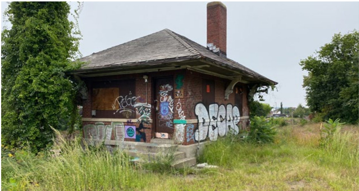
Photo 8. View of the ca. 1915 former Boston and Maine Switch Tower (CCP-005), looking northwest.
