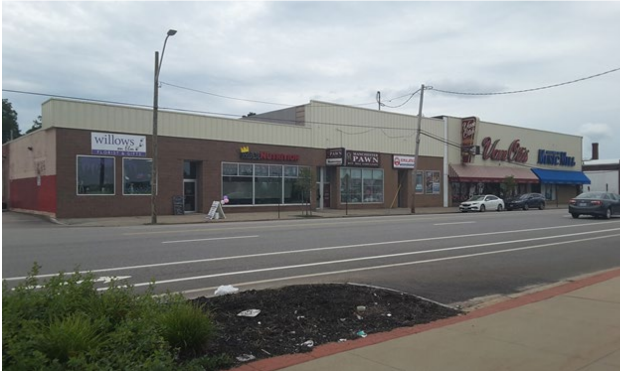
Photo 5. A view of the modified façade of a pre-1885 property in Manchester (CCP-002), looking southeast across Elm Street near its intersection with Green Street.
