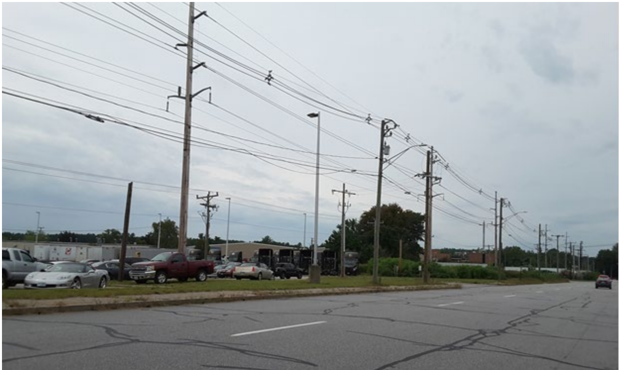
Photo 14. Street view looking southwest along Winston Street in the Goffe's Falls Area.
