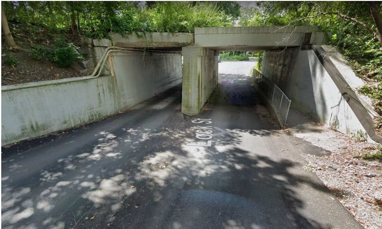
Photo 26. A supplementary Google Streetview image looking west along Lock Street, showing a close-up perspective of the BR#72 #39.39 (CCP-015) bridge/tunnel. The left side of the bridge appears to have replaced a cut stone precursor which is now visible behind the current concrete support wall.
