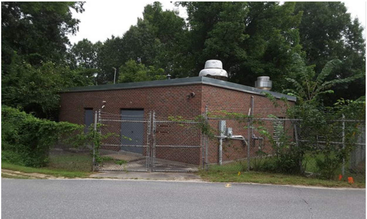
Photo 22. A view looking northeast across Griffin Street in Merrimack, NH, showing an oblique view of a pumping station that is part of the Merrimack Wastewater Treatment Facility historic district (MER0168).
