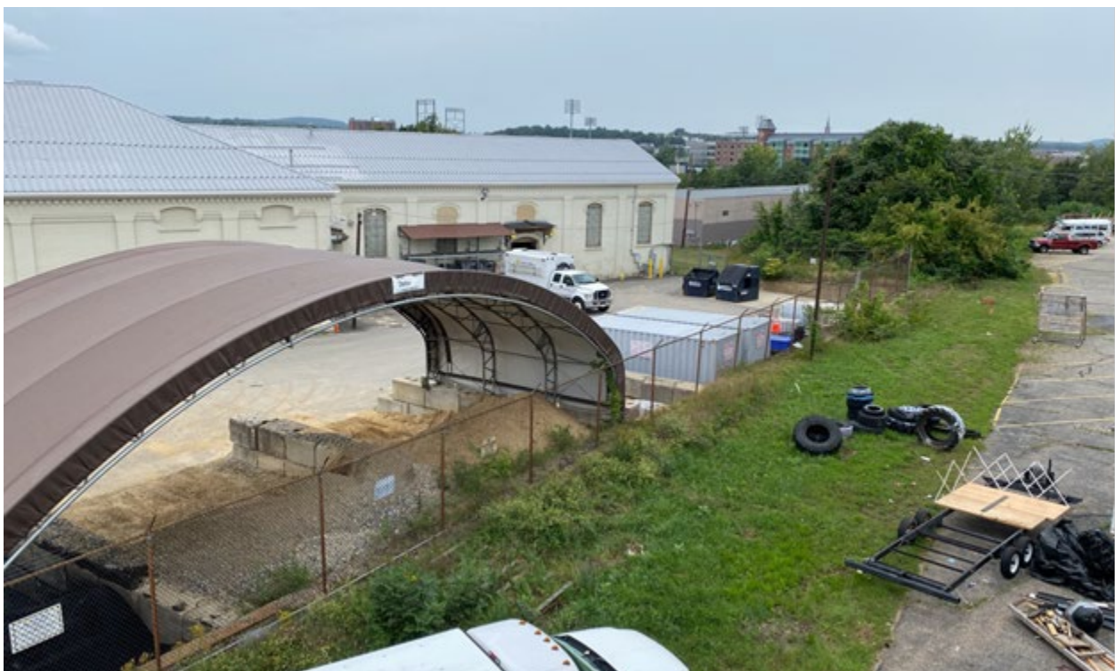
Photo 12. View looking northwest from Elm Street in Manchester at the east elevation of the former Manchester Gas Light Co./Peoples Gas Light Co. Complex (CCP-008). The grass strip is the former route of the Manchester & Lawrence Railroad corridor heading to the railyard.
