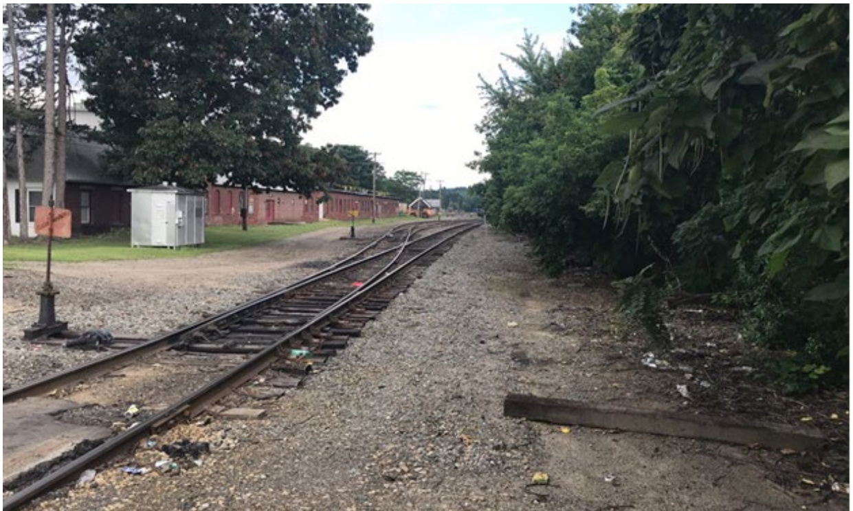
Photo 32. A view looking southeast from Crown Street in Nashua showing the western edge of the railroad ROW that is the proposed site of the Crown Street Station rail platform. This area is occupied by a broad area of ballast that currently features no rail infrastructure.
