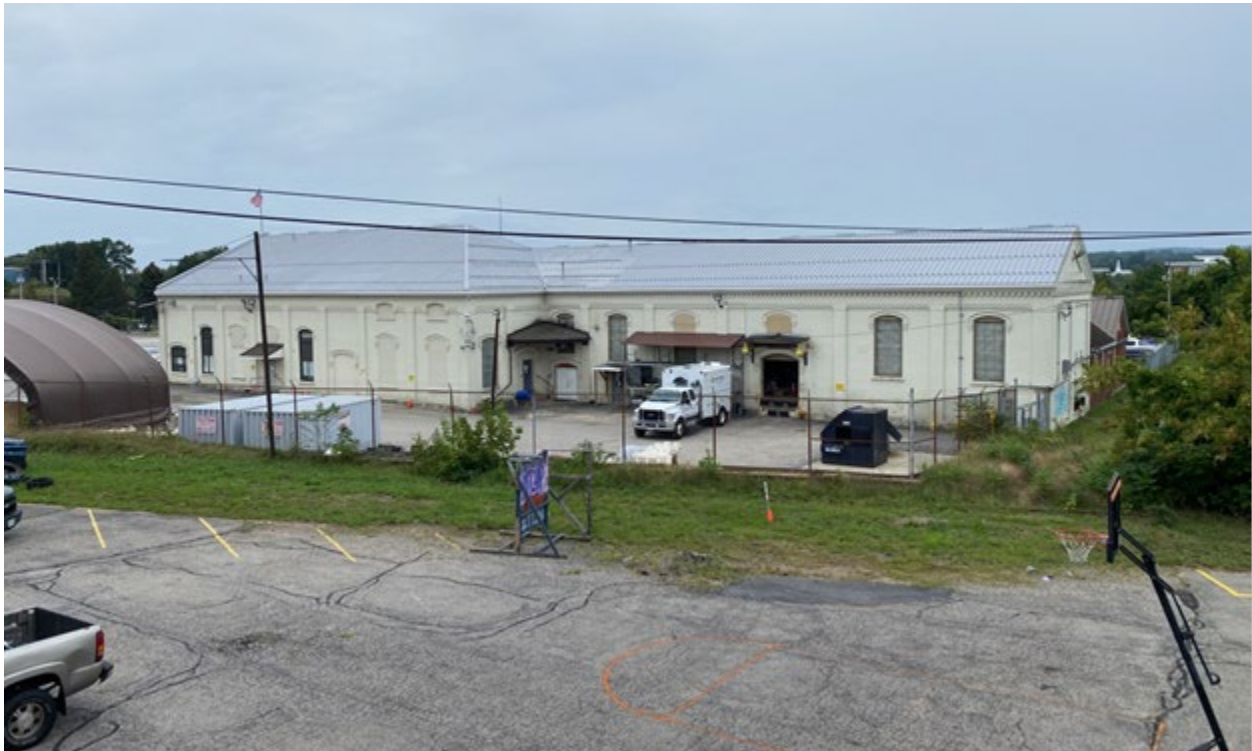
Photo 11. View from Elm Street in Manchester looking southwest at the eastern elevation of the pre-1885 former Manchester Gas Light Co./Peoples Gas Light Co. Complex (CCP-008).
