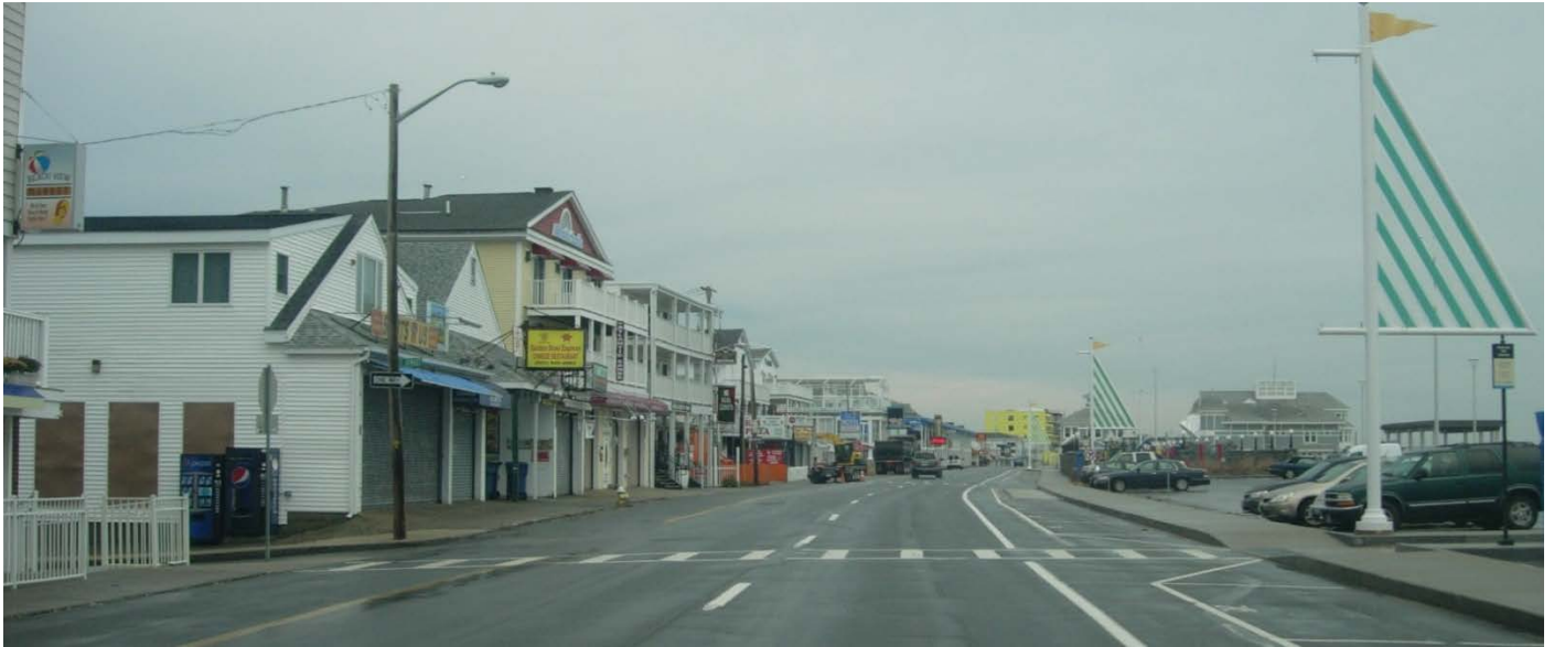
Lack of north-south crosswalks and pedestrian ramps with DWS along the west (left) side of Ocean Boulevard.
