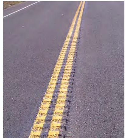
Photo 4.7 Typical Centerline Rumble Strip
