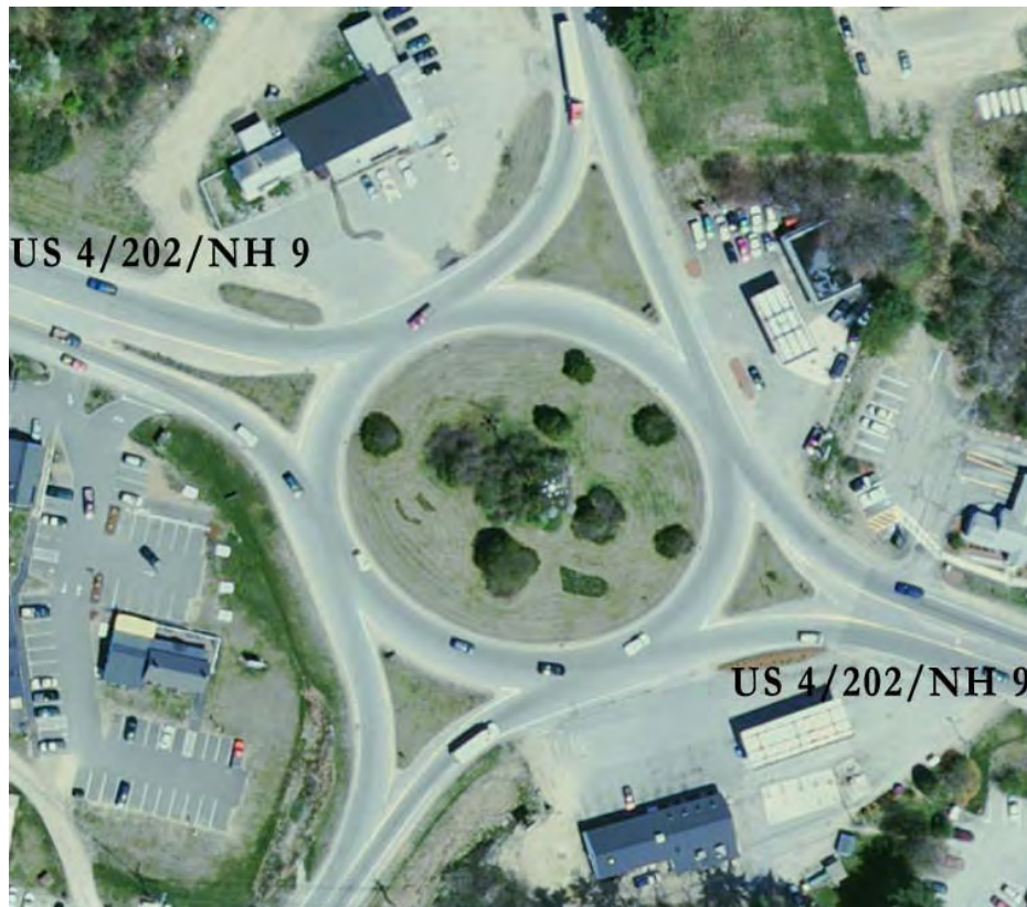
Photo 5.5.1 Aerial View of Epsom Circle
