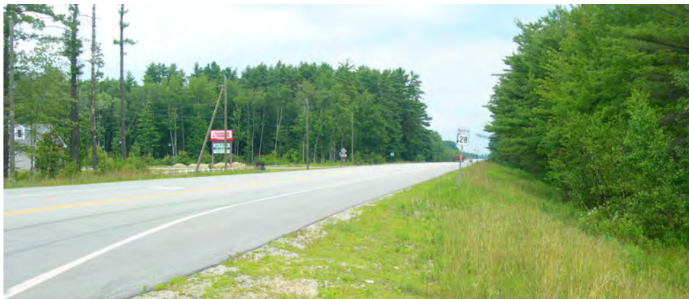
Photo 5.9.1 NH Route 28 North of Concord Hill Road
