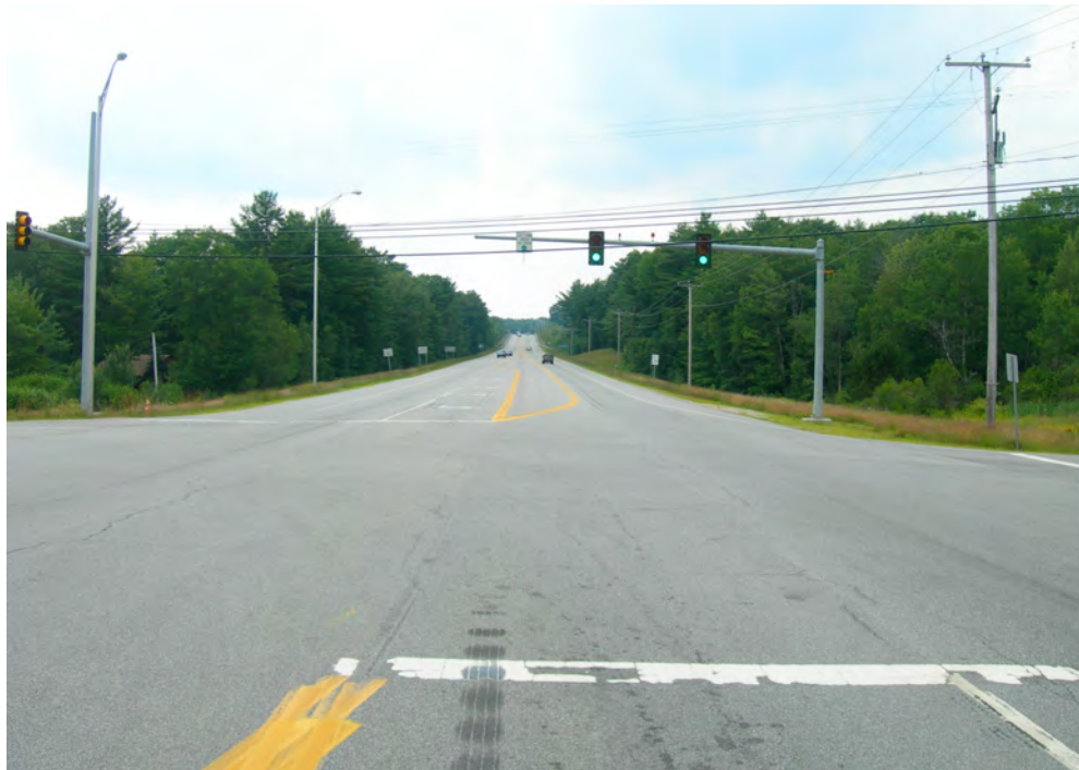
Photo 5.7.1 NH Route 28 Opposing Left Turn Lanes at NH Route 107
