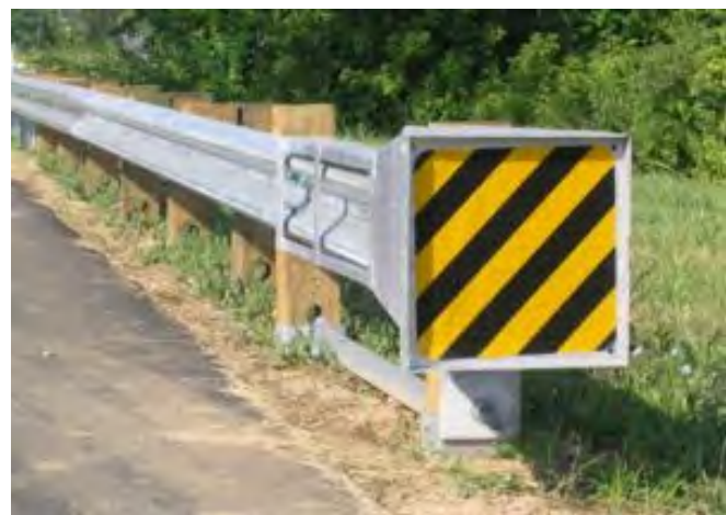
Photo 4.6 Guardrail End Treatment
