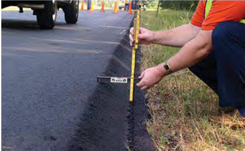
Photo 4.2 Safety Edge Treatment
