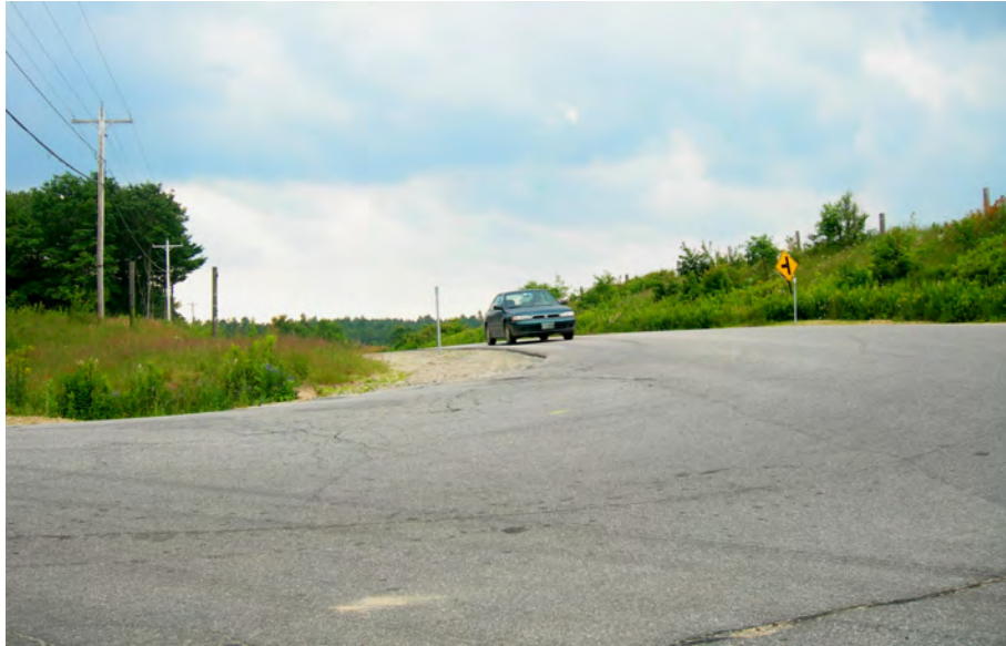
Photo 5.2.2 North Barnstead Road Driver's View at NH Route 28
