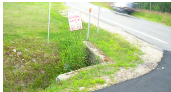
Photo 4.3 Stockbridge Corner Road Culvert Headwall in Clear Zone
