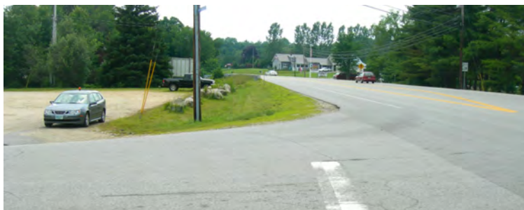
Photo 5.9.2 Curvature of NH Route 28 South of Concord Hill Road
