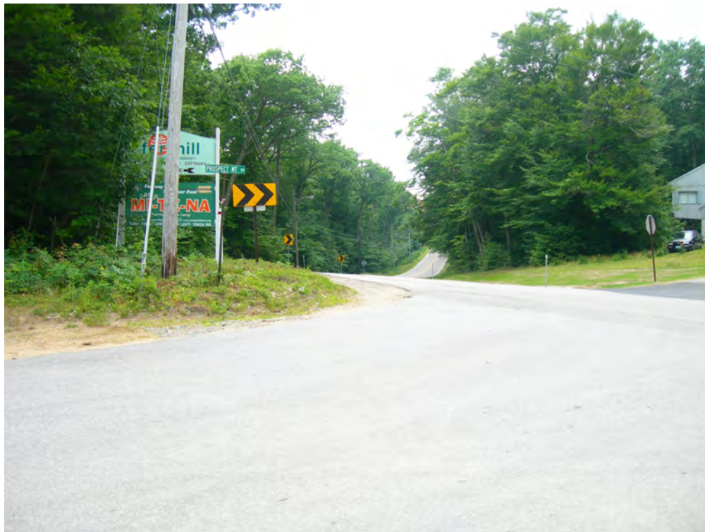
Photo 5.6.1 NH Route 28 Horizontal and Vertical Curvature
