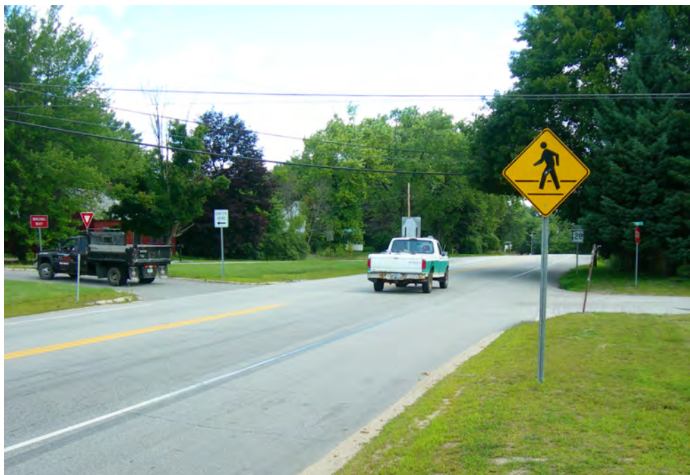
Photo 5.4.6 Improper Use of Crosswalk Sign on NH Route 28
