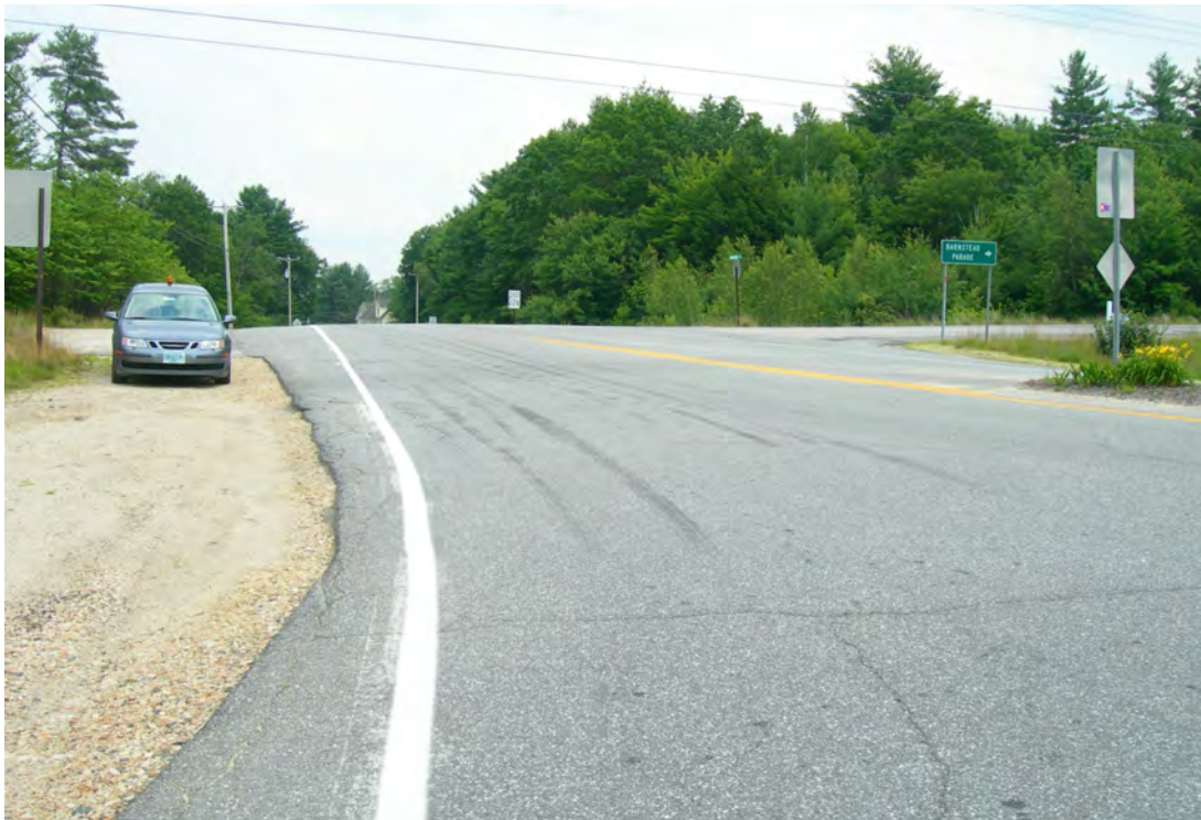
Photo 5.8.4 Crest of Rise on NH Route 126 East of NH Route 28
