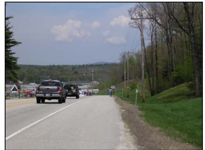
Photo 2: This photograph shows US Route 3 as it enters Allenstown’s commercial district from Hooksett. The presence of a pedestrian walking in the shoulder demonstrates the need of sidewalks at this particular portion of the corridor.
