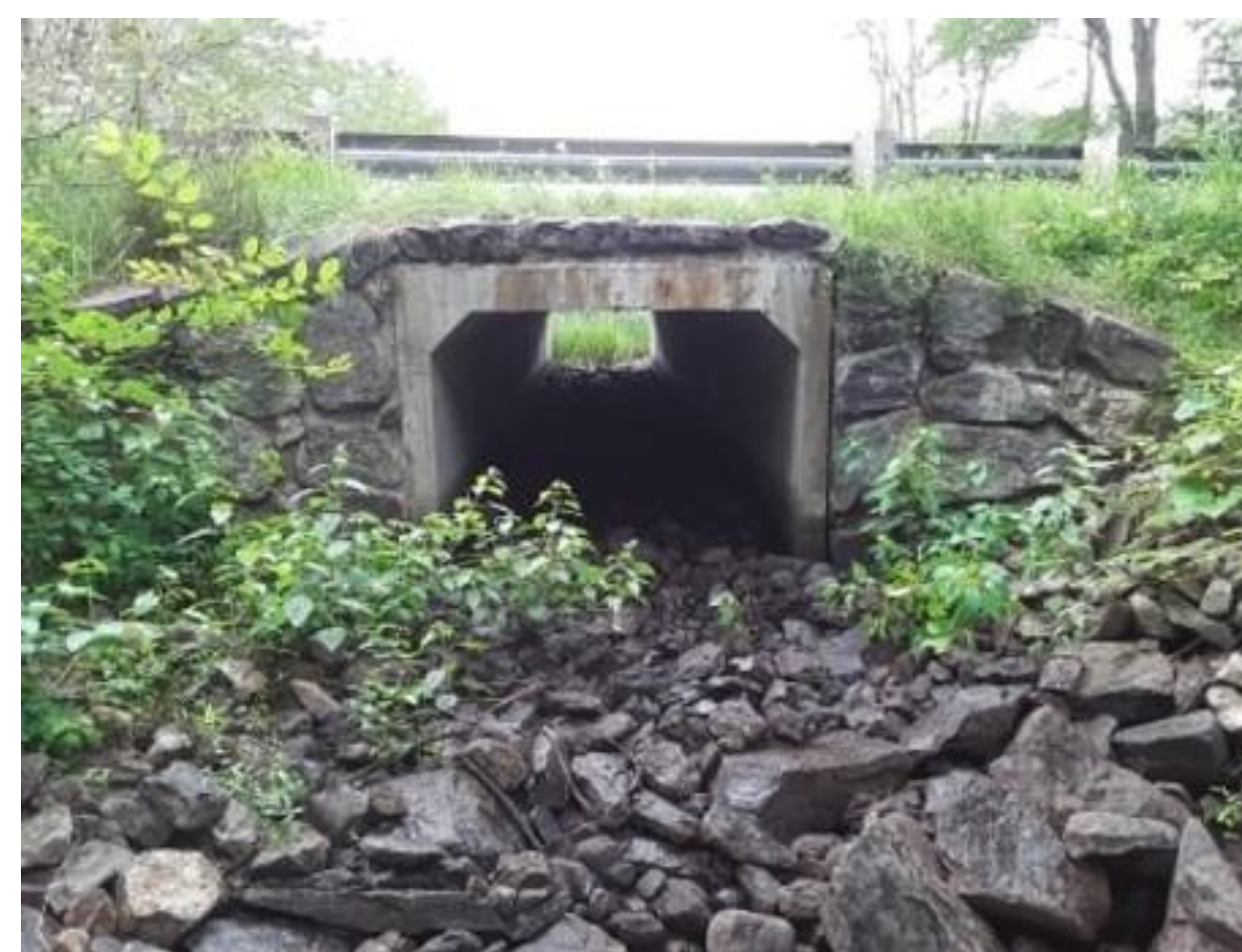
Culvert outlet in hyporheic condition, located in southern NH
