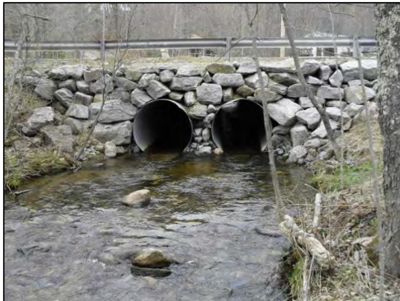
Photo 4: View downstream of culverts, view is north.
