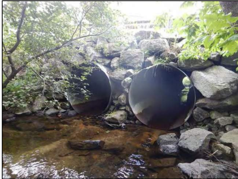
Photo 5: View downstream of culverts, view is north.
