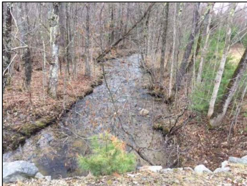
Photo 6: View downstream of culverts, riparian zone, view is south.
