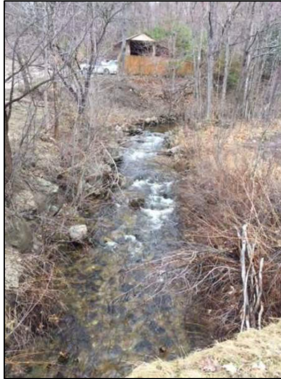
Photo 3: View Upstream of culverts, riparian zone, view is north.
