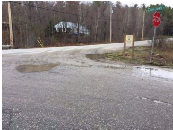
Roadway above culvert
