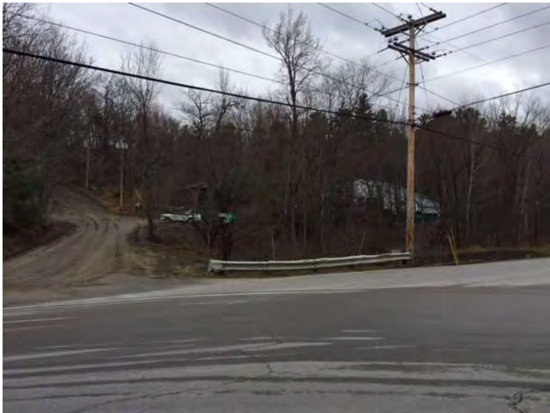
Roadway View – Looking North up Stryker Road
