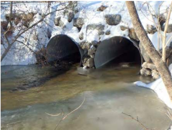
View looking at downstream invert
