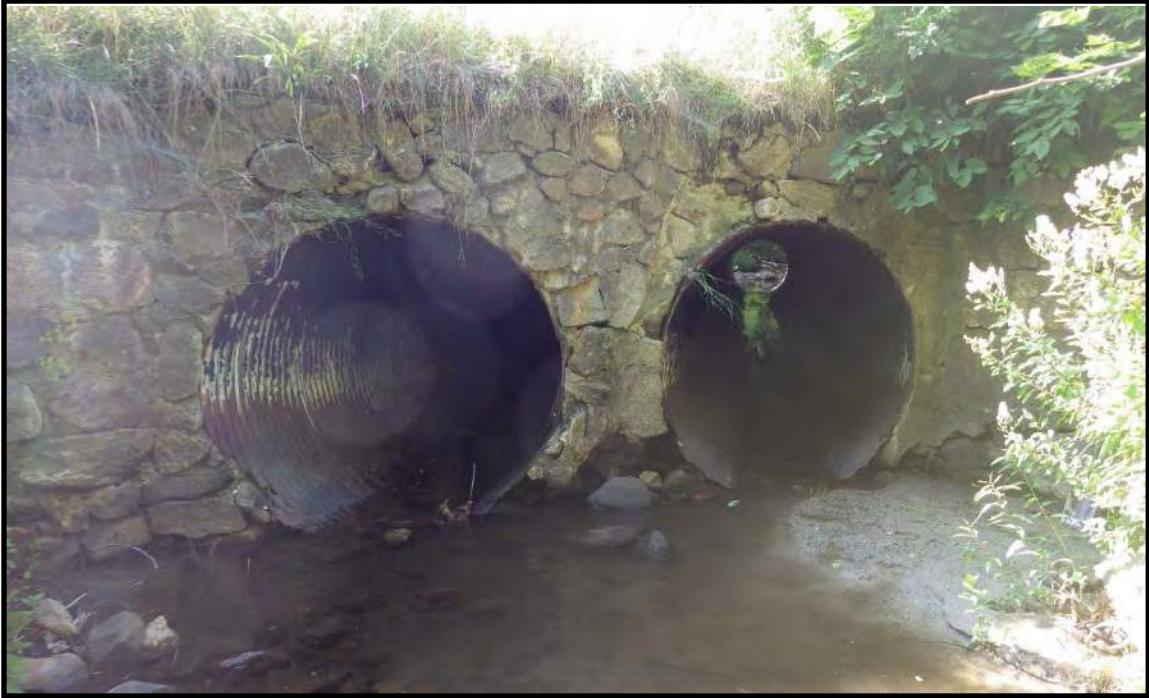
Photo 3: Inlet looking downstream
