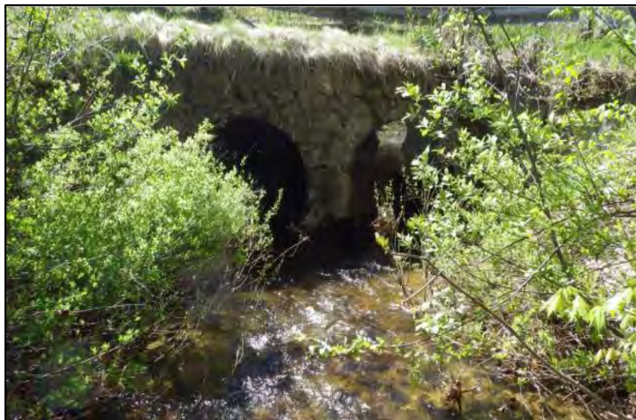
Photo 2: Upstream culvert photo, wetland riparian zone, view is south.
