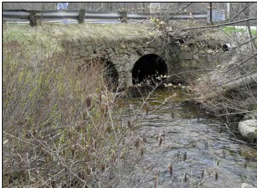
Photo 1: Upstream photo from culvert location, view is south.
