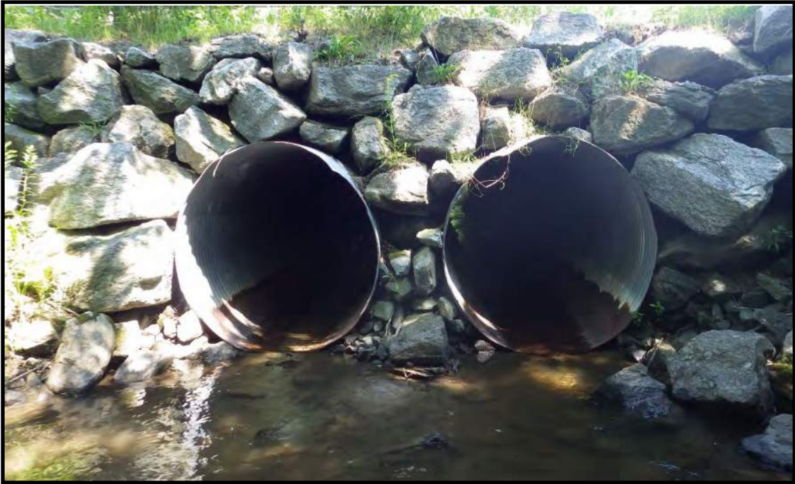
Photo 1: Outlet looking upstream
