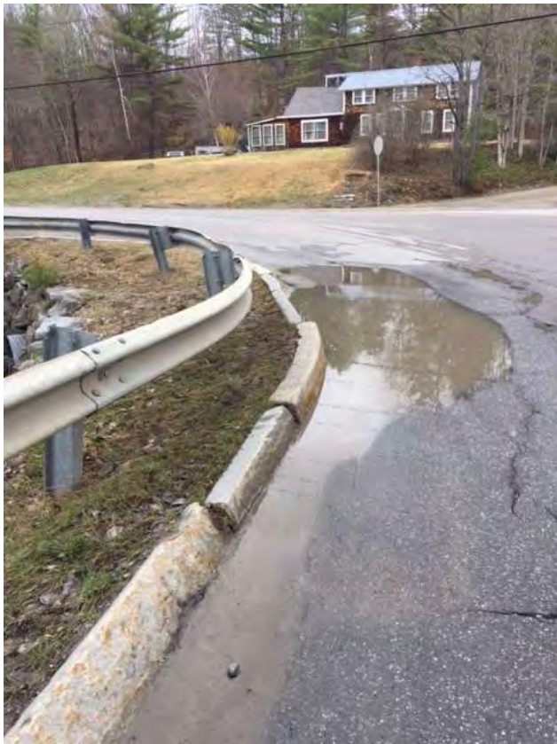
Roadway View (Looking West)
