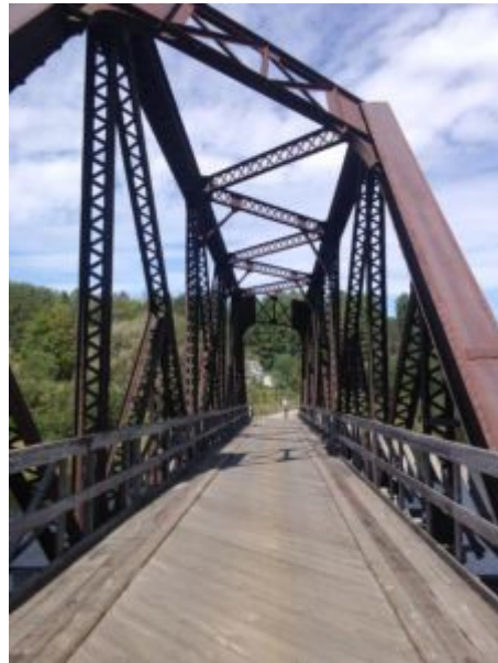
Upper Coos Recreational Rail Trail
