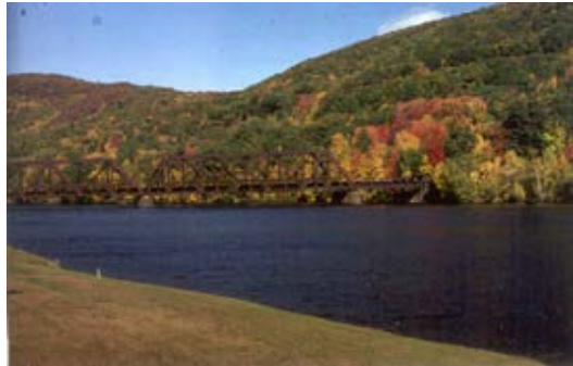
Rail bridge over Connecticut River
