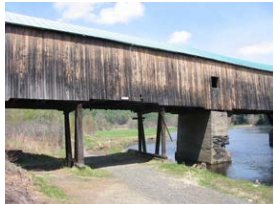
Rail trail under covered road bridge in Bath
