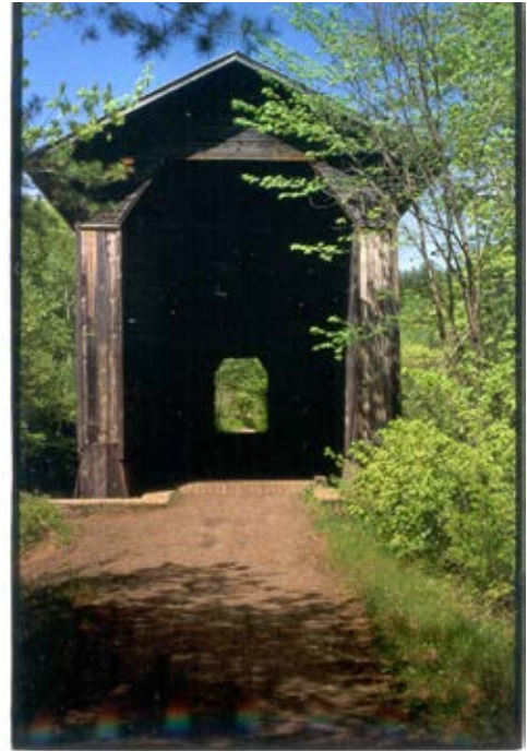
Kellyville Covered Rail Bridge over Sugar River
