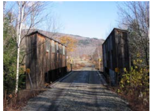
Boxed Pony Truss Bridge on Rail Trail
