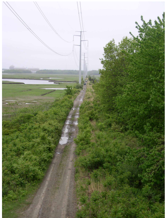
Hampton Branch corridor through wetlands as seen from Route 1
