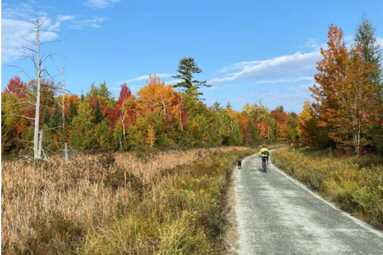
PRESIDENTIAL RAIL TRAIL, PONDICHERRY SECTION
