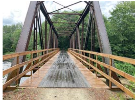
Sugar River Truss Bridge
