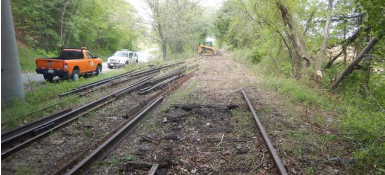
Rails and ties being removed on the Northern Rail Trail in Boscawen.
