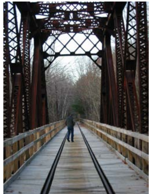
Railroad Bridge on Conway Branch
