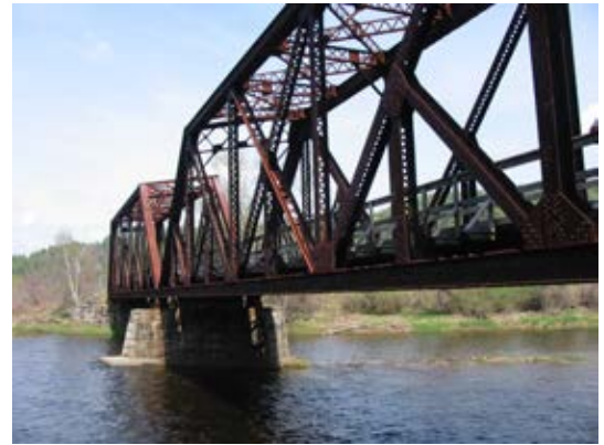
Rail bridge over Ammonoosuc River in Lisbon
