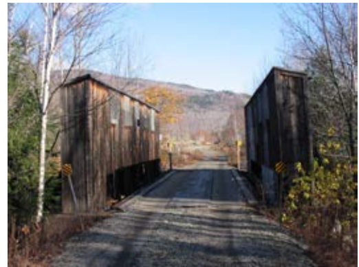
Boxed Pony Truss Bridge on Rail Trail
