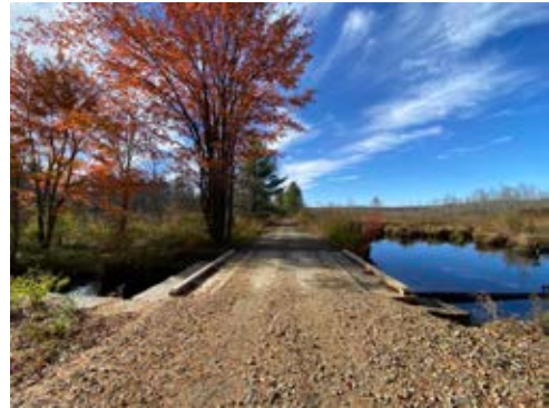
Fitzwilliam Bridge Cheshire Rail Trail
