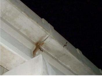
Photo 7: Staining along longitudinal joint. Guano deposits on the ground.
