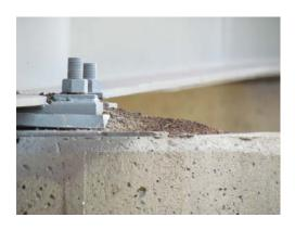
Photo 5: Guano deposit on pier, obscuring structural Photo 6: Bat Guano on Riprap features.
