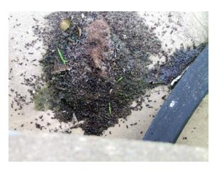
Photo 4: Guano deposits visible from bridge deck, on top
