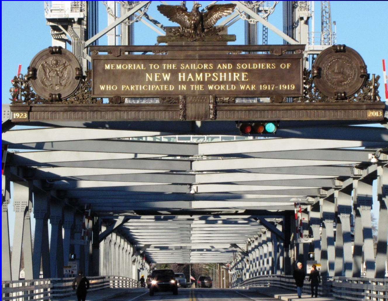
The Memorial Bridge / QAW Atlantic City NJ / 2.5.2014 / Jerry Zoller, NHDOT #158
