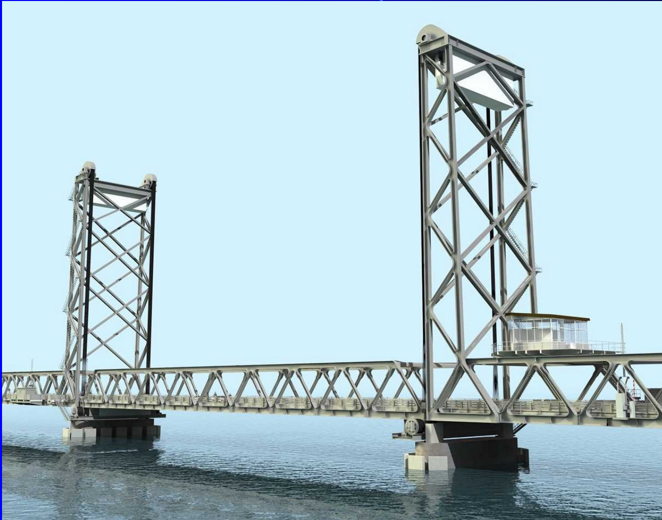
The Memorial Bridge / QAW Atlantic City NJ / 2.5.2014 / Jerry Zoller, NHDOT #46
