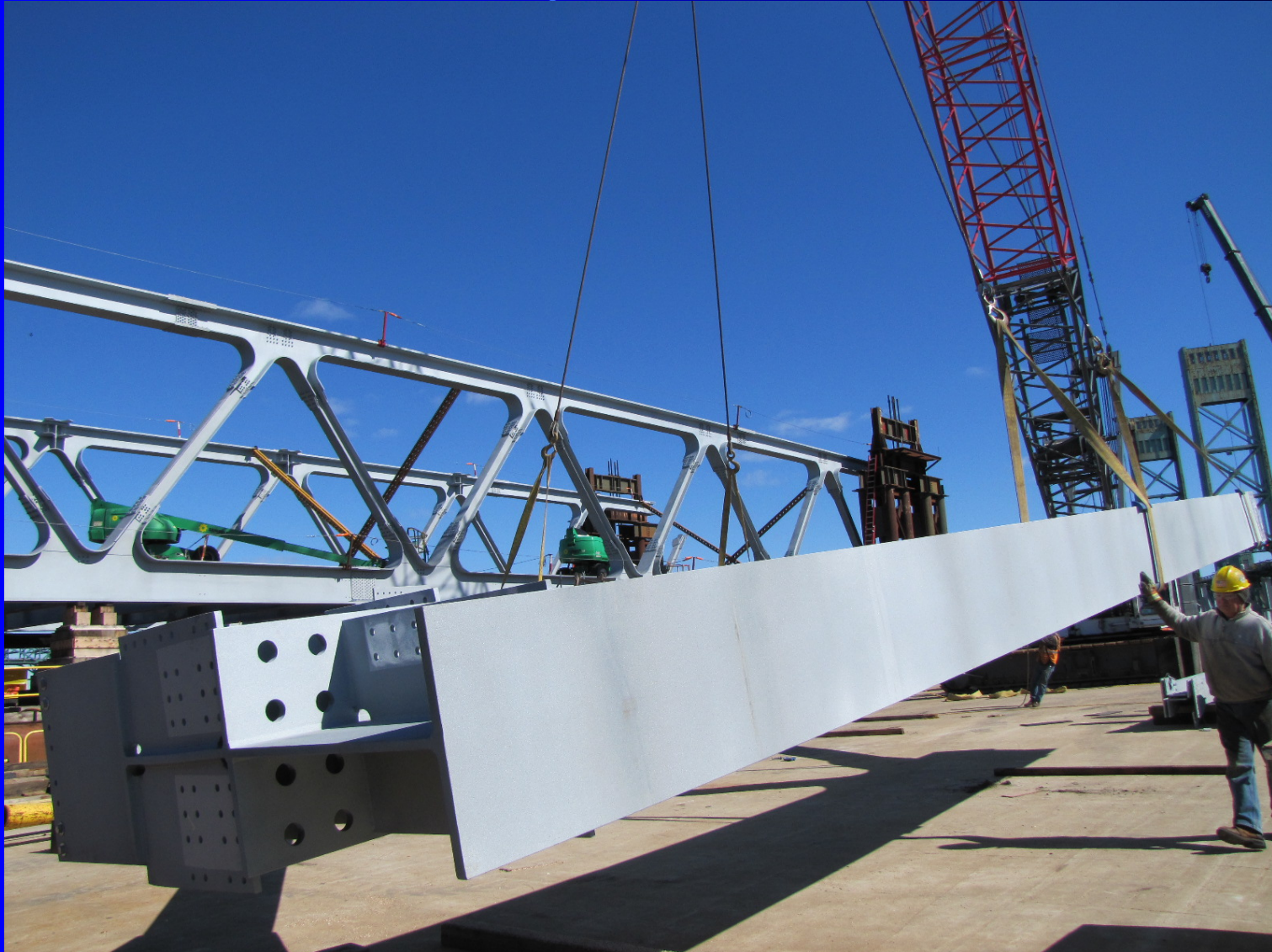
The Memorial Bridge / QAW Atlantic City NJ / 2.5.2014 / Jerry Zoller, NHDOT #118
