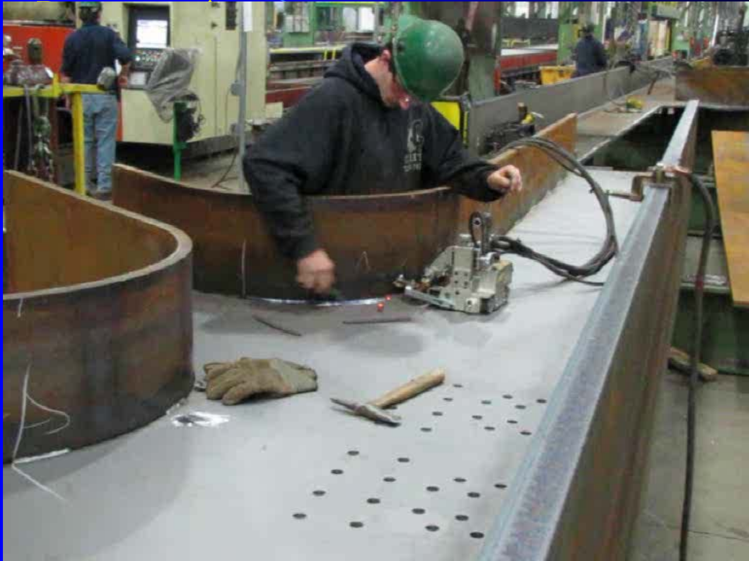
The Memorial Bridge / QAW Atlantic City NJ / 2.5.2014 / Jerry Zoller, NHDOT #67
