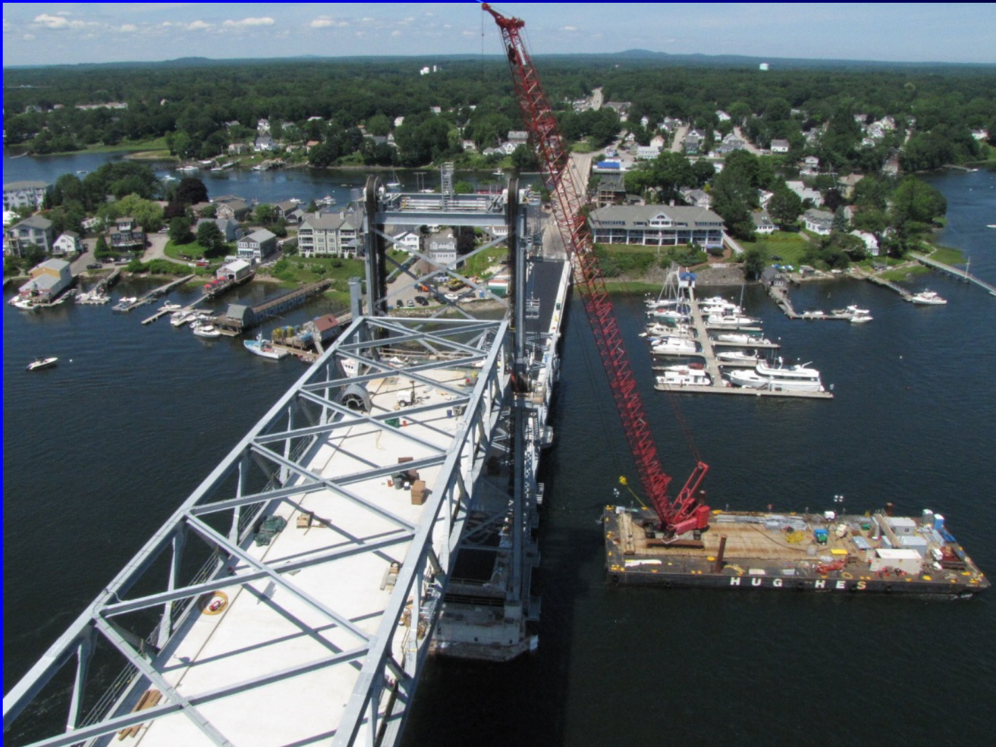
The Memorial Bridge / QAW Atlantic City NJ / 2.5.2014 / Jerry Zoller, NHDOT #157
