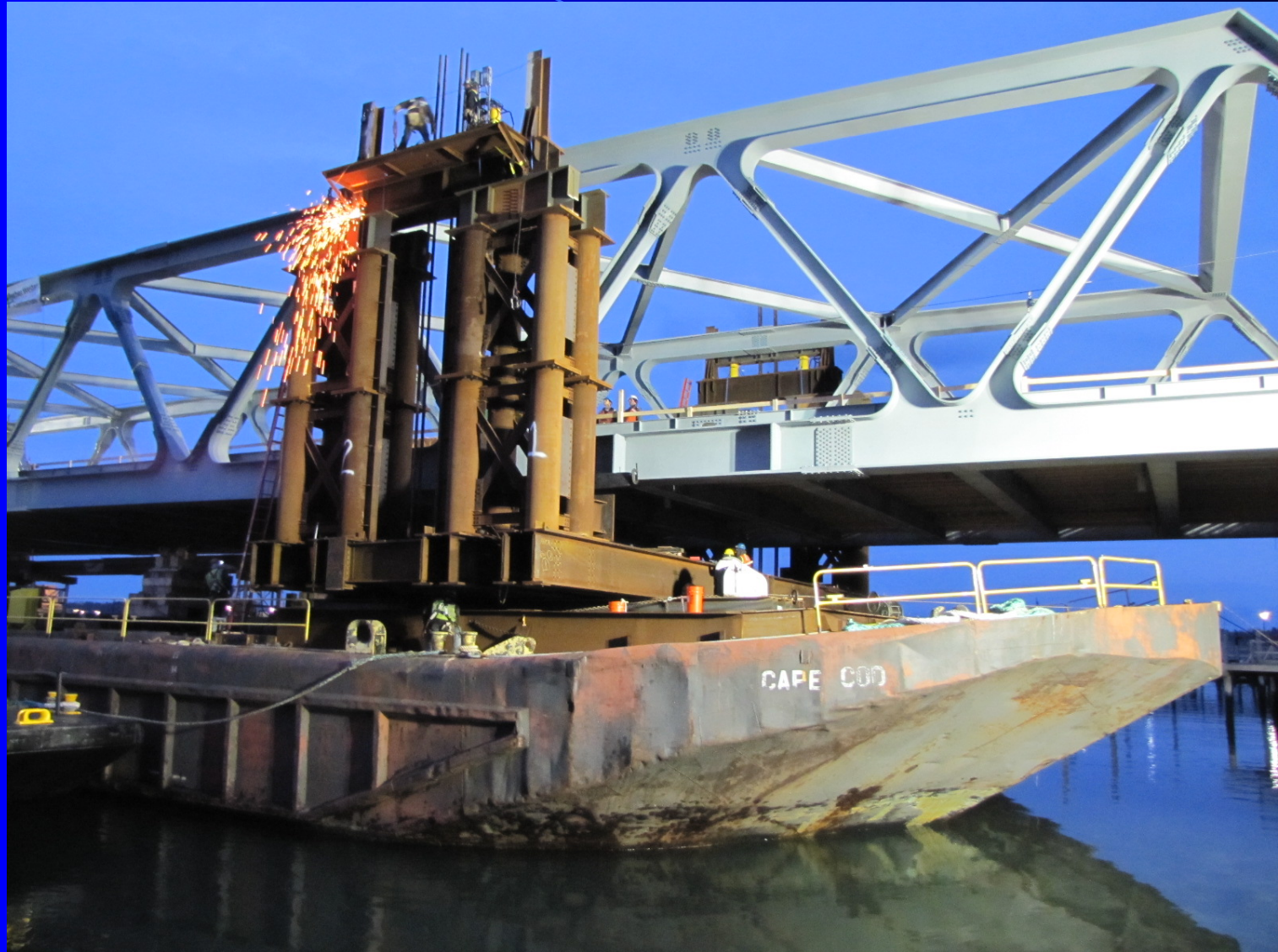
The Memorial Bridge / QAW Atlantic City NJ / 2.5.2014 / Jerry Zoller, NHDOT #128
