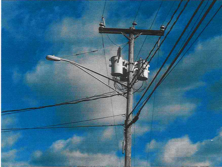
Wooden Pole with 12 Ft. Davit (12-35) – Full Cutoff (NH 4 Chicester)
