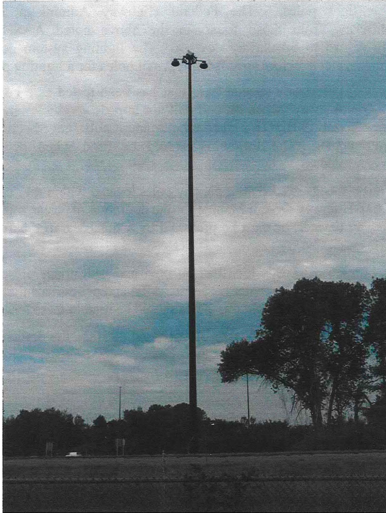
Typical High Mast Towers 3-100 ( vicinity I-93 @ I-393 Concord)
