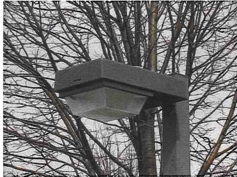
Rest Area Luminaires (Shoebox with Drop Lens)
