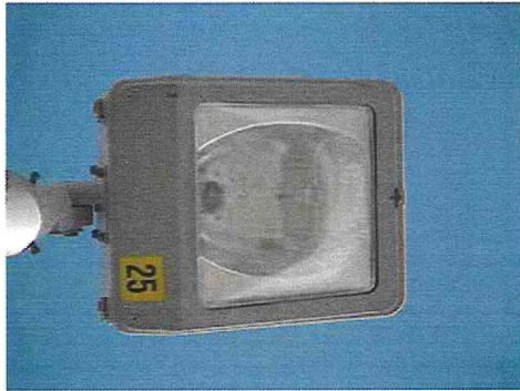
Vertical Mount Style Luminaires
