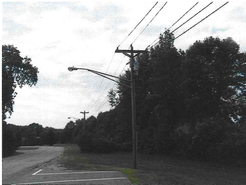
Wooden Pole with 12 Ft. Davit (12-35) – Full Cutoff (NH 4 Chicester)
