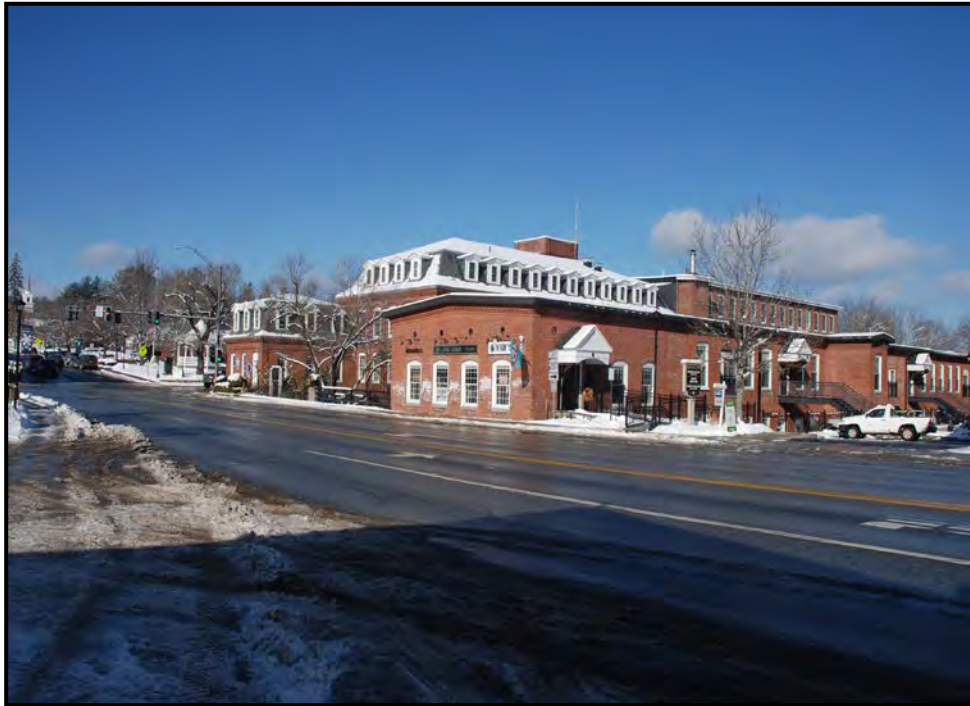
Photo 8: View north from Main Street of Jaffrey Mills, located at the northeast corner of the intersection of Main Street and North Street. 01/19/2018.
