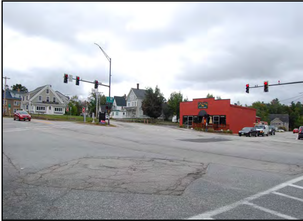
Photo 1: View south of the existing signal-controlled five-way intersection where a five-way roundabout is proposed. View toward Blake Street (right), Stratton Road (center), and NH 124 (left). The Lab N' Lager restaurant located at 4 Stratton Road (center, red building) is proposed to be removed to make room for the roundabout. 09/20/2018.
