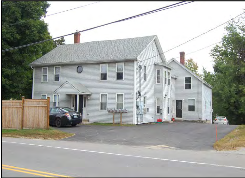
Photo 15: View of apartment building located at 15 River Street, proposed to be removed to make room for the new three-way intersection. 09/20/2018.
