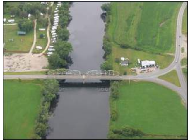
Figure 1 - Aerial View of the Bridge Carrying US Route 2 over the Connecticut River (Looking Downstream / South)
