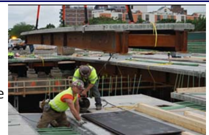
Massachusetts' example of a different method of rapid bridge construction.
