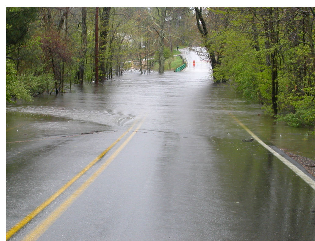
Flooding on the Isinglass River in May 2006
